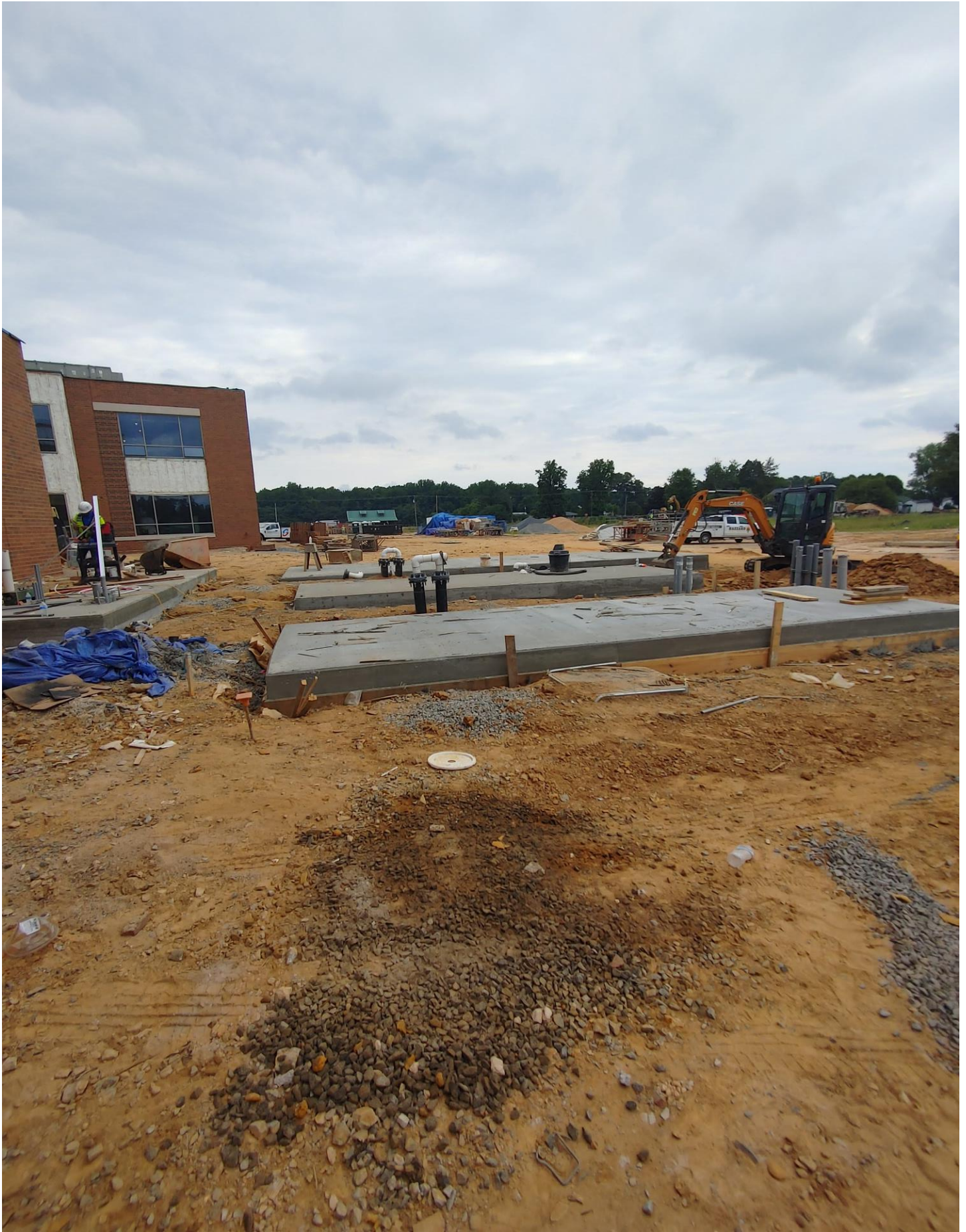
Photo 2 - Generator, Fuel Tank and Chiller Pads have been completed.
