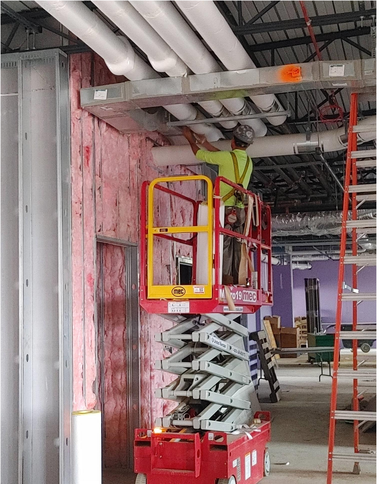
Photo 9 - Pipe is being insulated in Area B.
