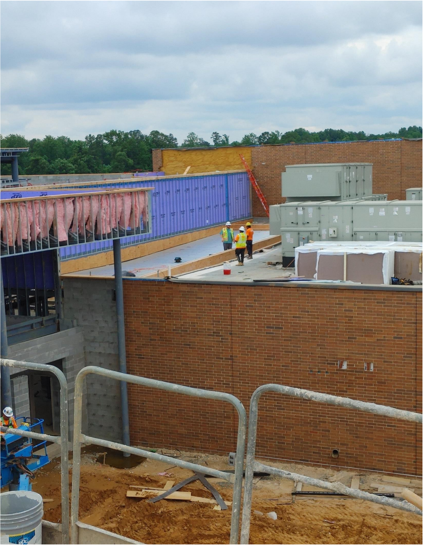
Photo 6 - Roofers are working on Parapet walls in Area E.
