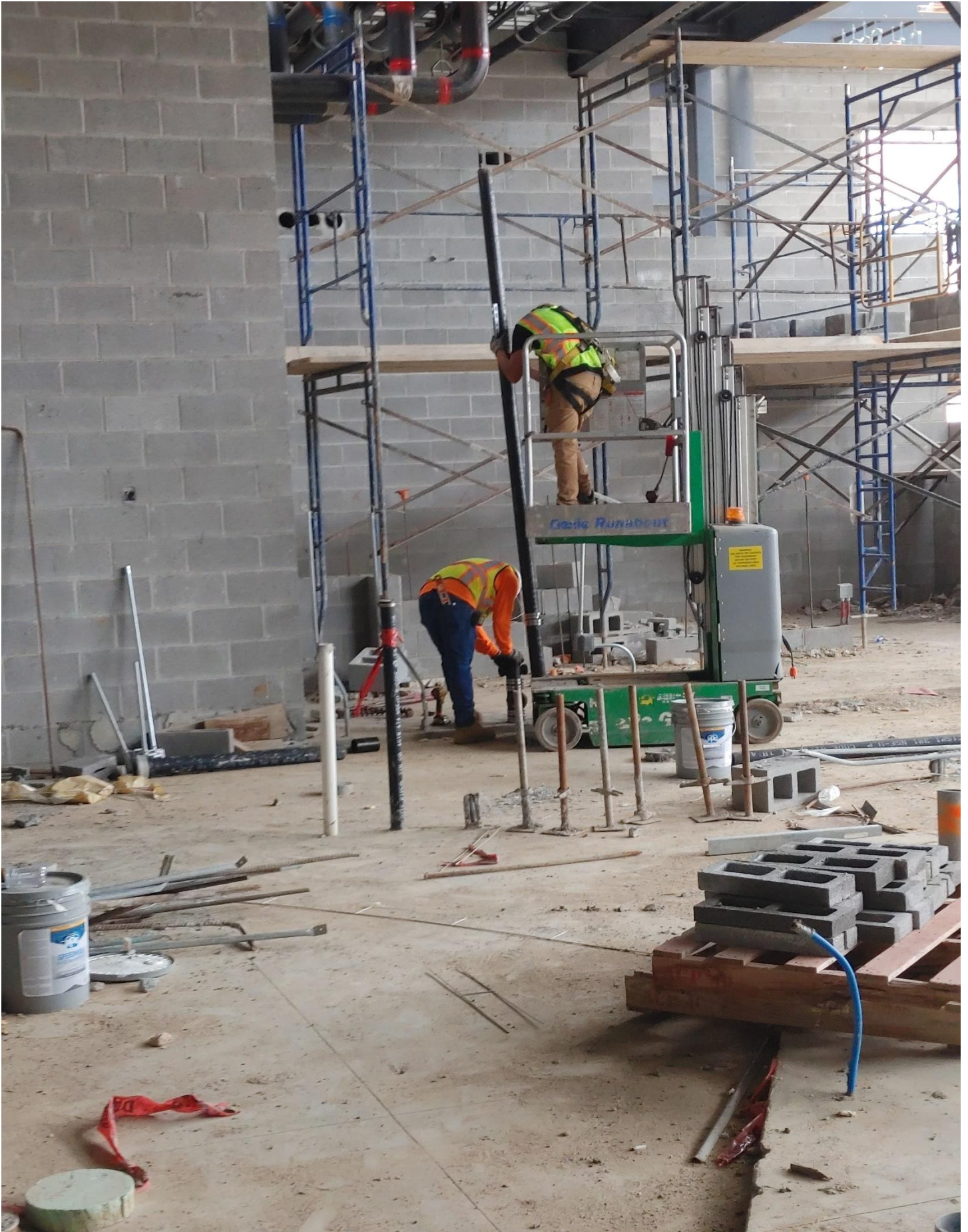
Photo 10 - Pipe being installed in Area C.
