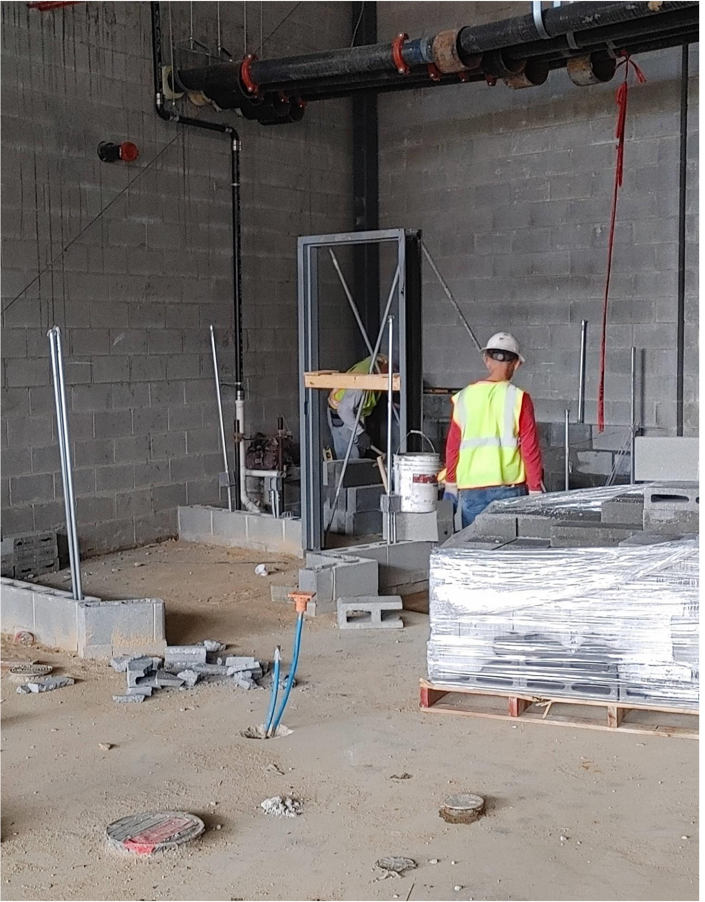
Photo 11 - Masons are laying block in Room C104B.
