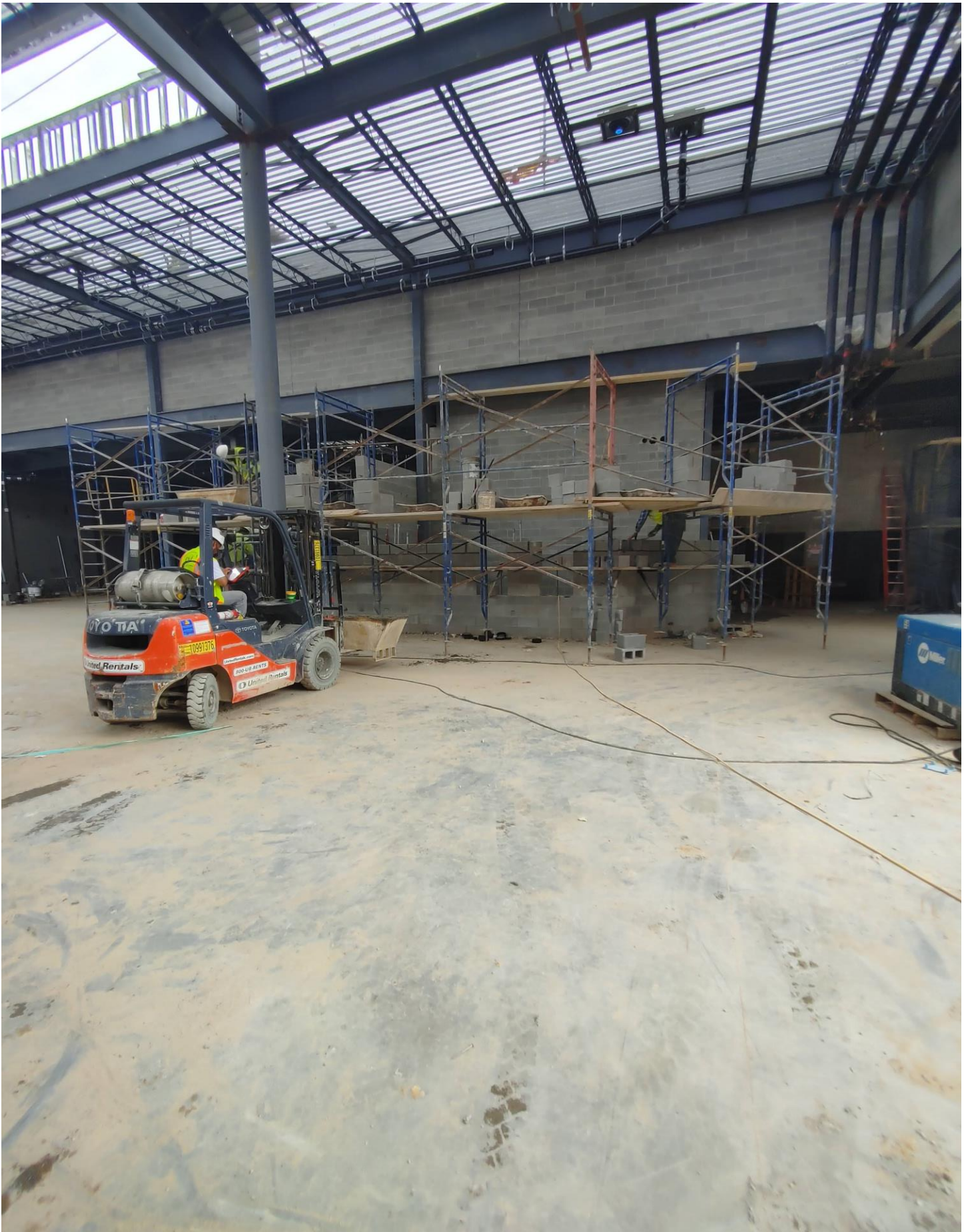
Photo 4 - Block is being laid in Area D.
