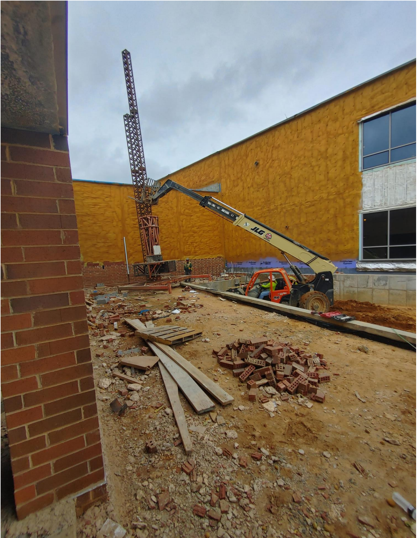
Photo 12 - Fraco Scaffolding being erected on the East side of Area C.
