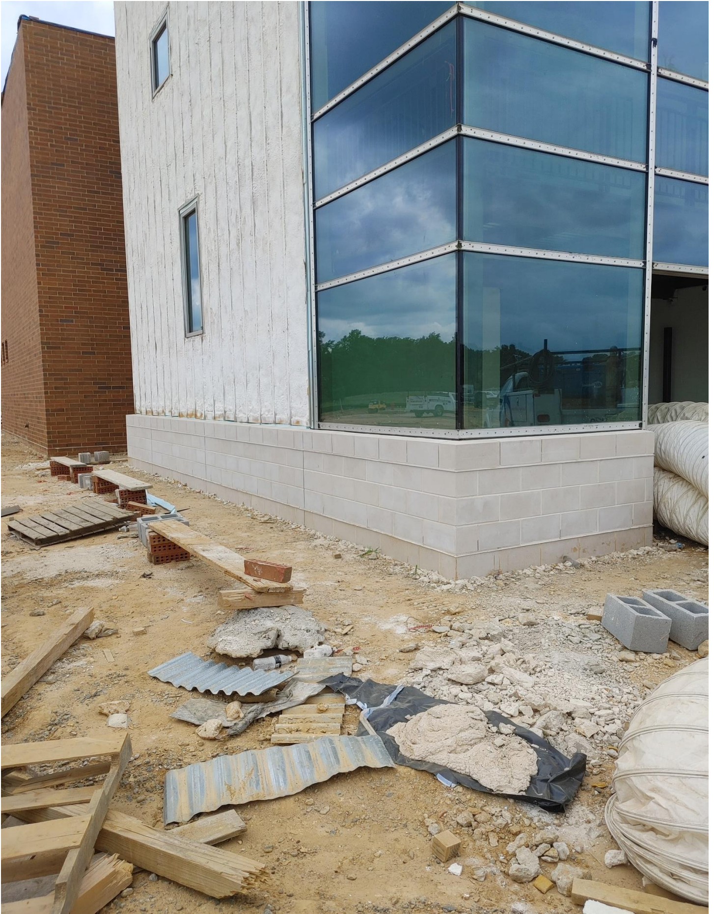
Photo 1 - Pre-cast has been completed at Stairwells #1 & #2
