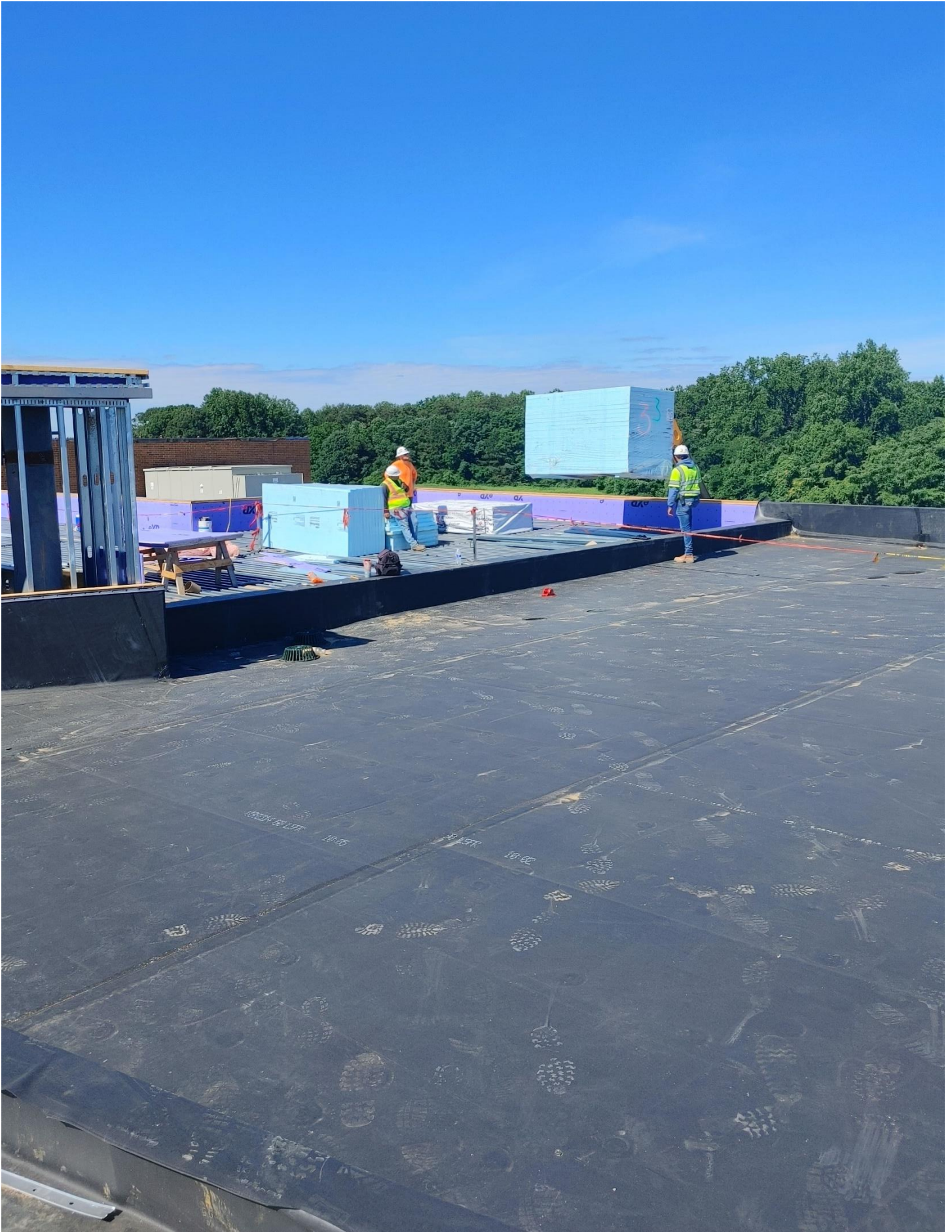
Photo 3 - Roofers are working on the Roof of Area C.
