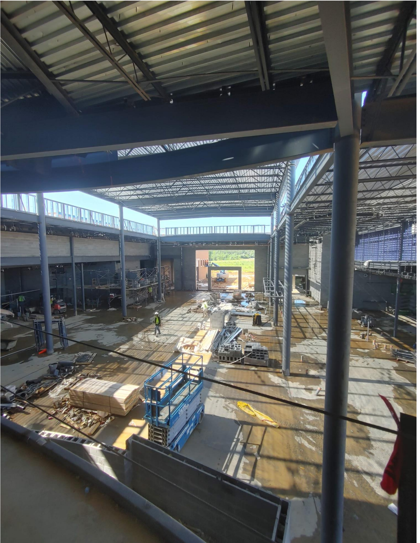
Photo 2 - View from the 2nd floor of Area A into Area C
