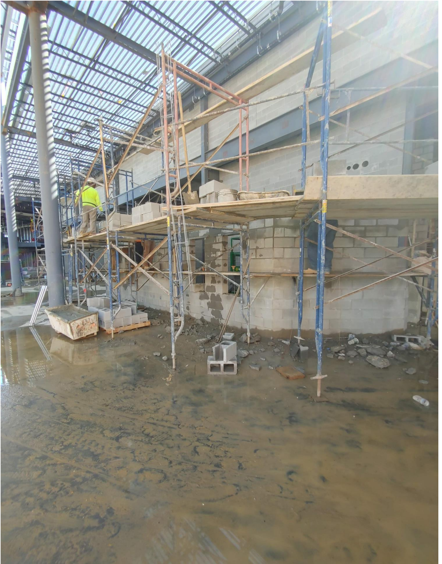
Photo 6 - Block is being laid in Area D, D117.
