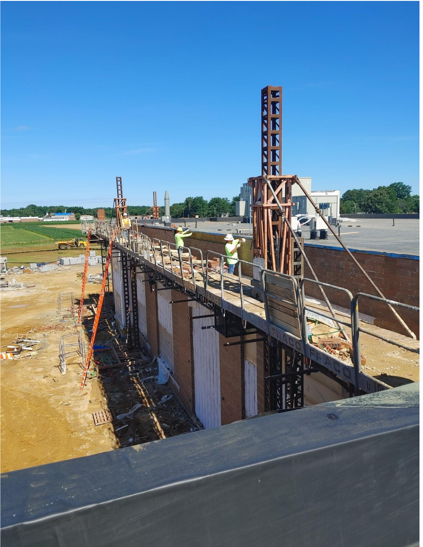
Photo 4 - Mason are laying Brick on the South side of Area B.
