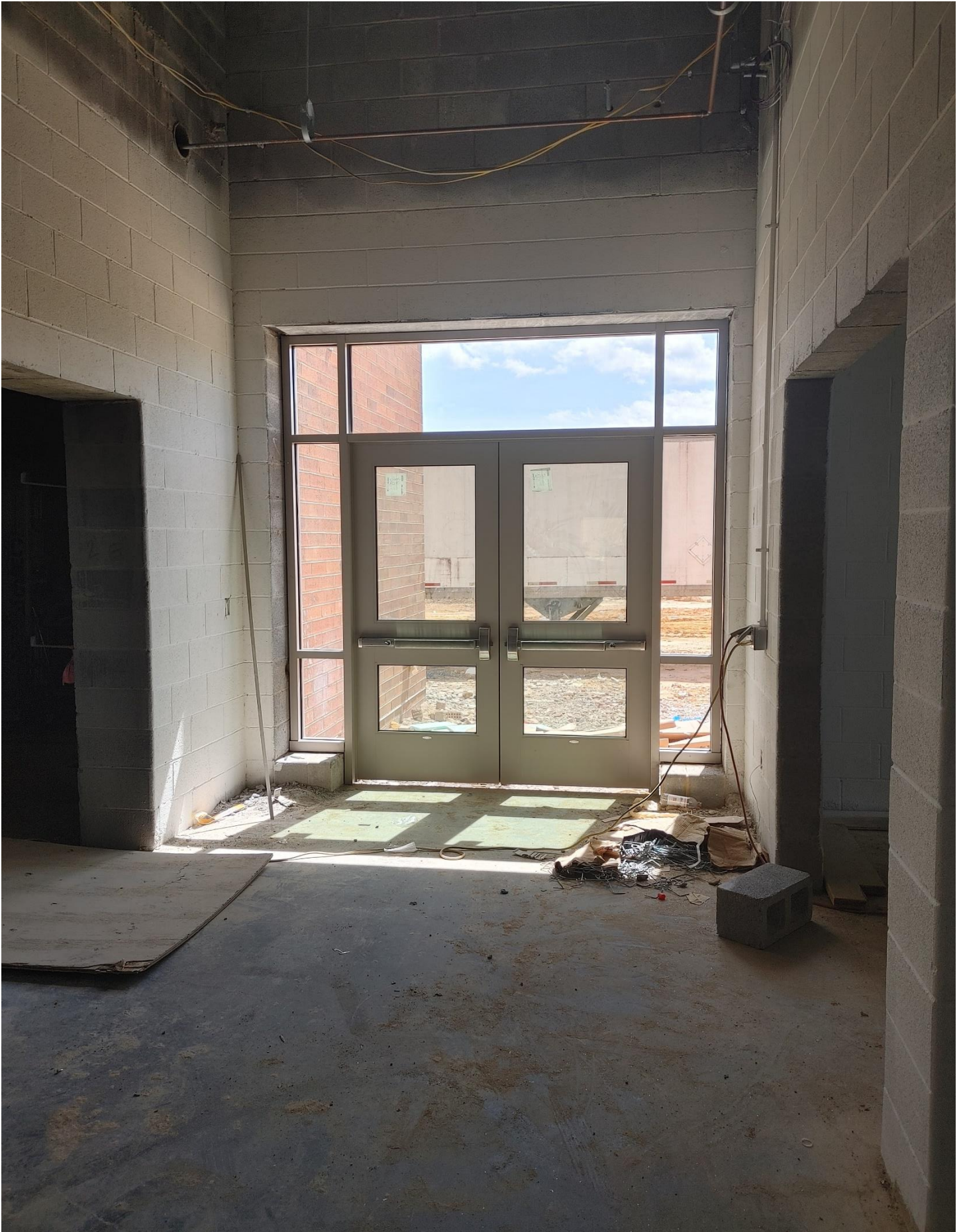
Photo 6 - Doors have been set in SF21.
