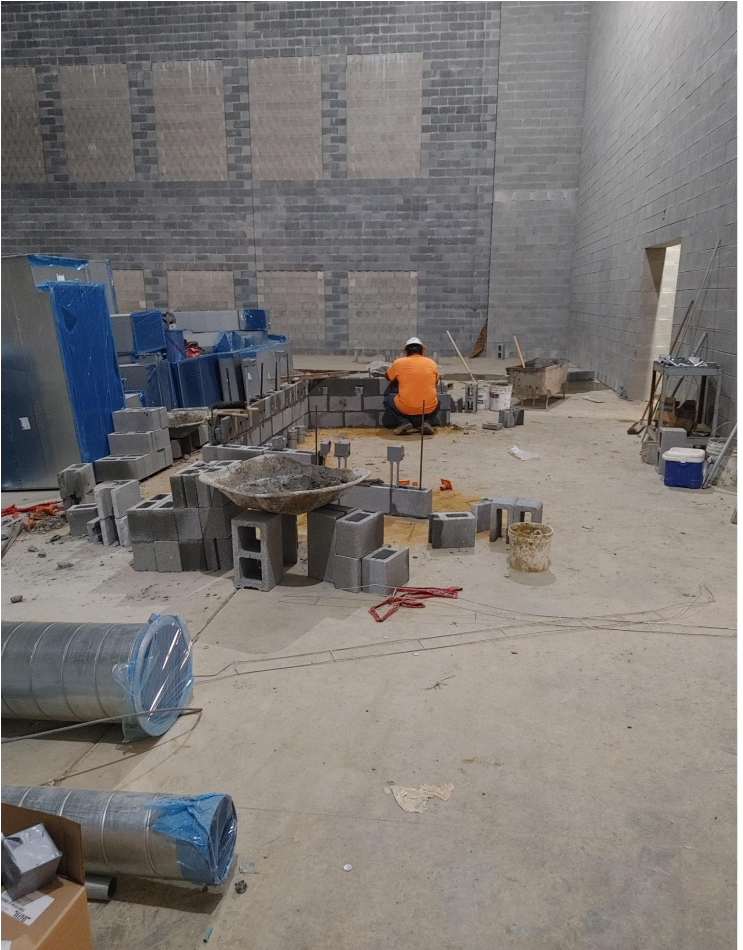
Photo 5 - Mason is laying block in the Auditorium.
