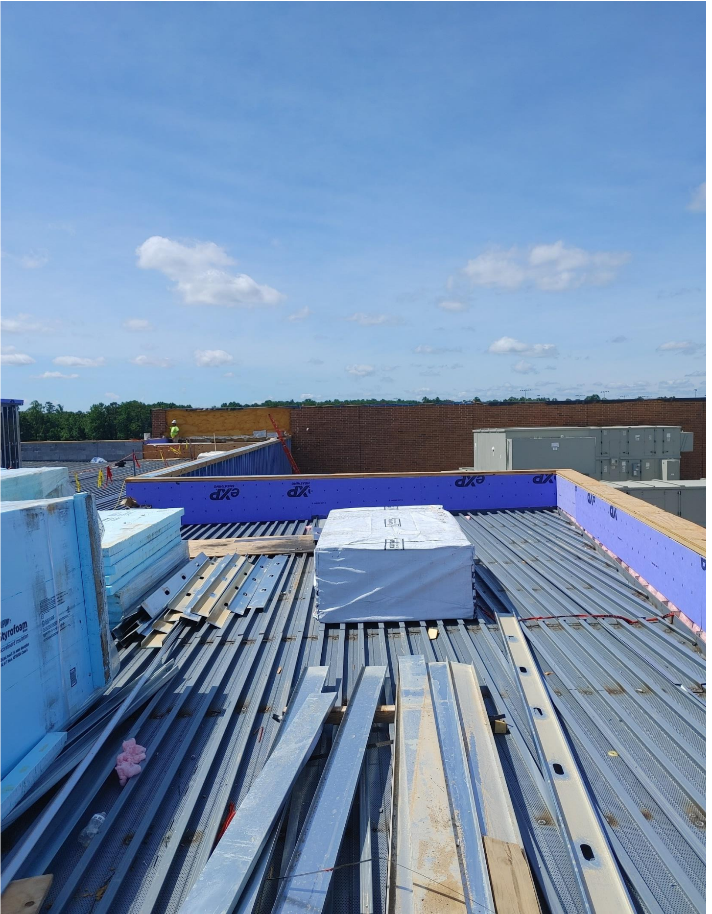
Photo 2 - Mason laying Brick on the North side of the Gym.
