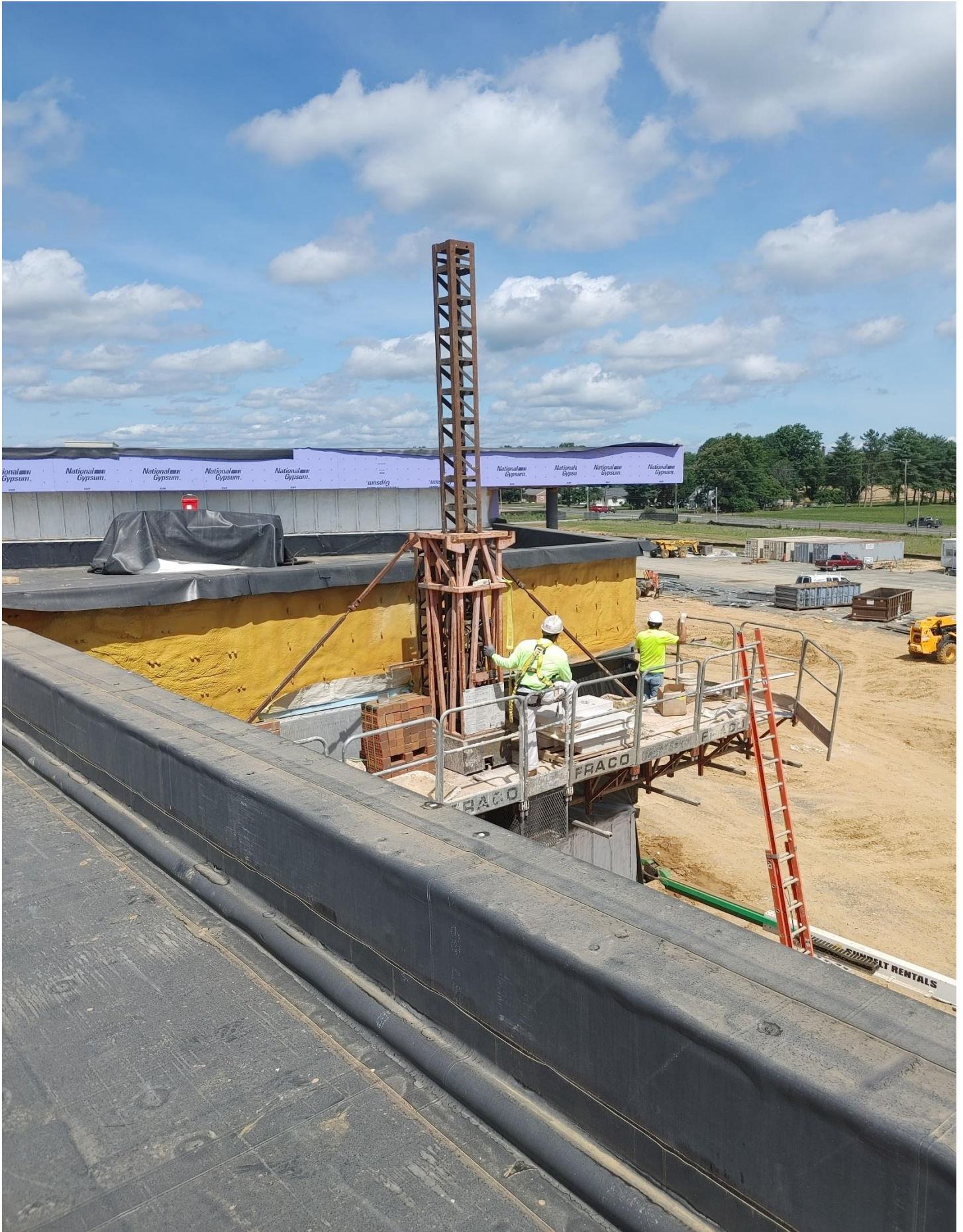
Photo 1 - Brick is being laid on the East side of Area A
