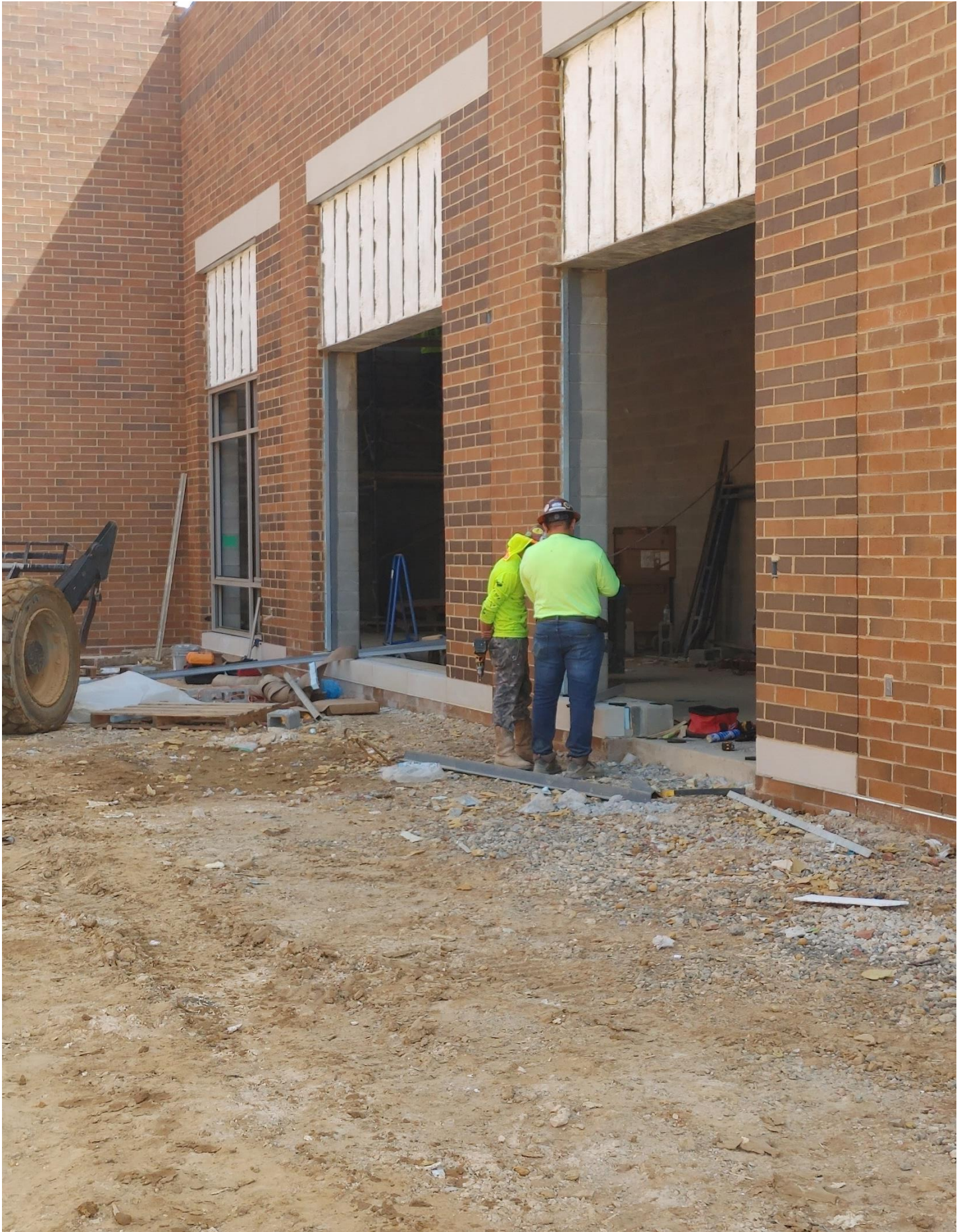
Photo 8 - FG&M is preparing openings to set SF22 & SF23
