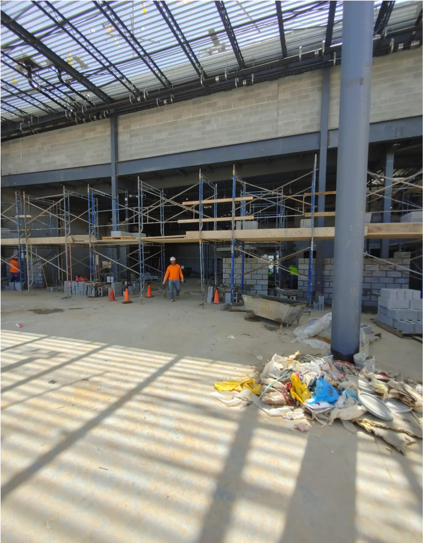
Photo 3 - Masons are laying Block in the Kitchen area.
