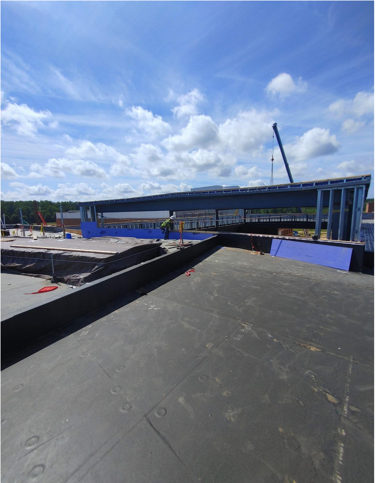
Photo 2 - Framing of high roof of Area C.
