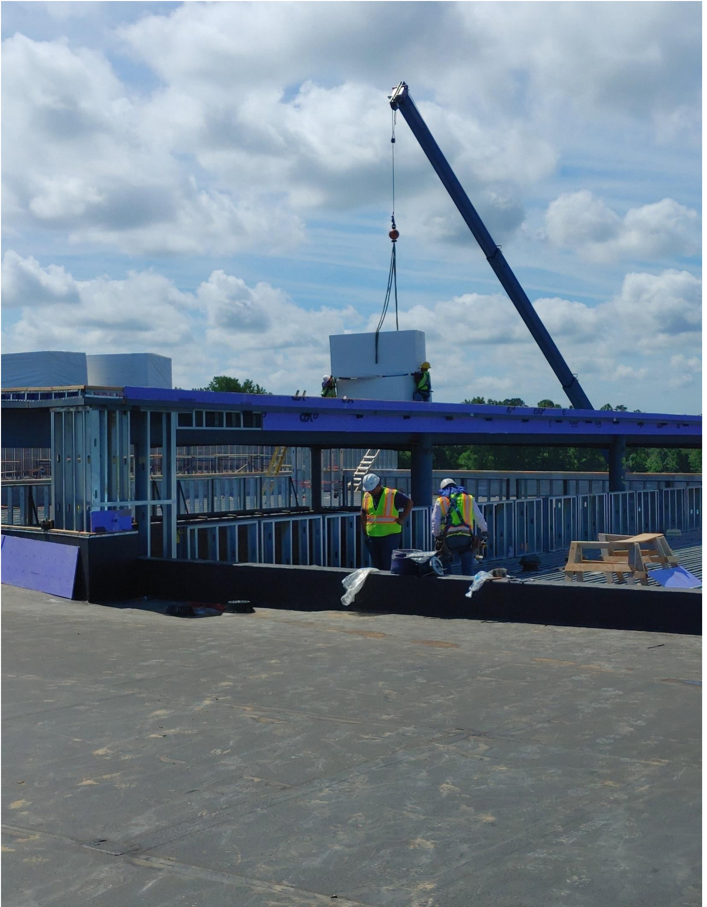
Photo 1 - Roofing material is being staged on the Roof of Area C.
