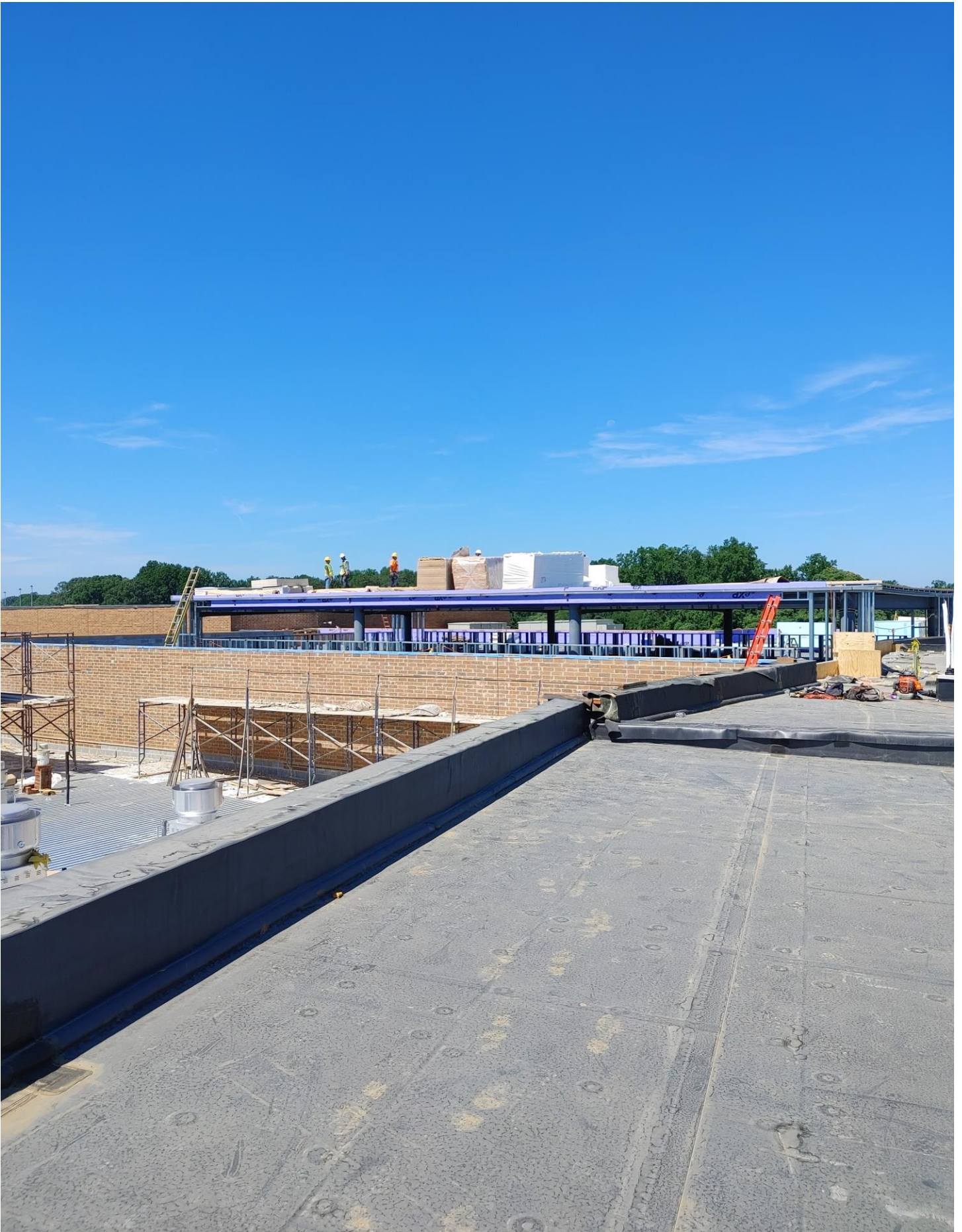
Photo 3 - Roofers are working on the high roof of Area C.
