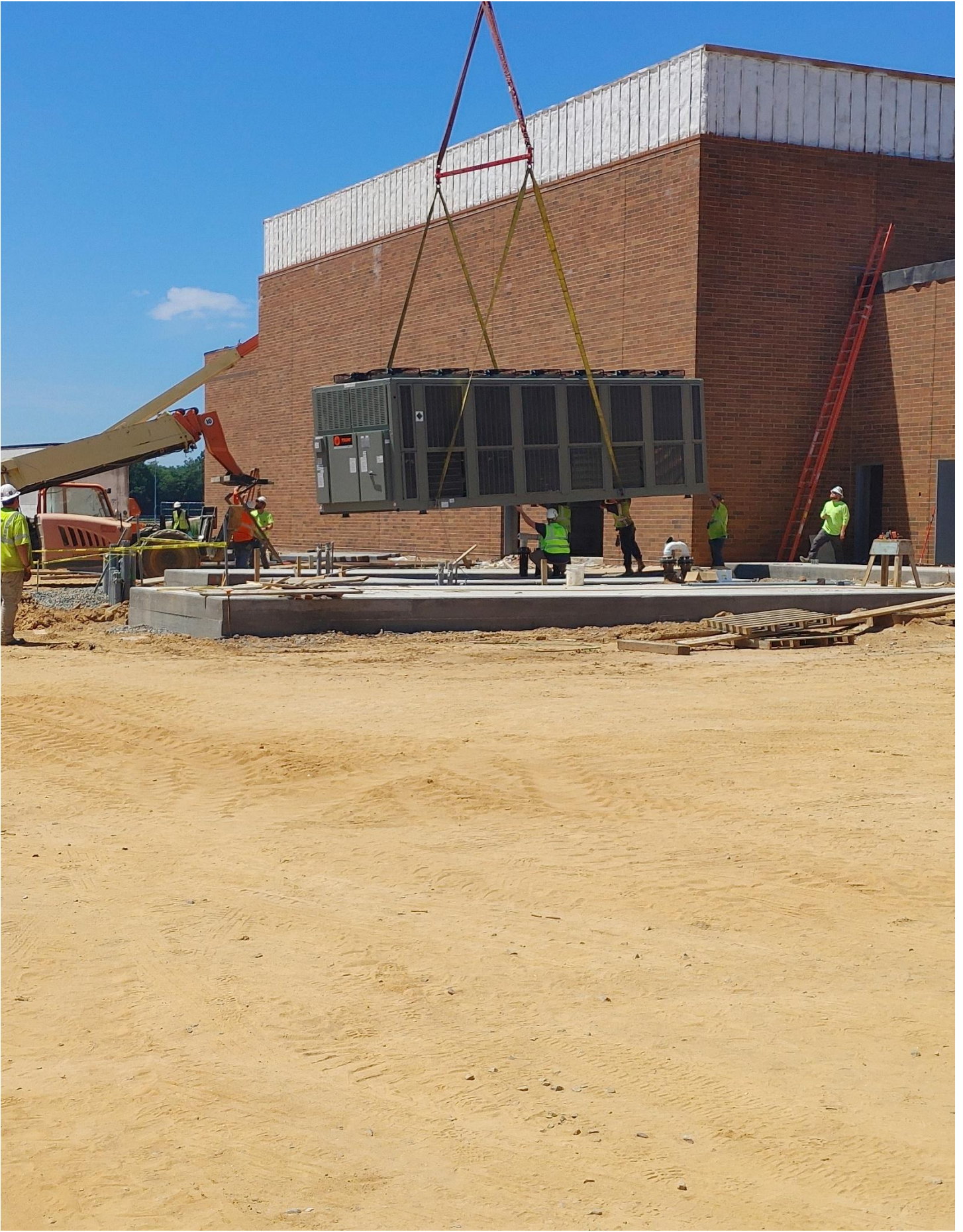
Photo 10 - One of two Chillers being set.
