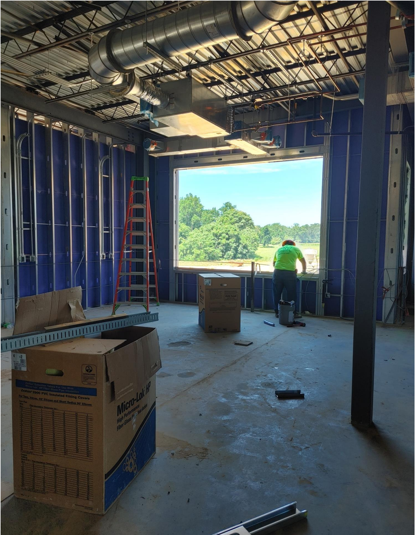
Photo 4 - SF8 opening being prepped.
