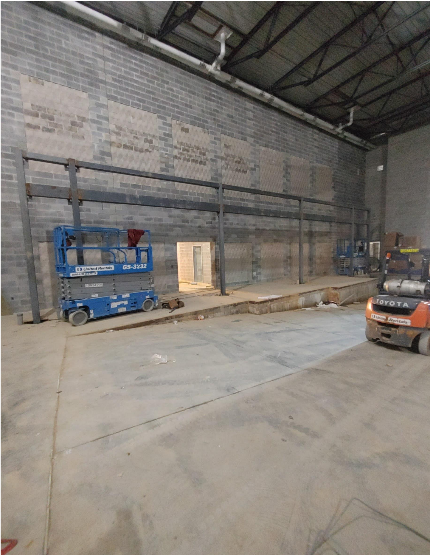
Photo 7 - Steel is being set in the Auditorium.
