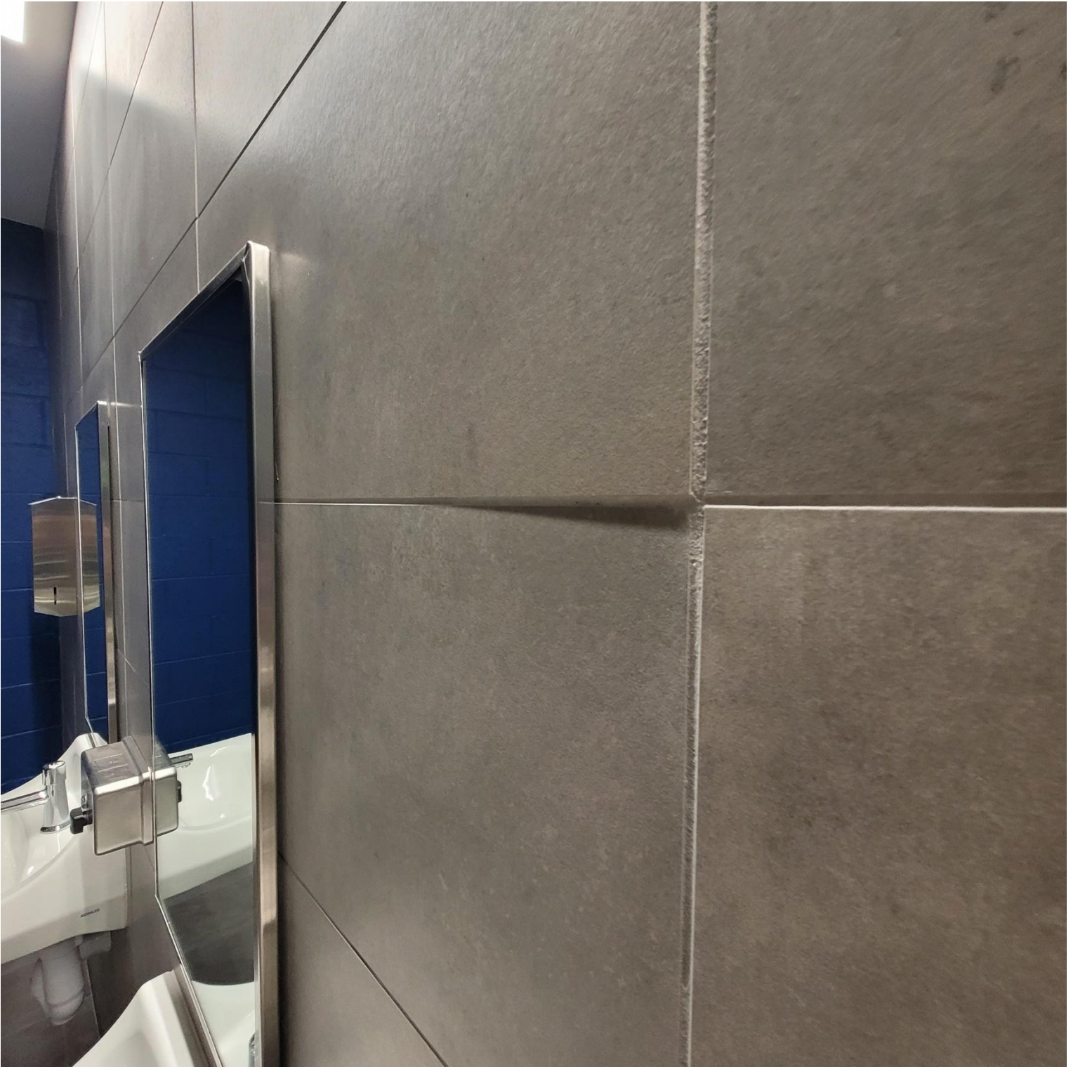
Photo 13 - Wall Tile in Boys Restroom E103
