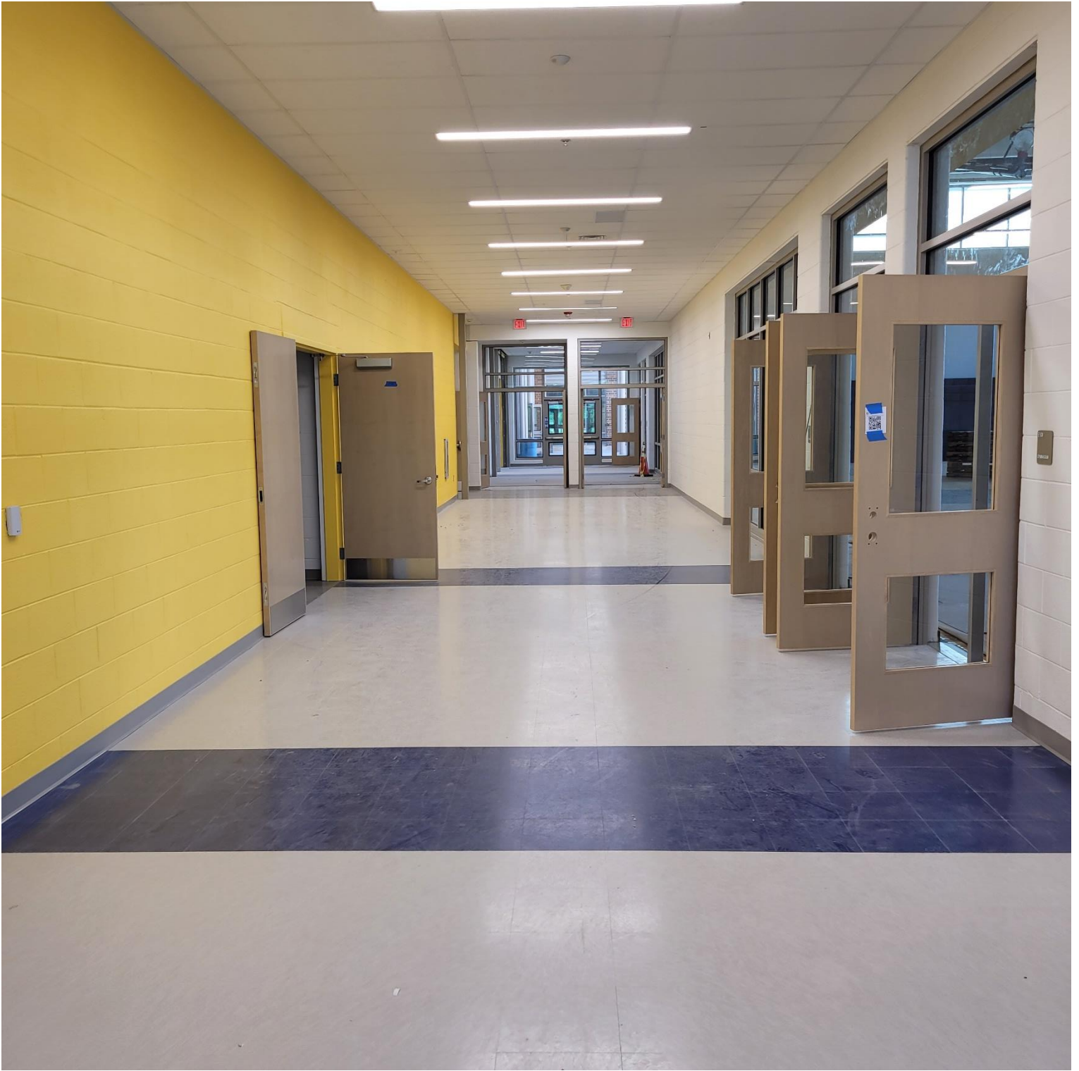
Photo 15 - Gymnasium Hallway looking East
