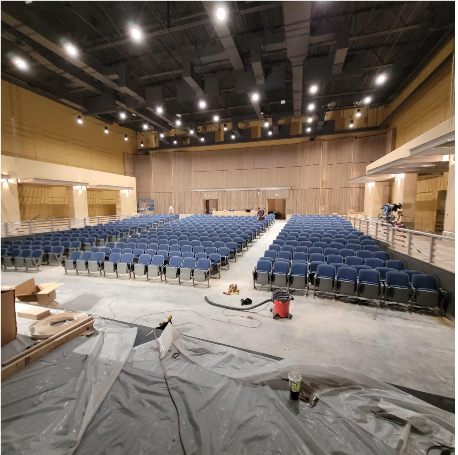
Photo 5 - Auditorium Seats are being installed
