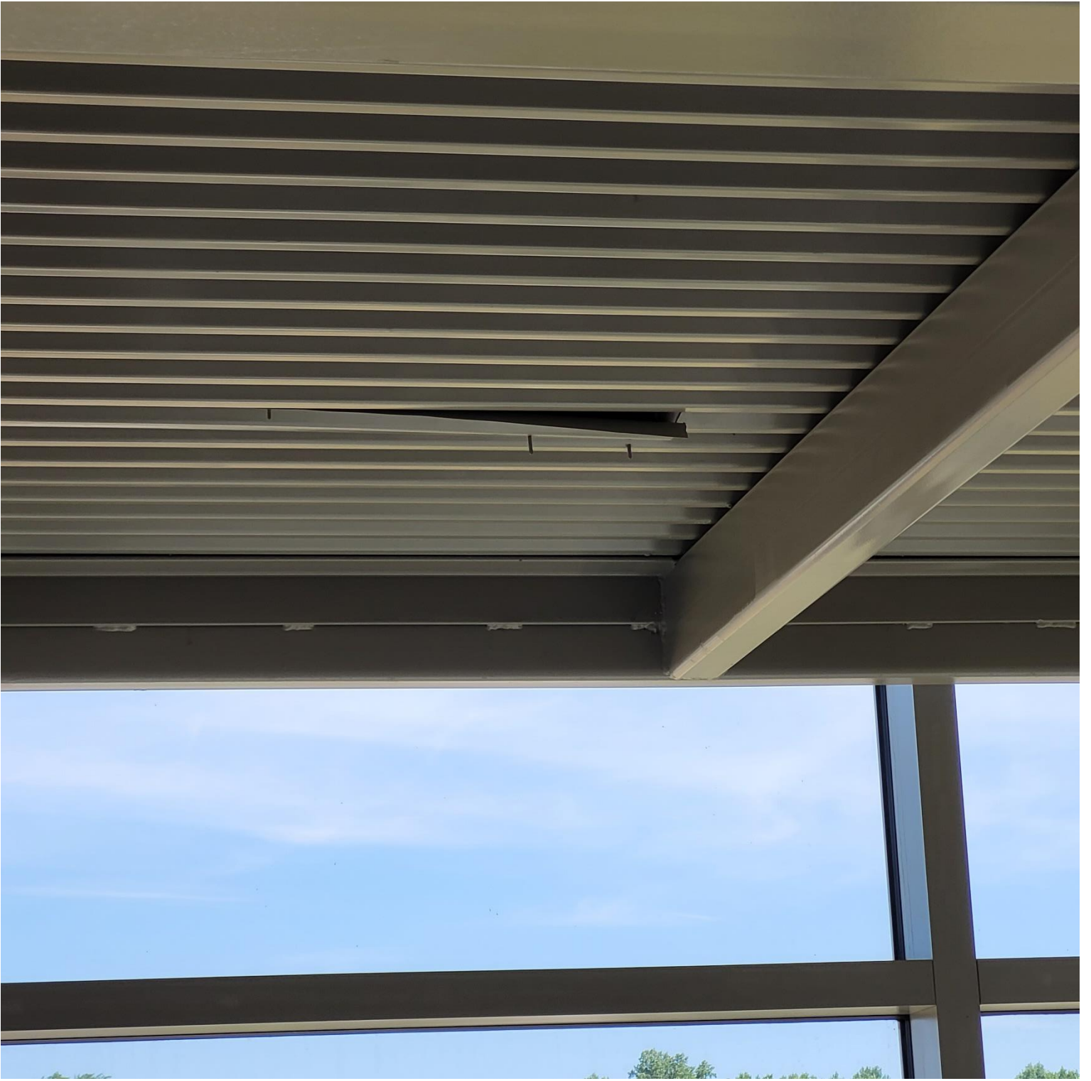
Photo 16 - Metal Decking in Stairwell #1
