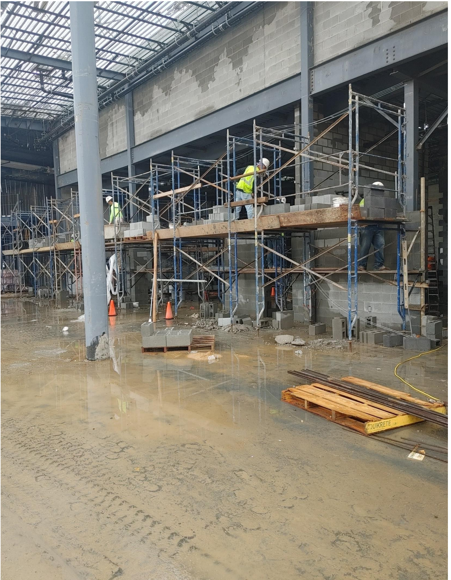
Photo 4 - Masons continue to lay block in the Kitchen
