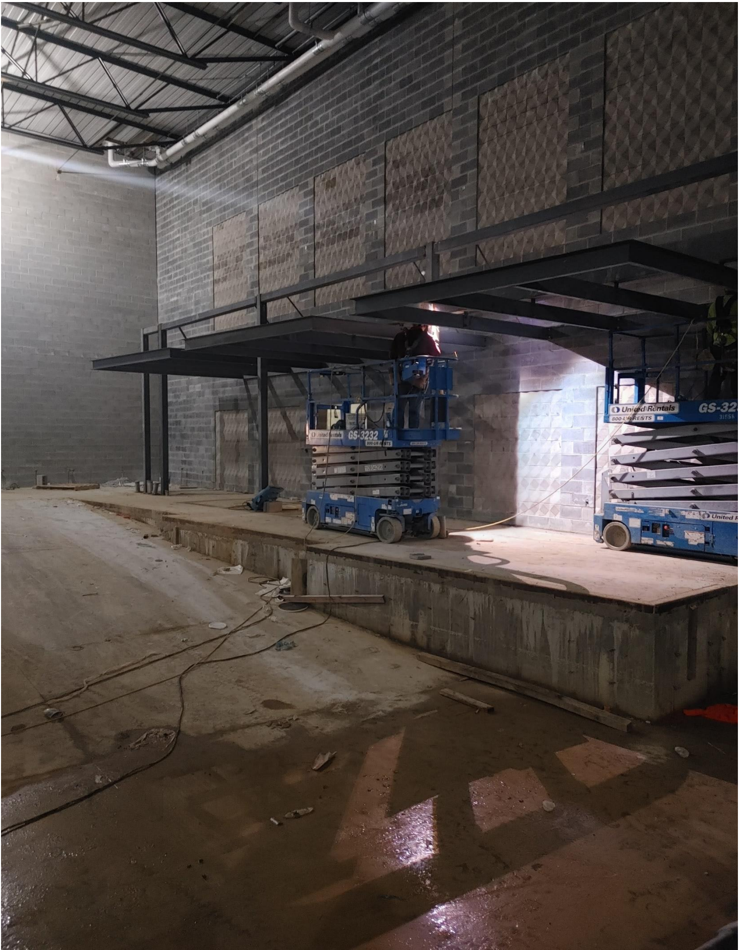
Photo 2 - Weldon Steel is cutting and welding steel in the Auditorium
