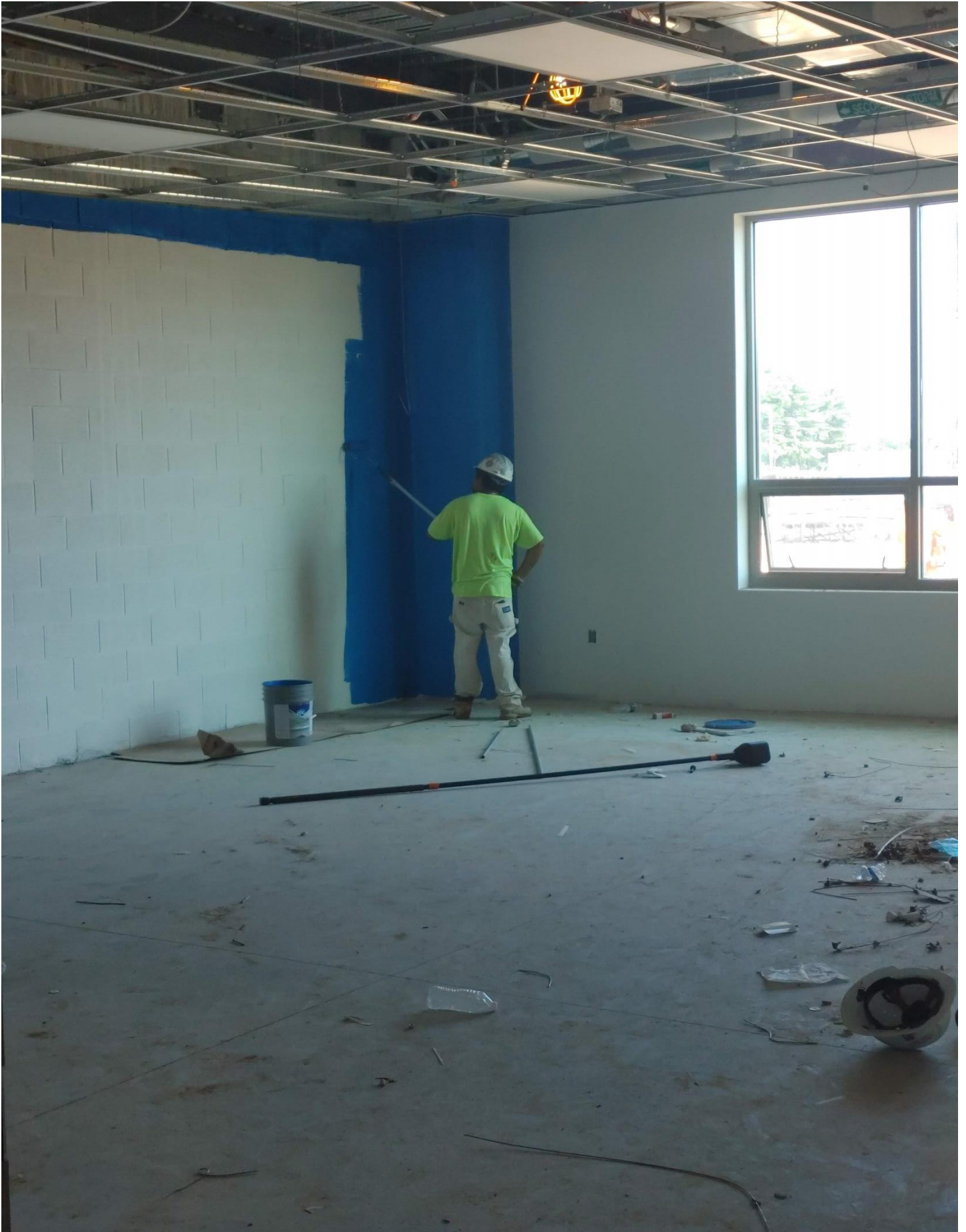
Photo 3 - Painters painting walls in Area A
