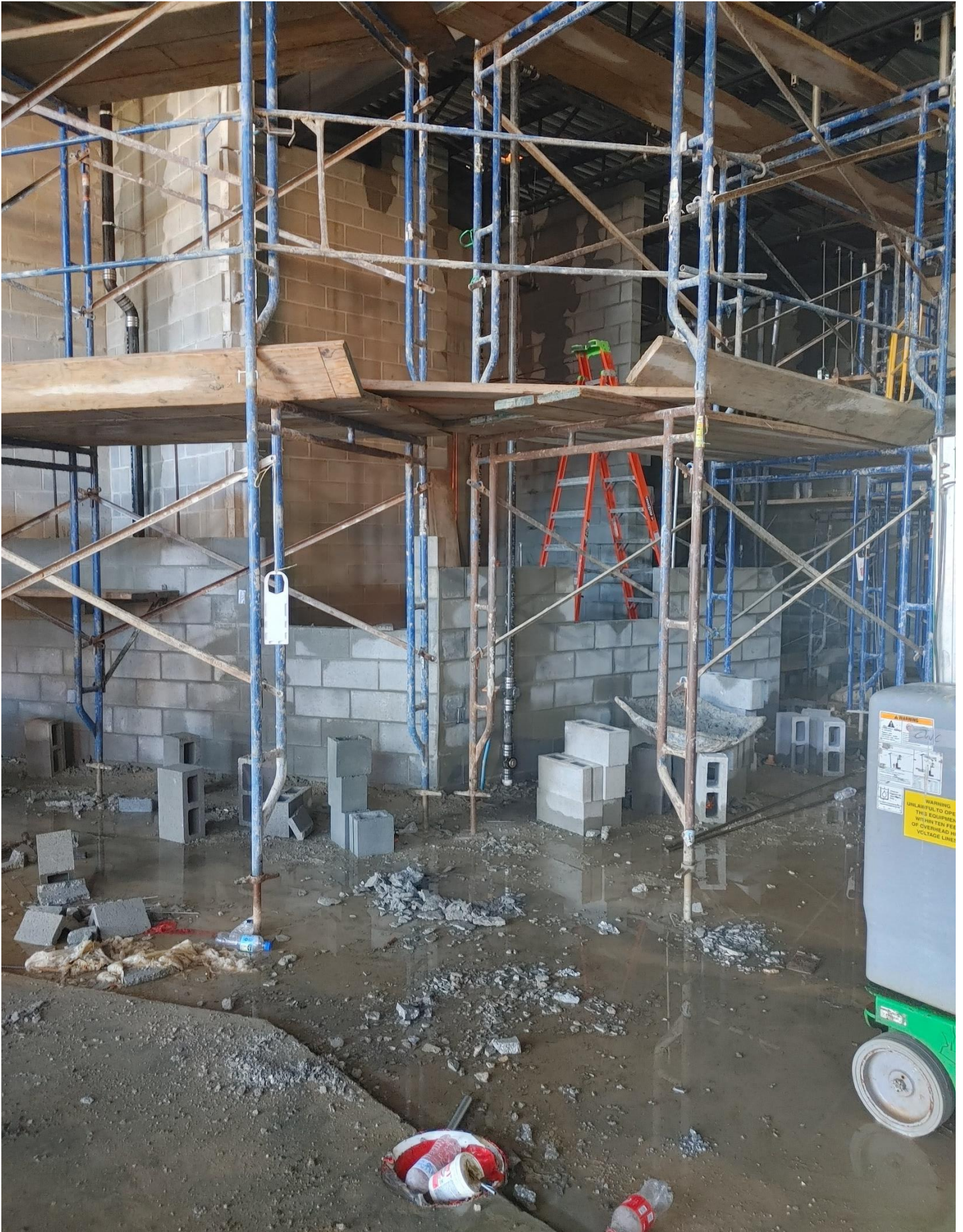
Photo 1 - Masons continue to lay block in Area C
