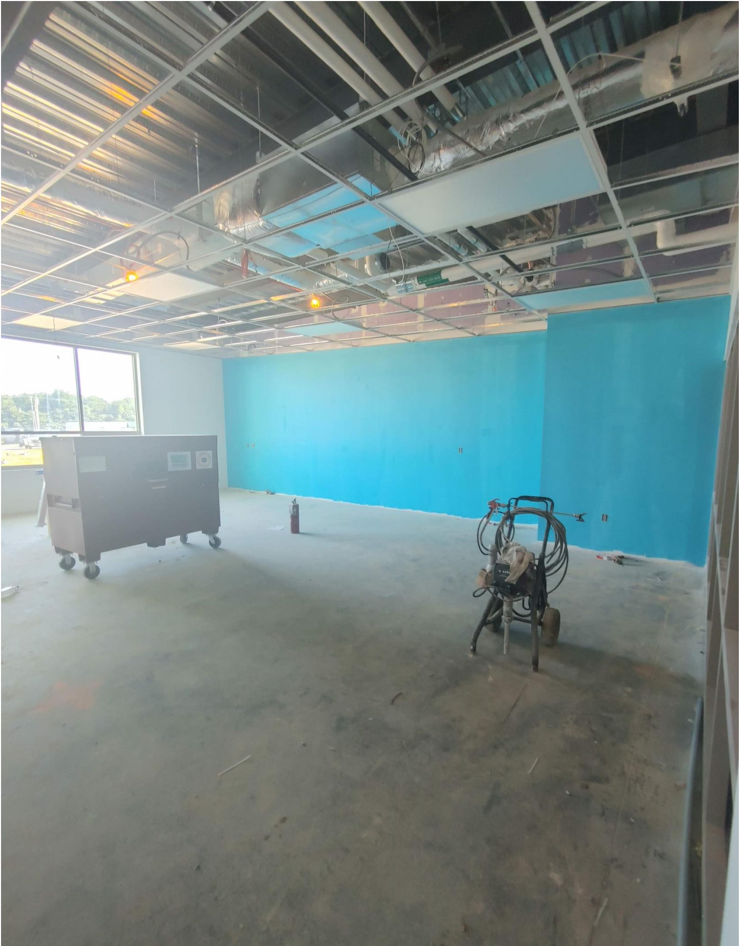
Photo 4 – Walls received first coat of paint in Area A
