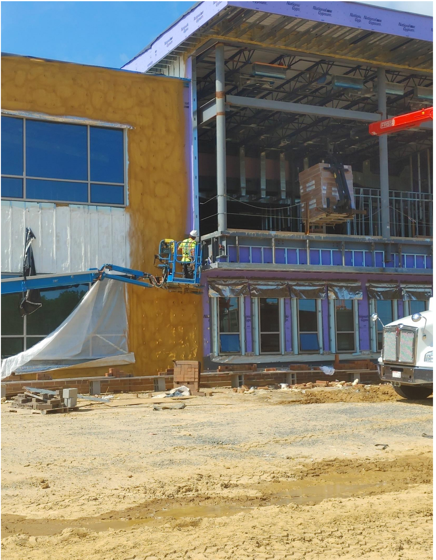
Photo 8 - Metal framing is going up on the front entrance
