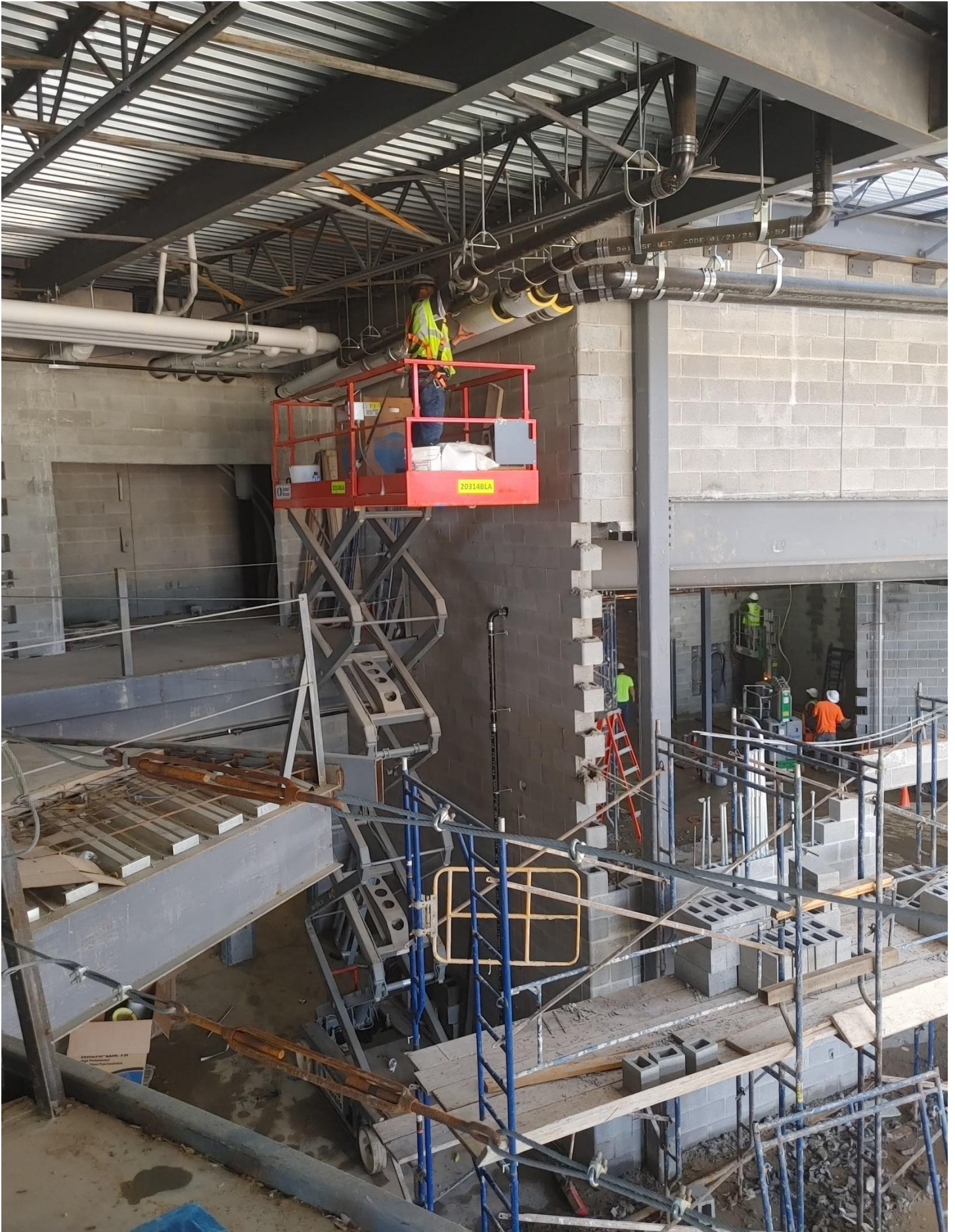
Photo 4 - Pipe being insulated in Area A
