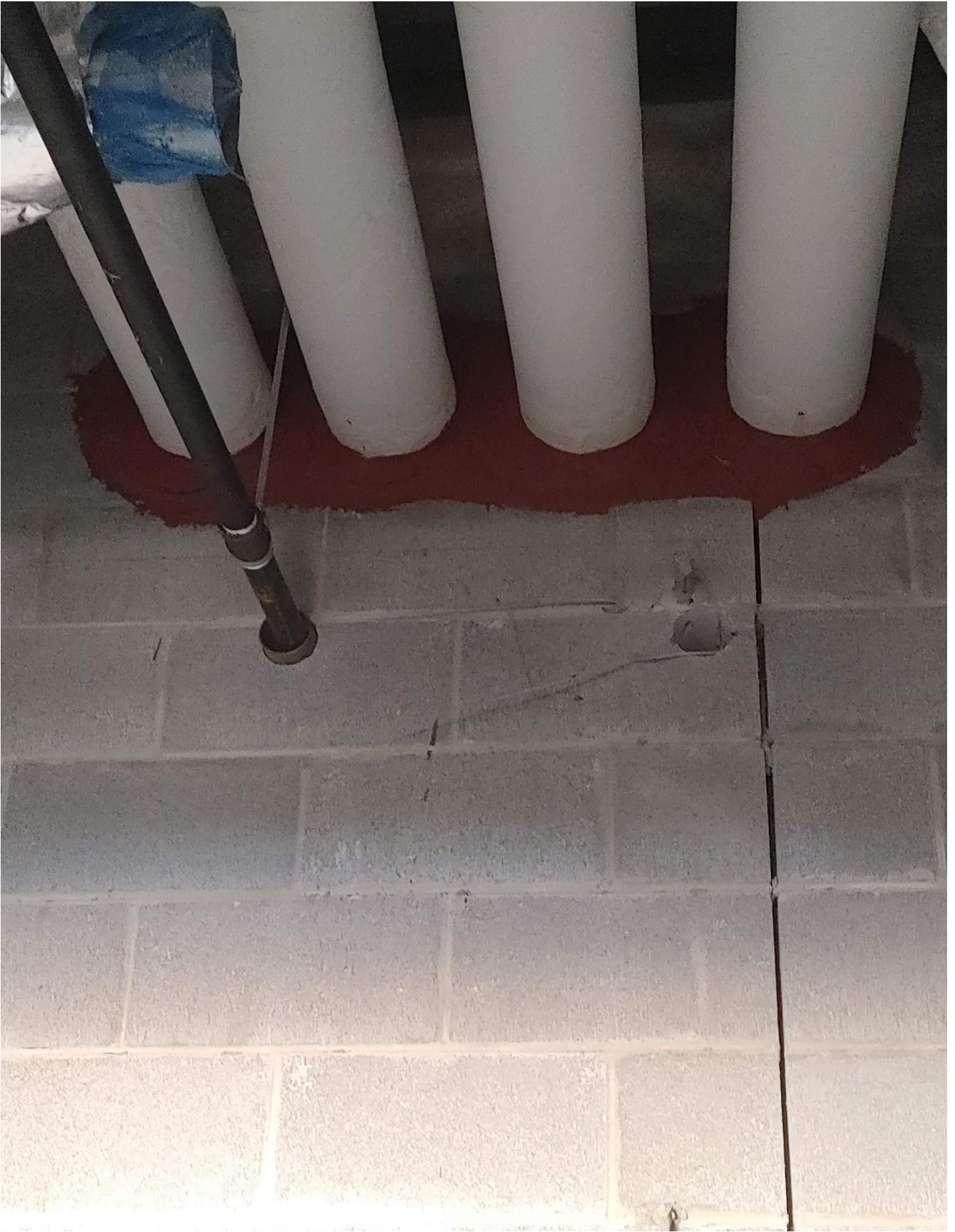
Photo 5 - Fire caulking has been applied around pipe in Area A
