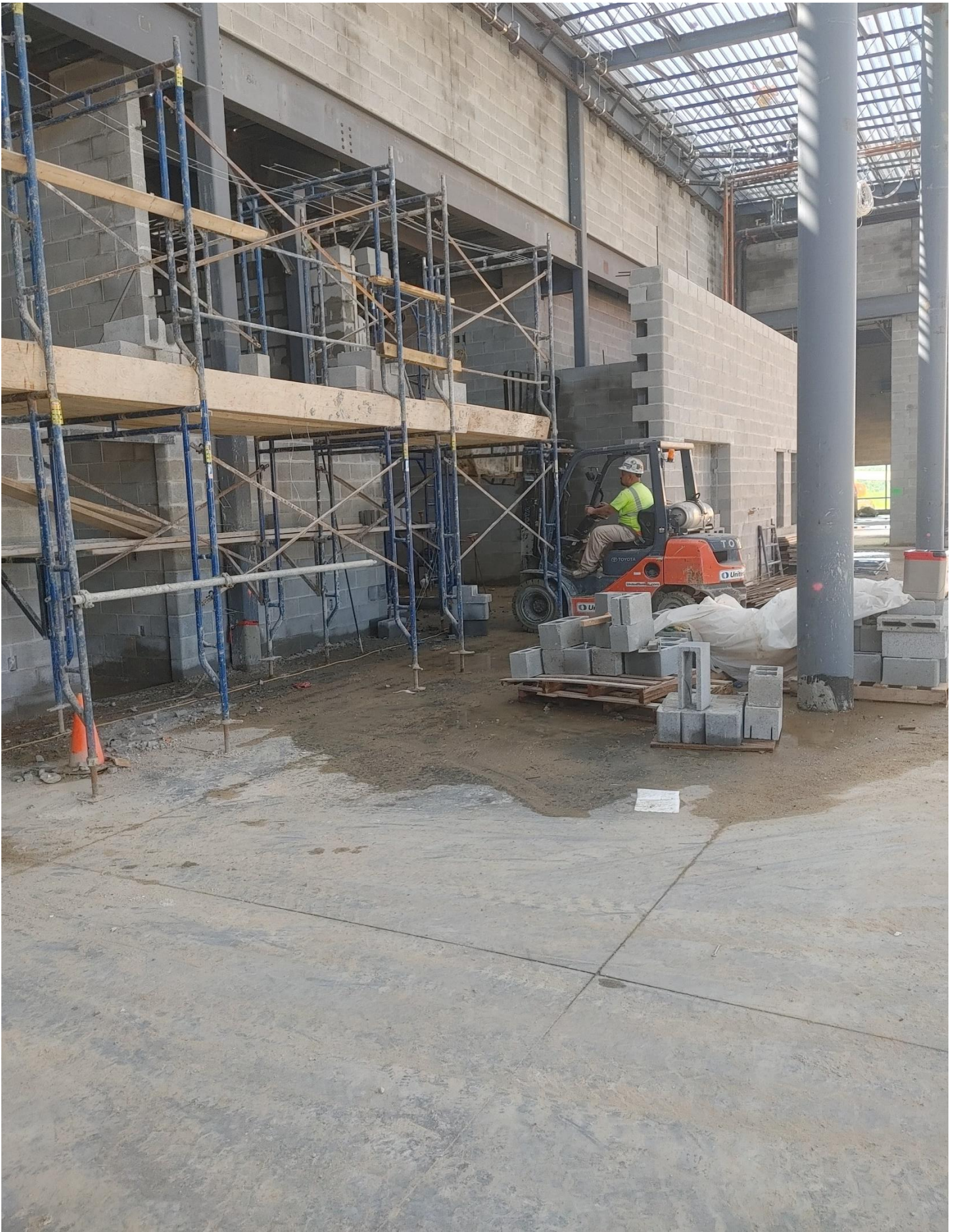
Photo 6 - Masons continue to lay block in the Kitchen area
