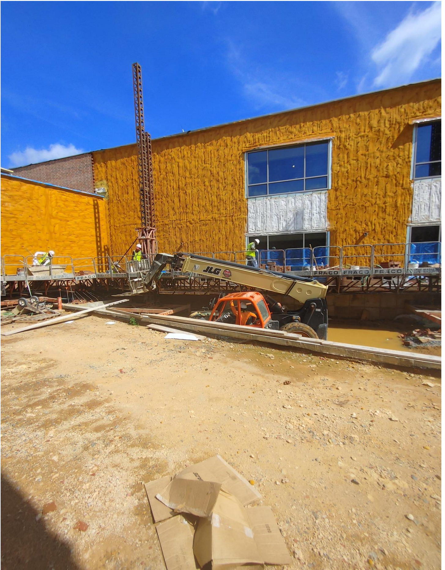
Photo 7 - Brick is being laid in the Loading Dock Area
