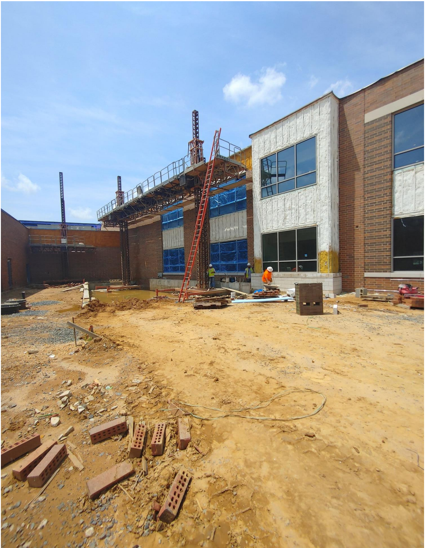
Photo 1 - Precast is being laid on the South side of Area A
