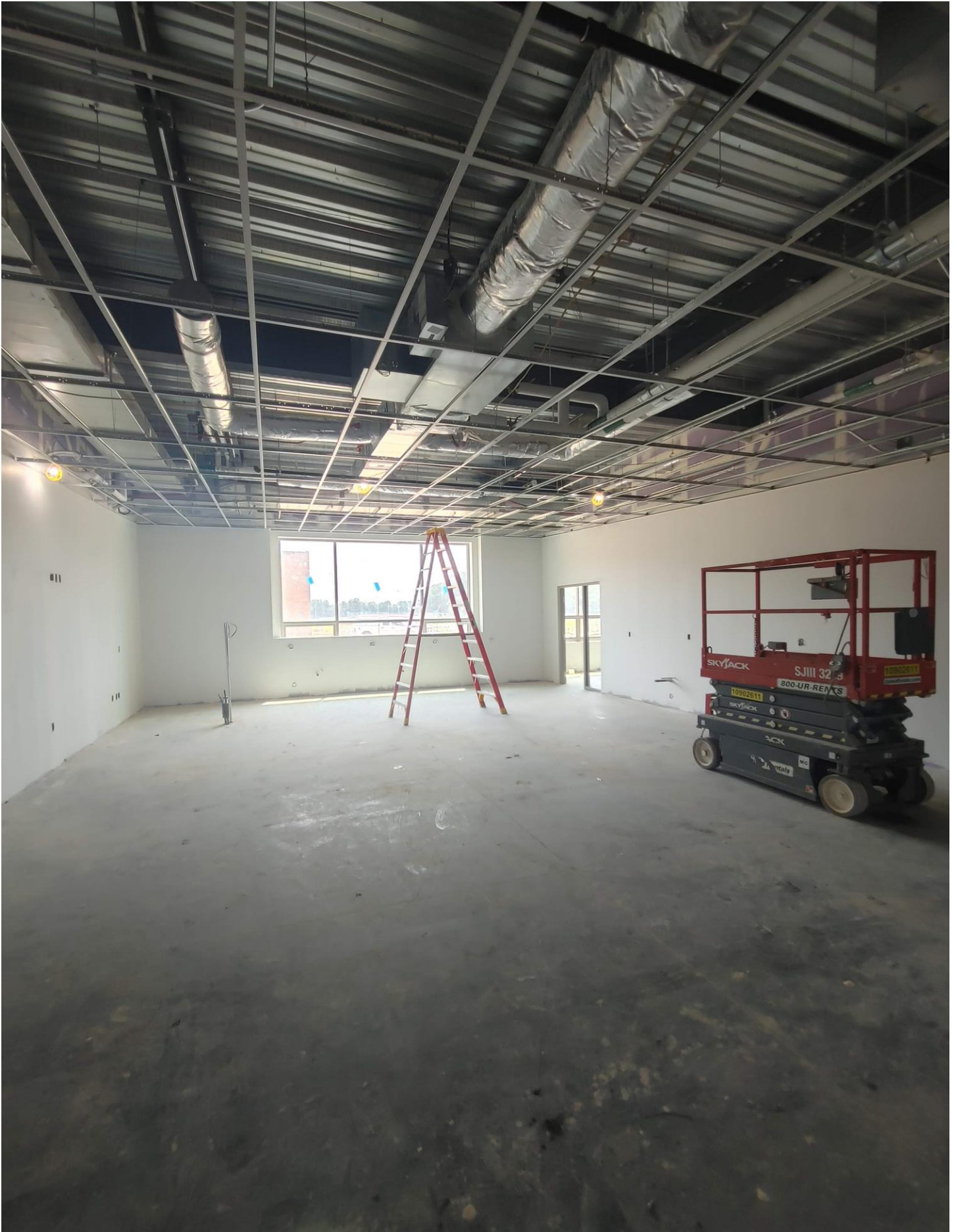
Photo 5 - Acoustical Ceiling Grid is being installed in Area B
