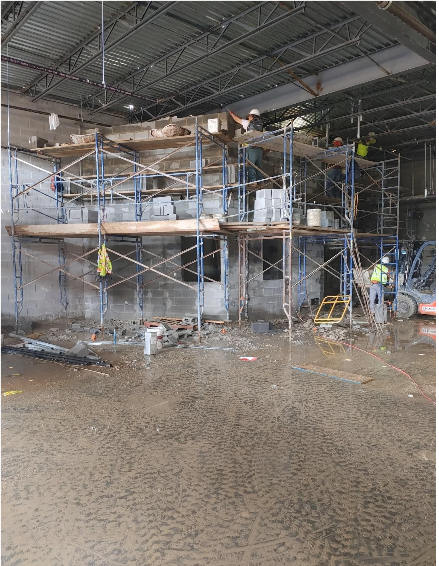
Photo 3 - Mason continue to lay block in the Kitchen area.
