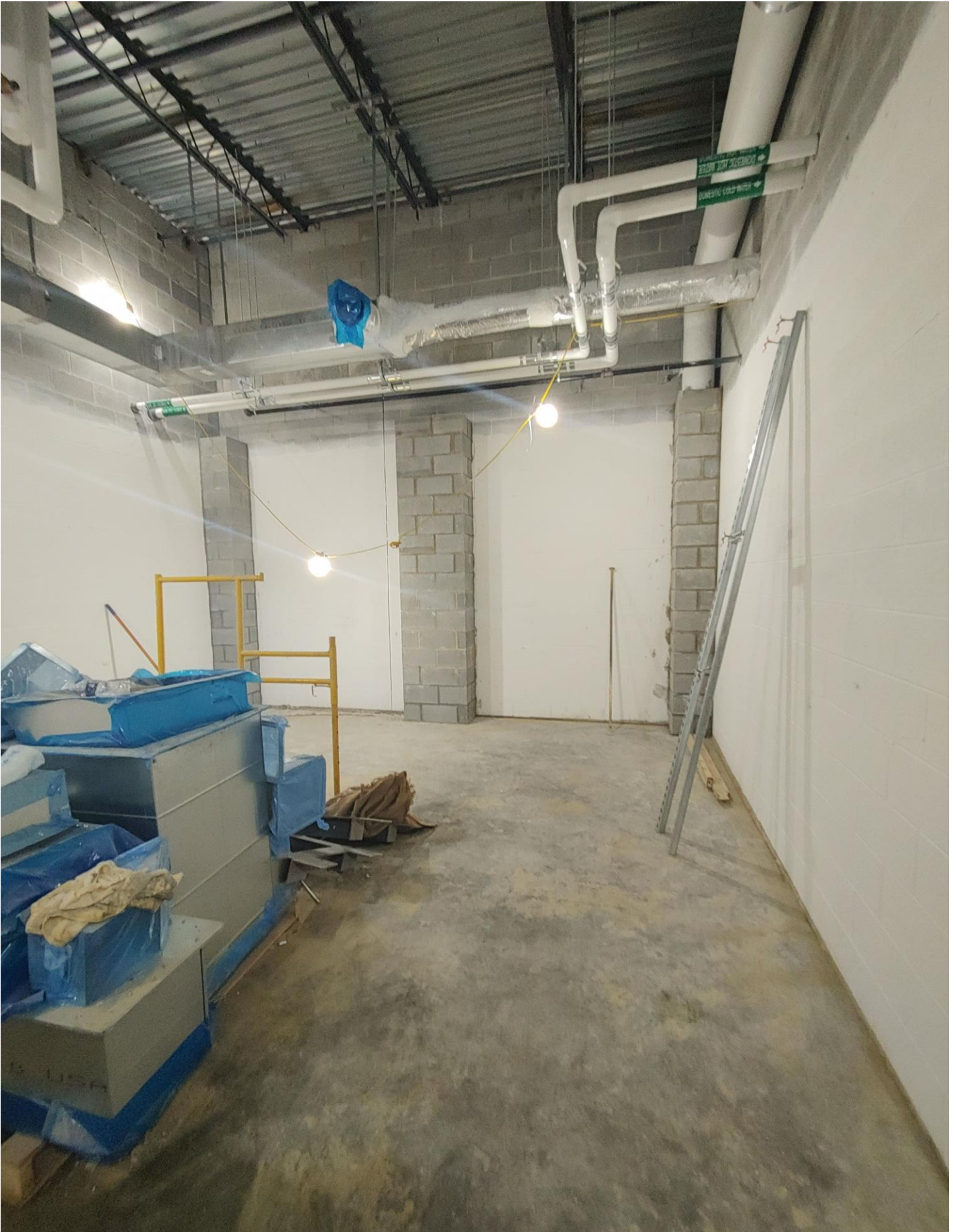
Photo 4 - The Masons are laying chase walls in Area e
