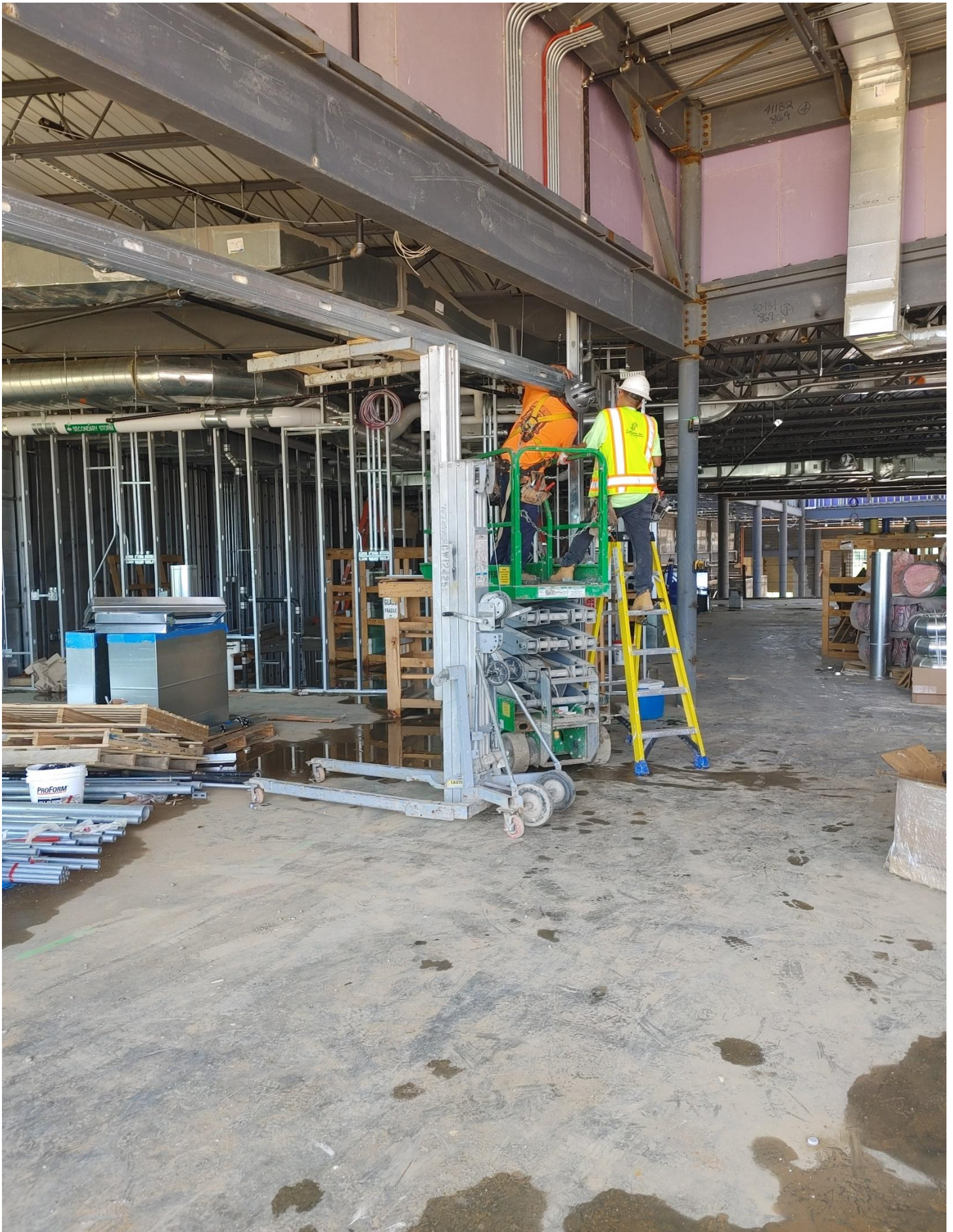
Photo 6 - Walls being framed on the 2nd floor of Area A
