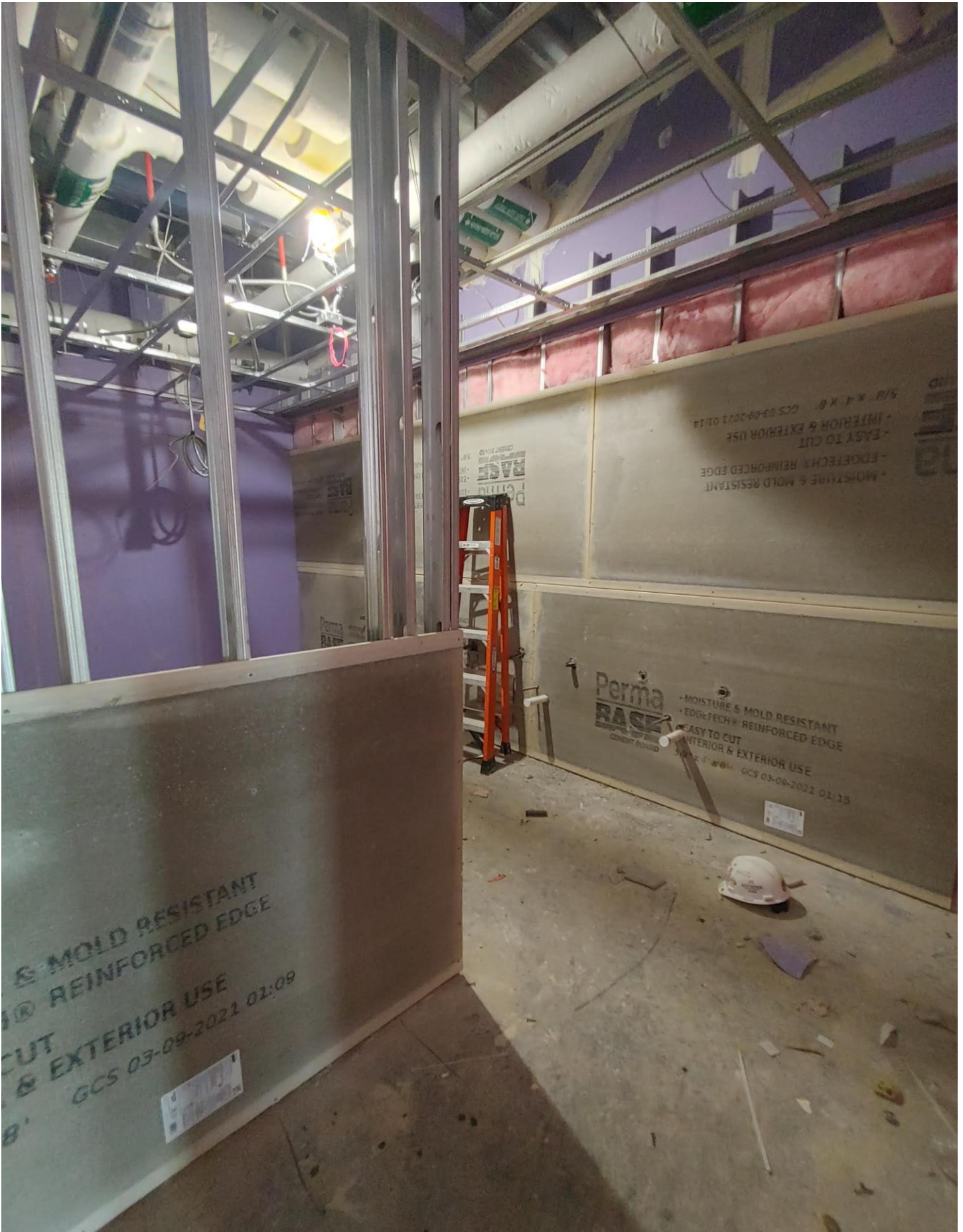
Photo 5 - Cement Board is being hung in rooms A216 & A218
