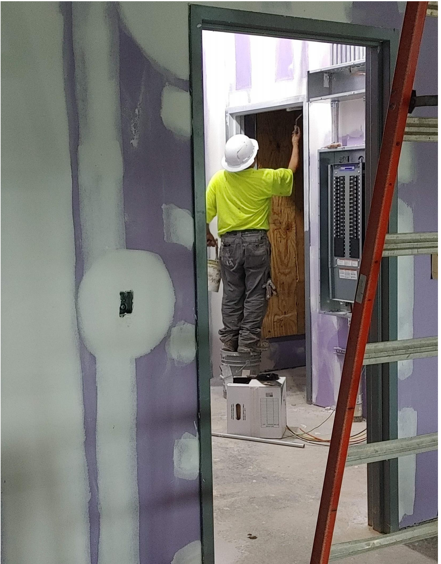
Photo 9 - Door frames are being primed in Area B
