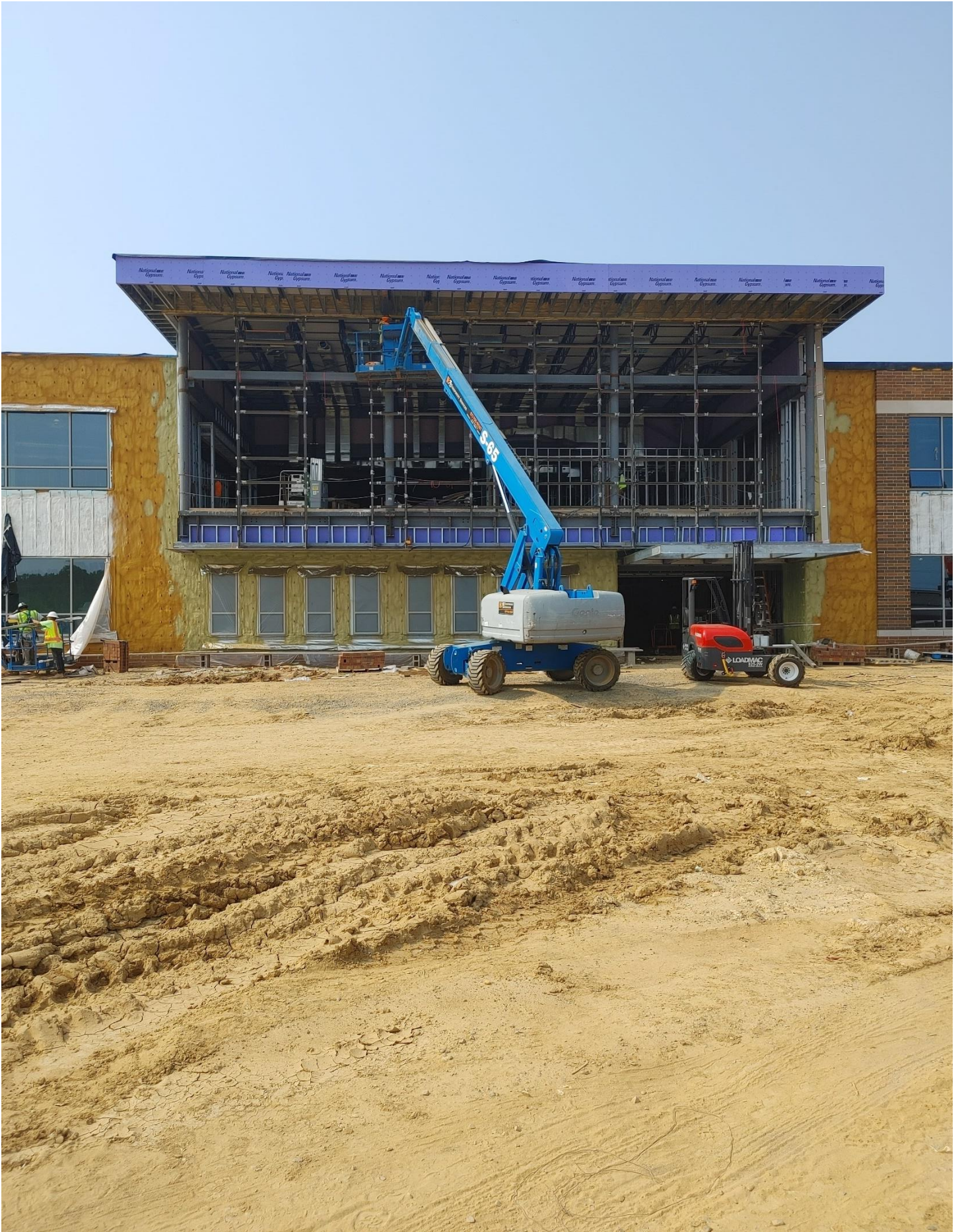
Photo 1 - Curtain Wall #9 going up.
