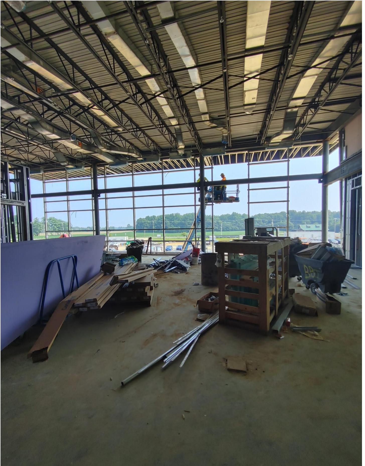
Photo 7 - Curtain Wall #9 being installed.
