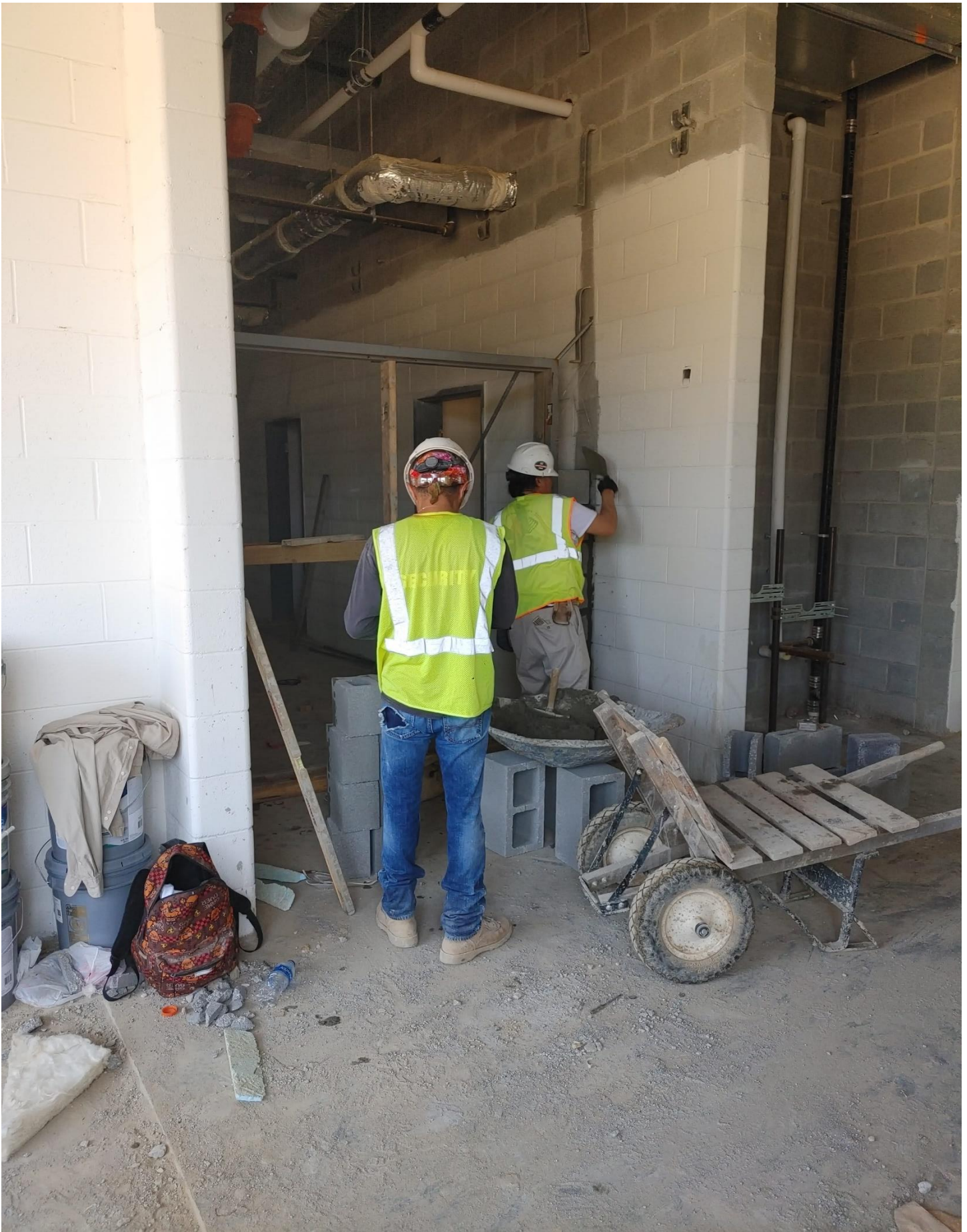
Photo 11 - Masons are laying block around door frame #E13.
