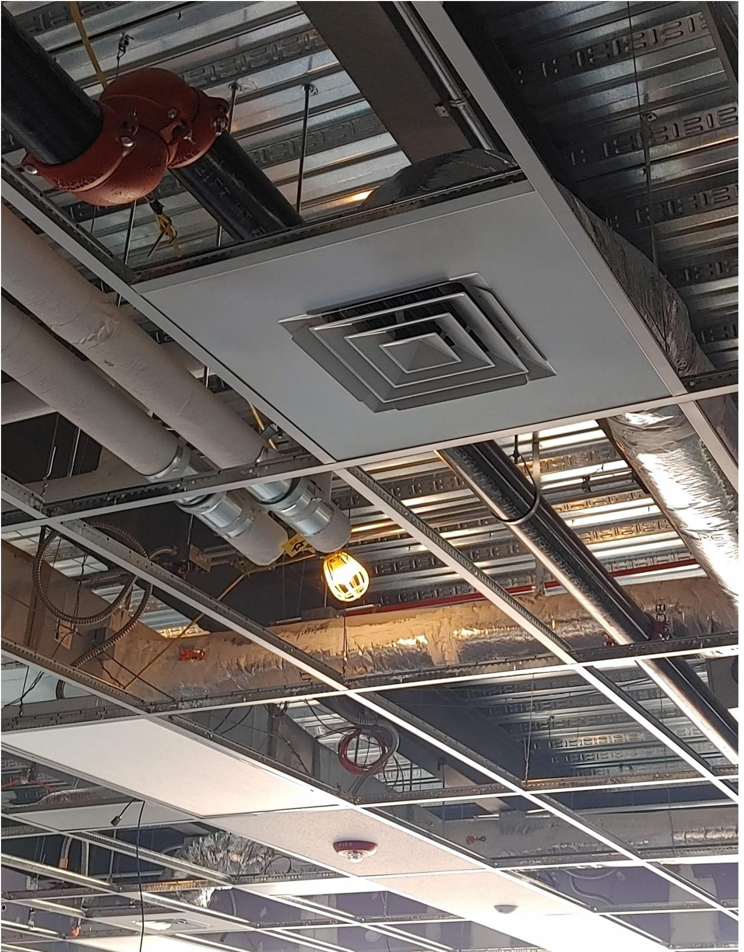
Photo 4 - Diffusers continue to be installed in Area A.
