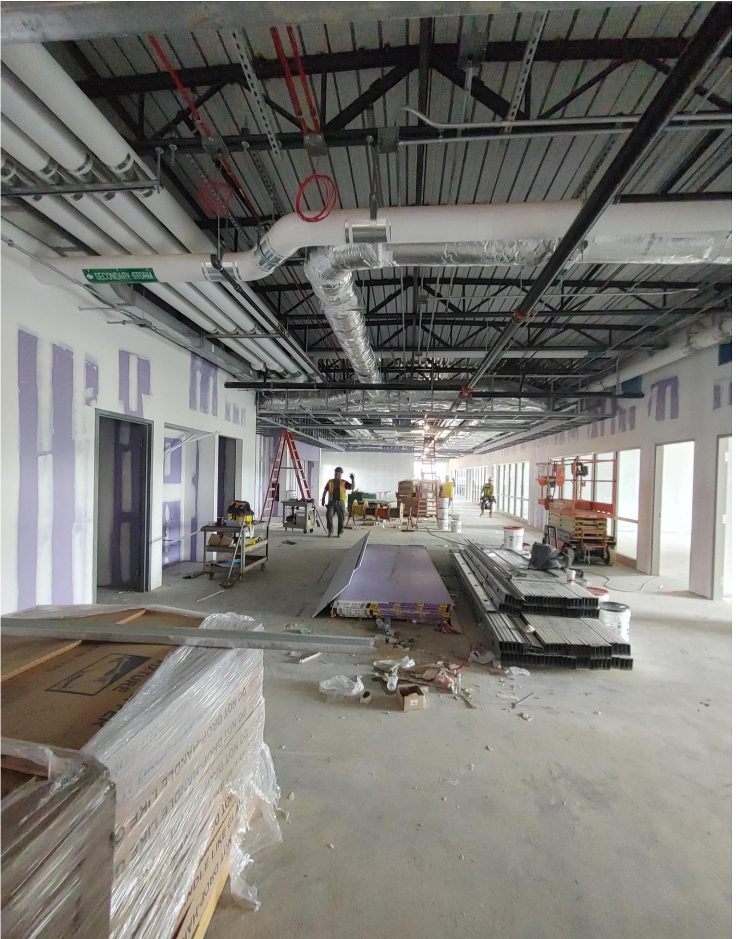
Photo 8 - Bulkhead being constructed on the 2nd floor of Area B
