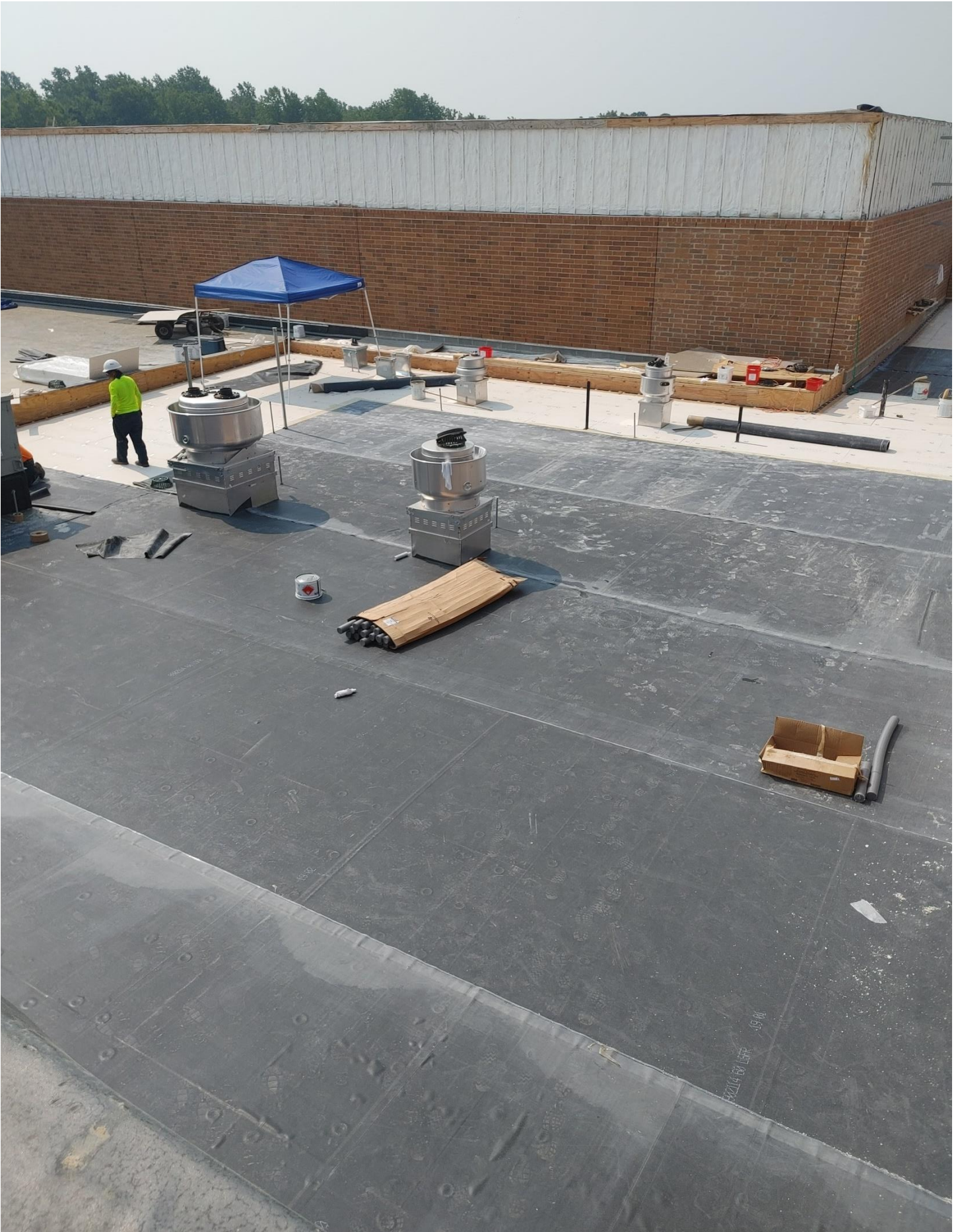
Photo 10 - Roofers continue to work on the roof above the Kitchen.
