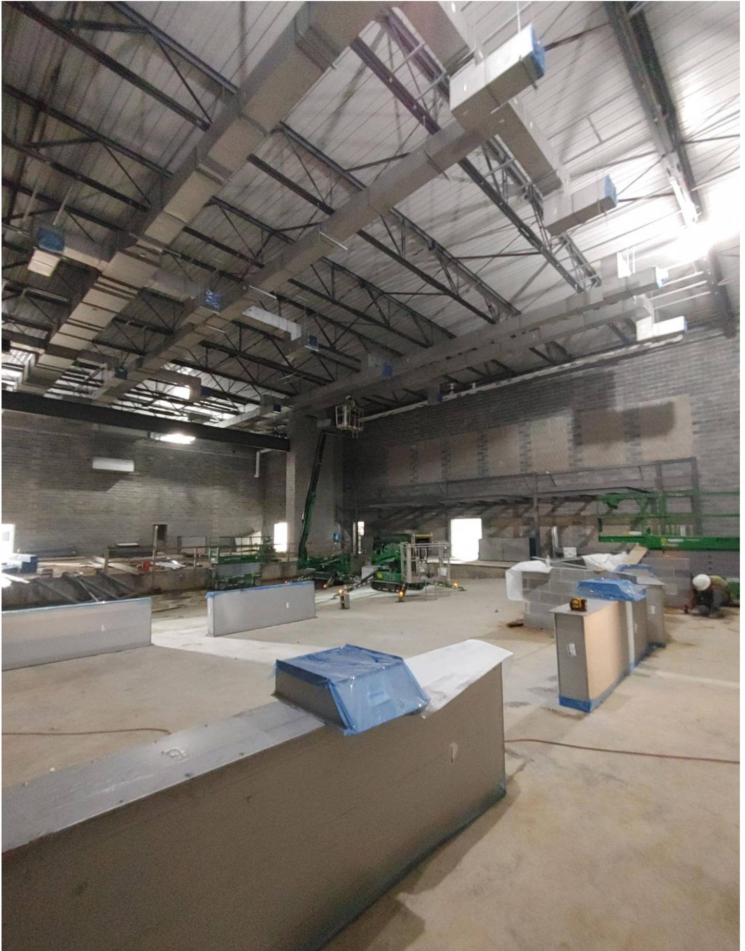
Photo 13 - HVAC Duct continues to be installed in the Auditorium.
