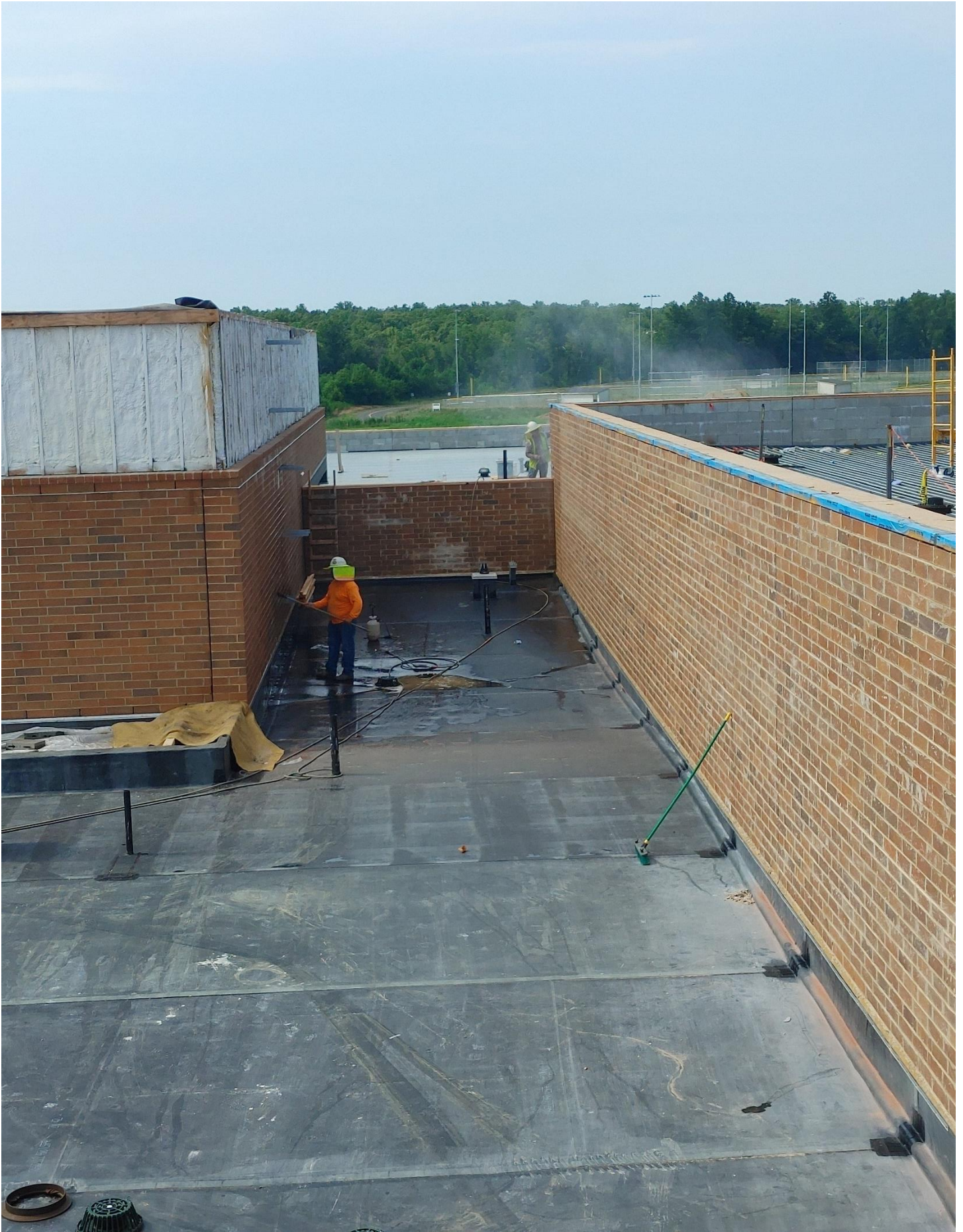
Photo 8 - Brick is being cleaned above the Kitchen in Area C
