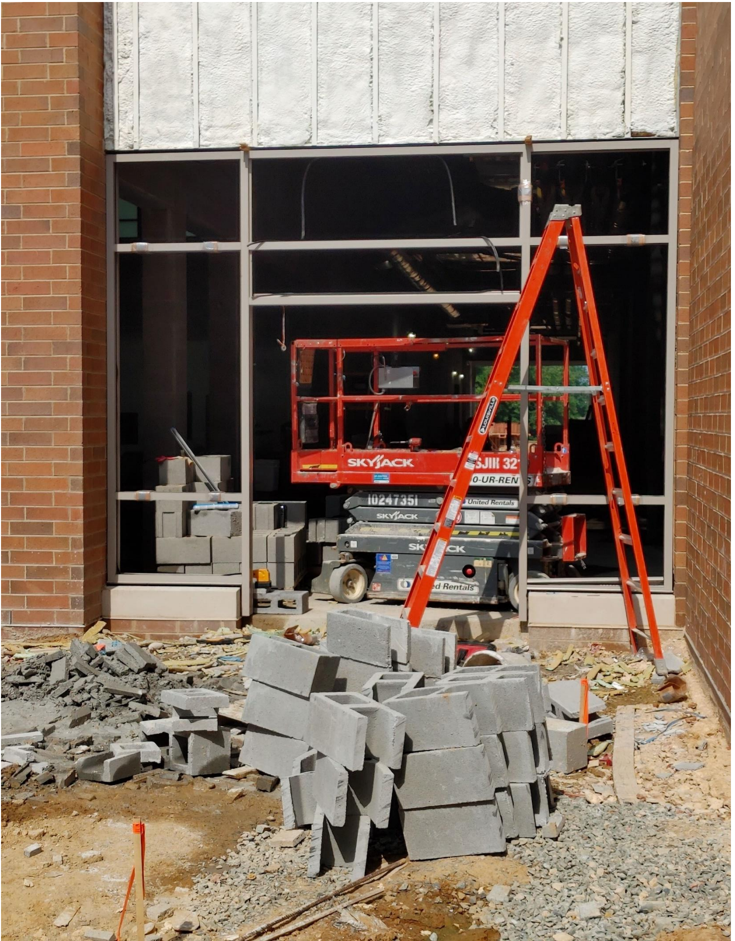
Photo 6 - SF20 is being set in Area E
