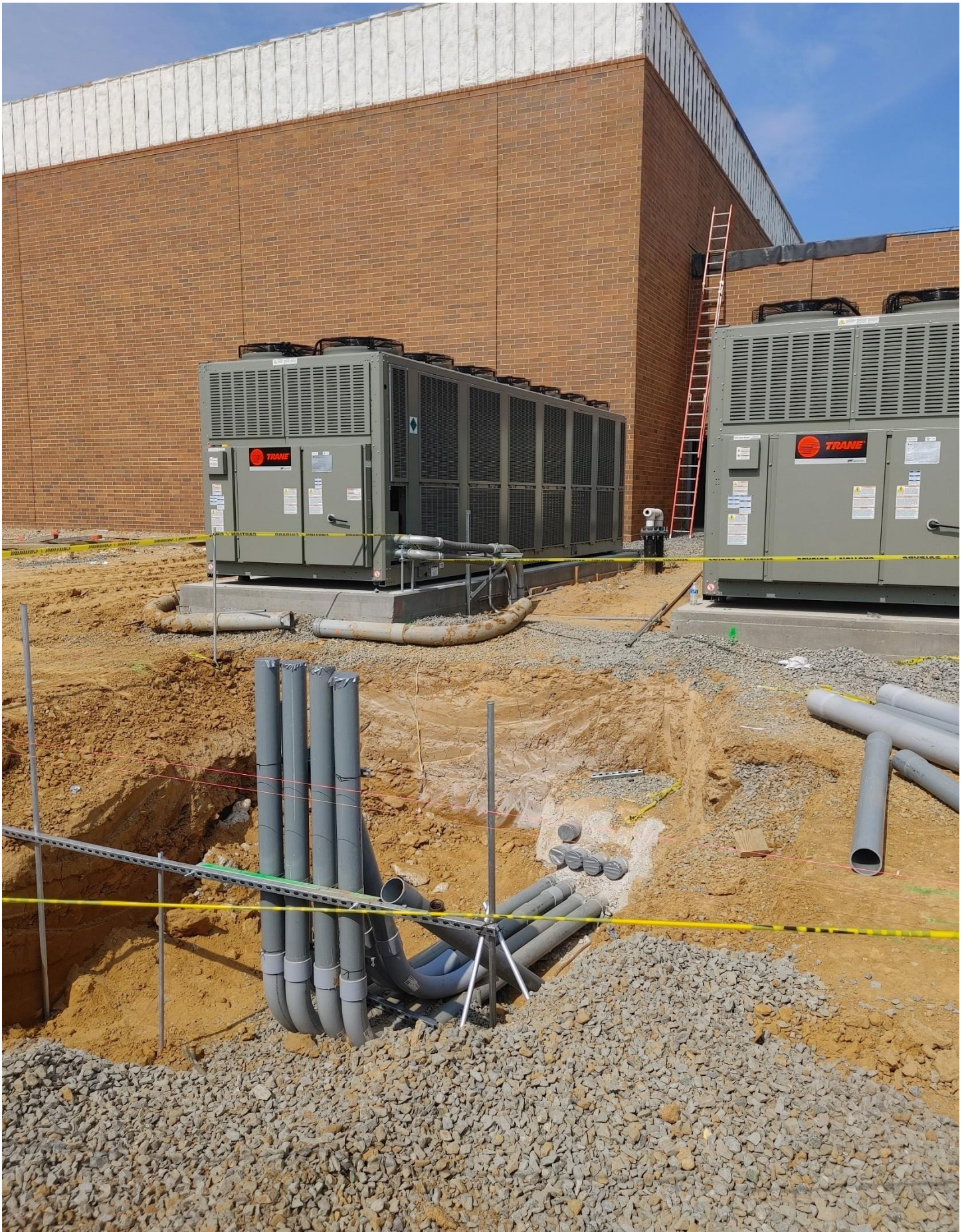
Photo 5 - Excavation and preparation for Dominion Power's Transformer continues
