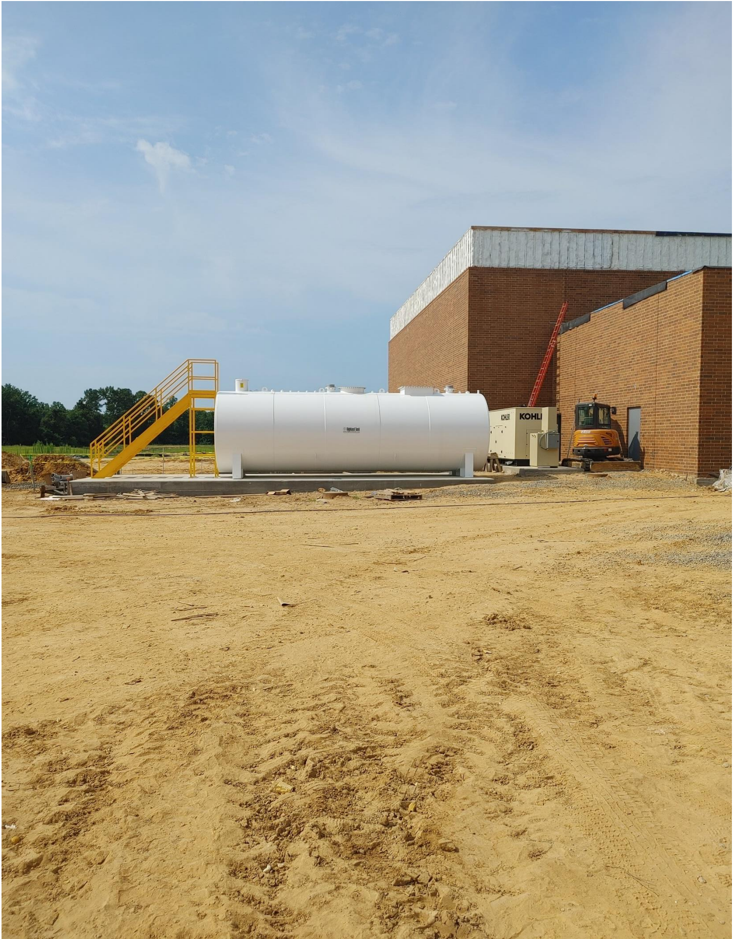
Photo 3 - Fuel Tank has been set
