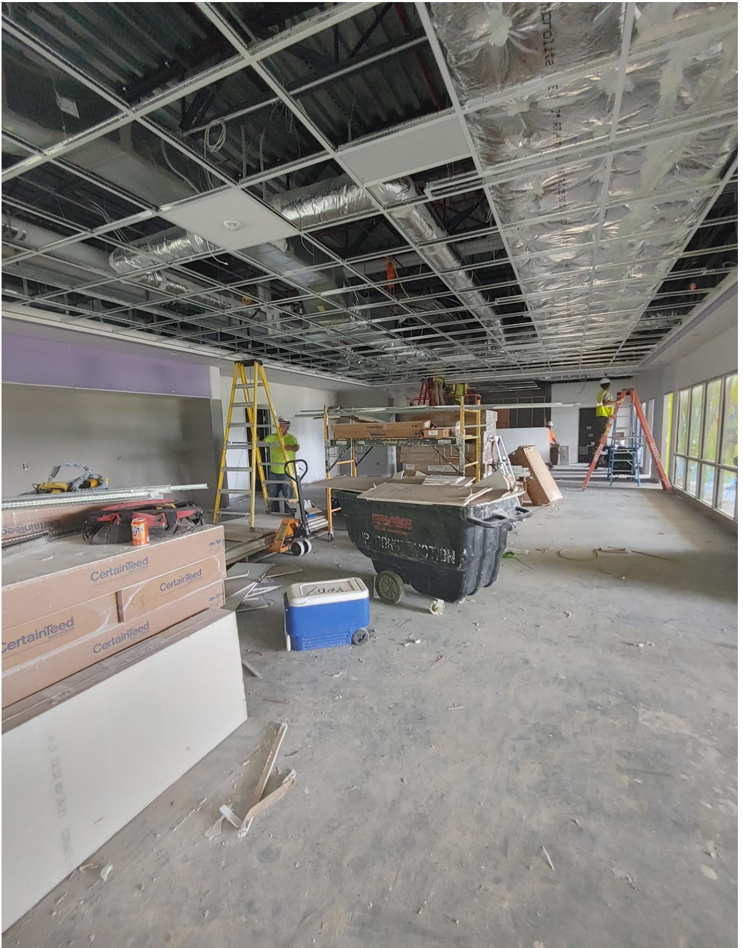
Photo 7 - Sheetrock is being hung around Bulkhead in Area A
