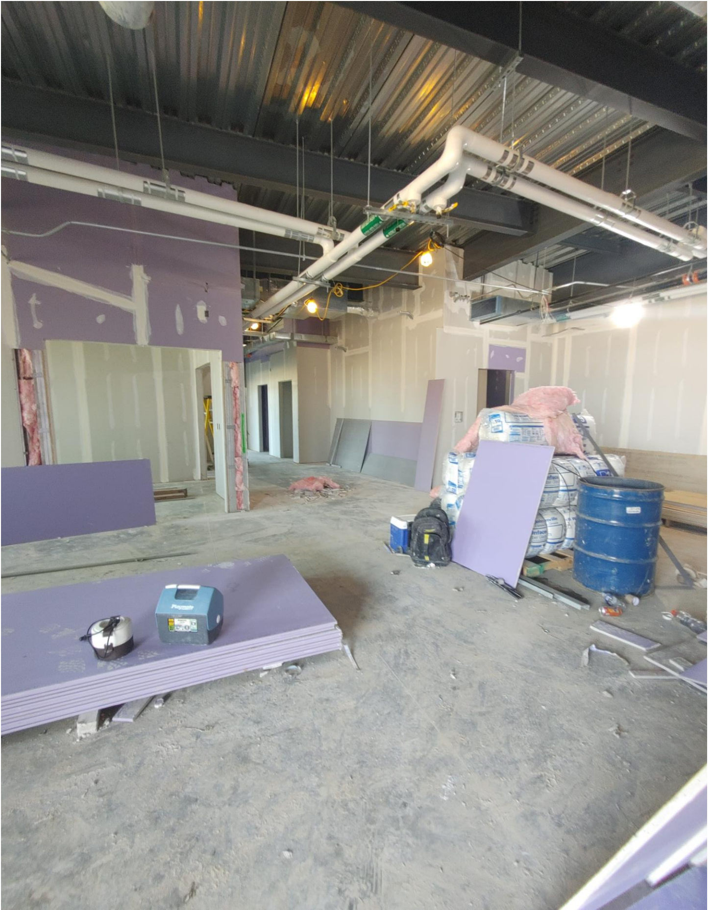
Photo 4 - Sheetrock continues to be hung and finished in Area A.
