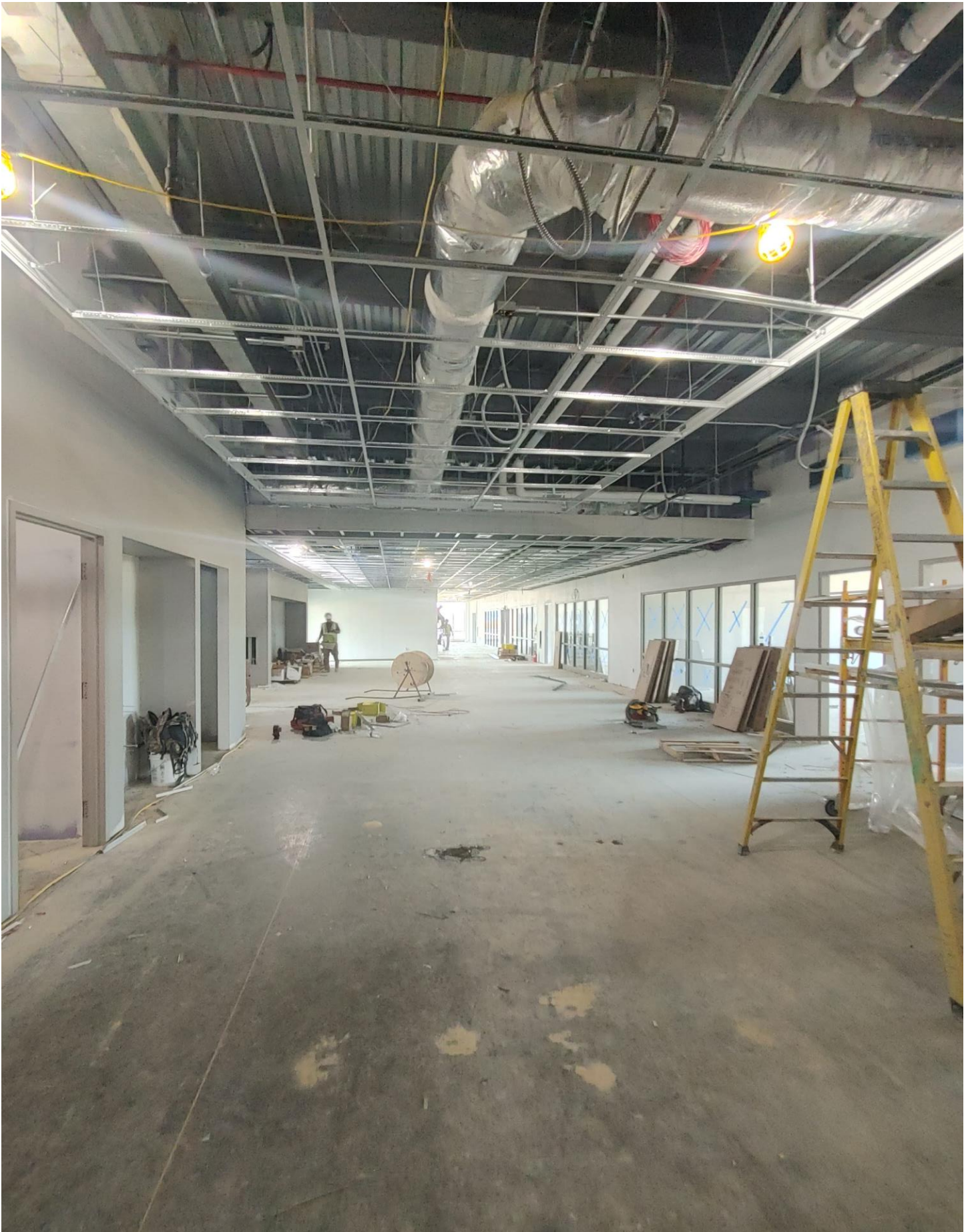
Photo 5 - Ceiling Grid is being installed in Area B
