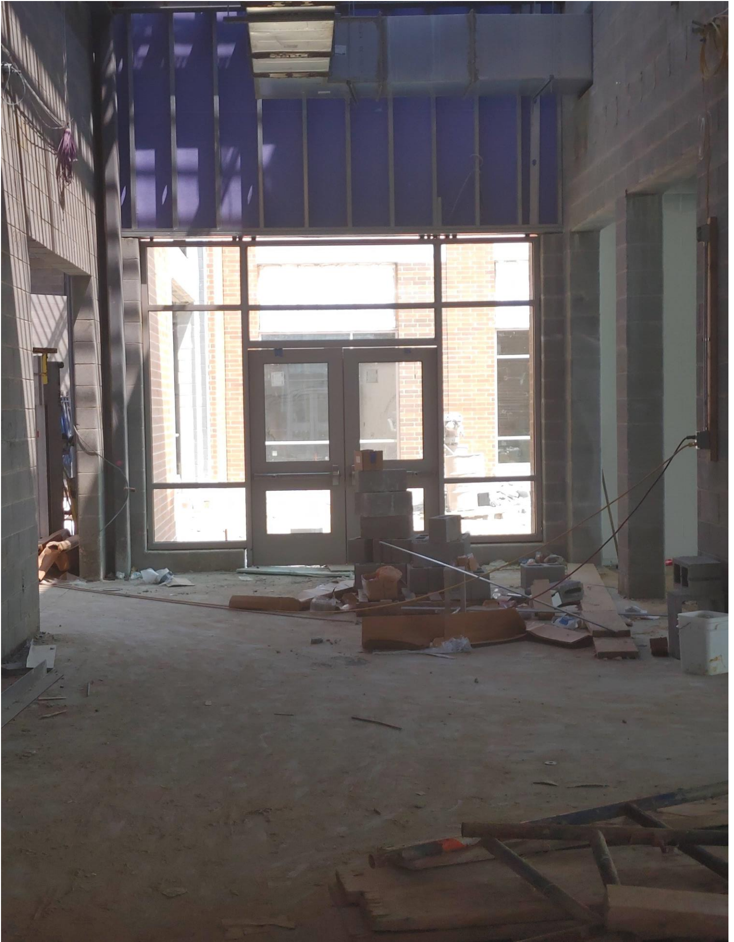
Photo 2 - Glass has been installed in Storefront #20, Area E
