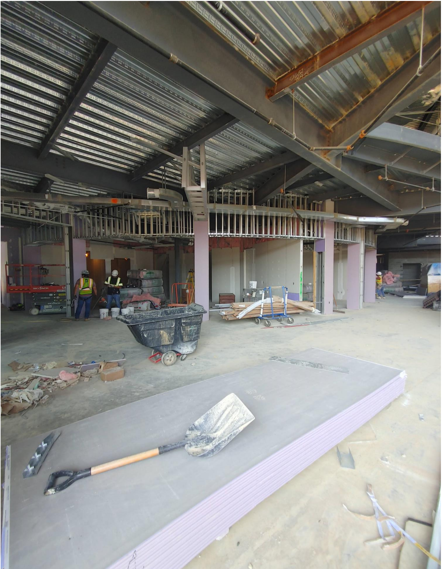
Photo 1 - Arched Bulkhead completed on the 1st floor of Area A
