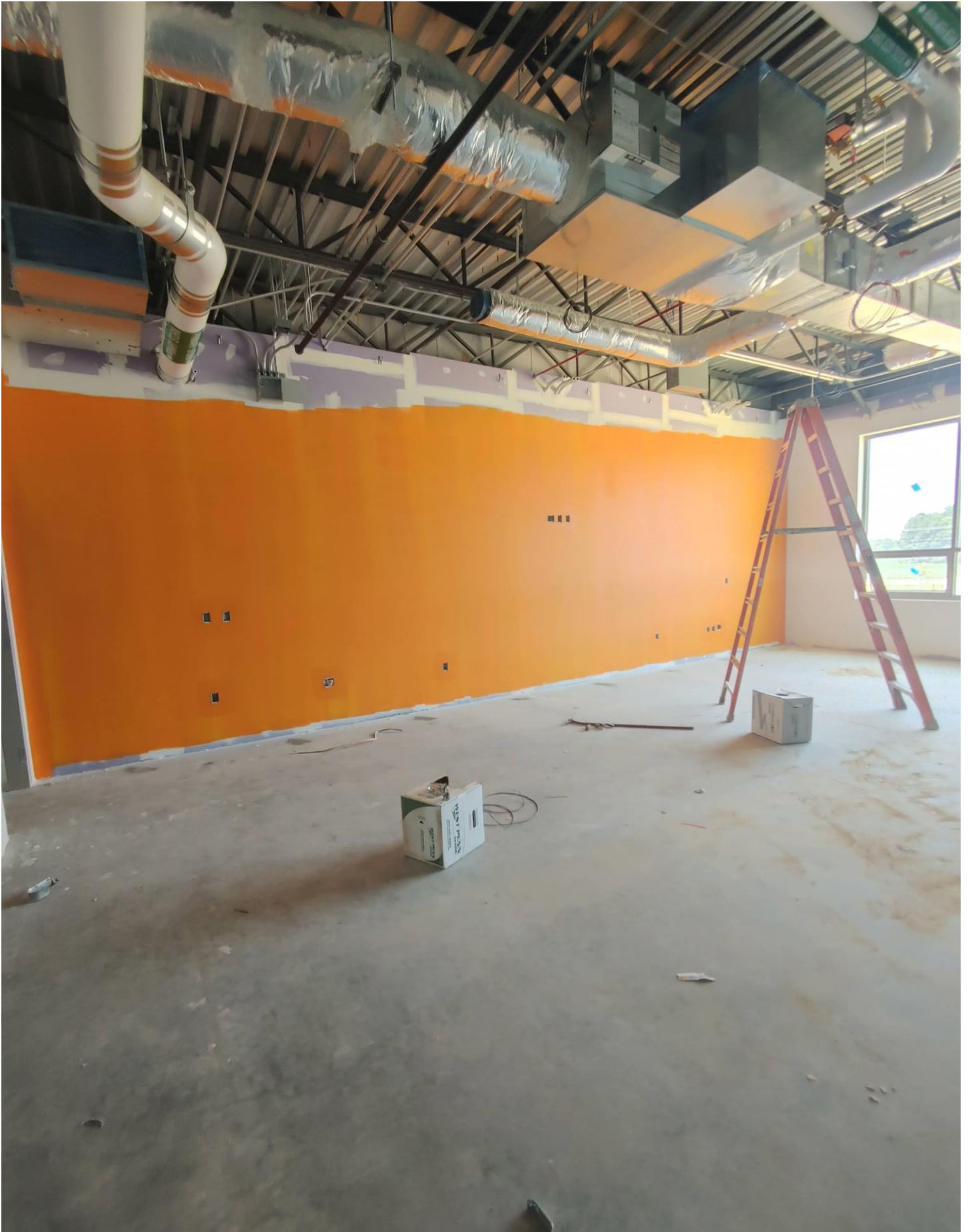
Photo 6 - Accent walls are being painted in Area B
