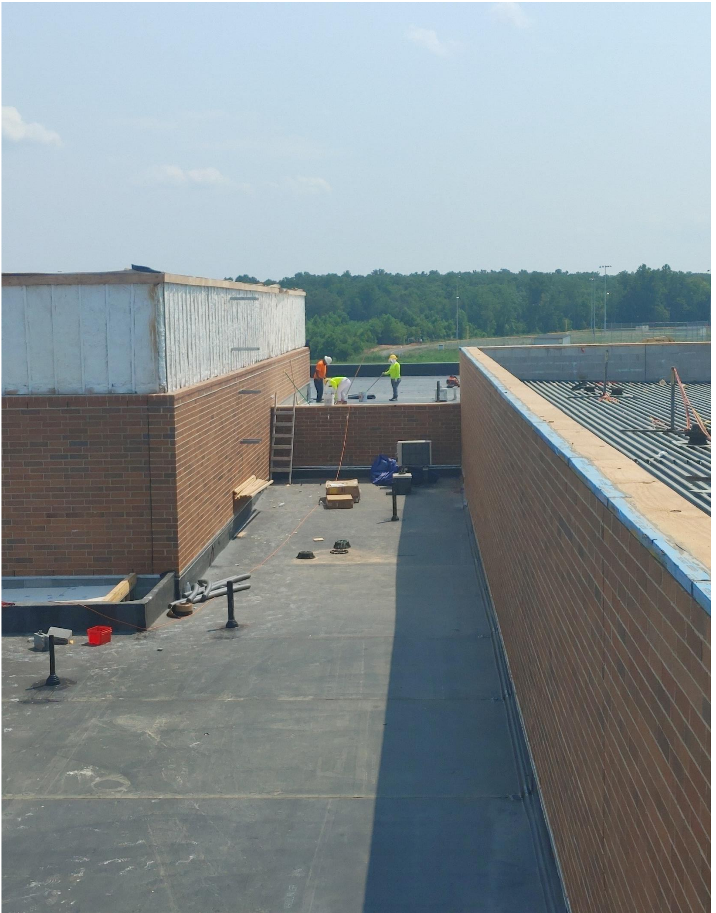
Photo 8 - Roofers working on low roof of Area D
