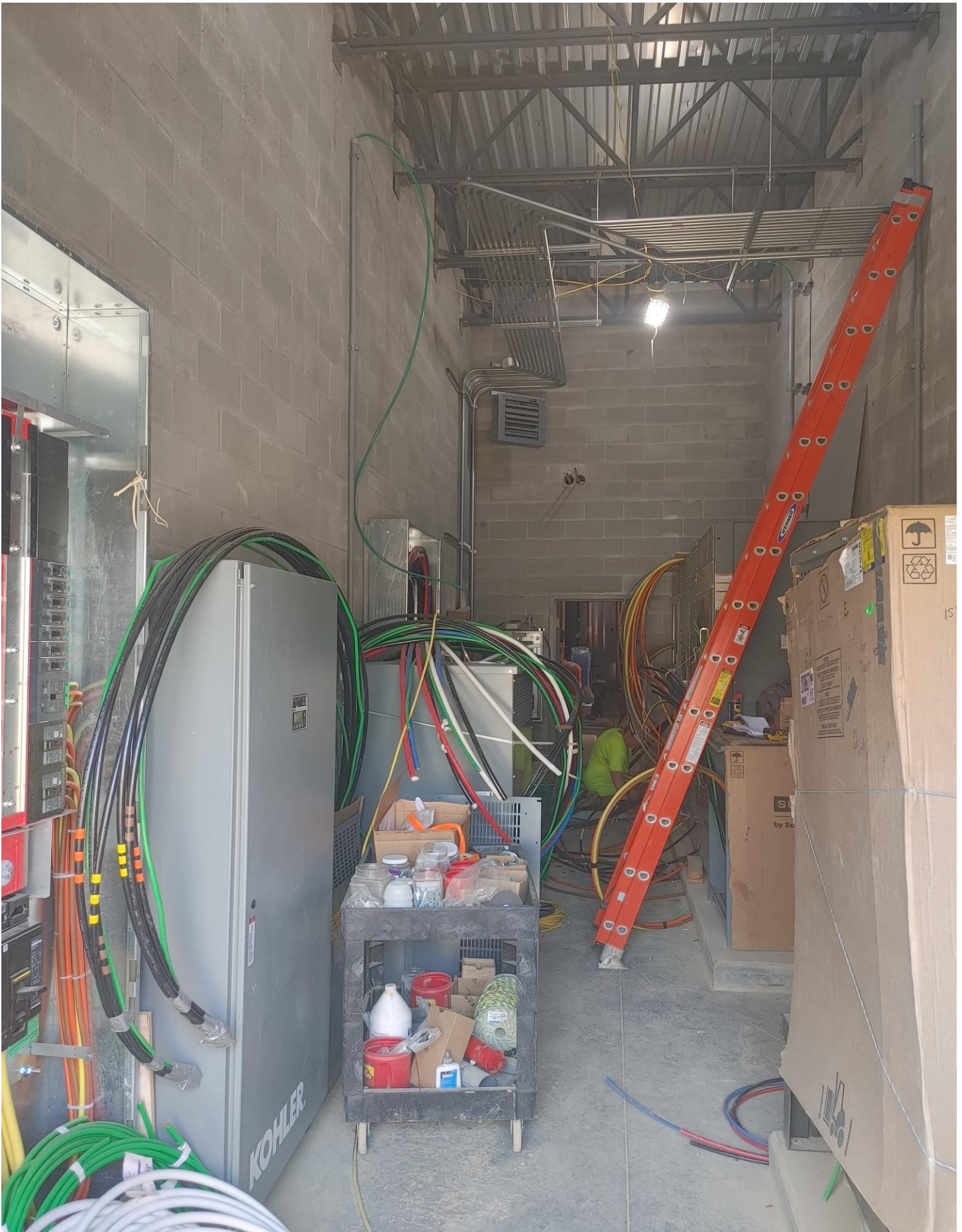
Photo 3 - Wire continues to be pulled into Electrical Room D158
