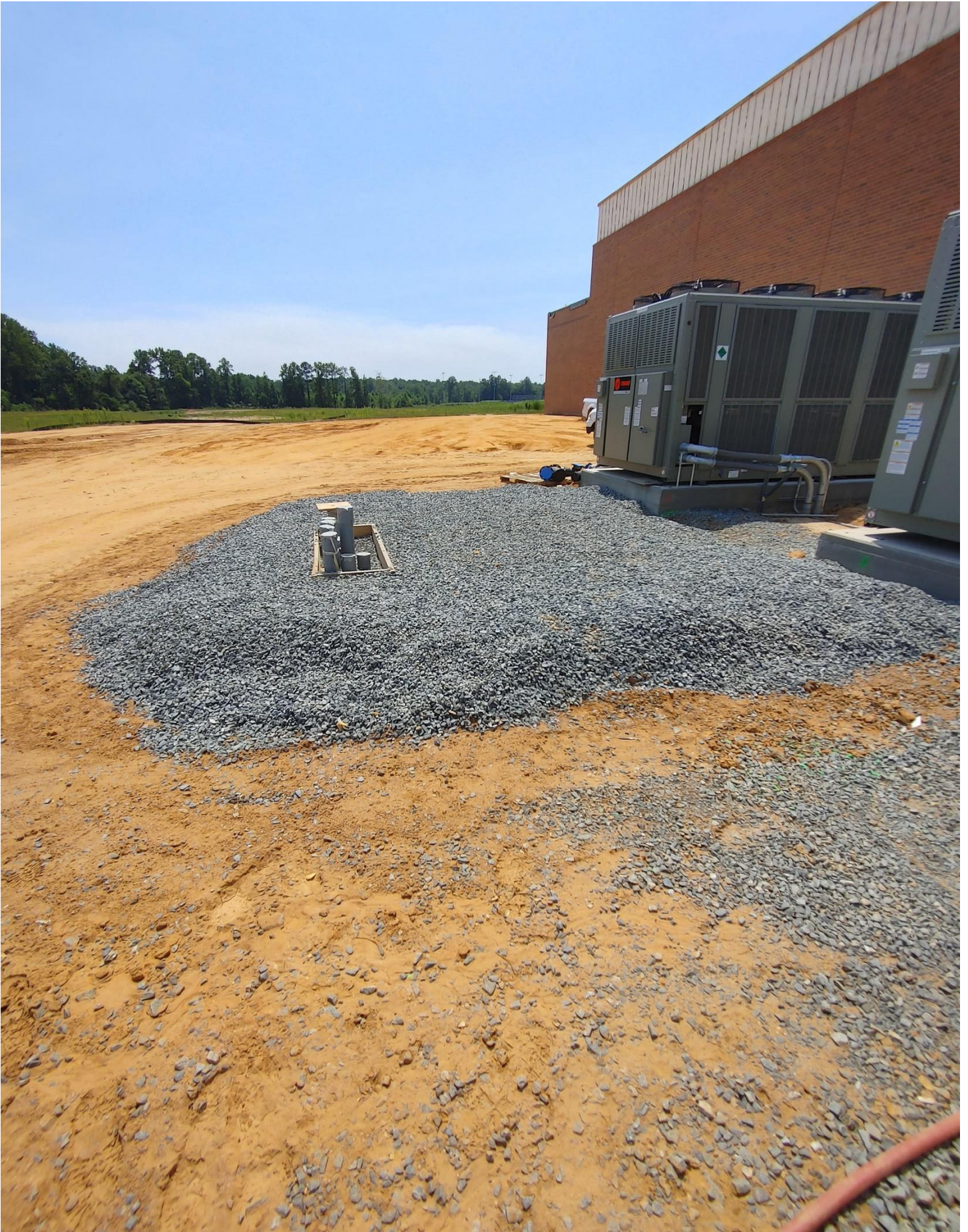
Photo 9 - Site prepped for Transformer Pad.
