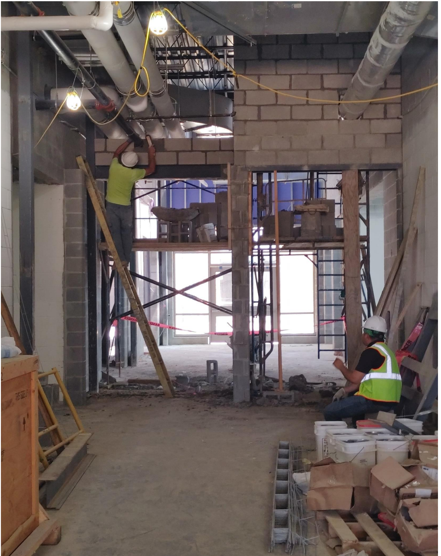
Photo 8 - Masons laying block in Corridor E11
