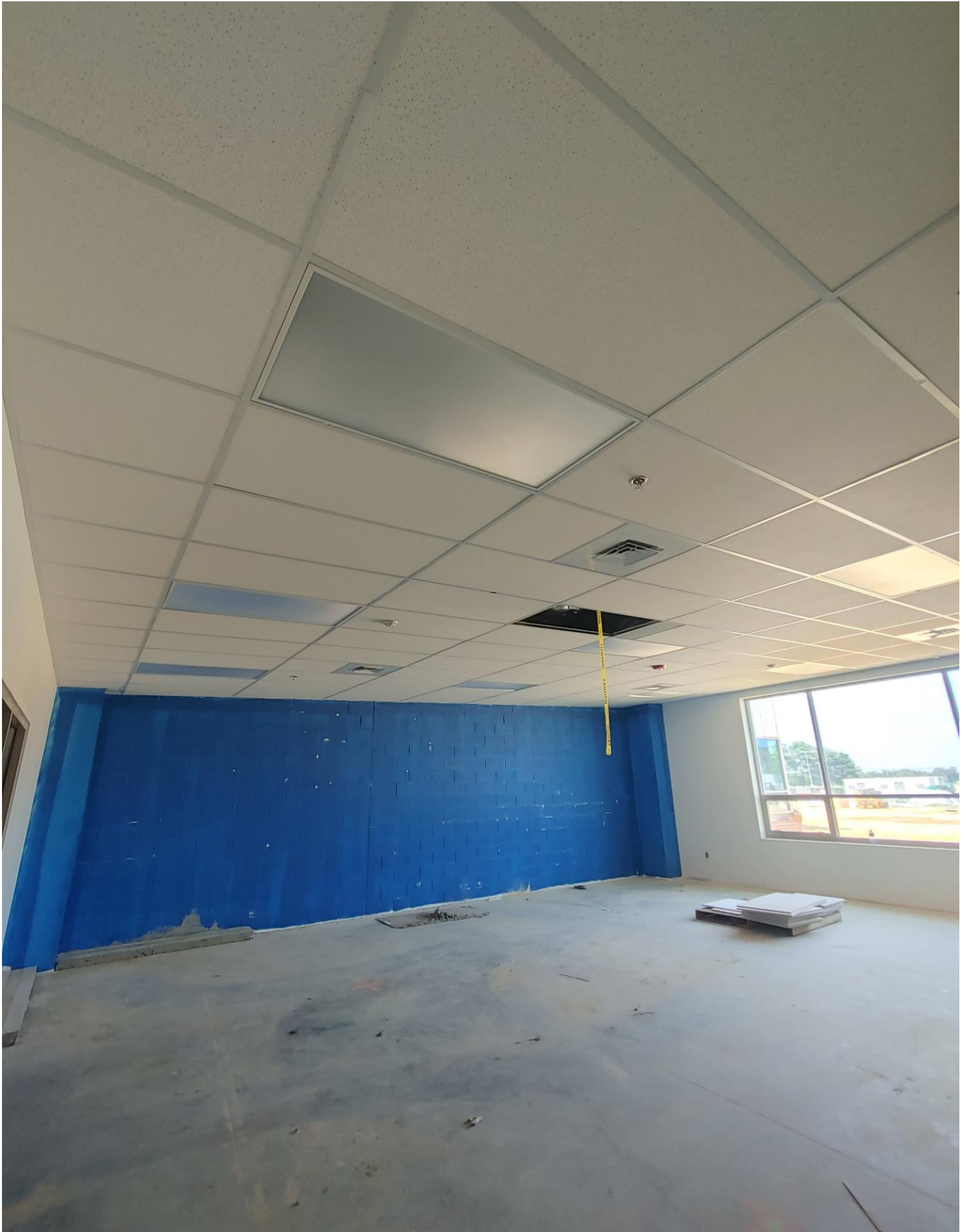
Photo 2 - They have begun to install Ceiling tiles in Area A
