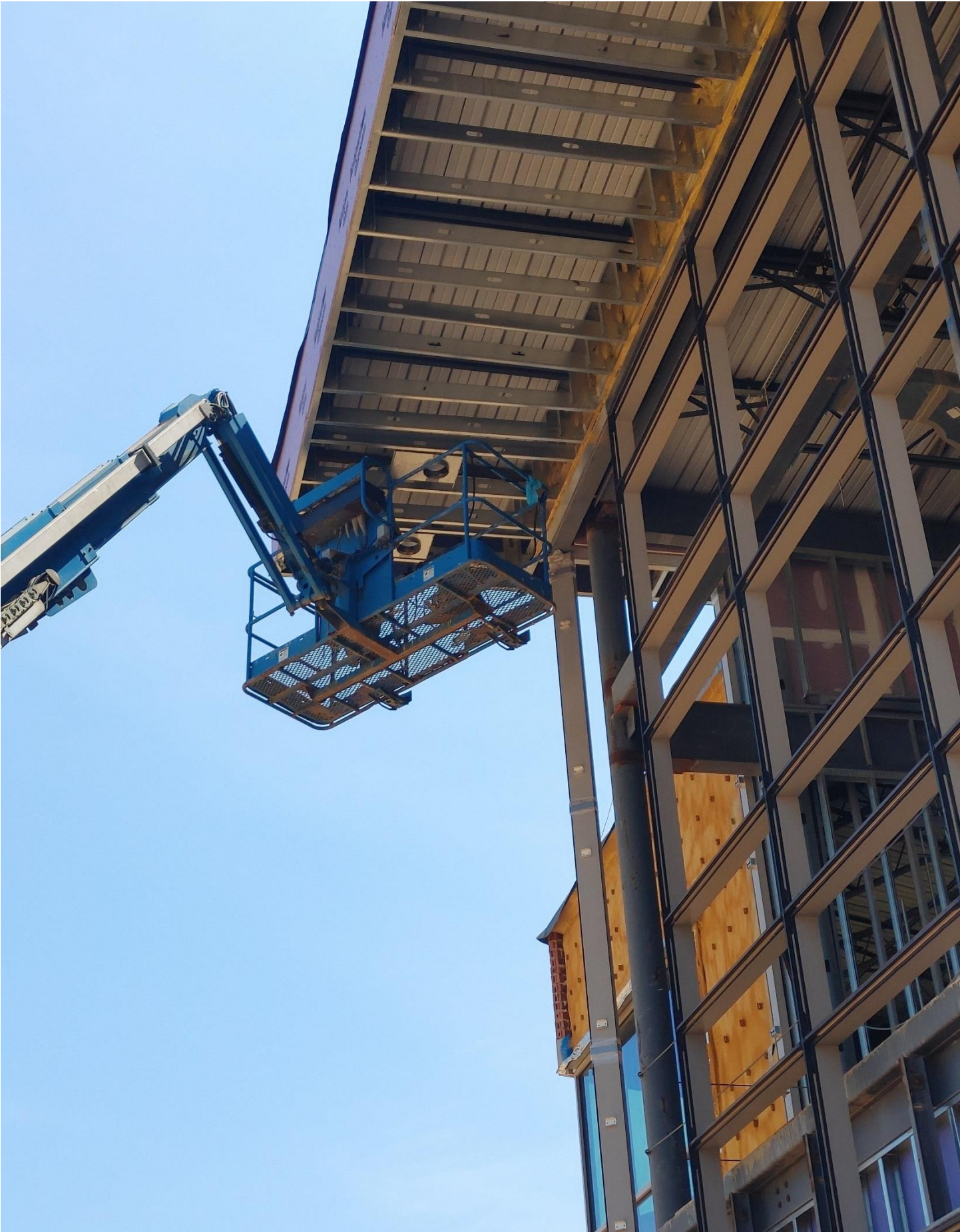
Photo 1 - Electricians are installing exterior lighting fixtures in Area A
