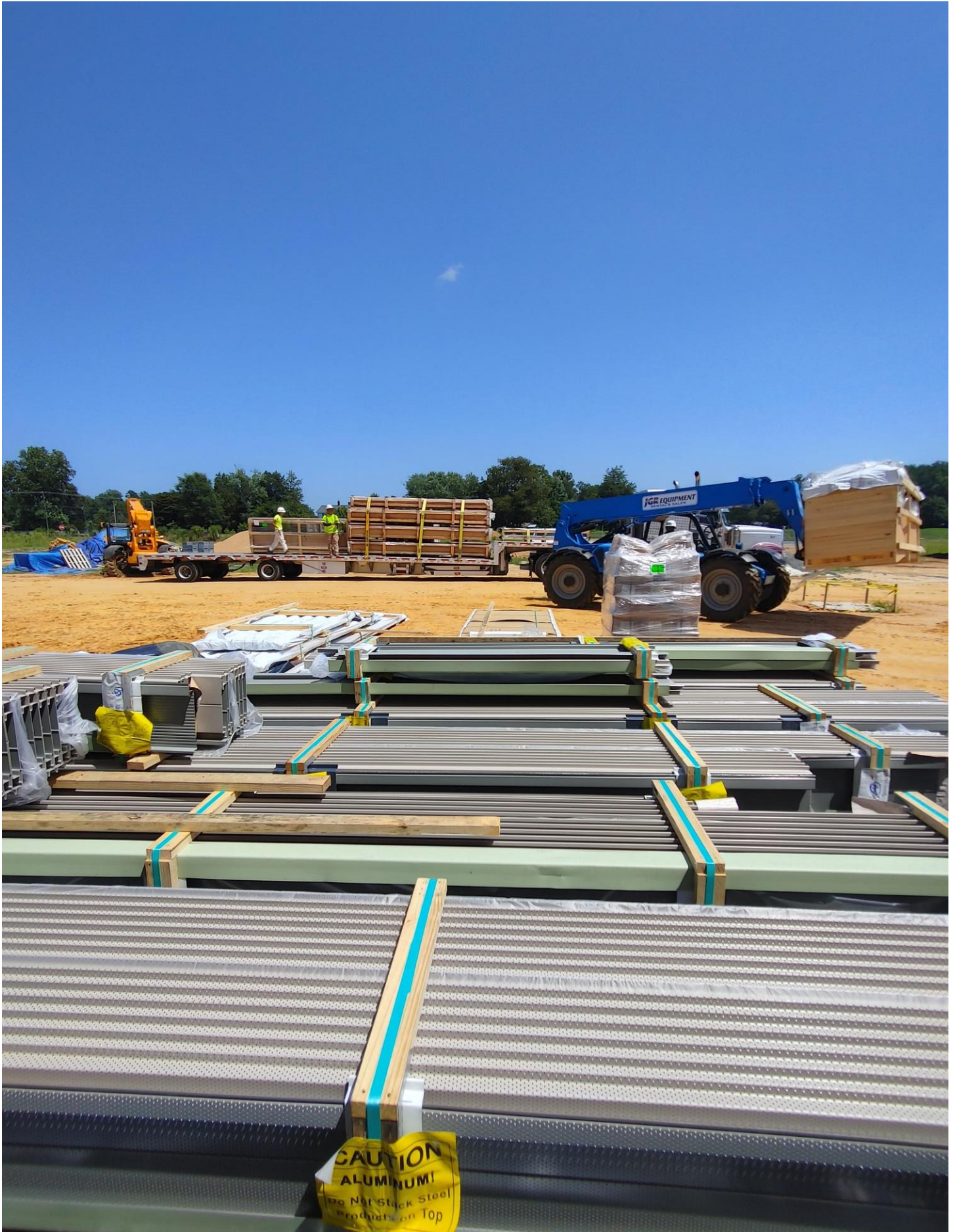
Photo 10 - Metal Panels are being off loaded and staged.
