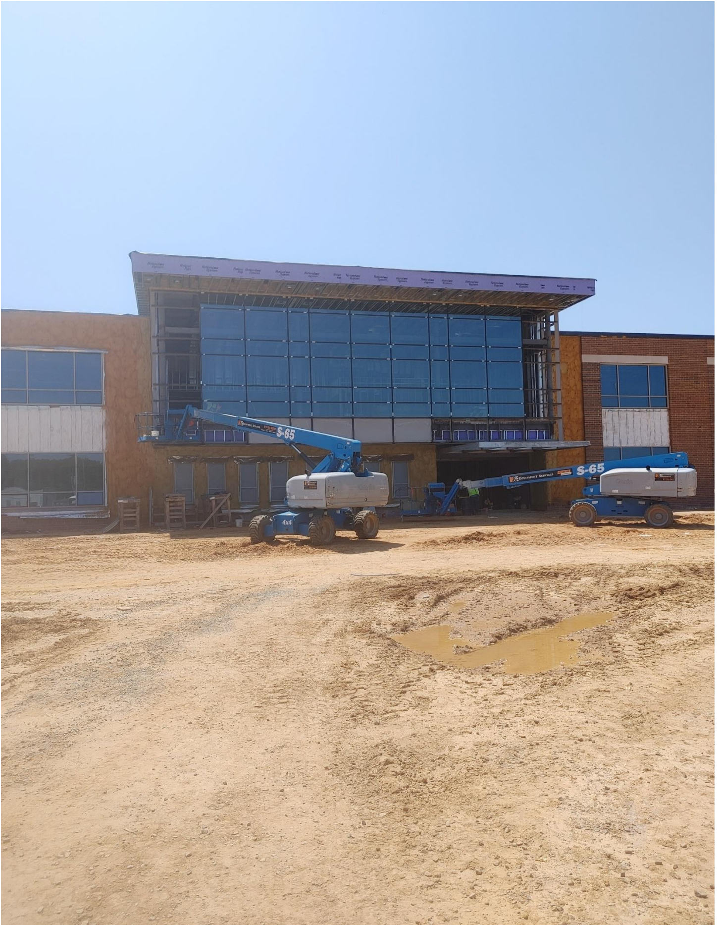
Photo 1 - Glass is being installed on the front of Area A
