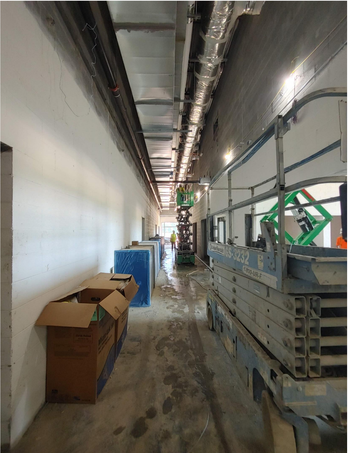
Photo 8 - HVAC duct is being installed in Area D
