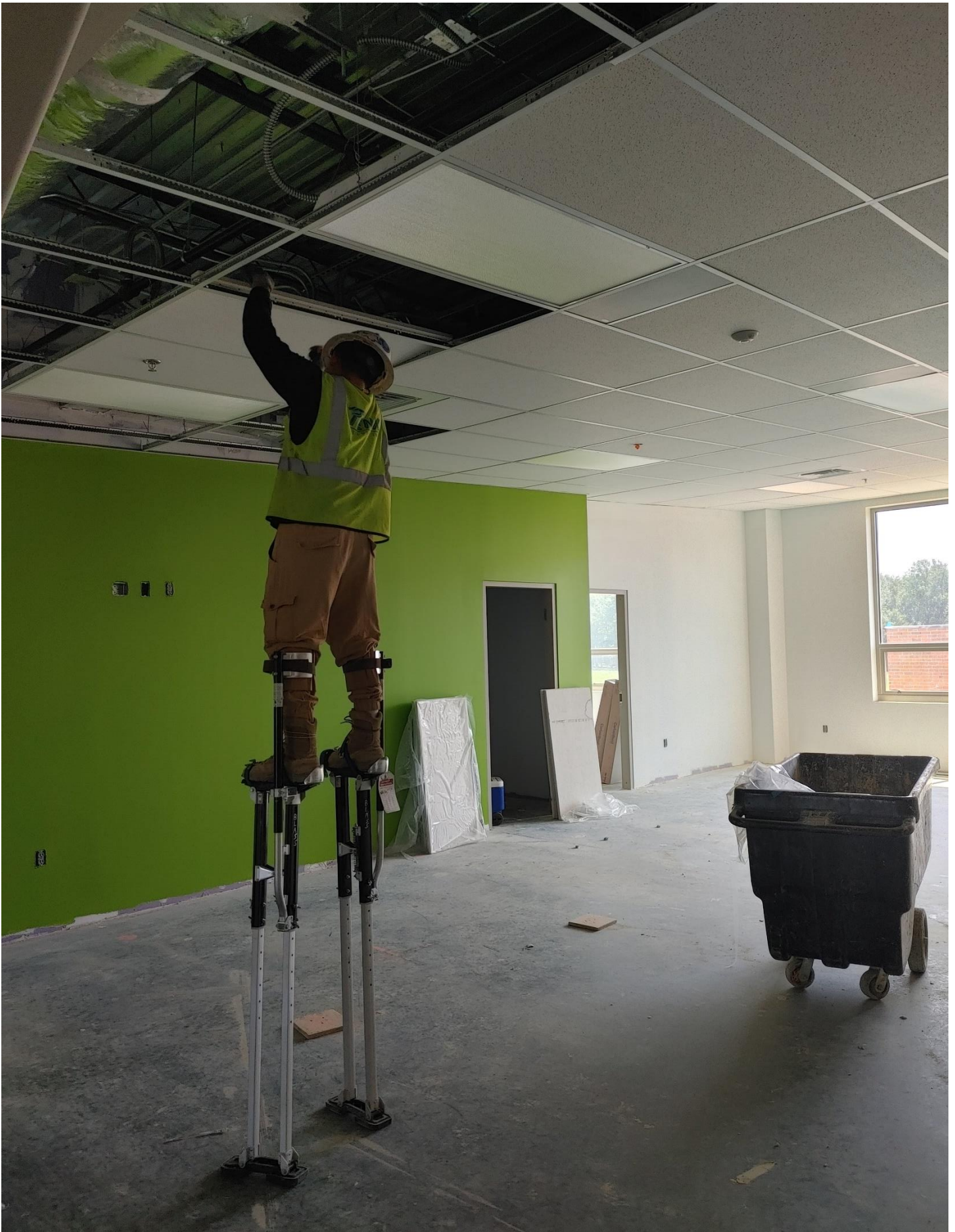
Photo 3 - Acoustical Ceiling tiles are being installed in Area A
