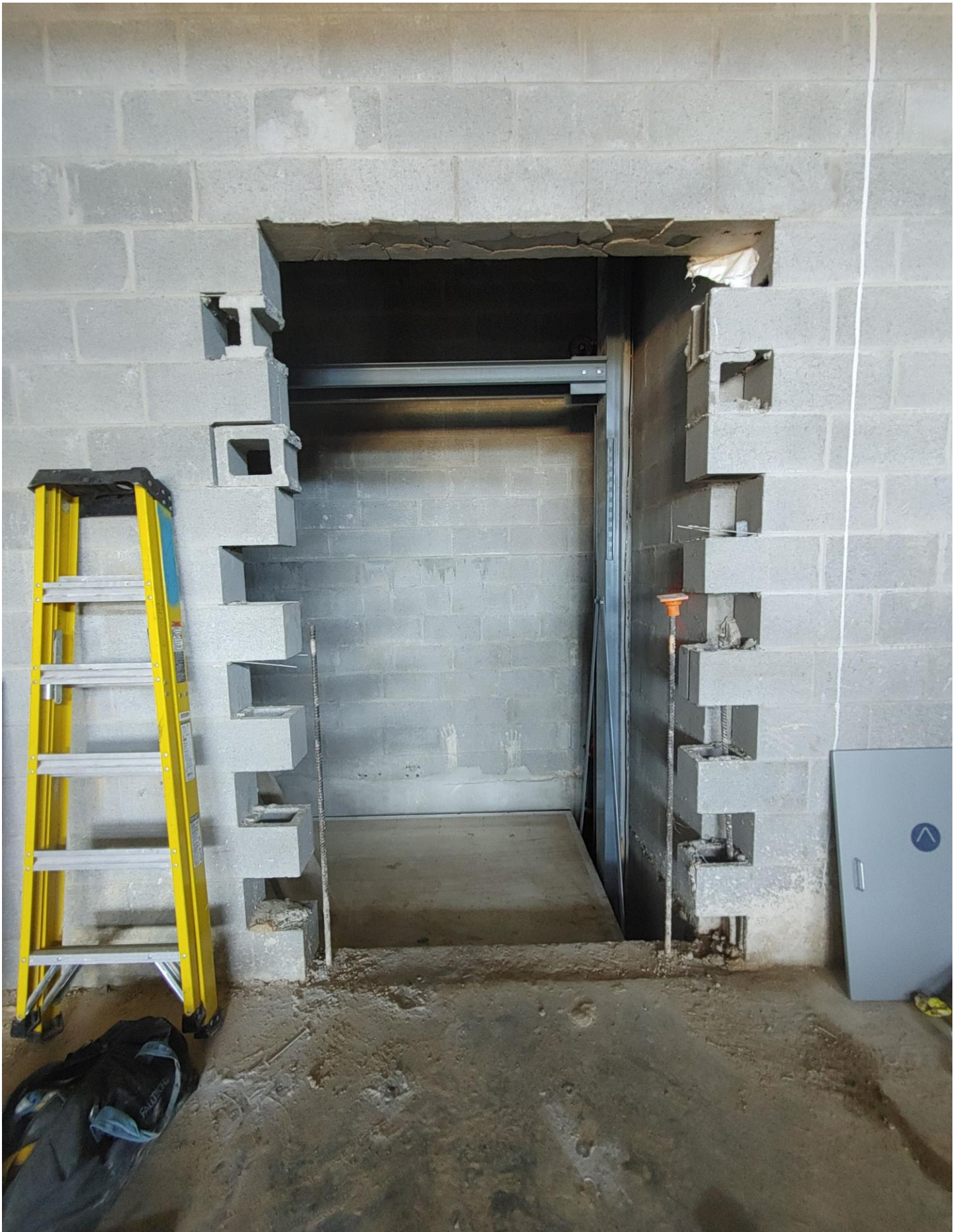
Photo 2 - They have begun to install the elevator
