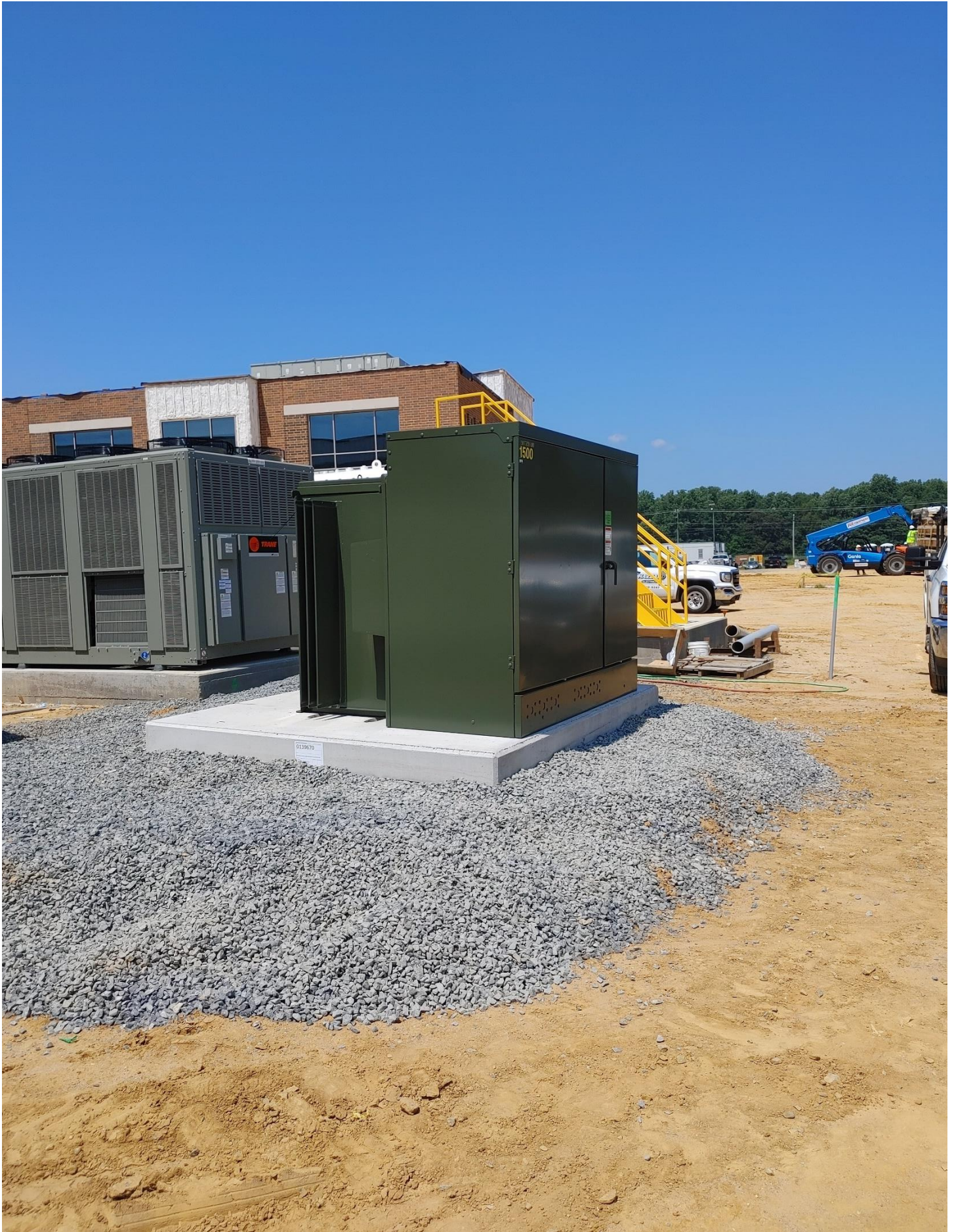
Photo 9 - Dominion Power Transformer has been set
