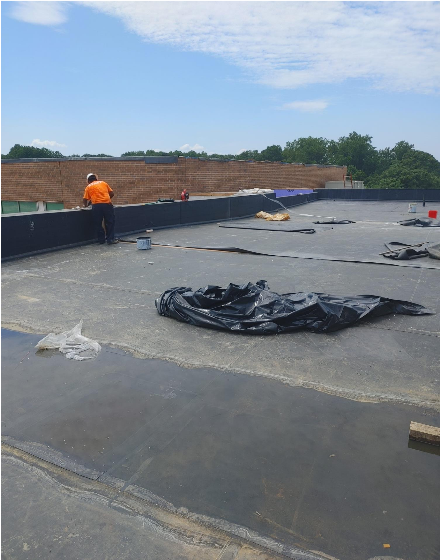
Photo 4 Roofers working on Area C Roof.
