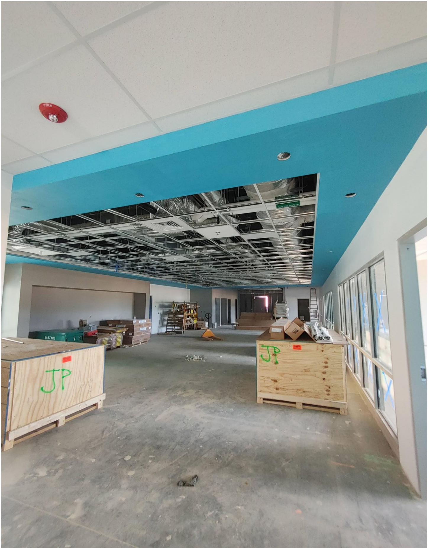
Photo 6 - Soffit has been painted in Area A.
