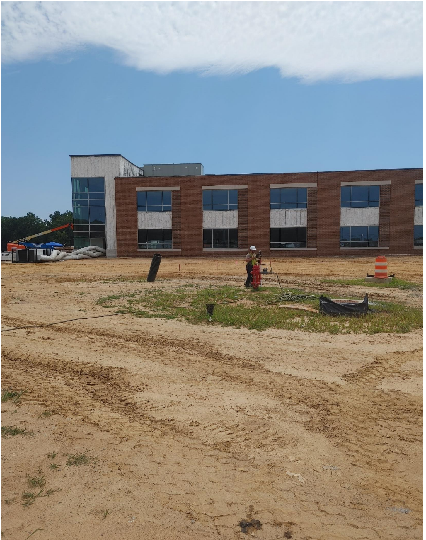
Photo 1 - Surveyors laying out reference points.
