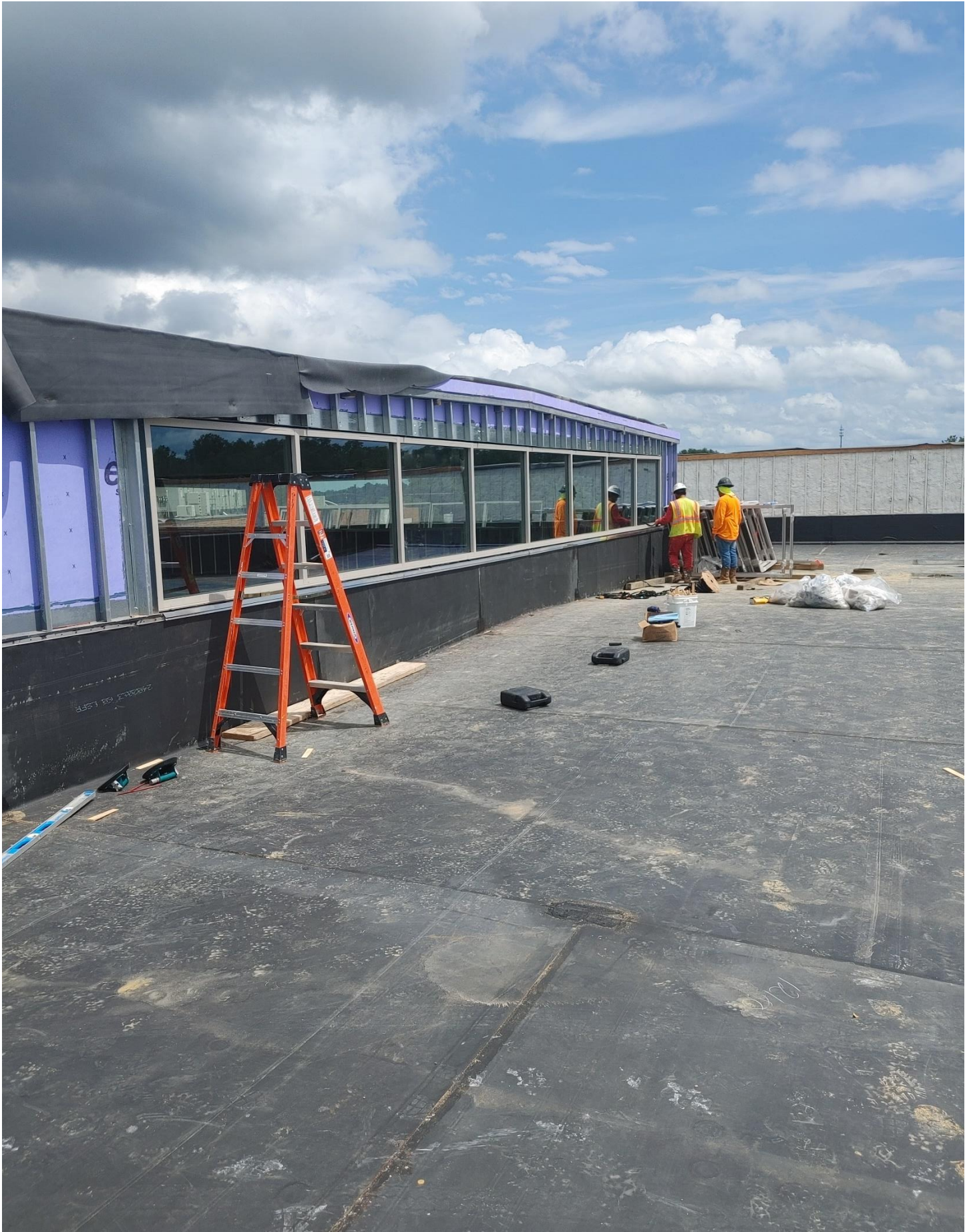
Photo 10 - Glass being installed in Storefront #17
