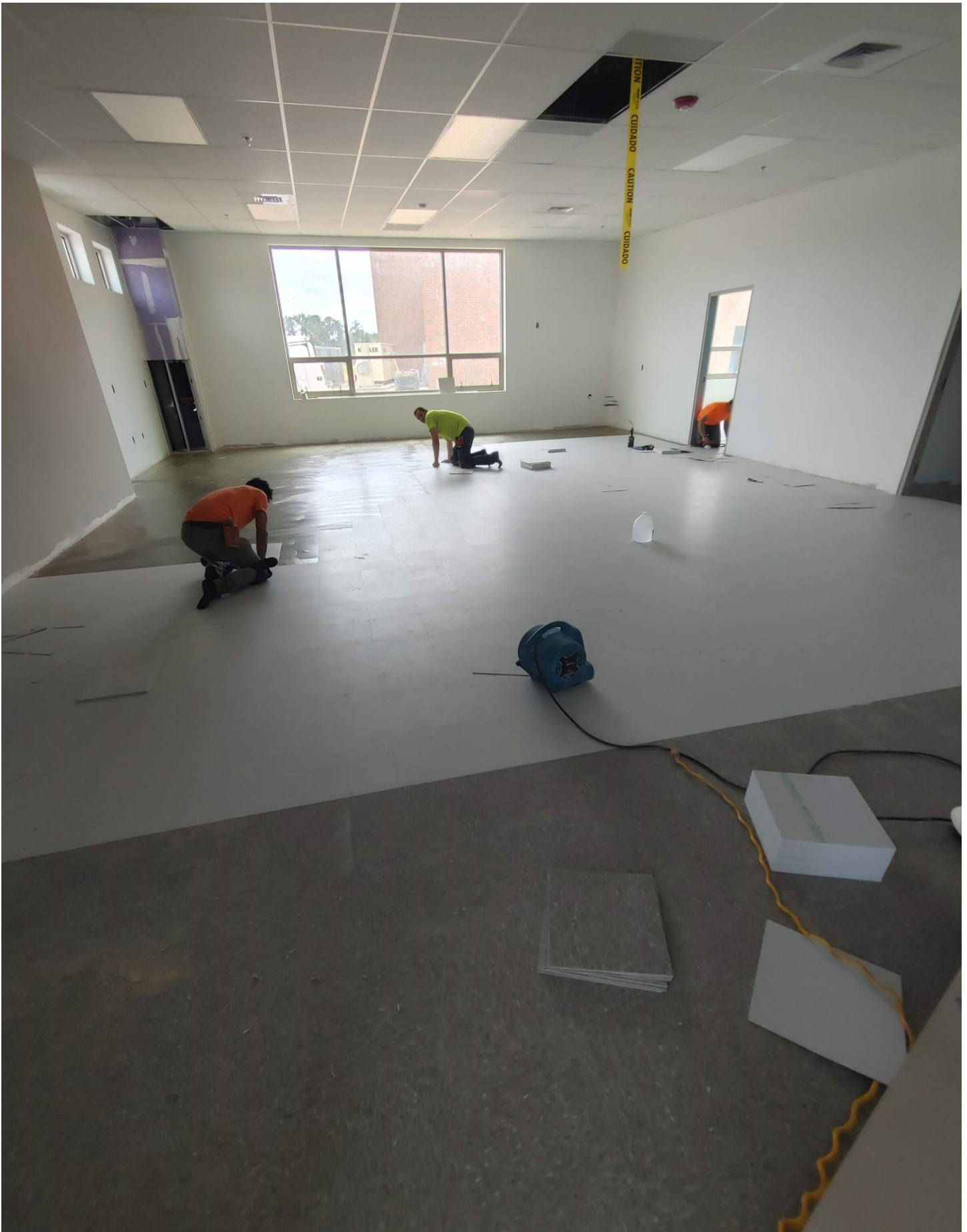
Photo 12 - VCT is being laid in A106
