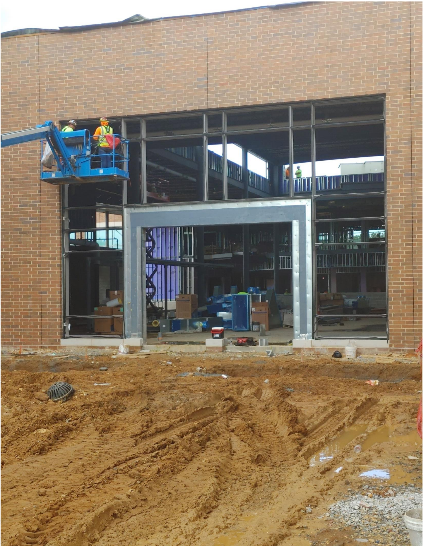
Photo 1 - Curtain Wall #1 is being installed
