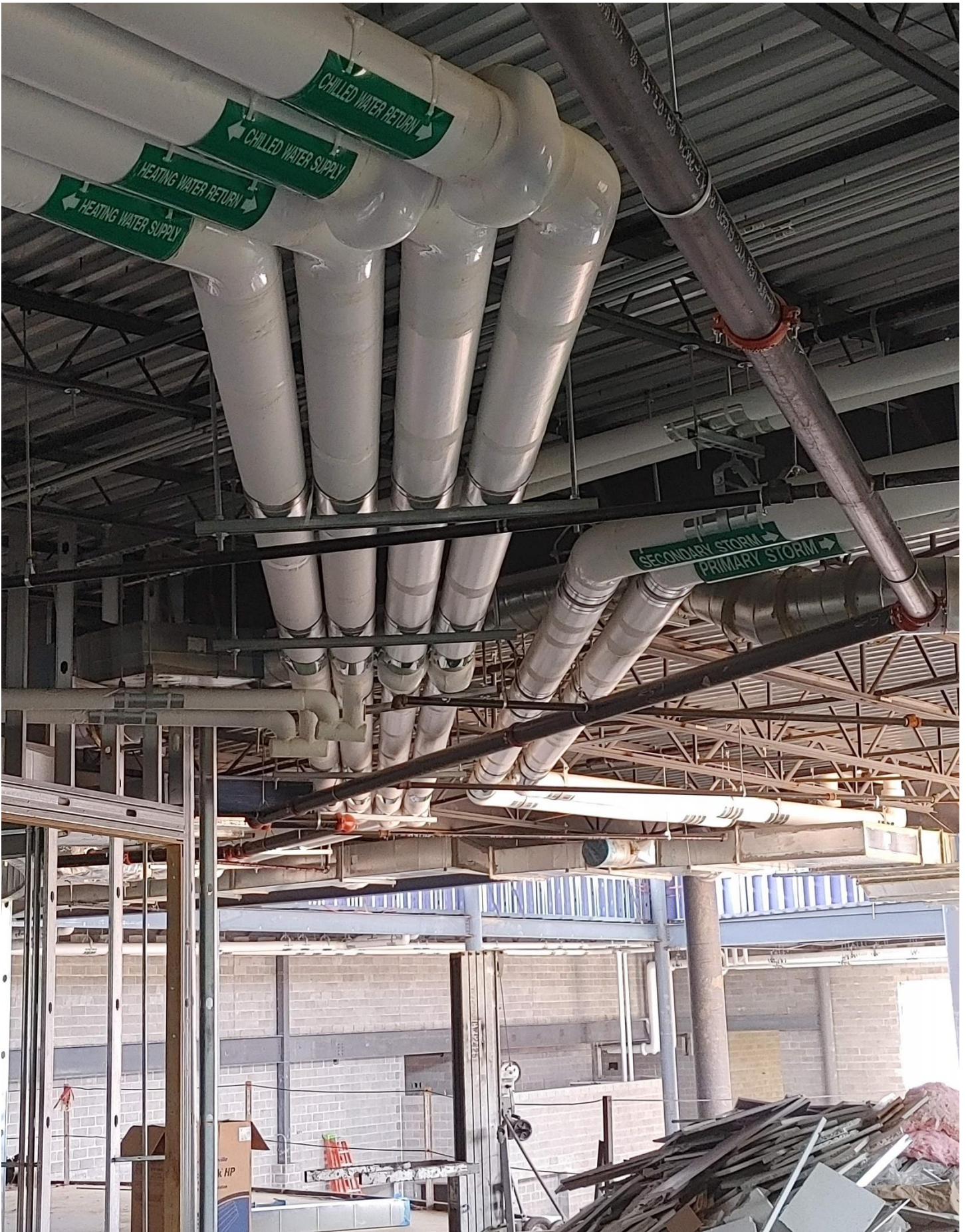
Photo 7 - Pipes are being labeled
