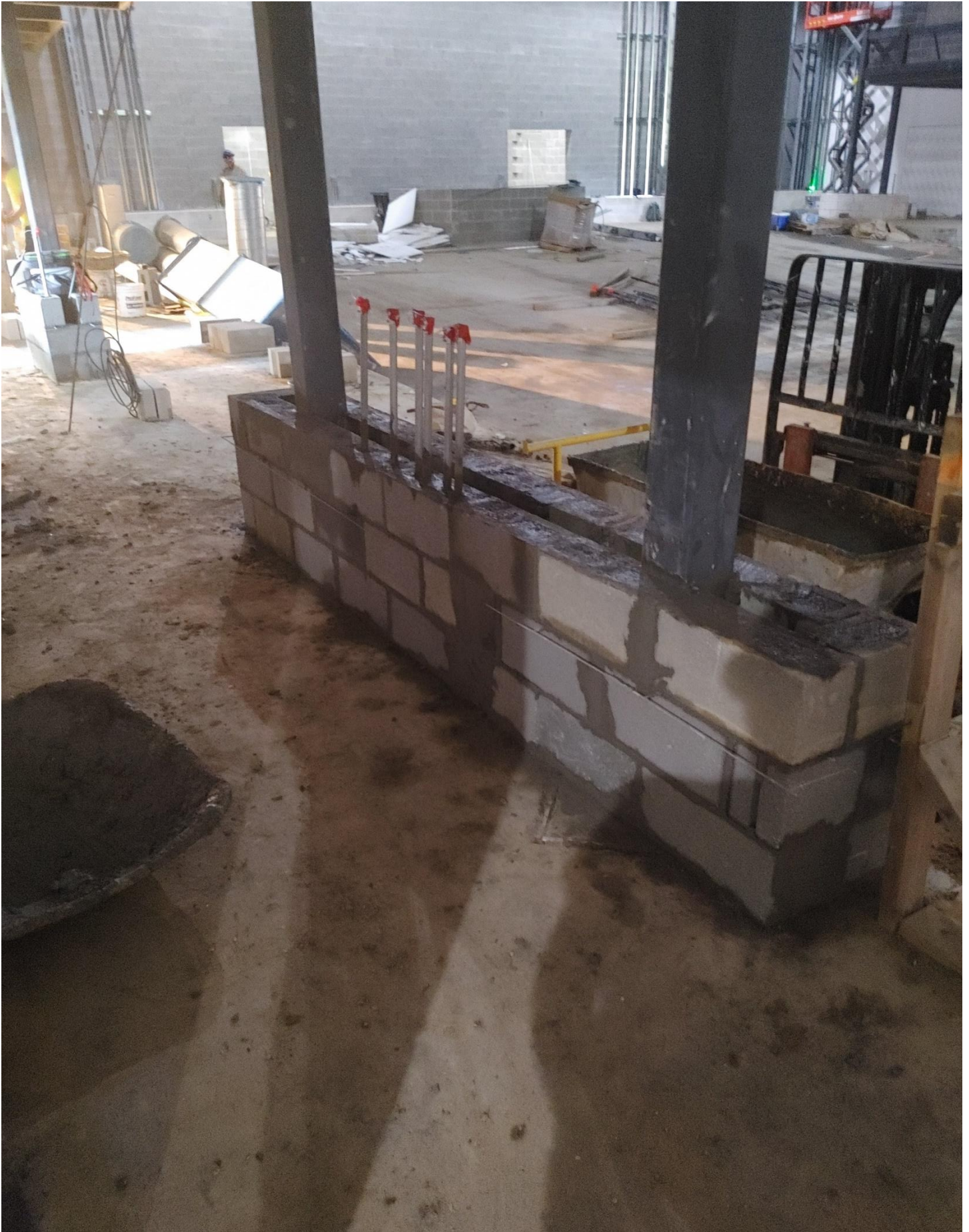
Photo 3 - Masons are laying block around columns in Auditorium.
