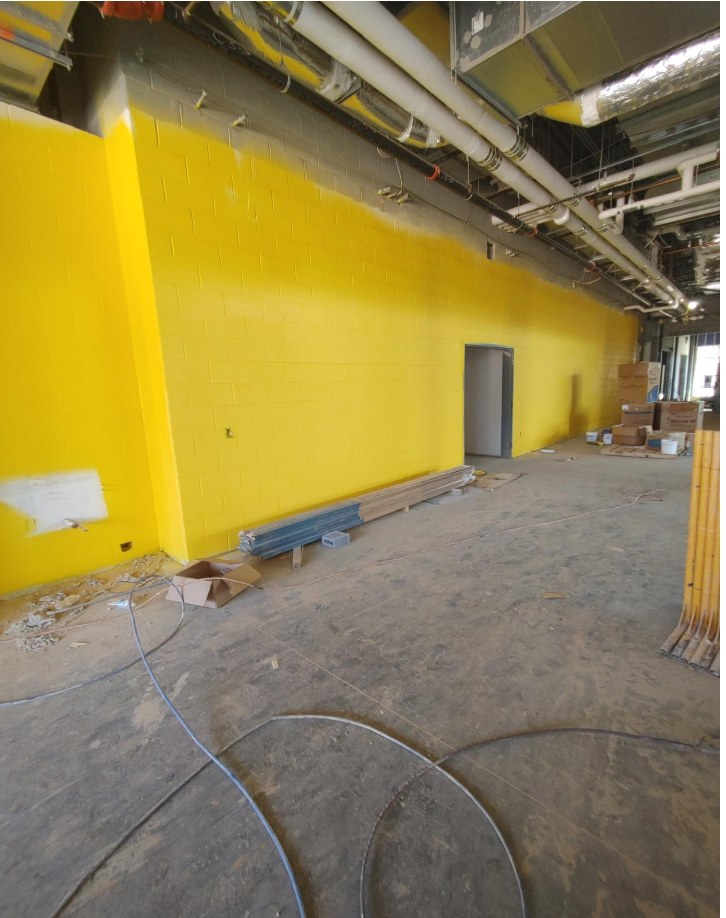
Photo 6 - Painters are working in Area E.
