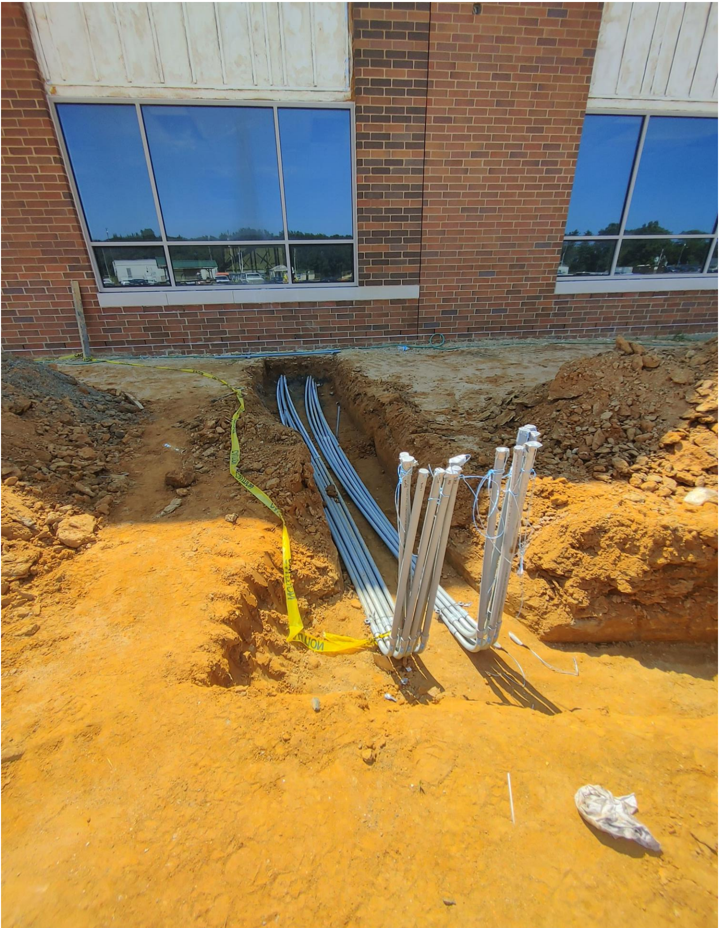
Photo 1 - Conduit for lighting stubbed up in front of Area A
