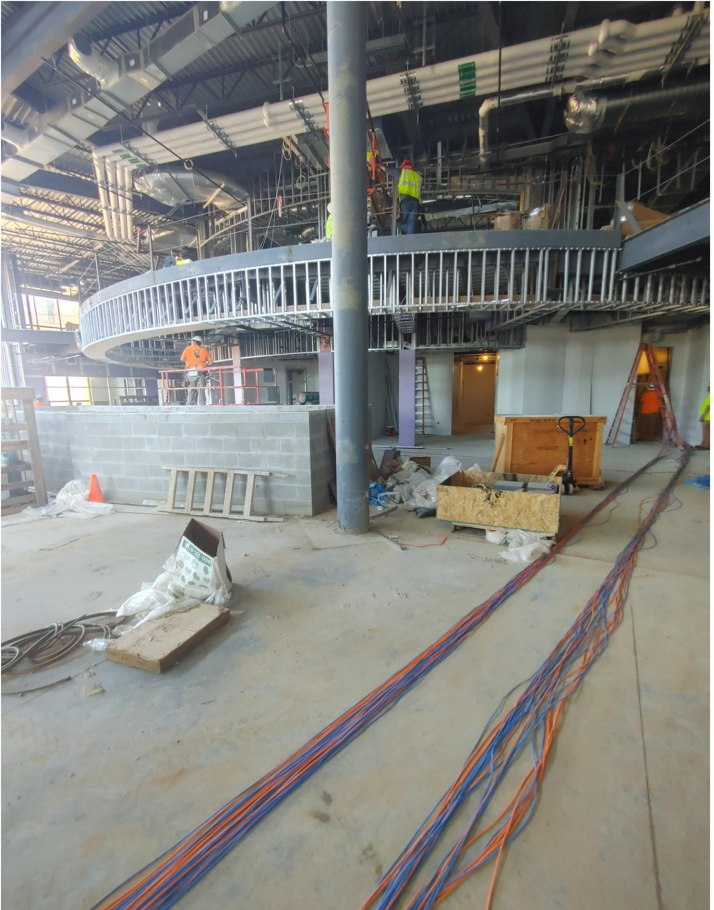
Photo 4 - Sheetrock is being hung on the radius bulkhead.
