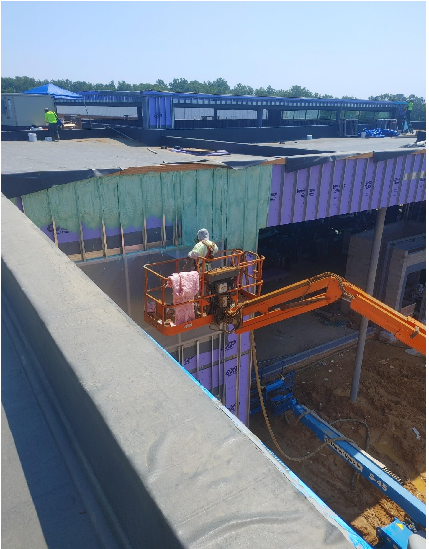
Photo 9 - Spray Foam being applied to the West side of Area C.
