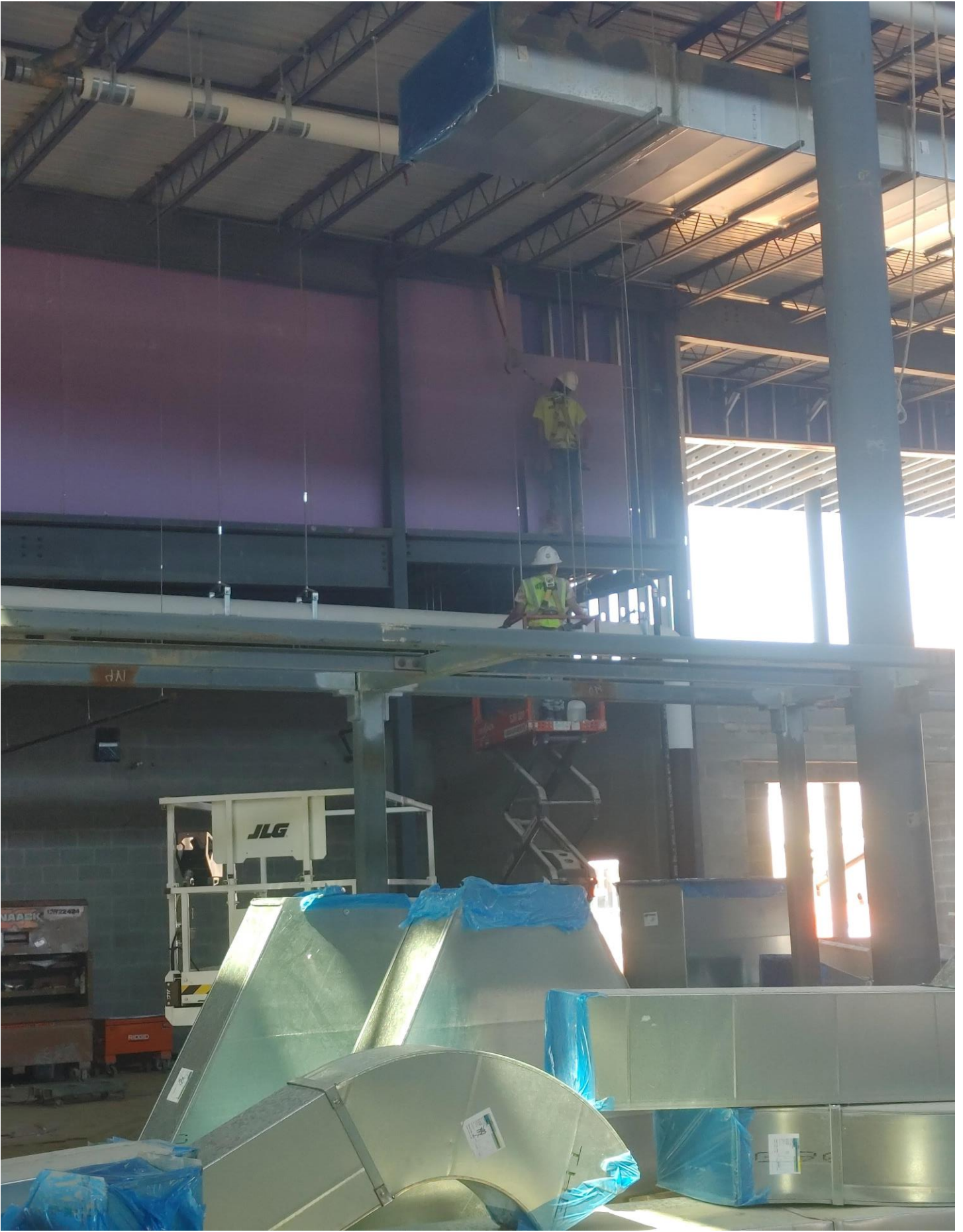
Photo 3 - Sheetrock is being hung in Area C.
