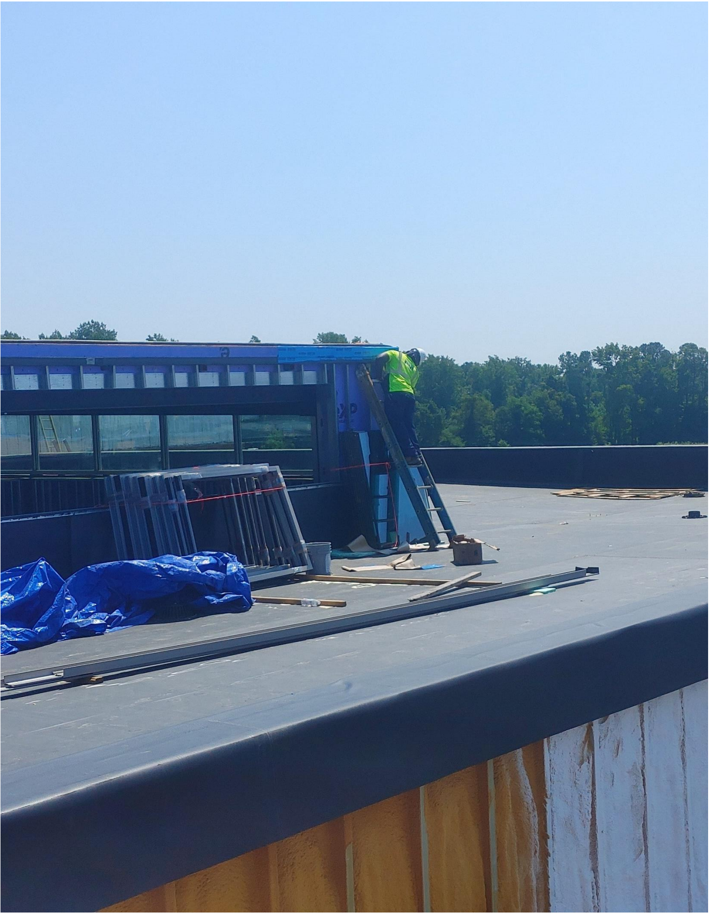
Photo 10 - Flashing being applied to the high roof of Area C.
