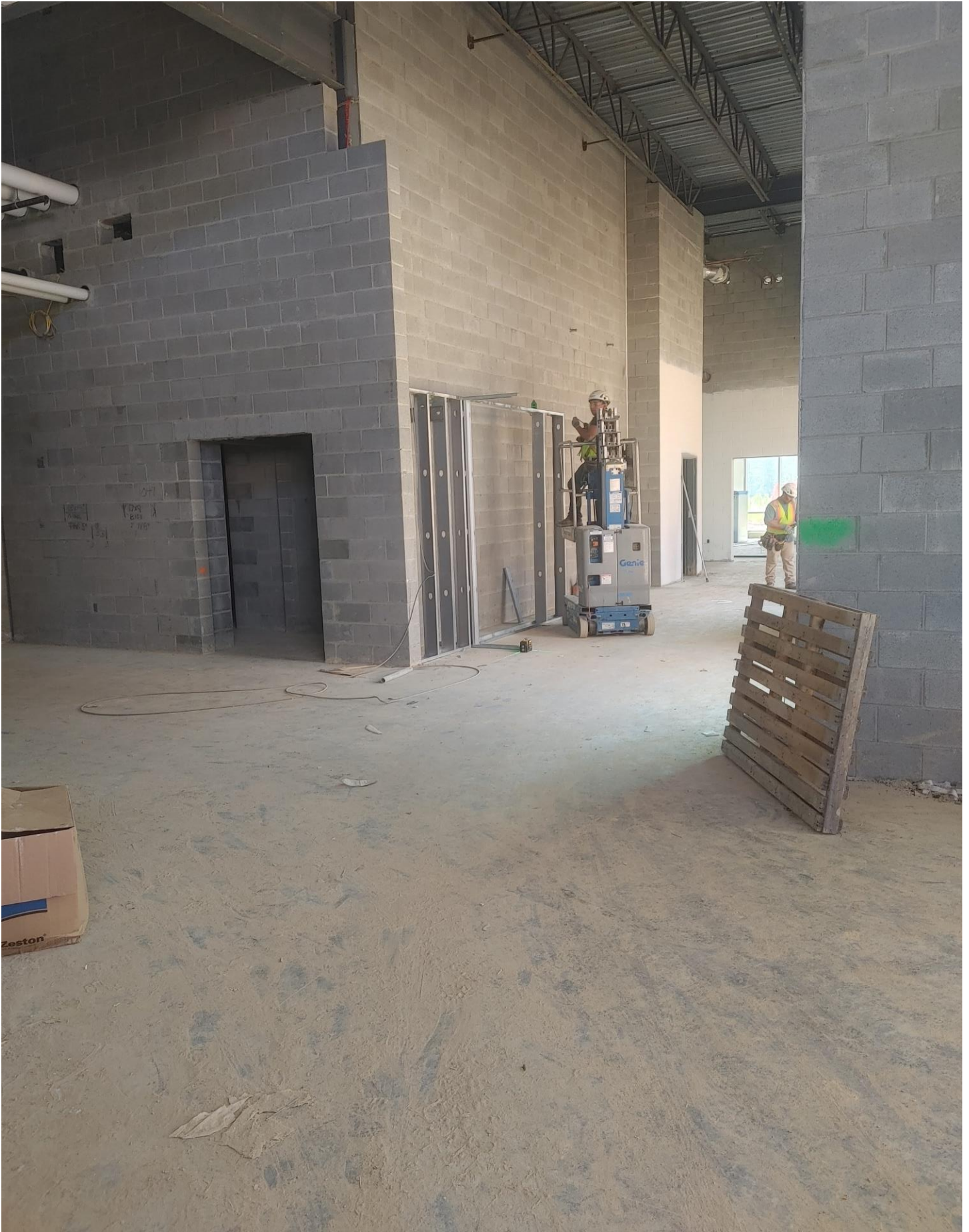
Photo 2 - Walls are being framed in Area D.
