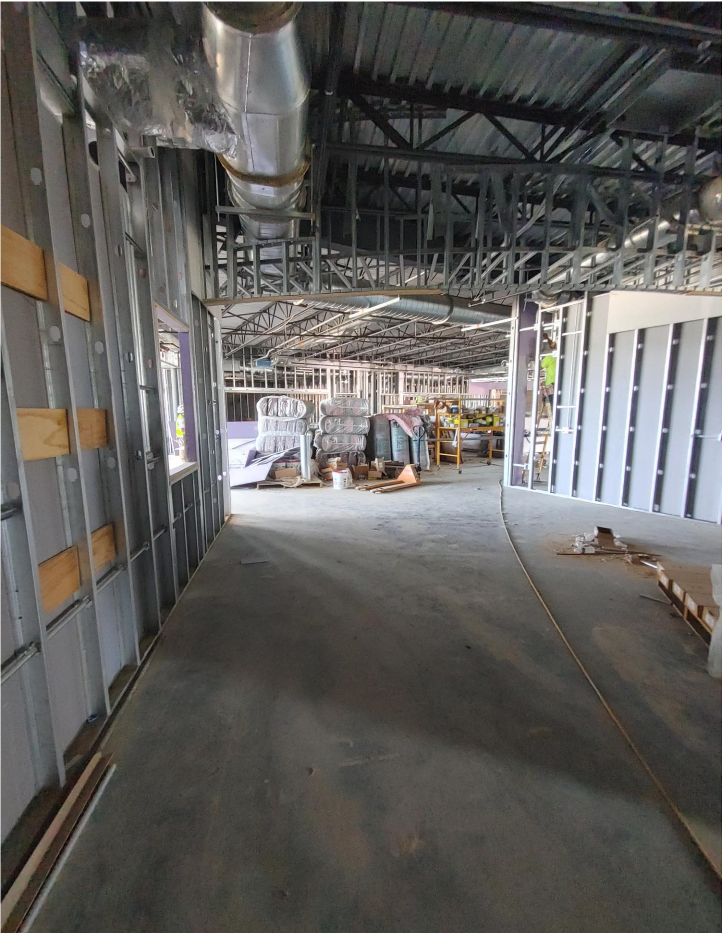
Photo 8 - Sheetrock is being hung on the 2nd floor of Area A.
