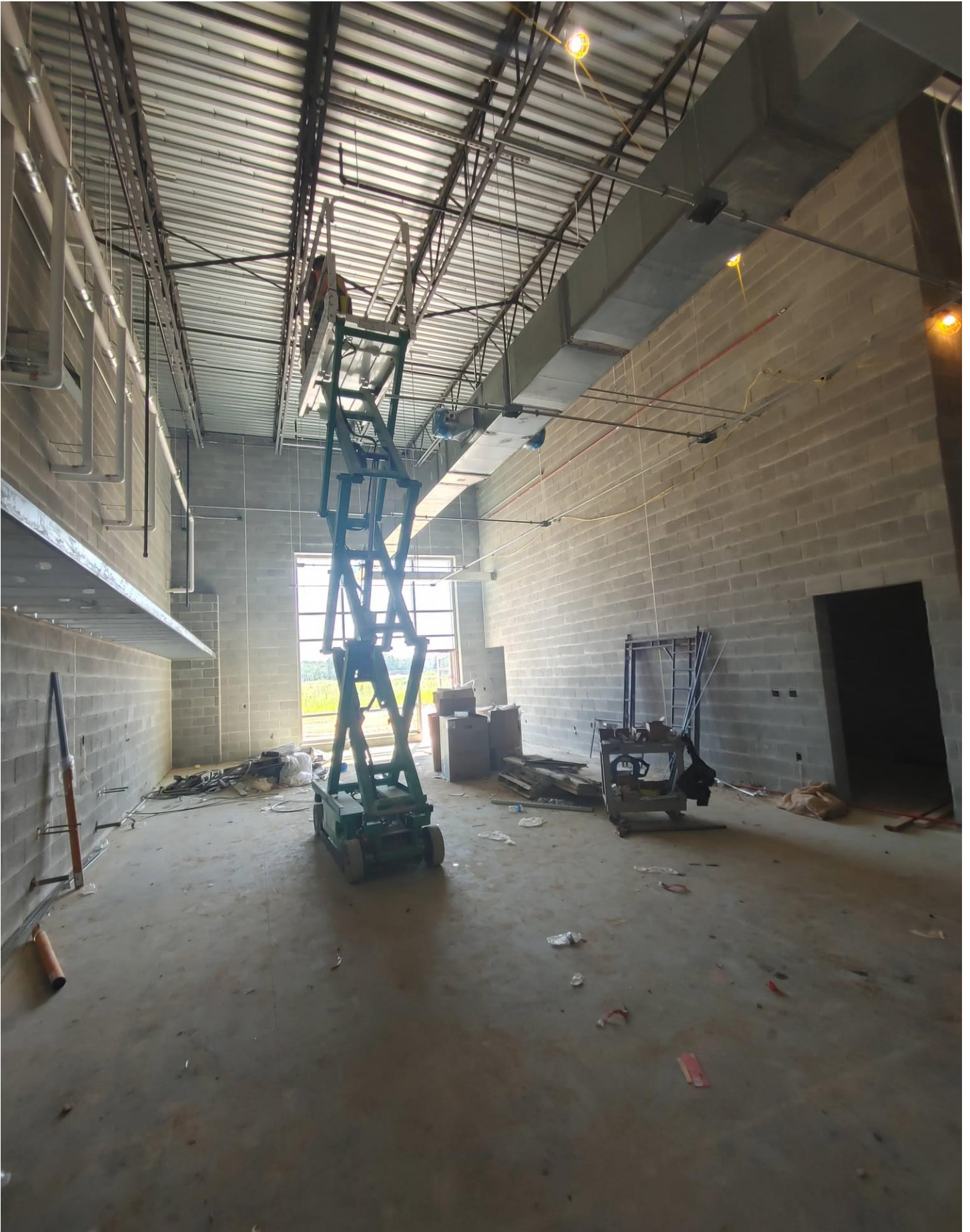
Photo 7 - Electrical Conduit is being run in Area D.
