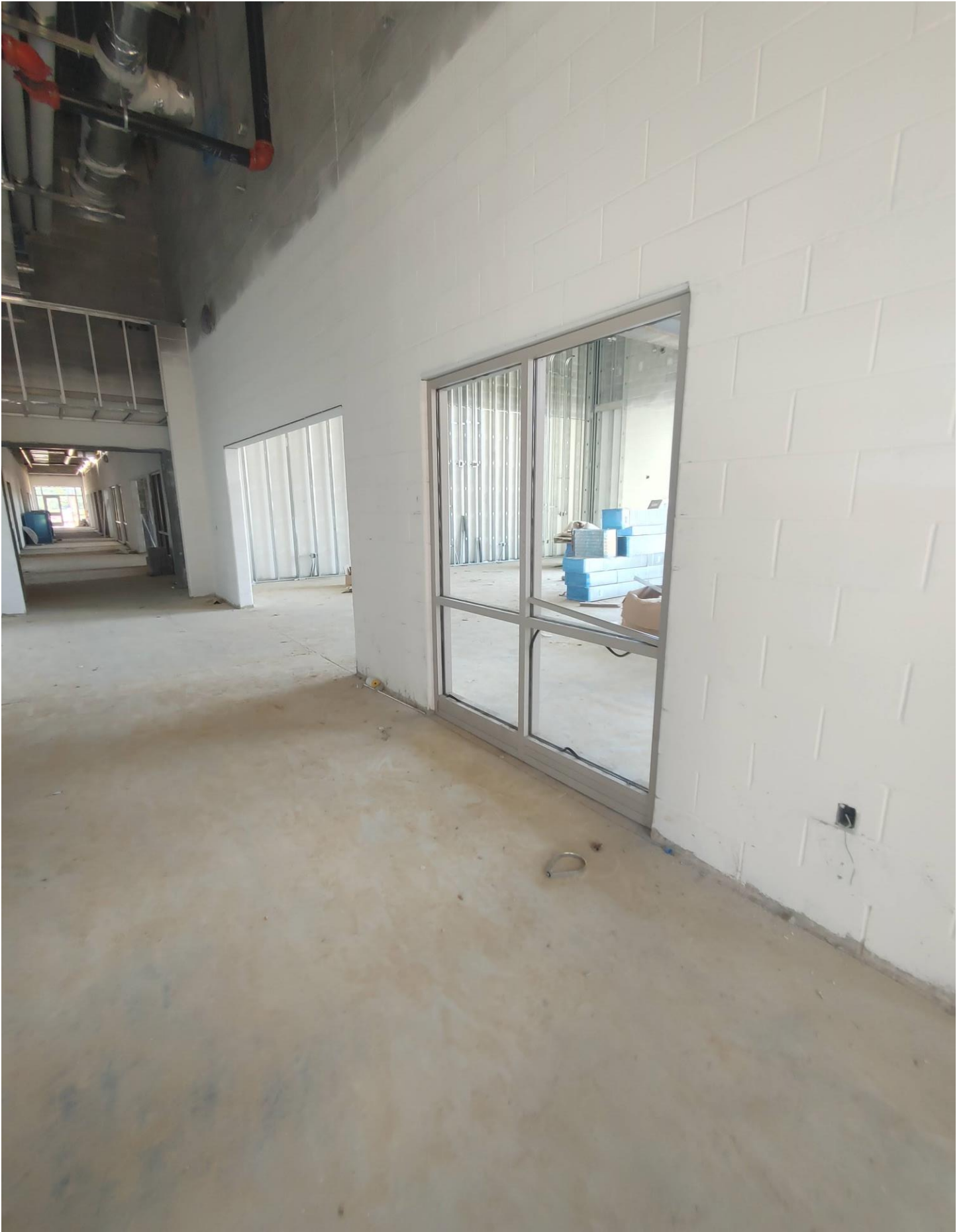
Photo 6 - Storefronts are being et in Corridor D12
