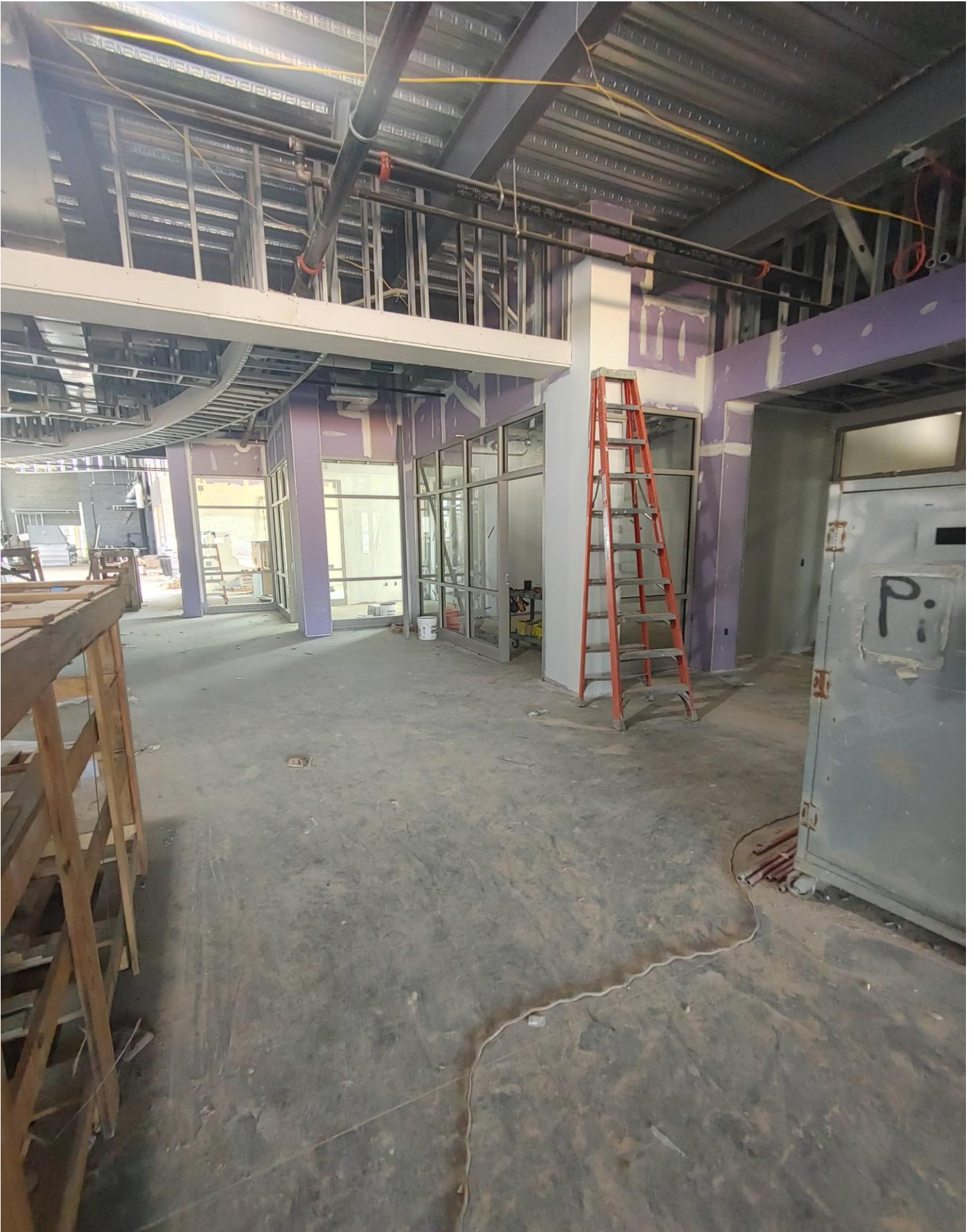
Photo 2 - Storefronts continue to be set on Area A.
