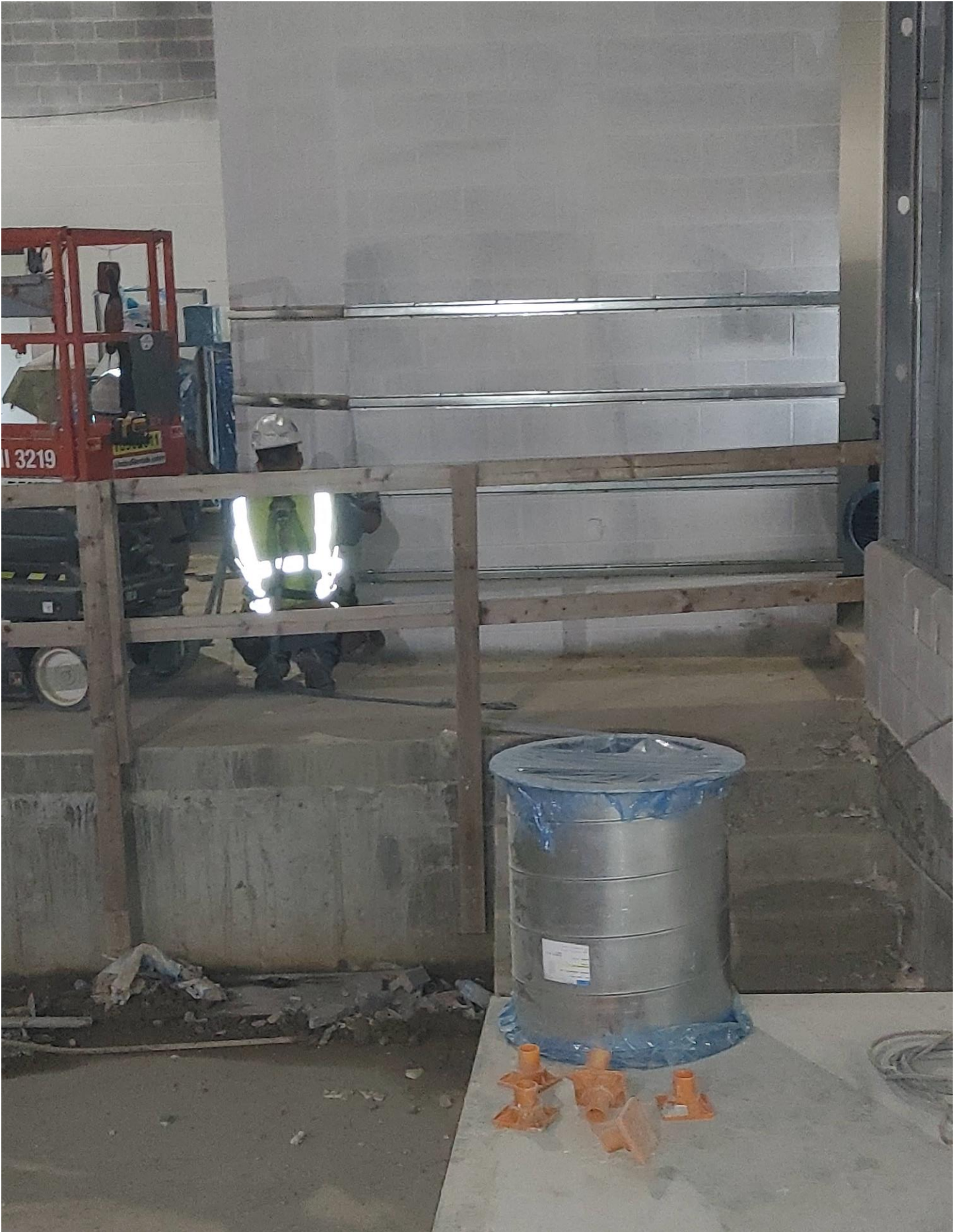
Photo 8 - Hat Channel is being installed in the Auditorium.
