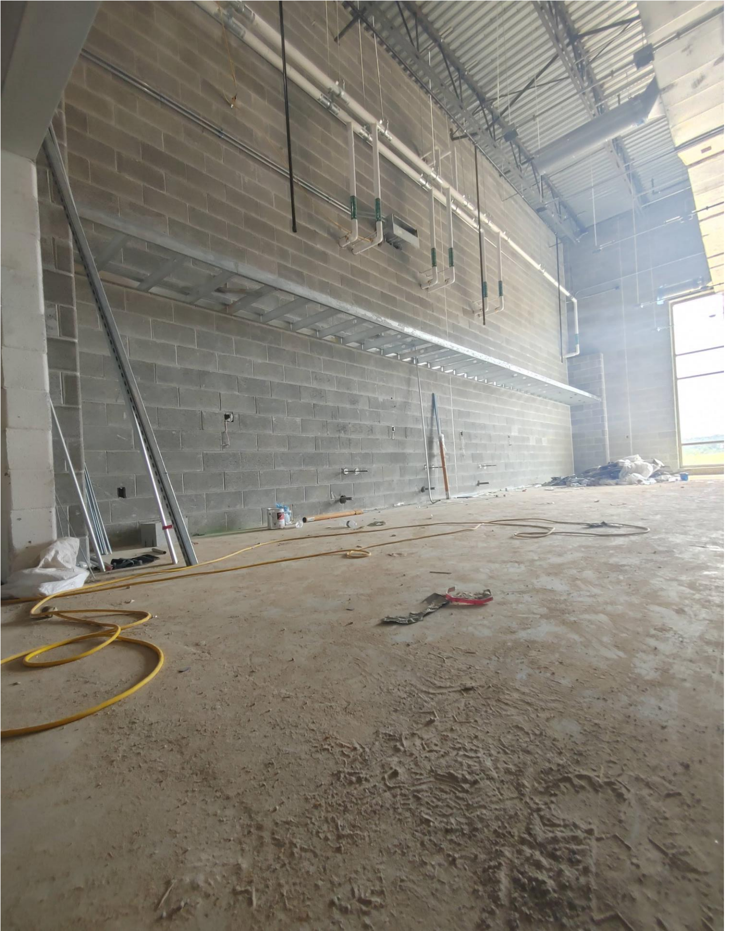
Photo 16 - Ceiling Framing in D121
