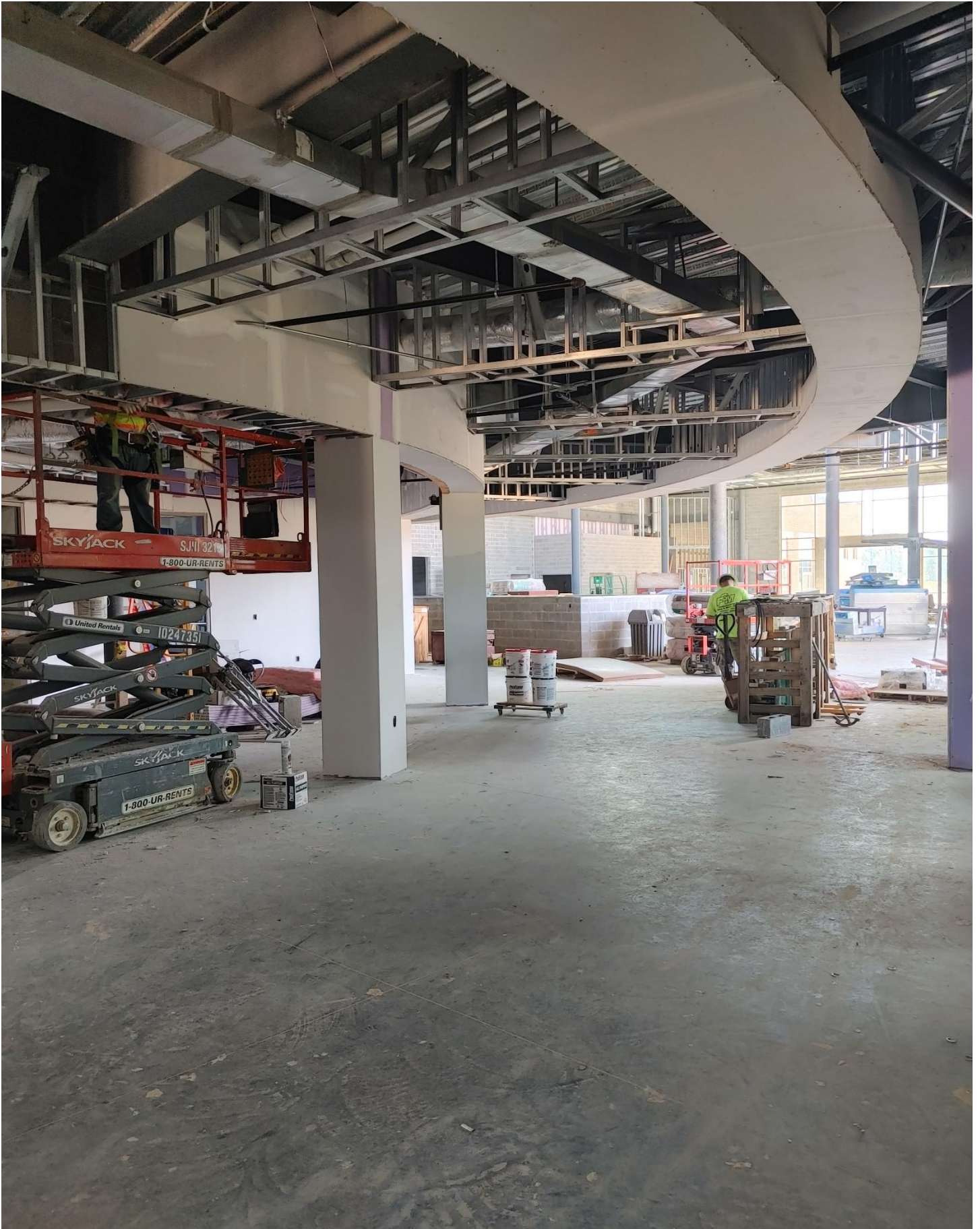
Photo 8 - Sheetrock is being finished in Area A.
