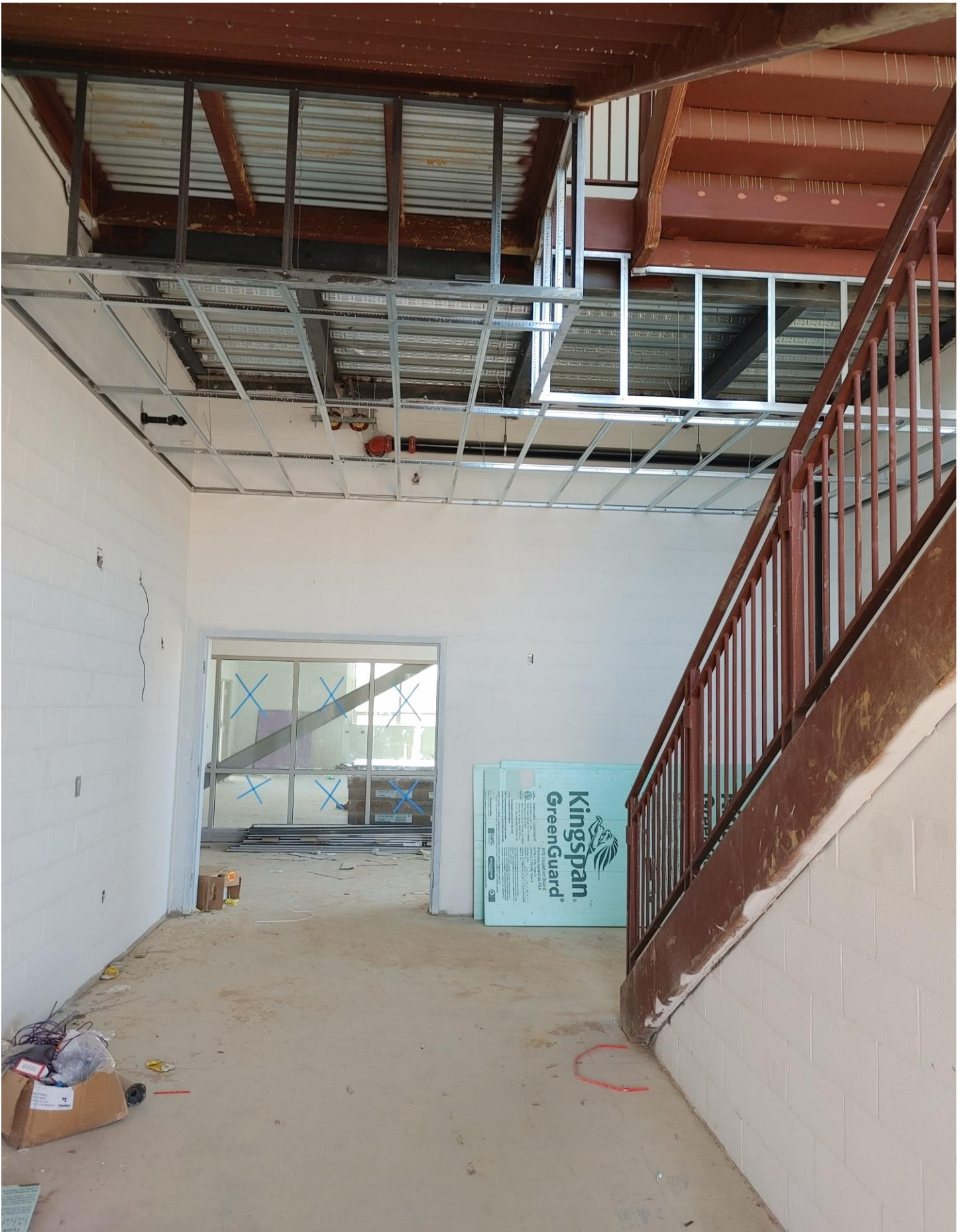
Photo 7 - Ceiling and Bulkhead has been constructed in Stair #2
