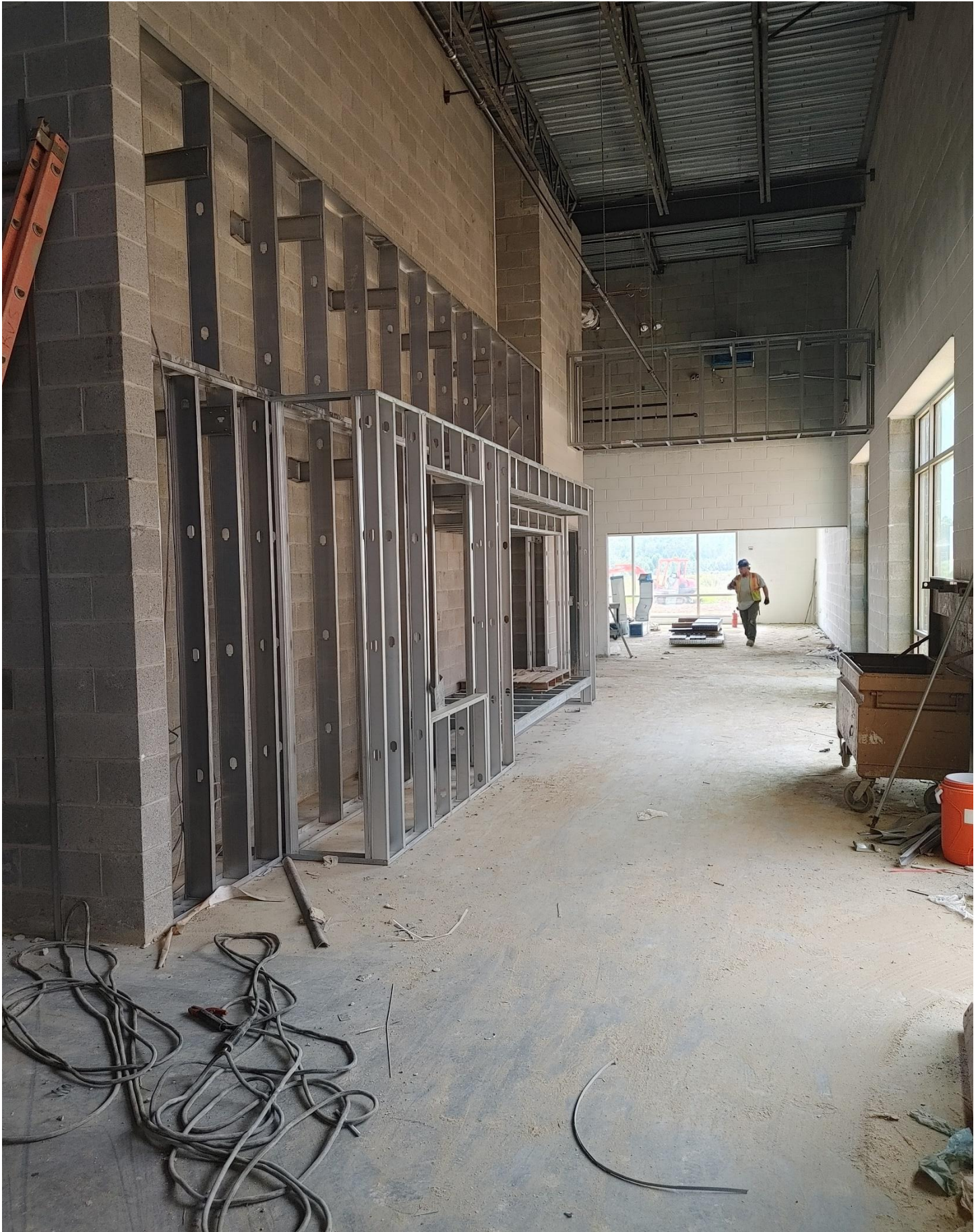
Photo 15 - Walls and Bulkhead have been framed in Area D
