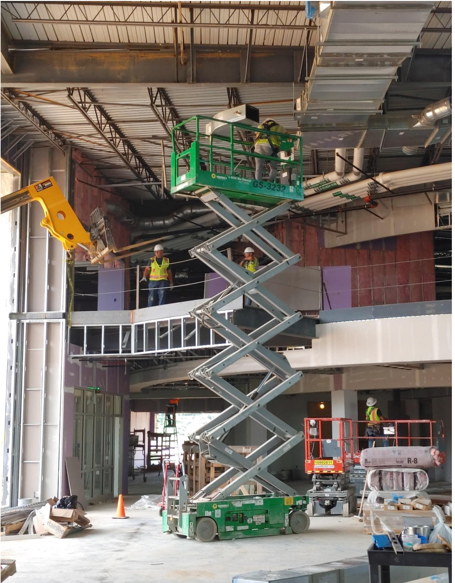
Photo 14 - Ductwork is being installed in Area C
