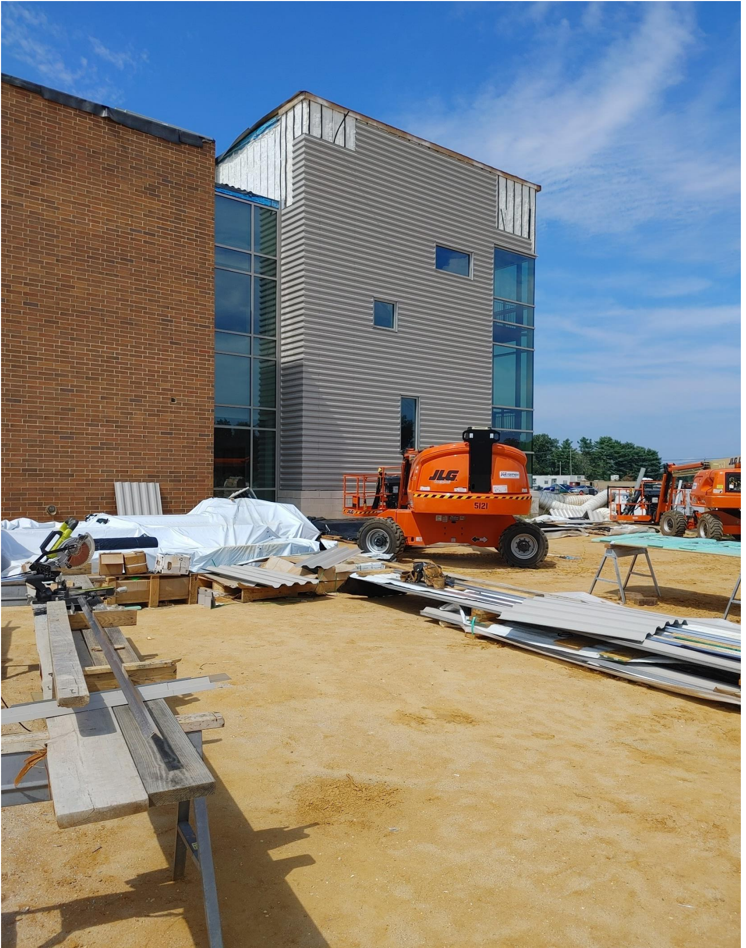
Photo 2 - Stairwell #1 is having metal panels installed.
