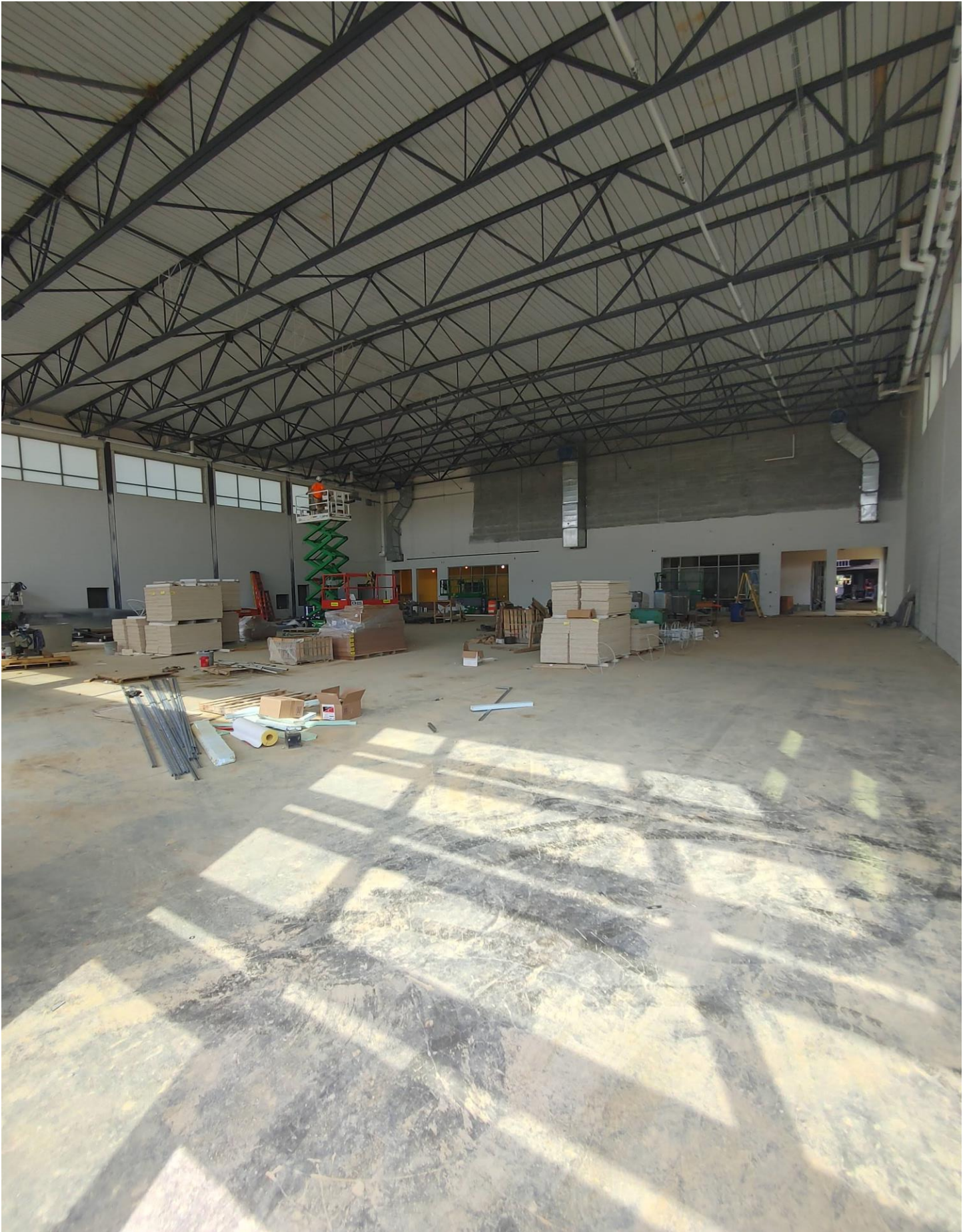
Photo 4 - Sprinkler Pipe is being installed in the Gym.
