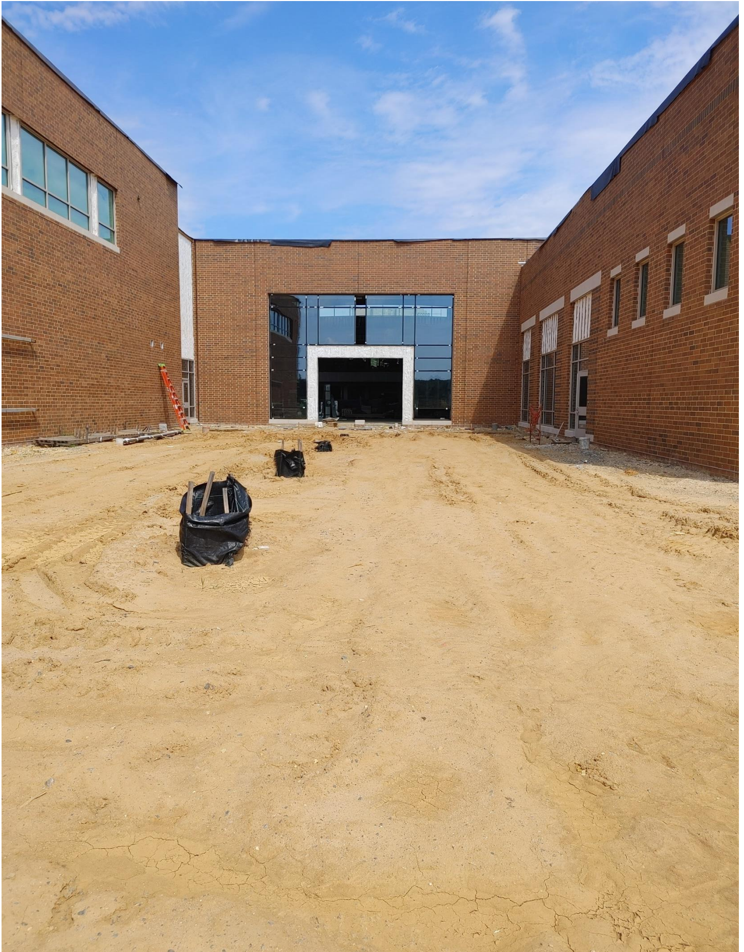
Photo 3 -A few glass panels still need to be installed on CW1
