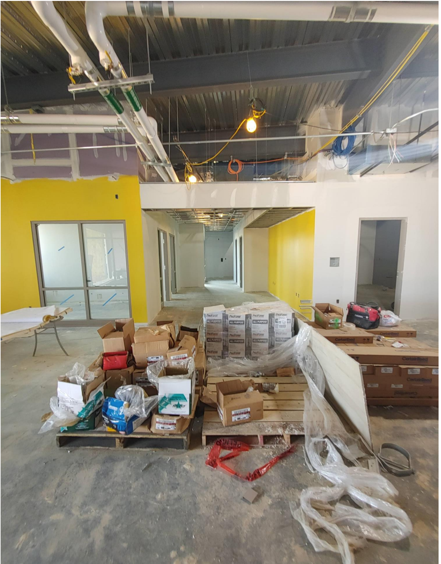
Photo 9 - Walls are being painted in the Administrative area of Area A.
