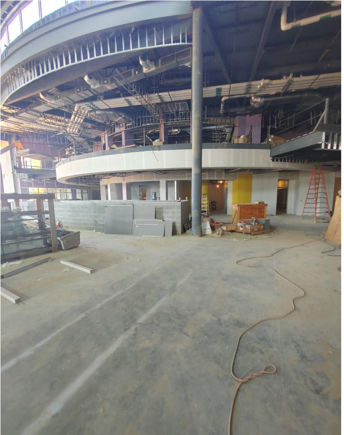
Photo 10 - Sheetrock being finished in Area A.
