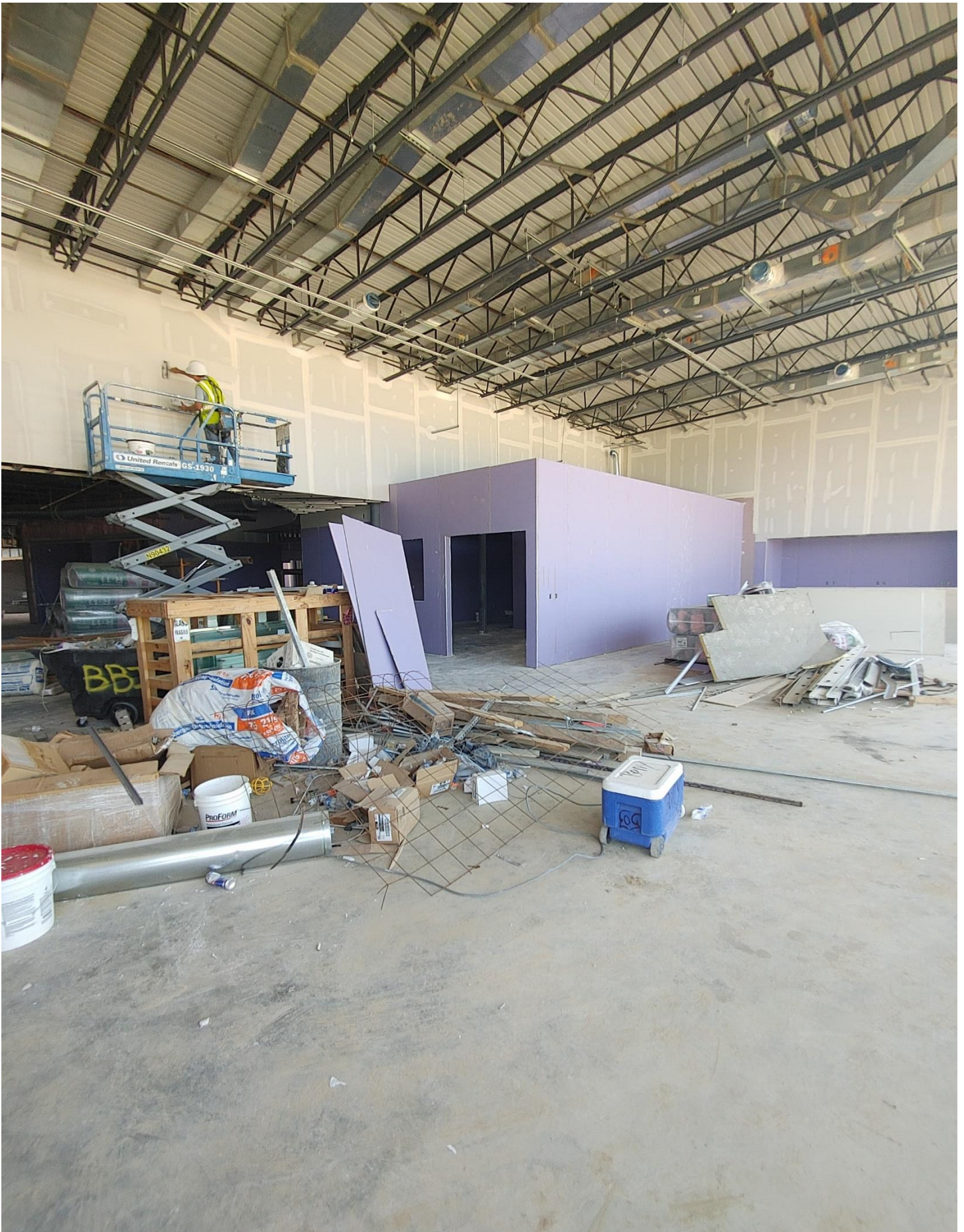
Photo 13 Sheetrock is being finished in Area A
