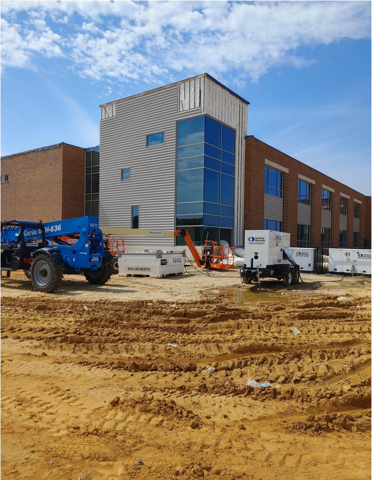
Photo 1 - Metal is being installed on Stairwell #1
