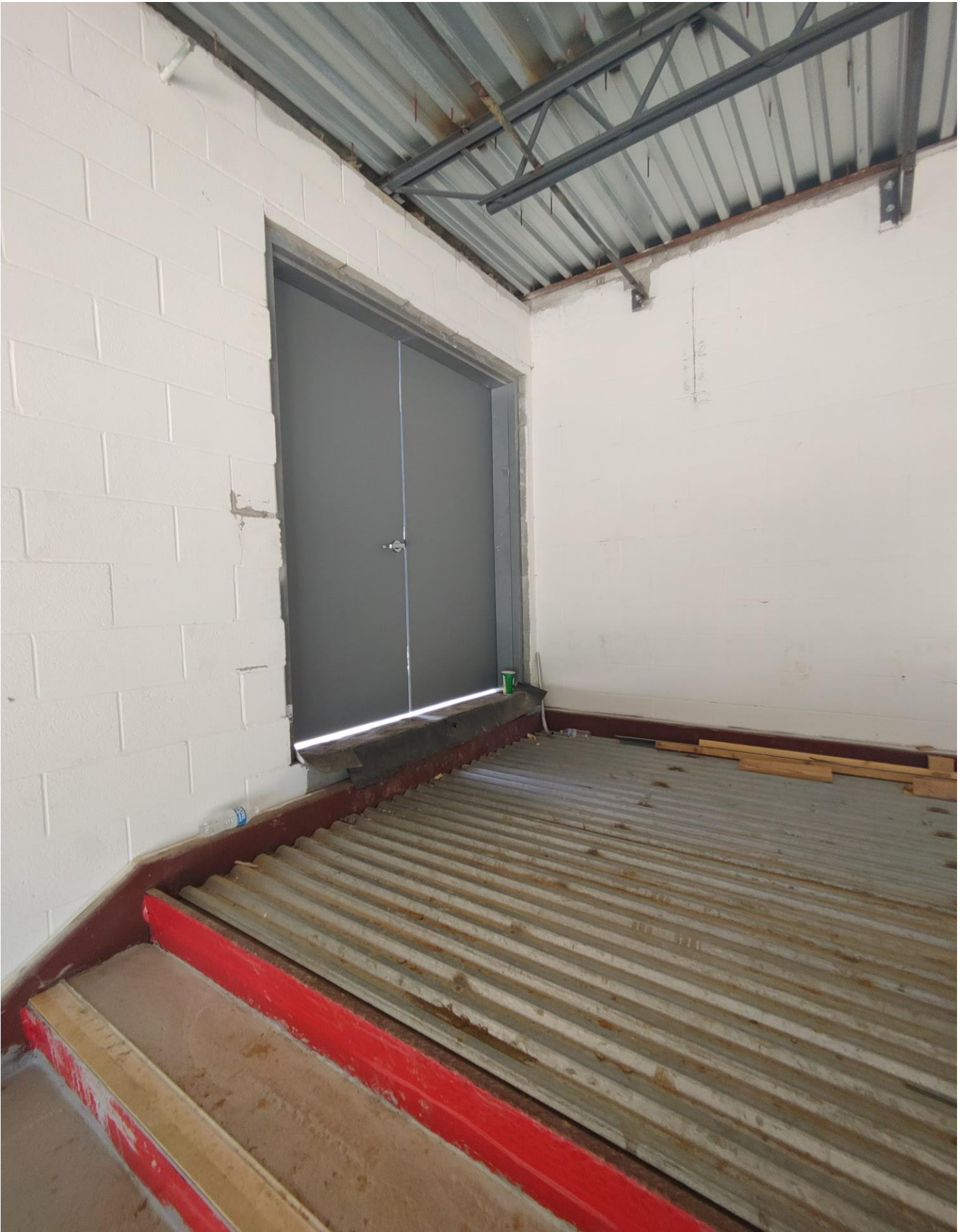
Photo 12 - Doors ST2C at the top of the Stairwell have been installed.
