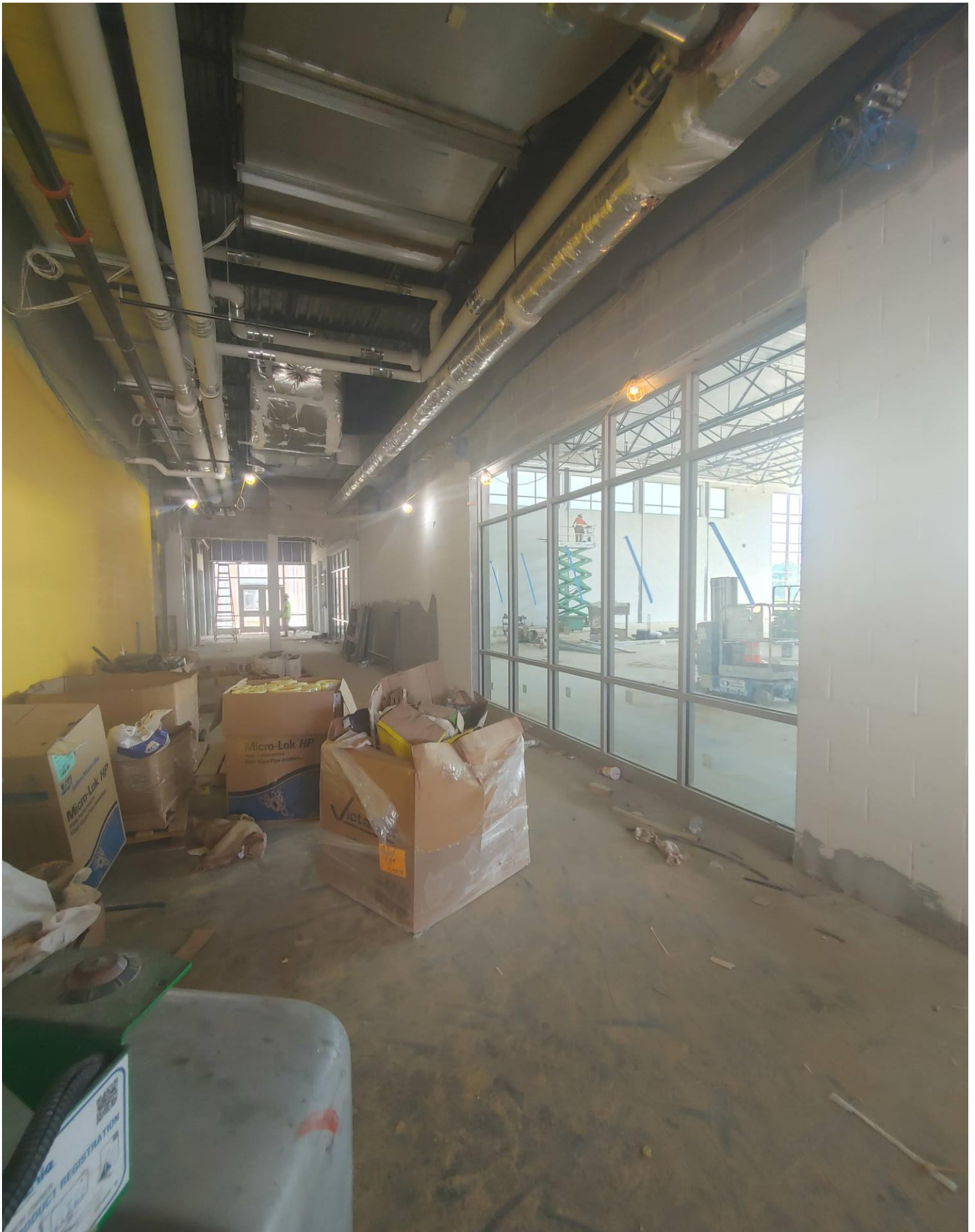
Photo 16 - SF #47 has been installed
