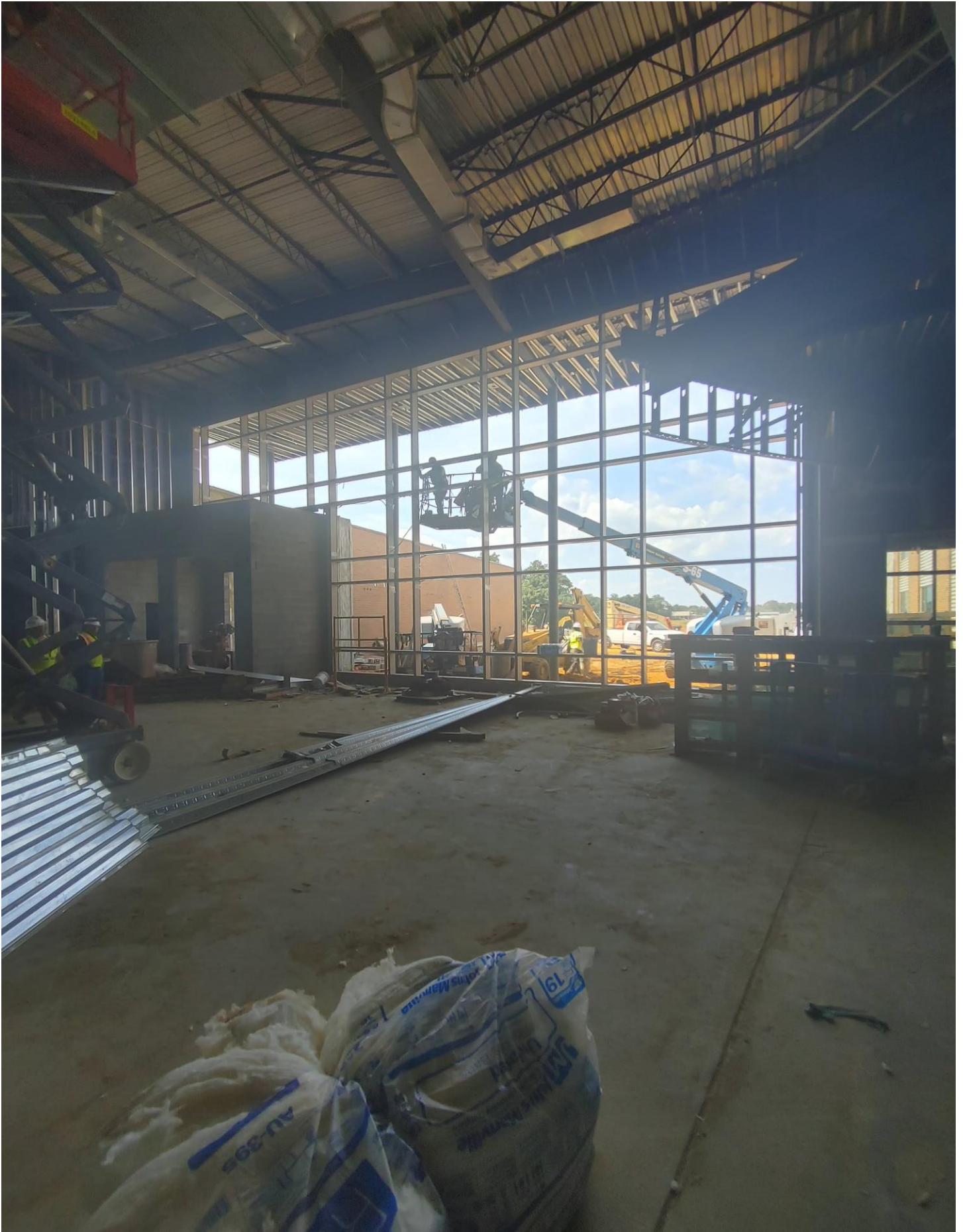
Photo 12 - CW#2 is being installed
