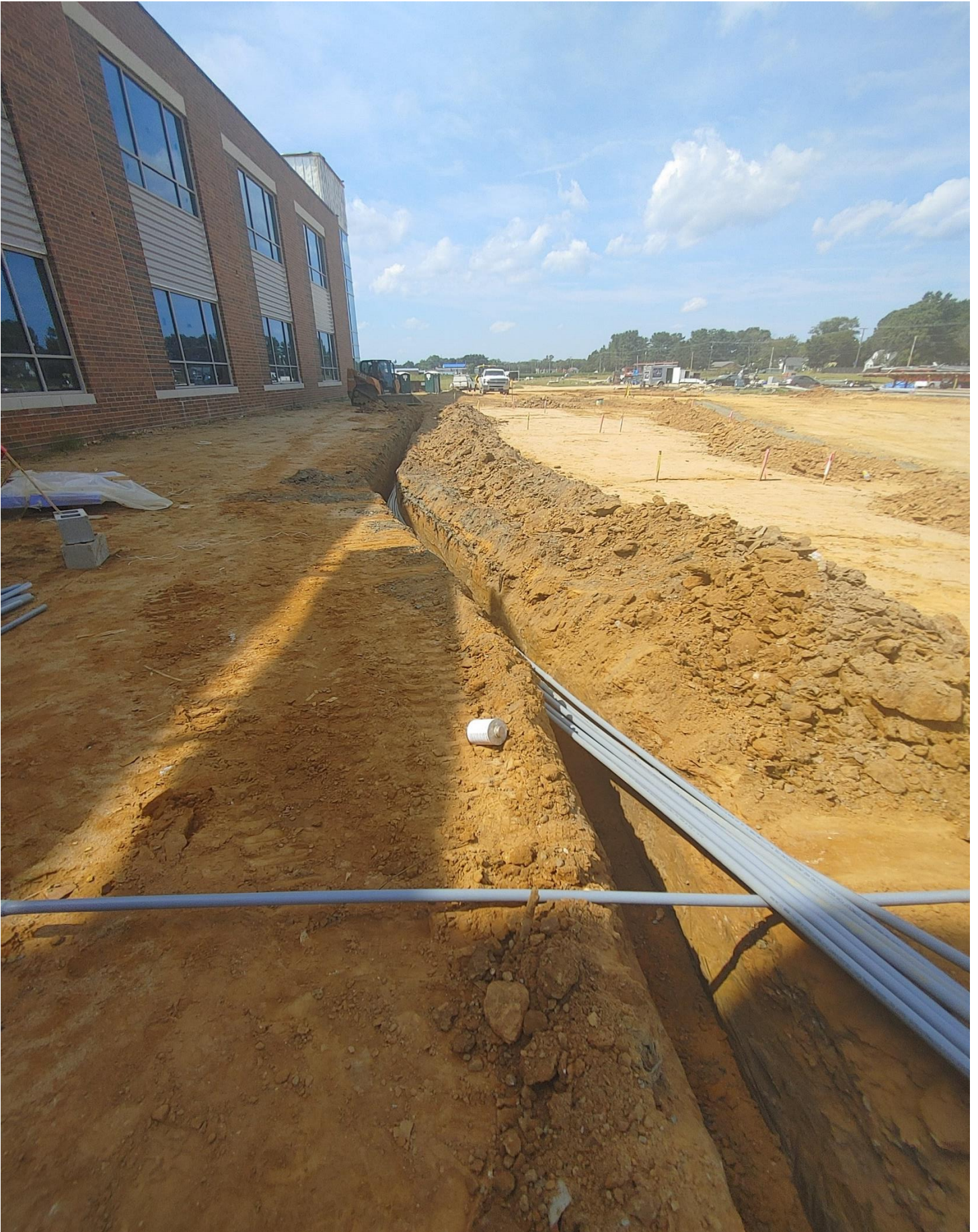
Photo 8 - The masons are running conduit for Pole Lights
