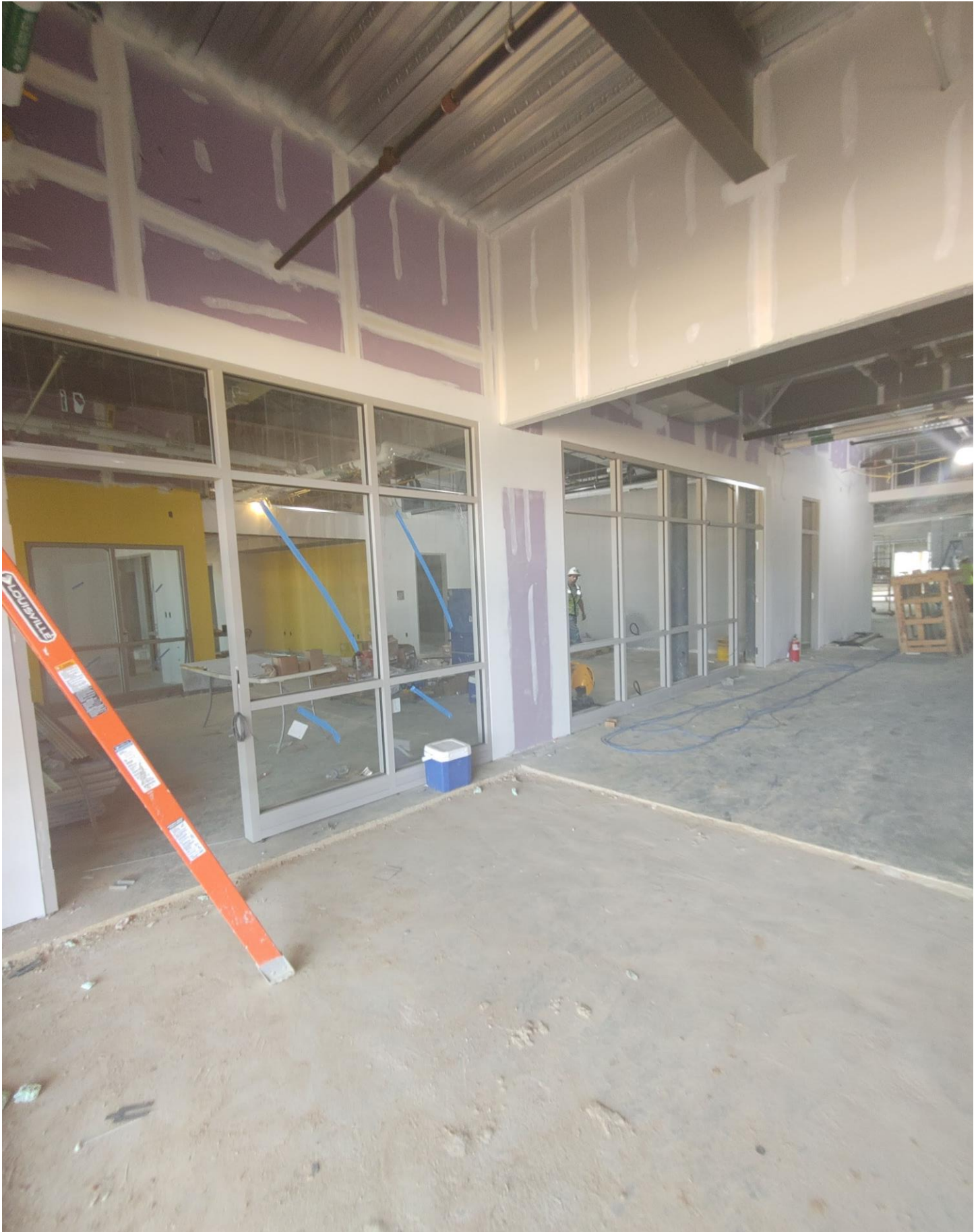
Photo 9 - SF #32A & #33 have been installed
