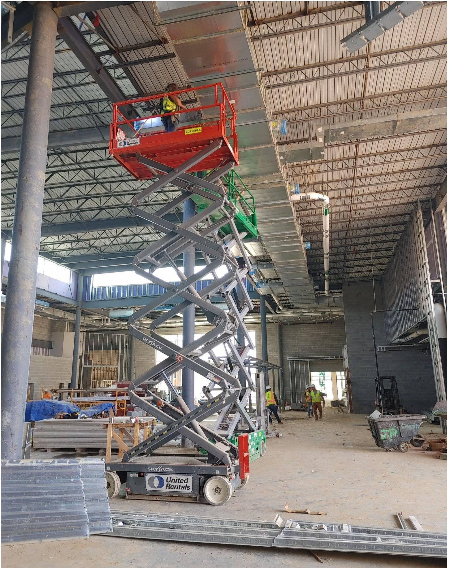
Photo 10 - Duct work is being installed in Area C.
