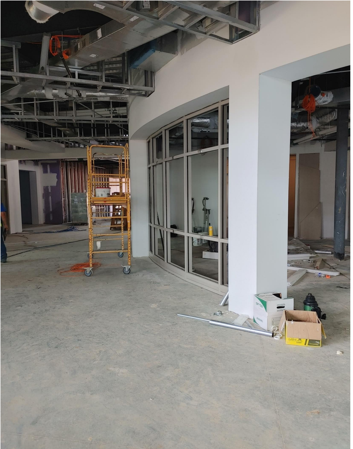
Photo 11 - SF #35 has been installed
