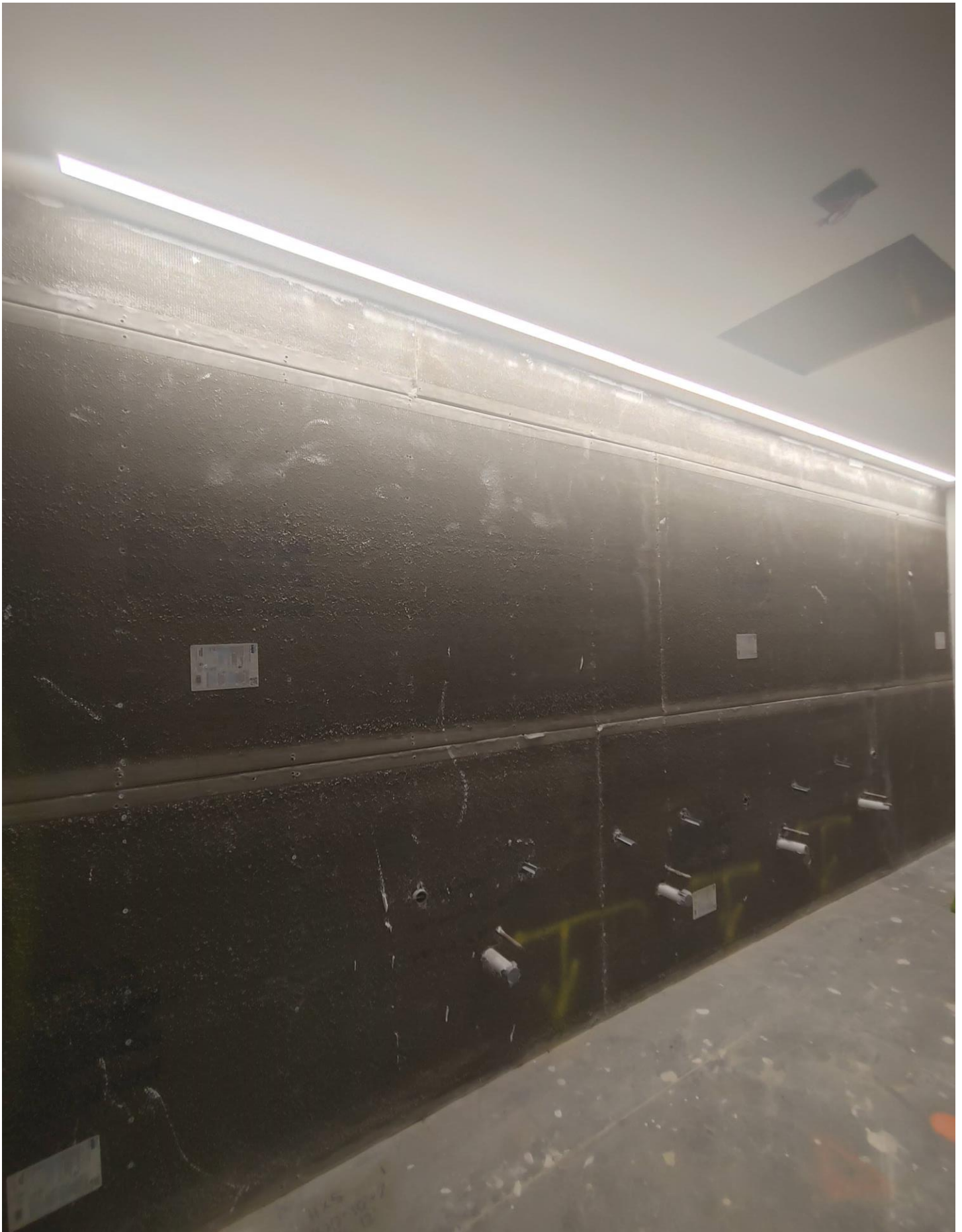
Photo 13 - Lighting has been installed in A118
