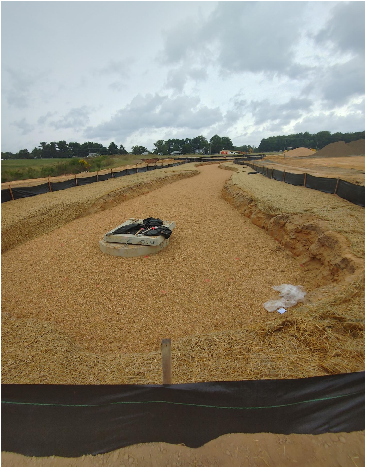
Photo 11 - Pea Gravel has been installed in BMP
