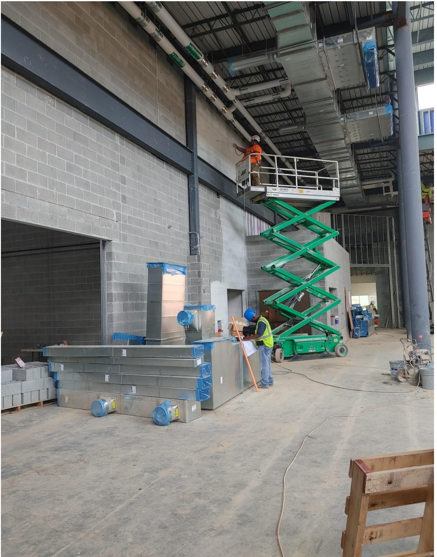
Photo 4 - Block Filler/Sealer is being applied in Area C.
