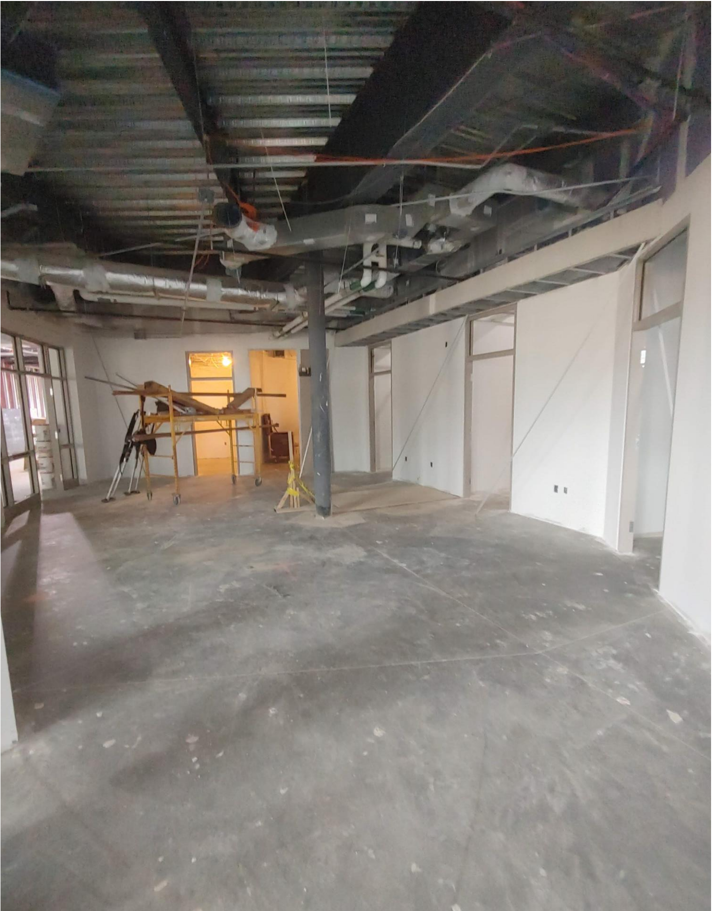
Photo 3 - Frames have been installed A134
