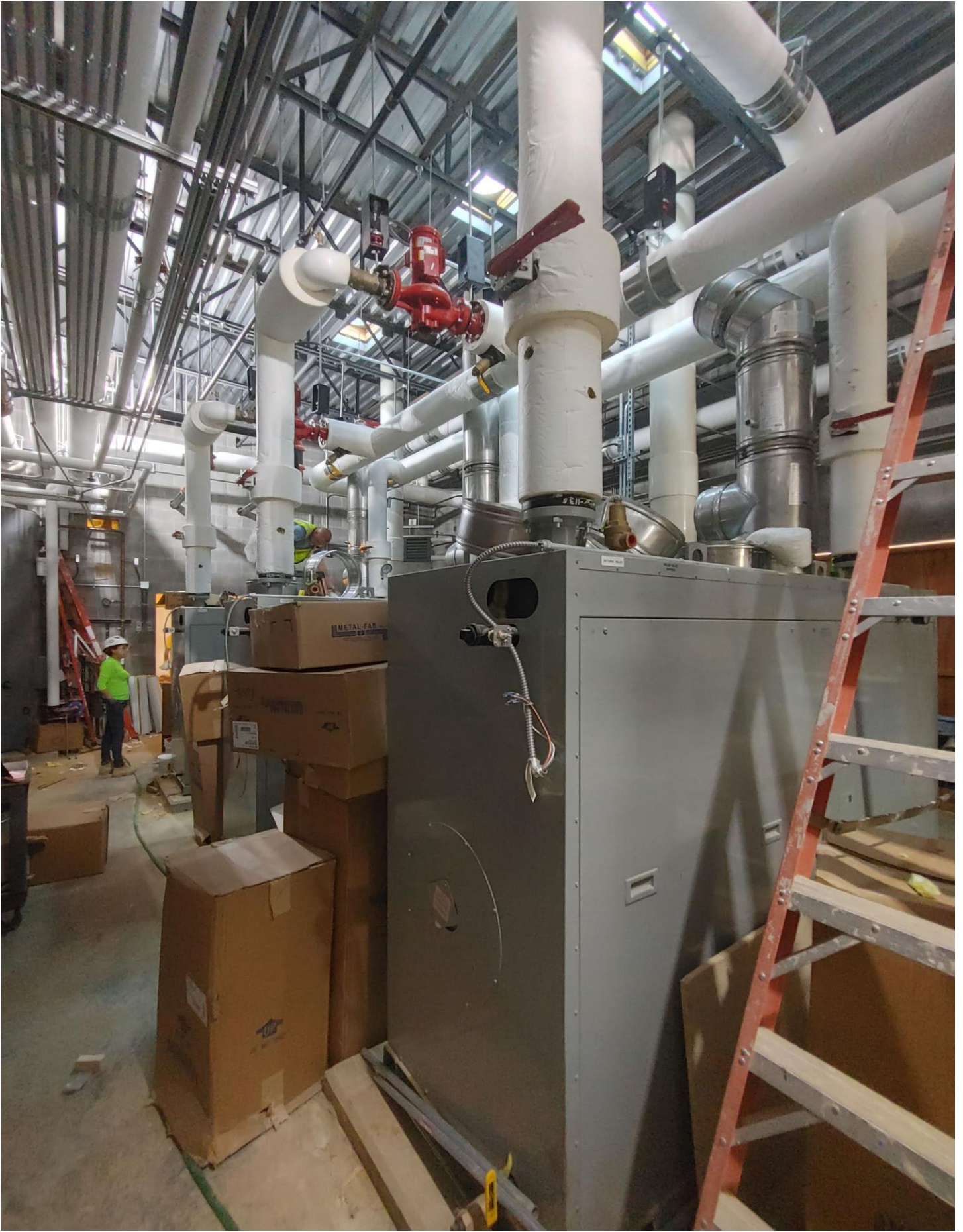
Photo 5 - Work continues on the Boilers in the Mechanical room.
