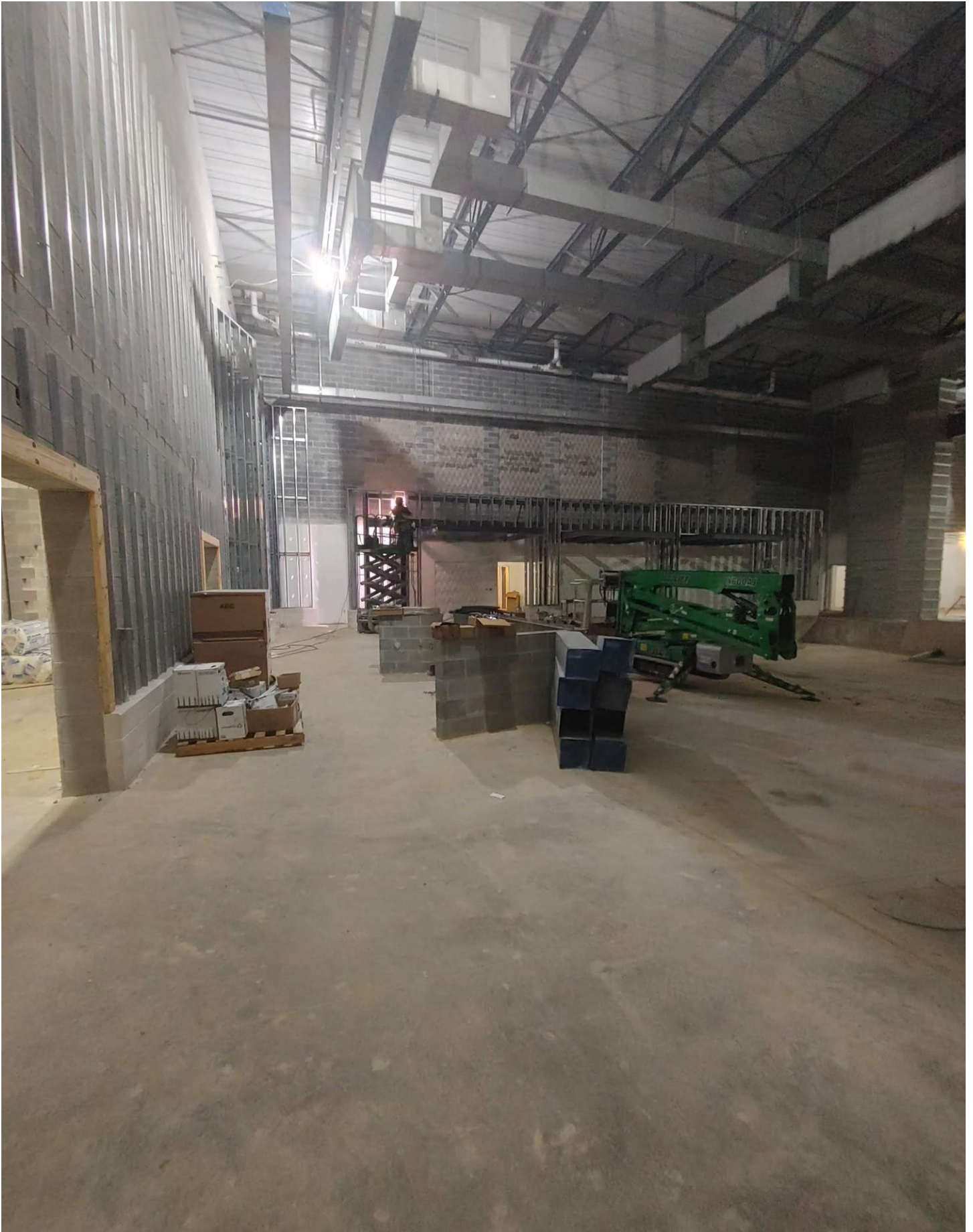
Photo 7 - Metal Beams are being welded in the Auditorium.
