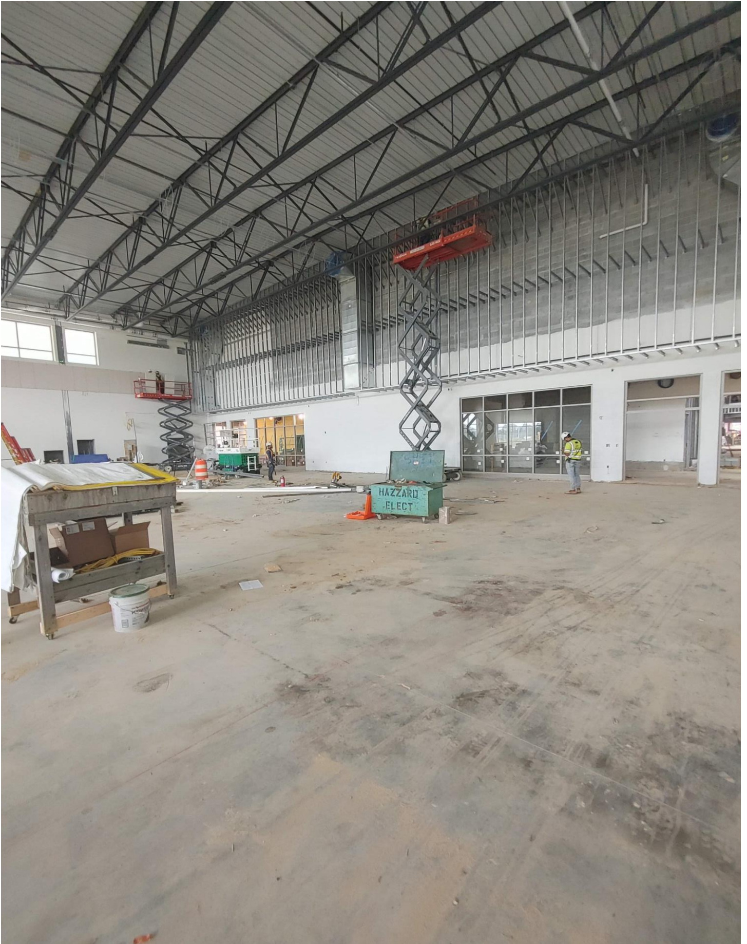
Photo 10 - Metal Stud Framing on the North wall of the Gym.
