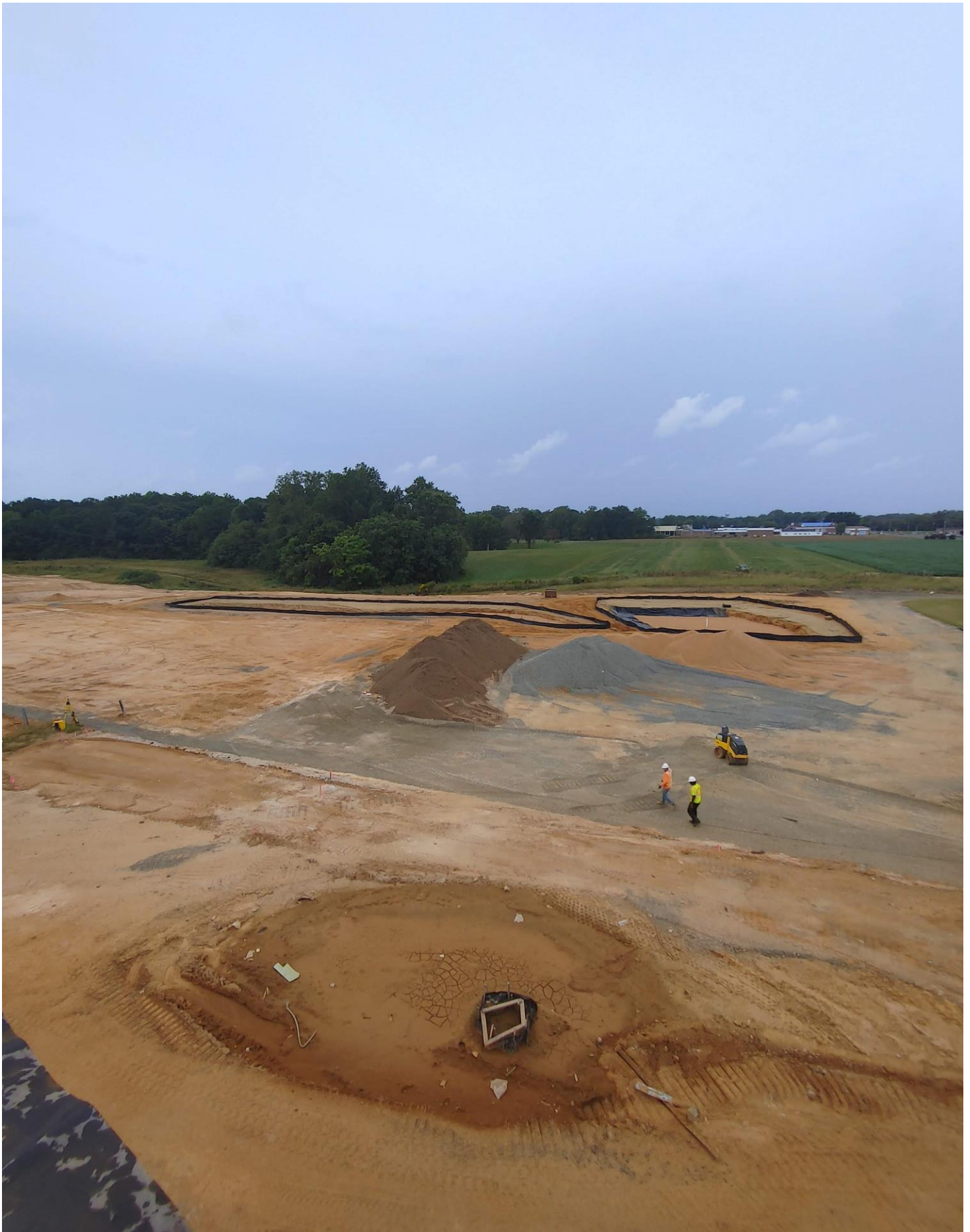
Photo 20 - BMPs and Bus Parking area.
