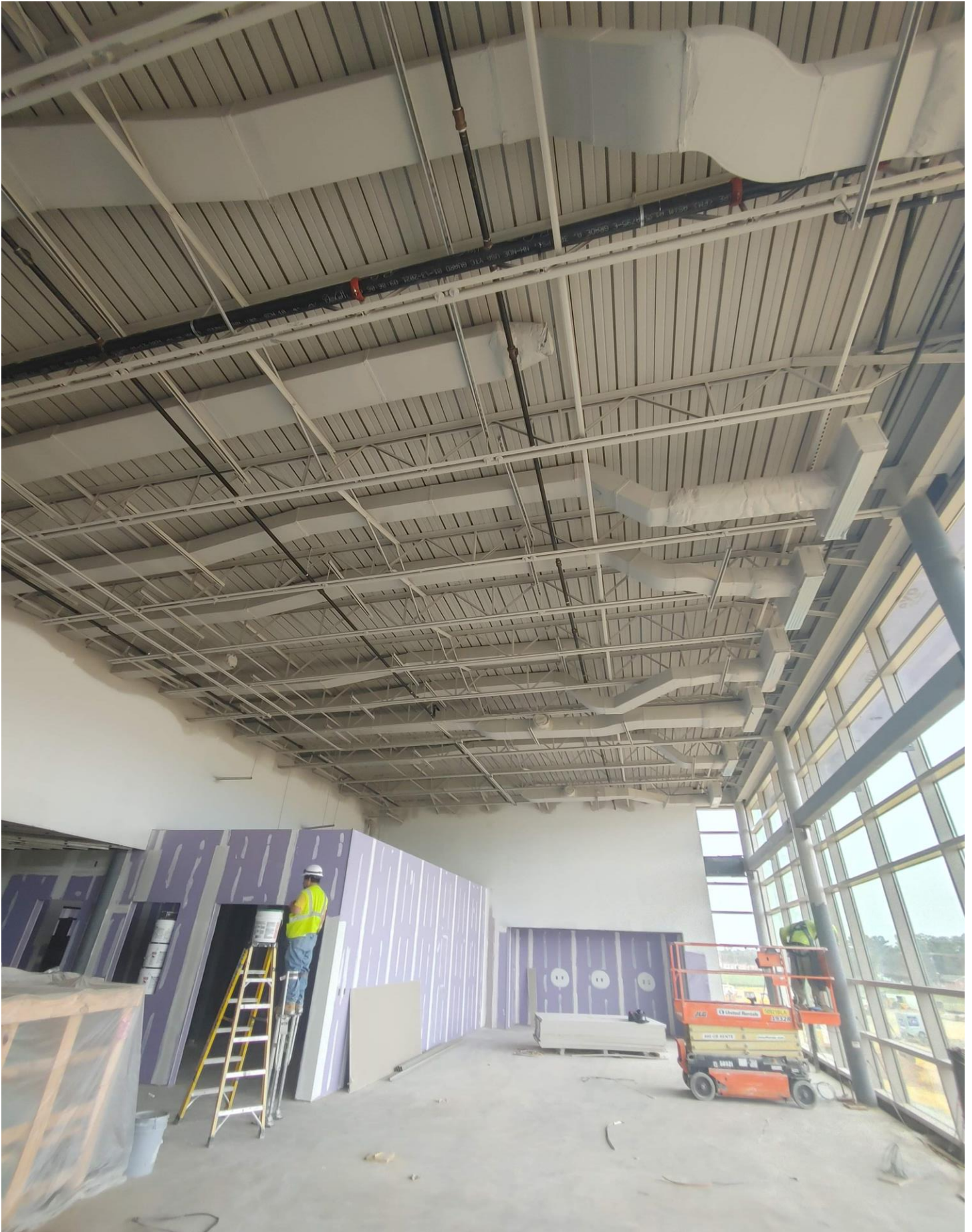
Photo 17 - Metal Deck and Duct has been sprayed in Area A.
