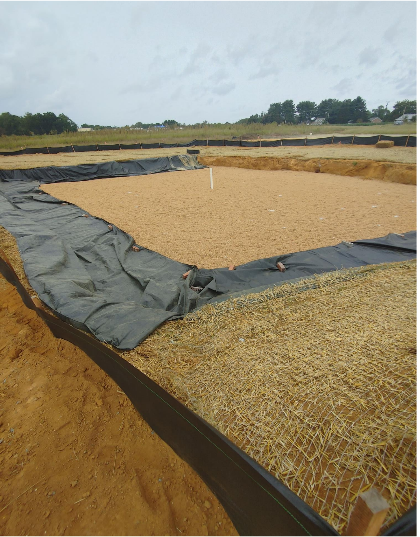
Photo 12 - Pea Gravel installed in smaller BMP
