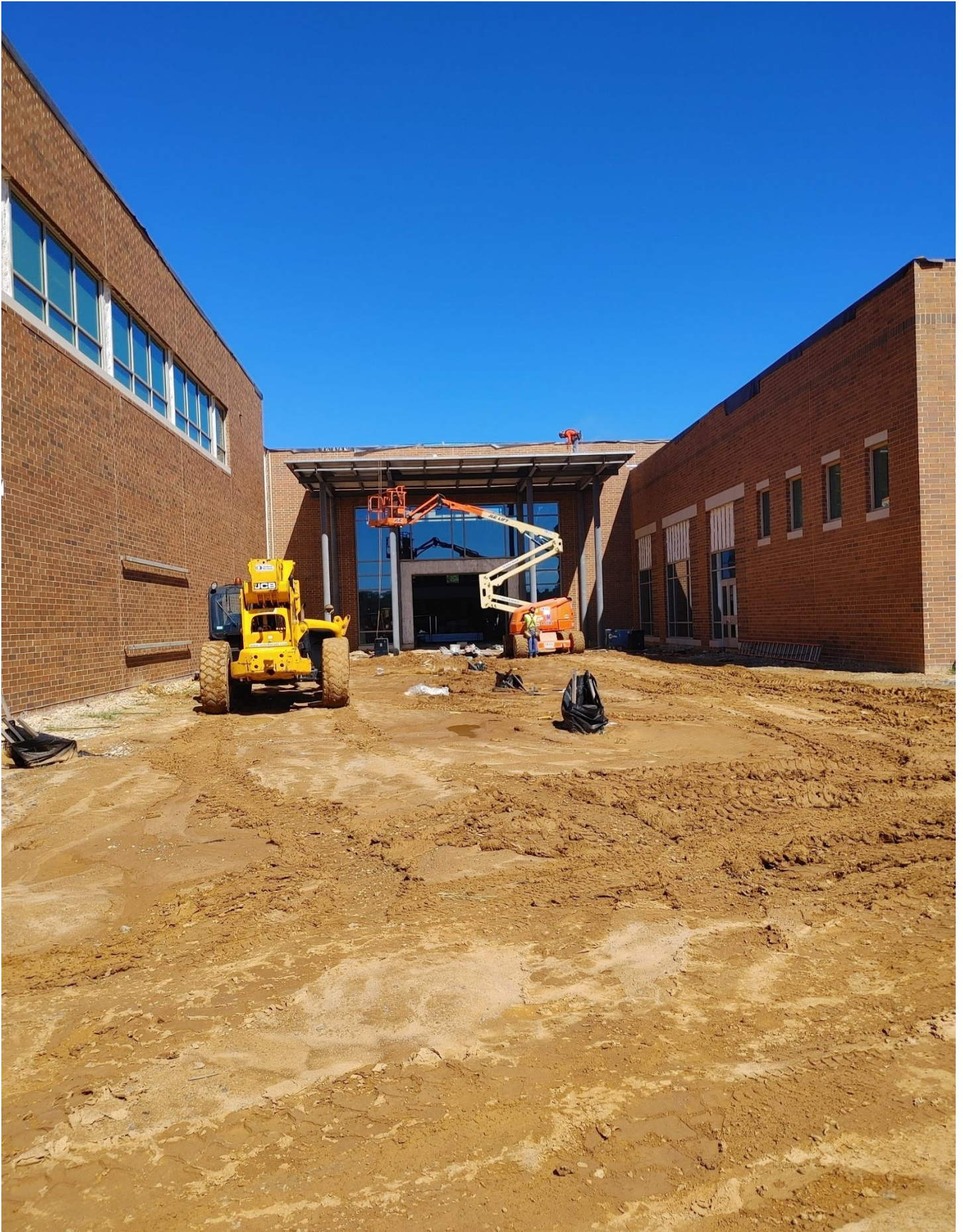
Photo 8 - South side of Area C. Steel is being welded on Canopy.
