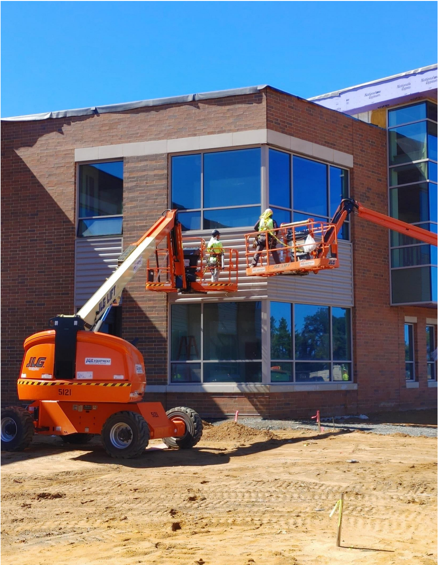
Photo 1 - Metal Panels are being installed on Area A
