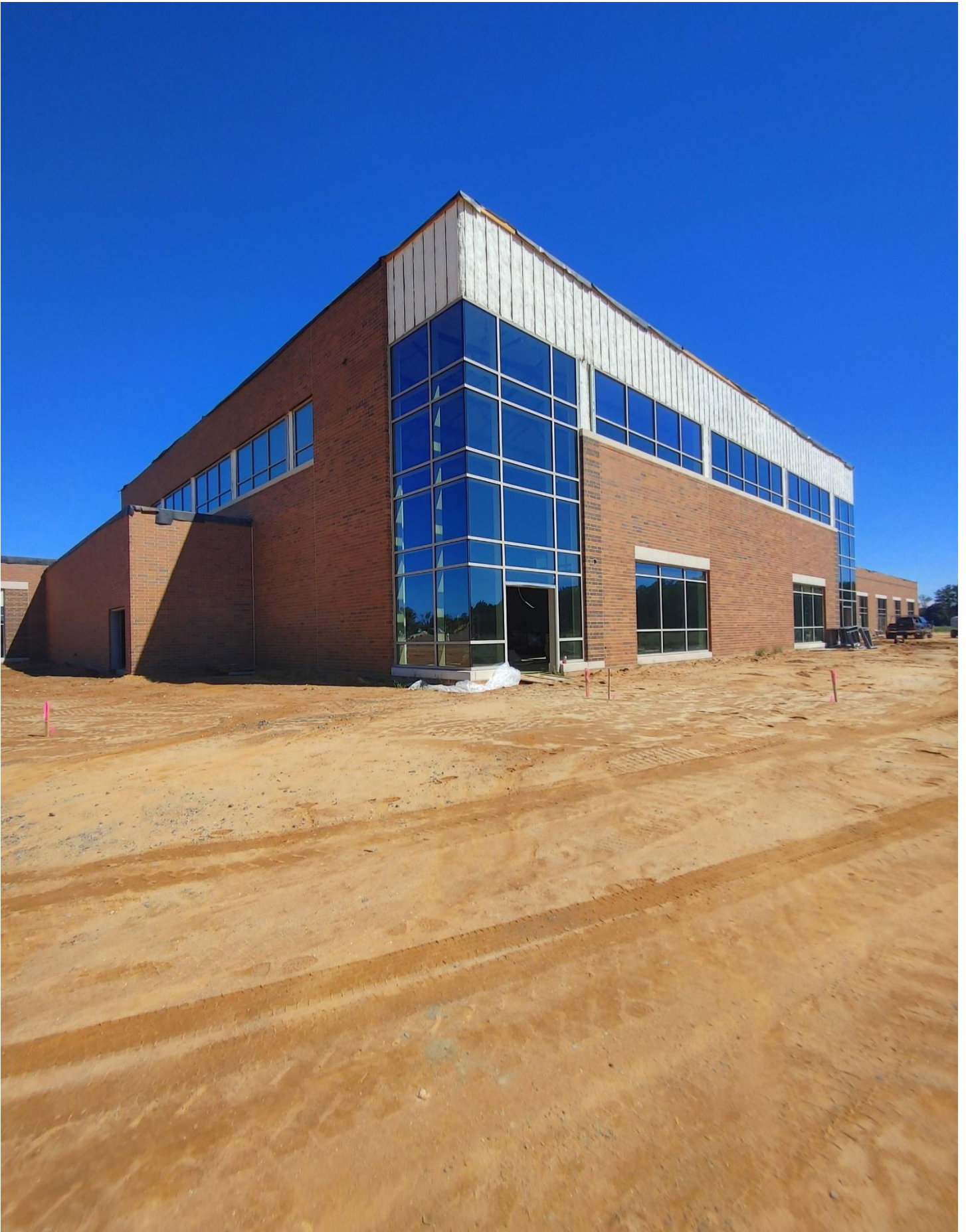
Photo 7 - South side of Gymnasium.
