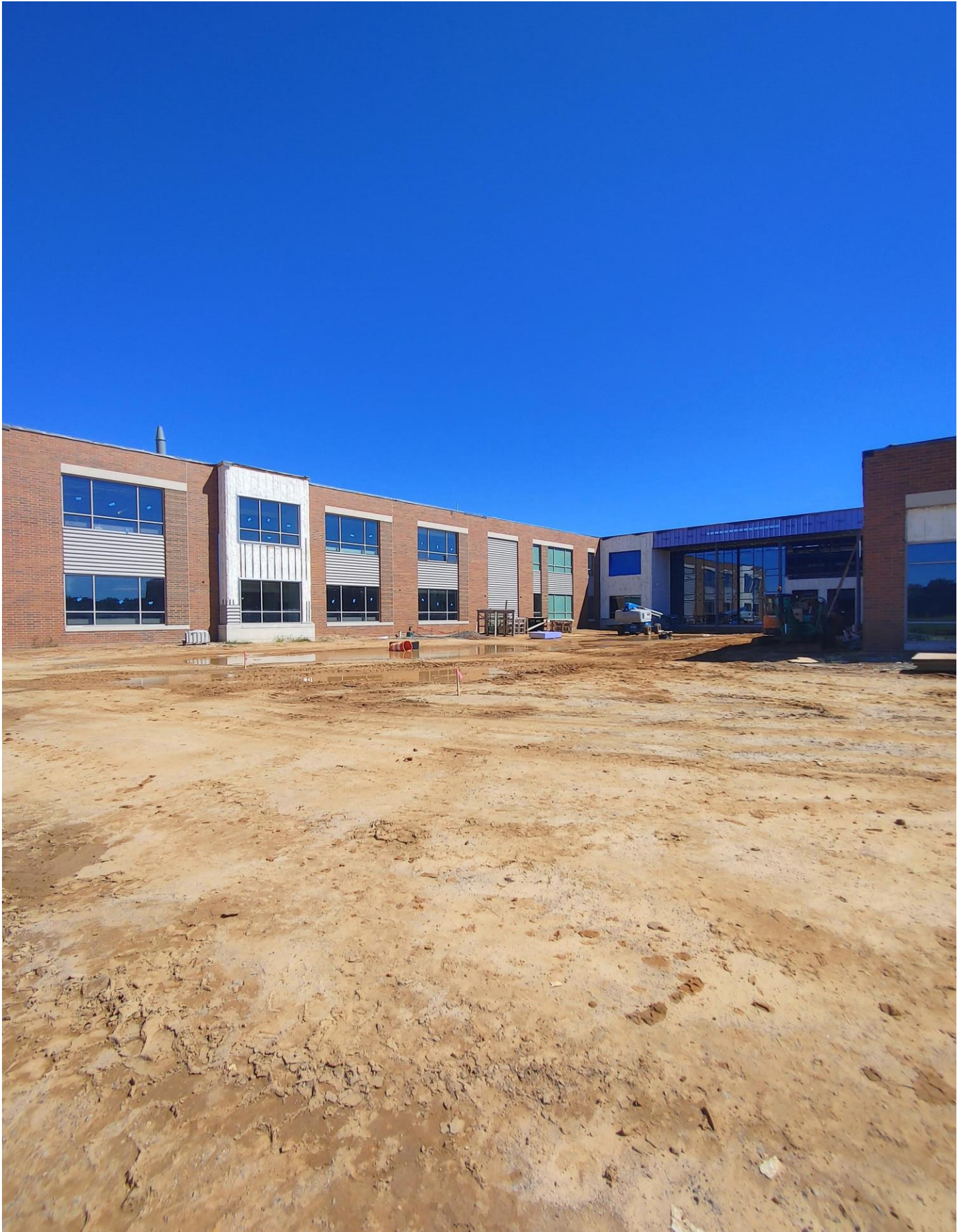
Photo 4 - South side of Area B and Curtain wall of Area C.
