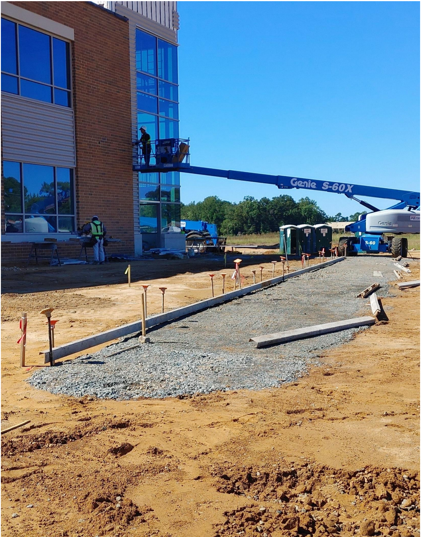
Photo 3 - Sidewalks are being formed in front of Area B.
