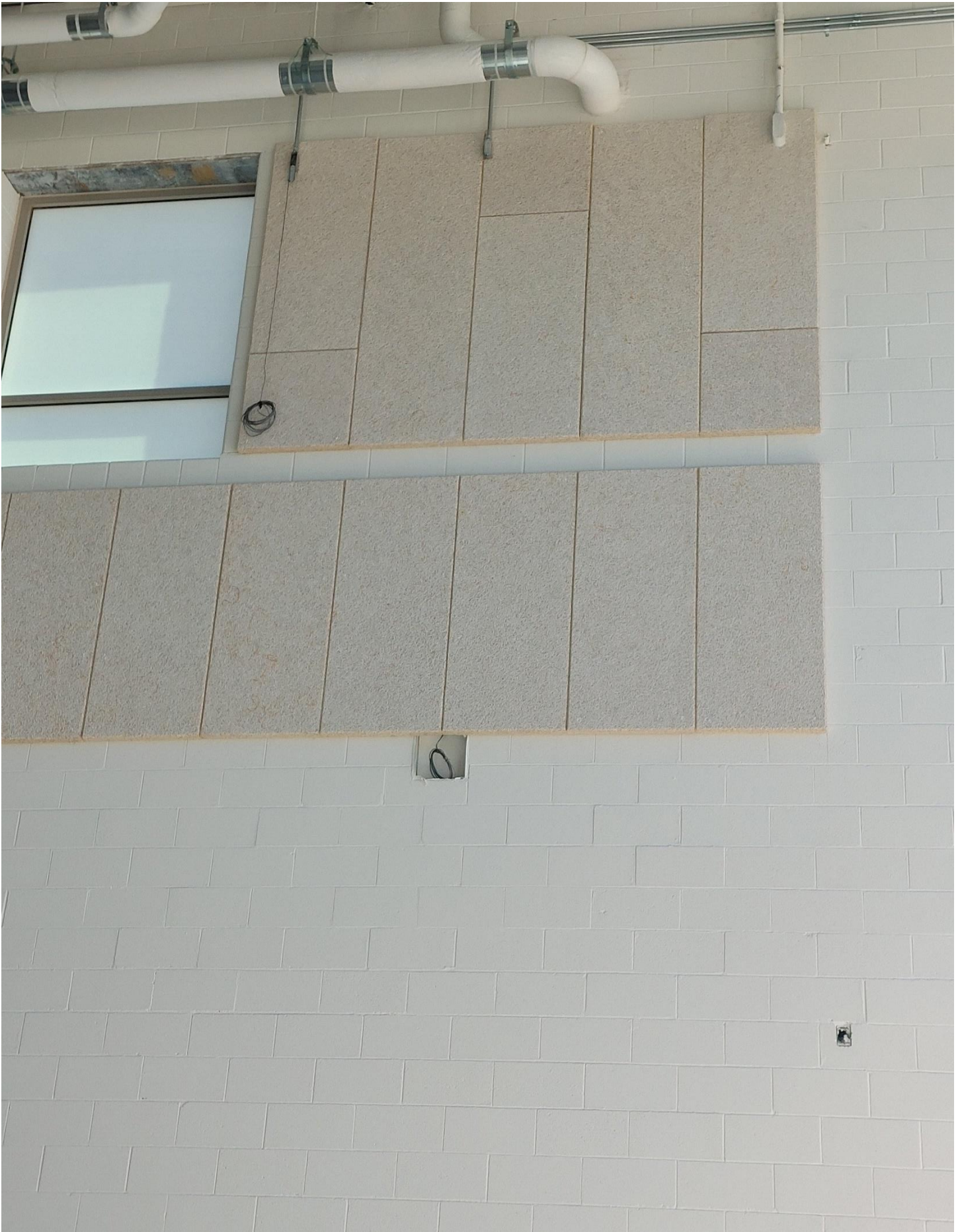
Photo 16 - Acoustical panels in Gym.
