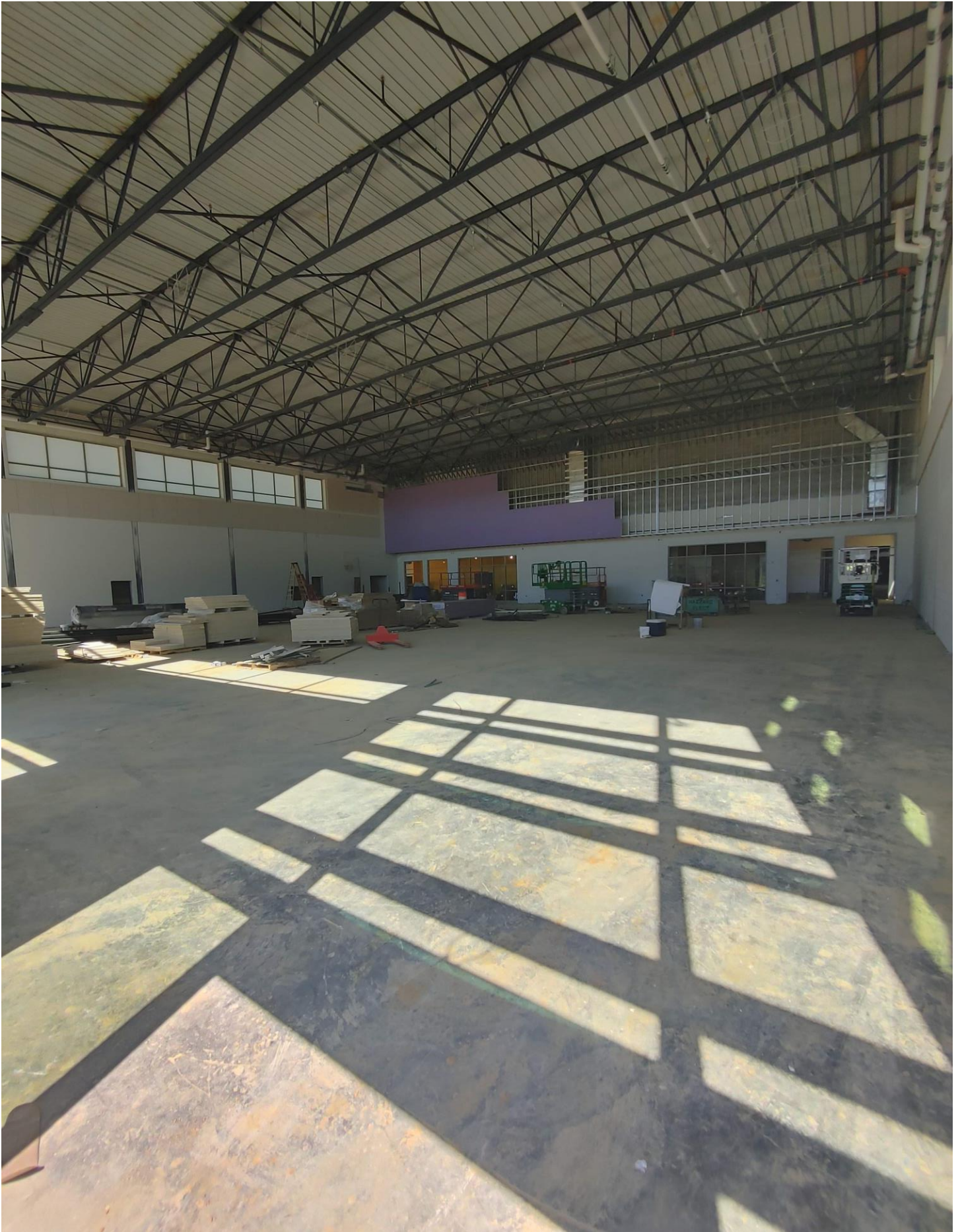
Photo 15 - Gymnasium. Sheetrock is being hung.
