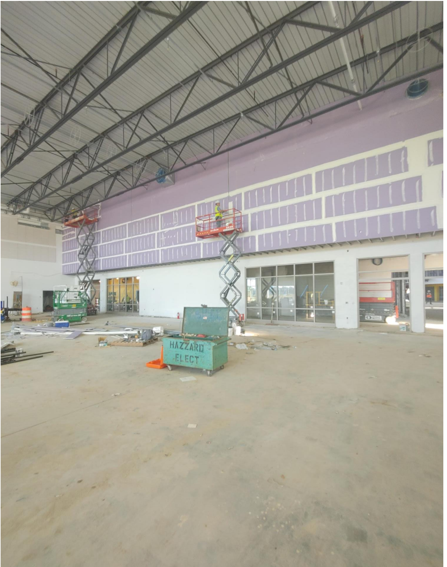
Photo 7 - Sheetrock is being finished in the Gym.
