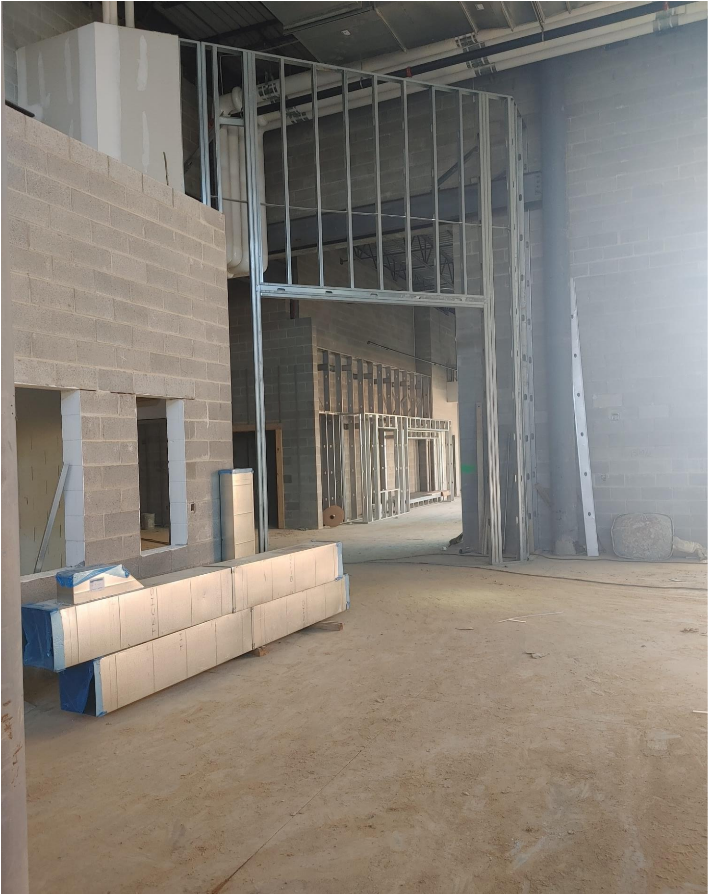
Photo 10 - Metal Studs have been erected between Areas C & D.
