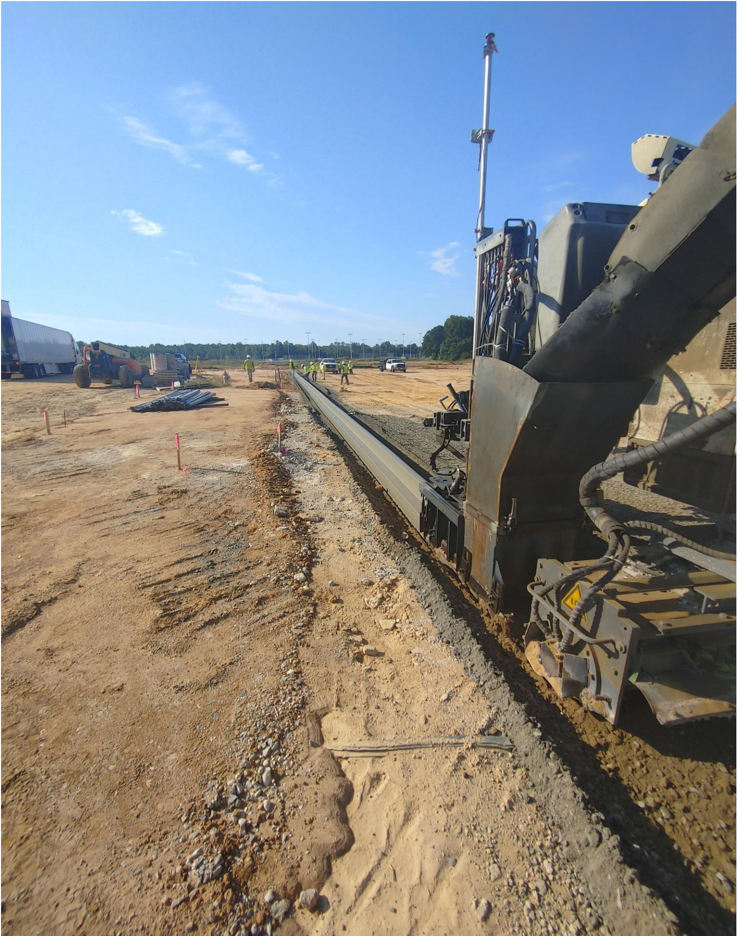
Photo 4 - Curb is being poured in the Bus Loop area.
