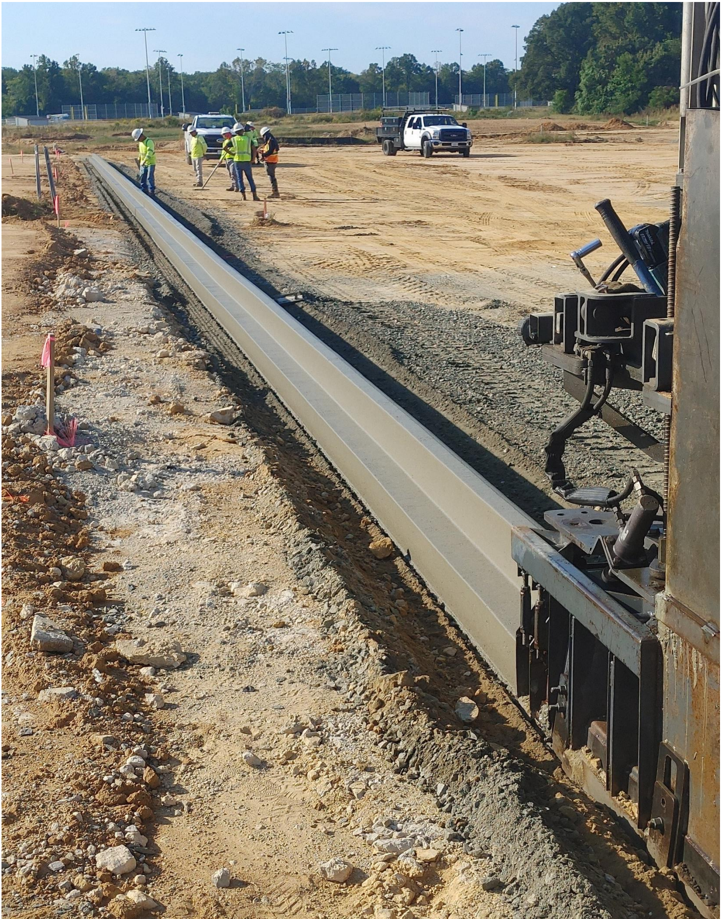
Photo 5 - Curb is being poured in the Bus Loop Area.
