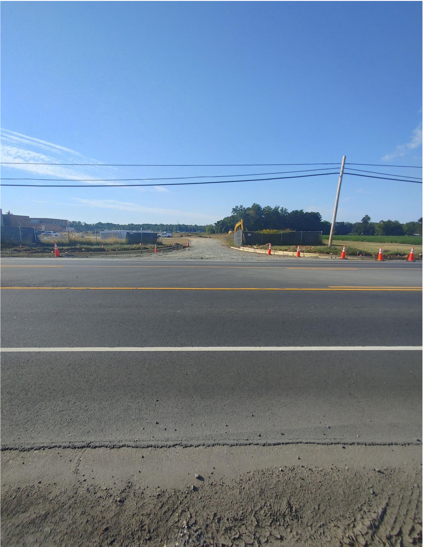
Photo 1 - Bus Loop Entrance Curb & Gutter is being formed
