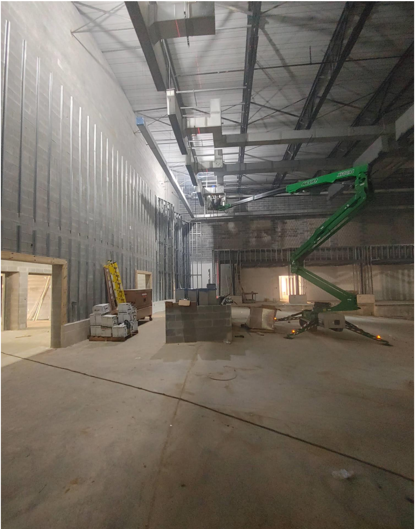
Photo 9 - HVAC Duct is being installed in the Auditorium.
