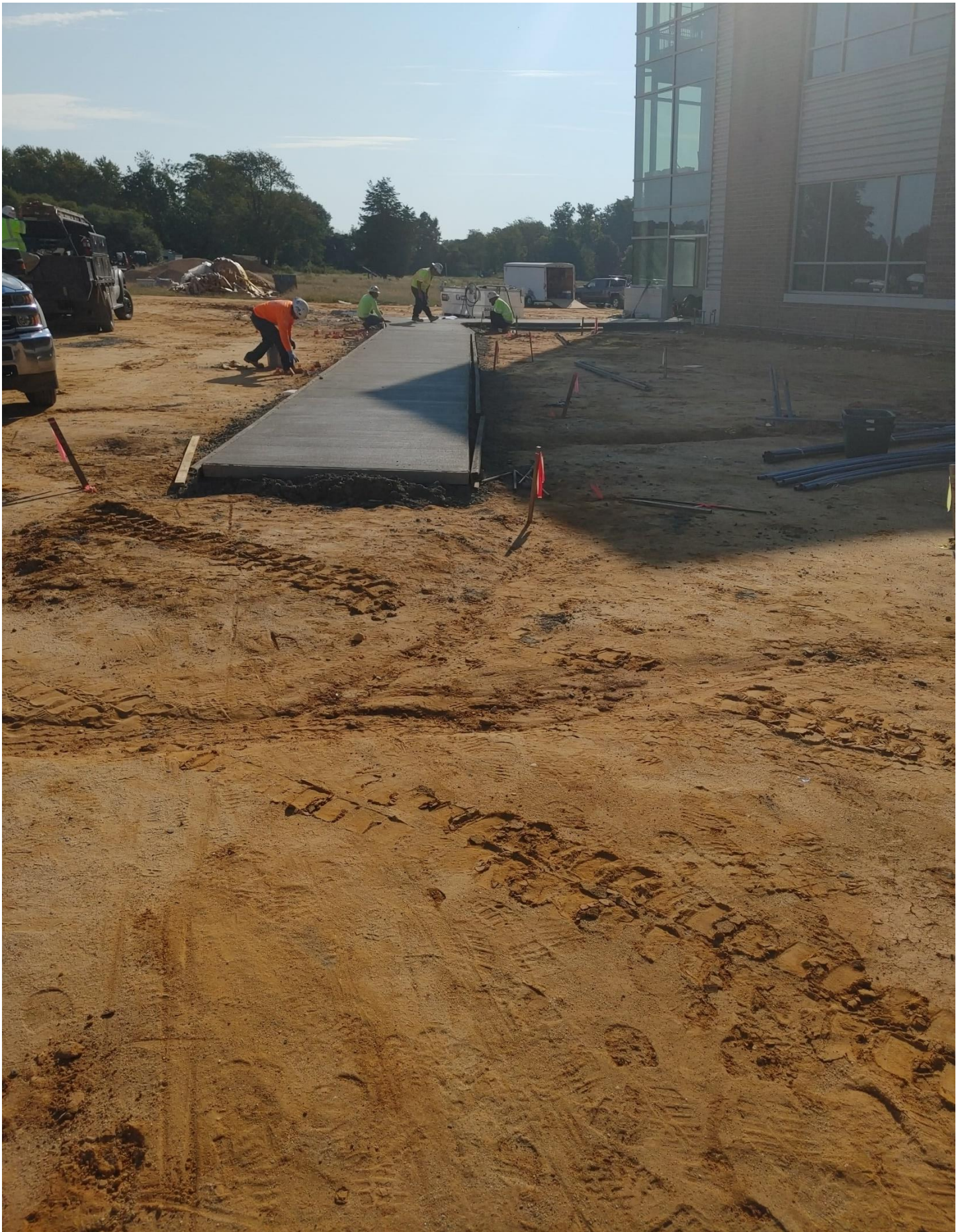
Photo 2 - Sidewalk is being poured in front of Area A.
