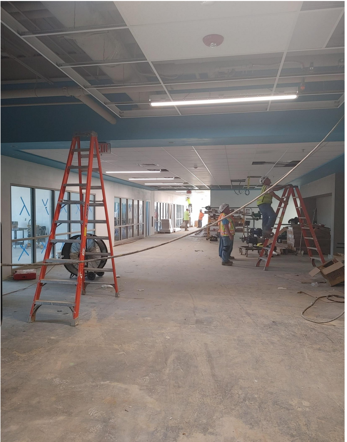
Photo 14 - Lighting installed and energized in Area A, 1st floor.
