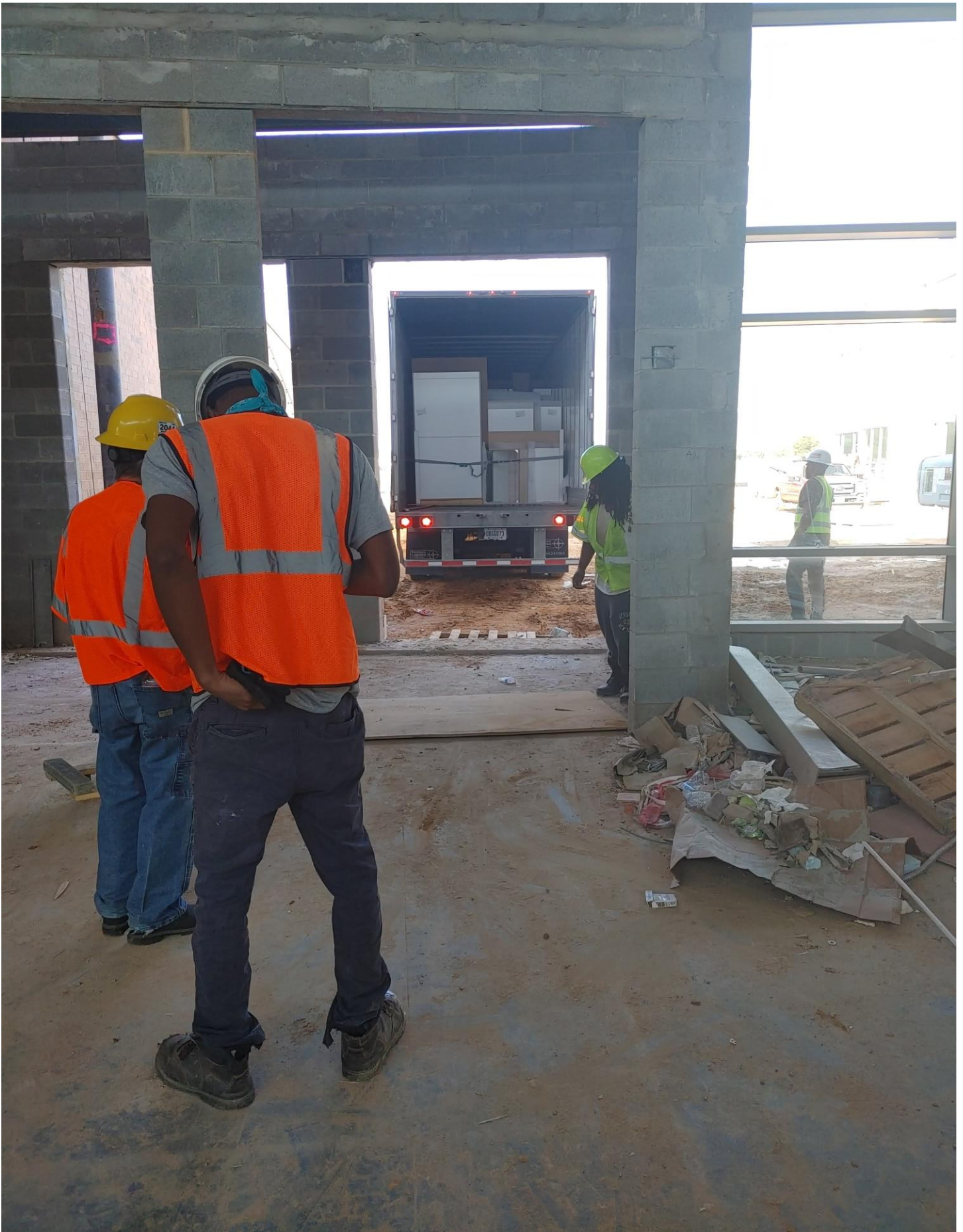
Photo 6 - Millwork delivery is being unloaded.
