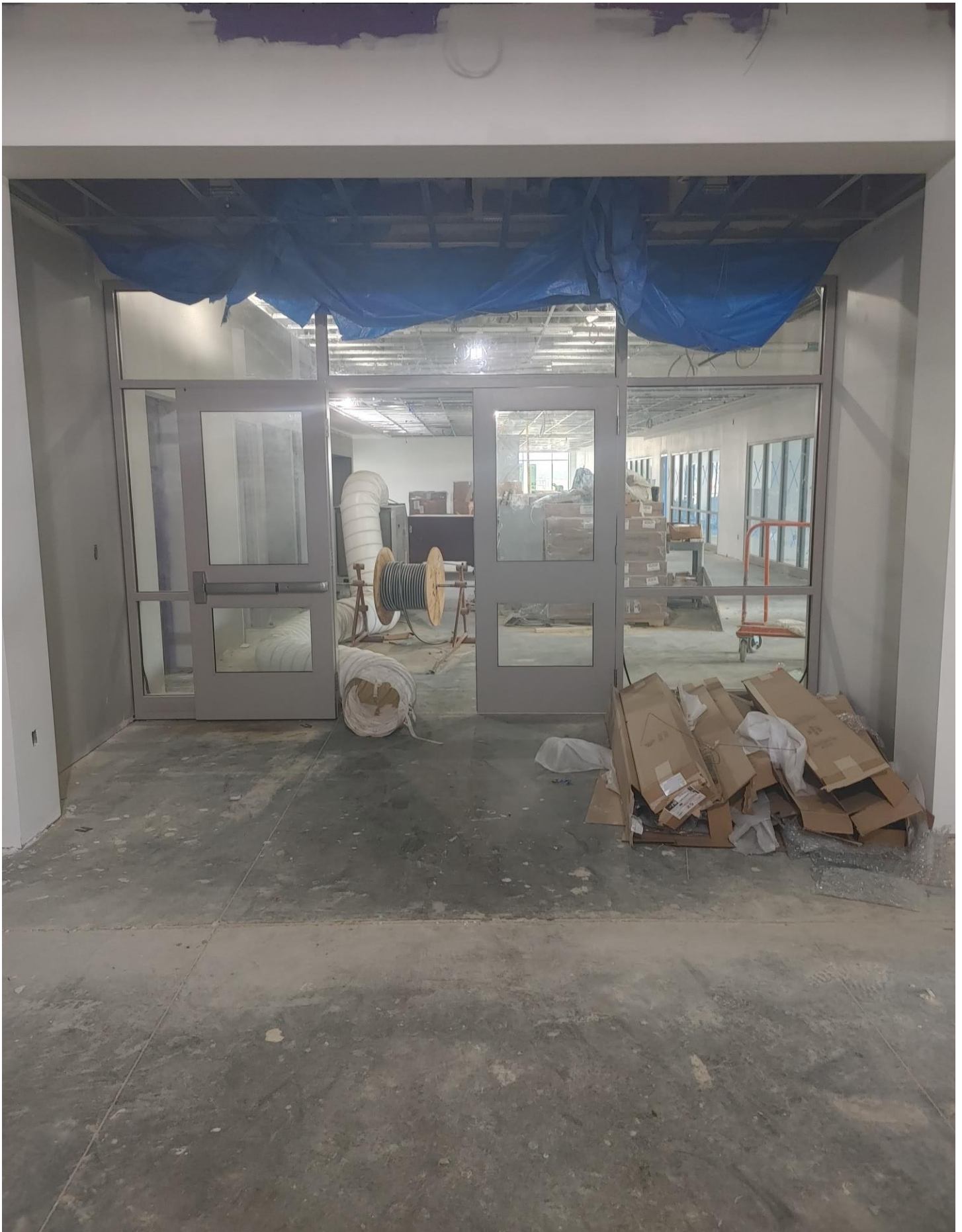
Photo 14 - SF53B has been completely installed
