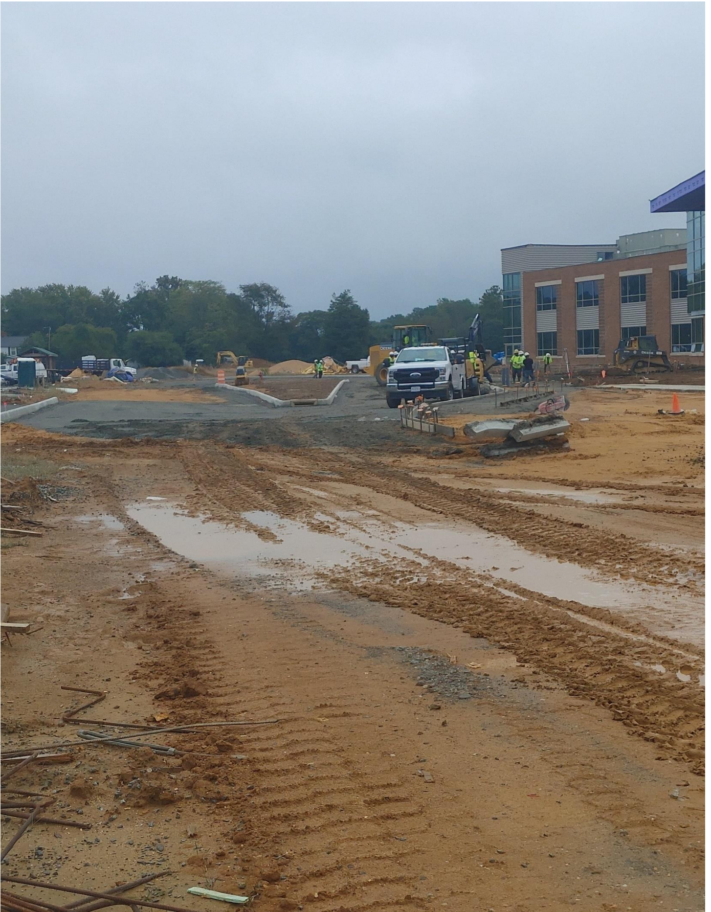
Photo 3 - Curb work continues in front of the School.
