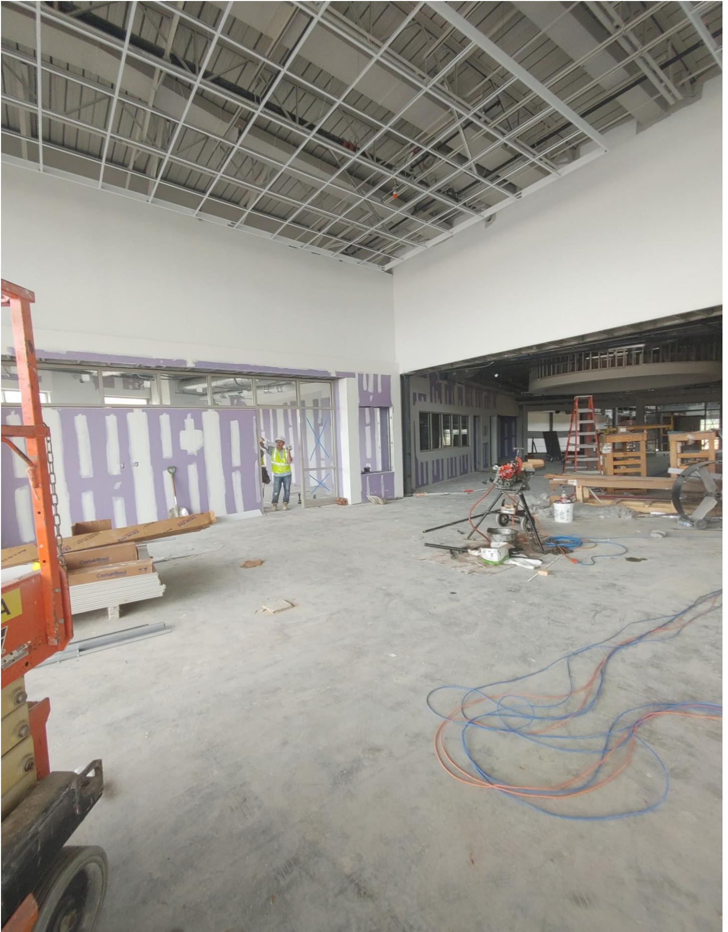
Photo 16 - Sheetrock is being finished on the 2nd floor of Area A
