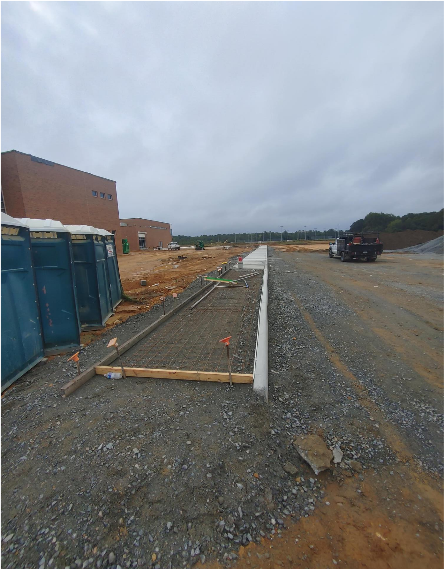
Photo 5 - Bus Loop Sidewalk prep and forms continues
