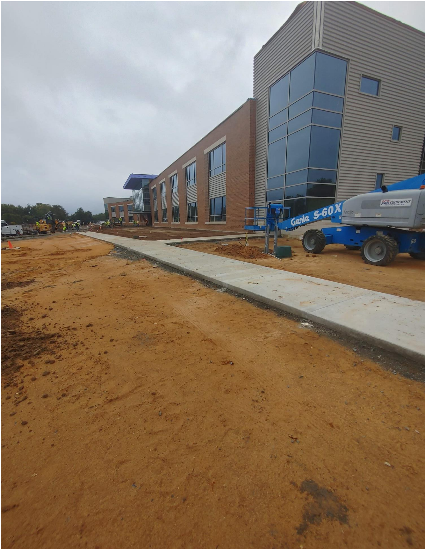
Photo 4 - Sidewalks have been poured in front of Area B
