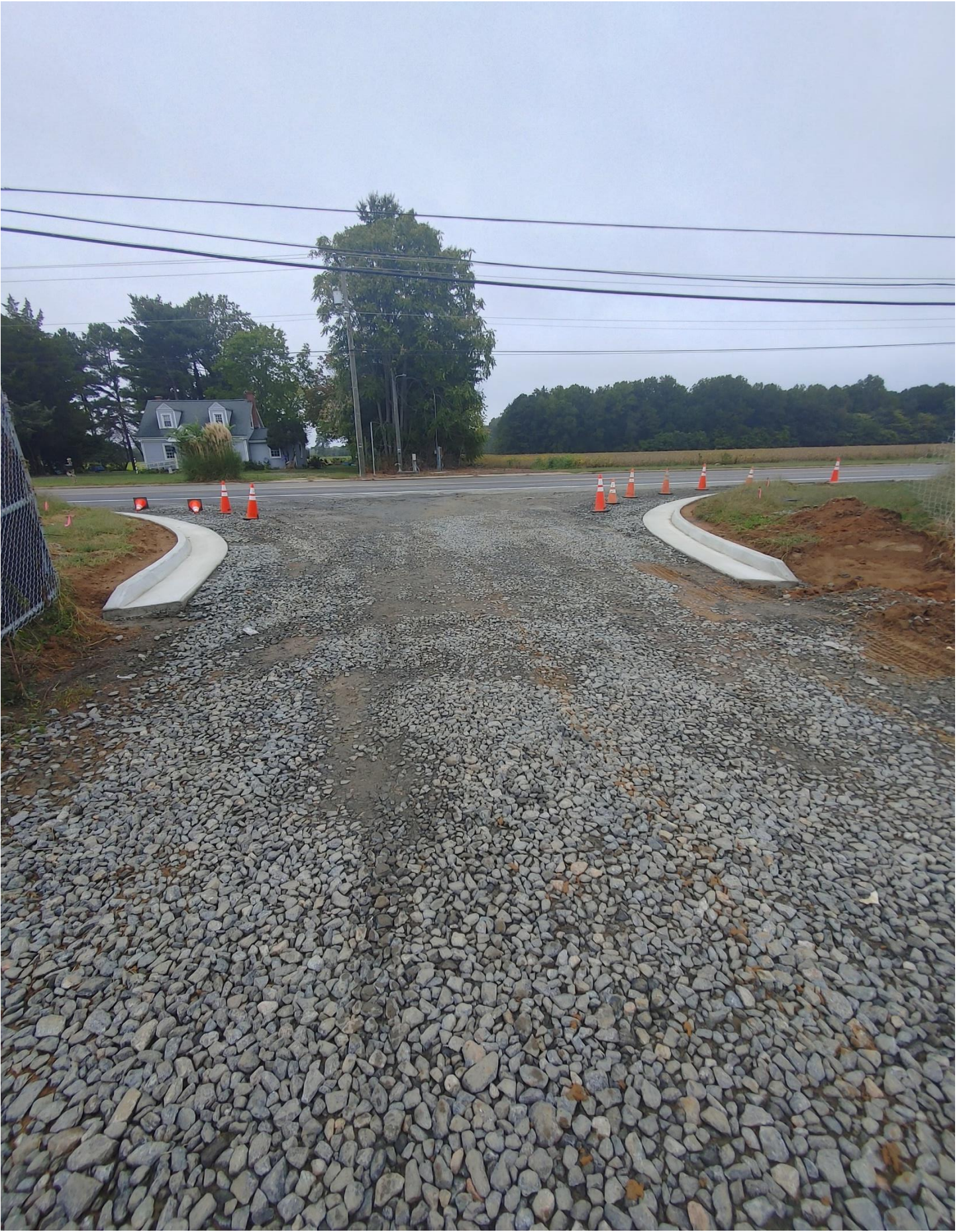
Photo 1 - Bus Loop Entrance Curb and Gutter has been installed
