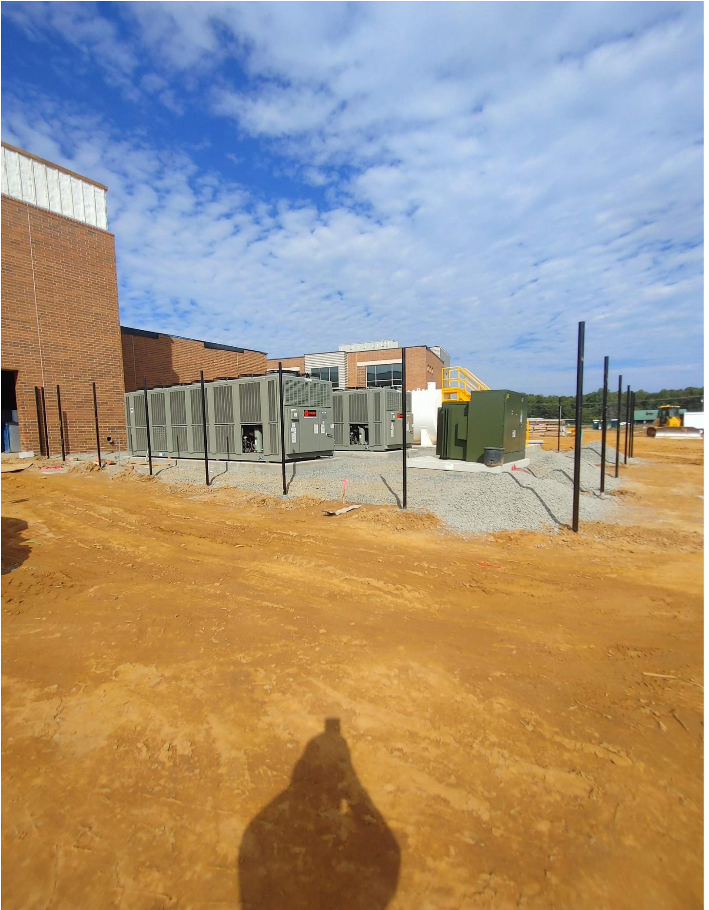
Photo 9 - Fence Posts have been installed
