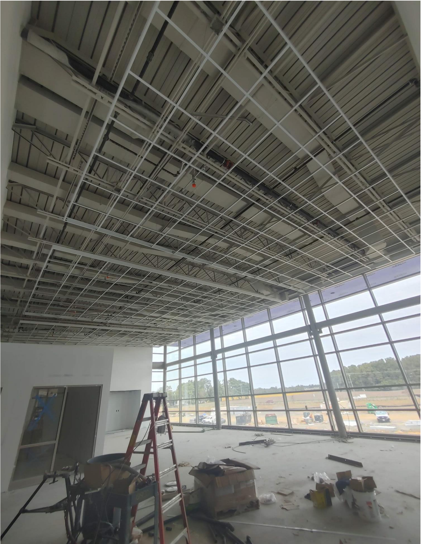
Photo 20 - Track has been installed for Cloud Ceiling in Area A
