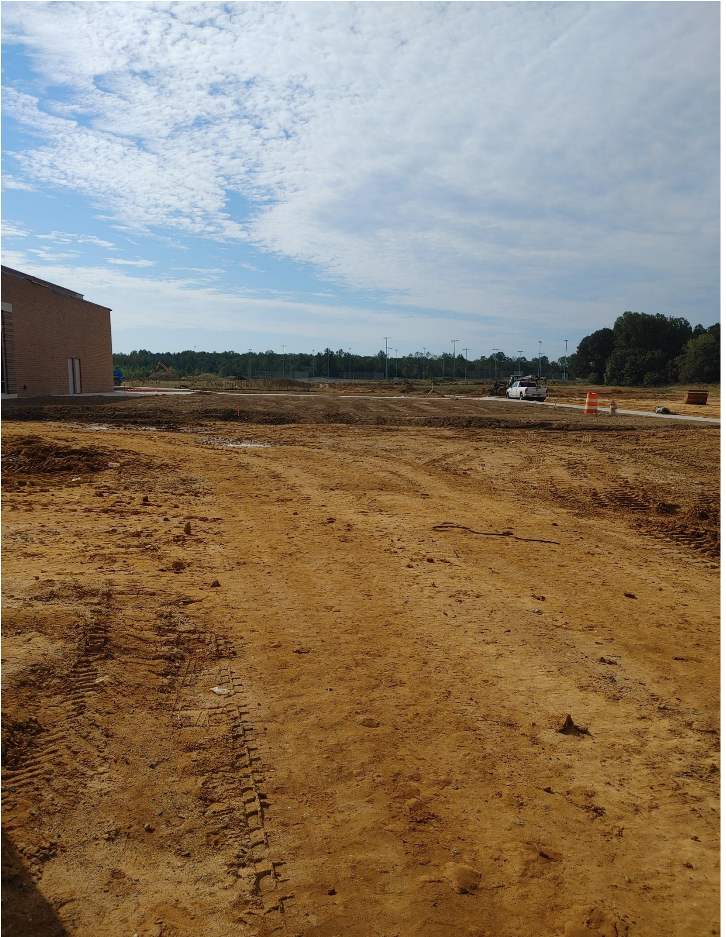
Photo 5 - Topsoil is being spread on the West side of Area E
