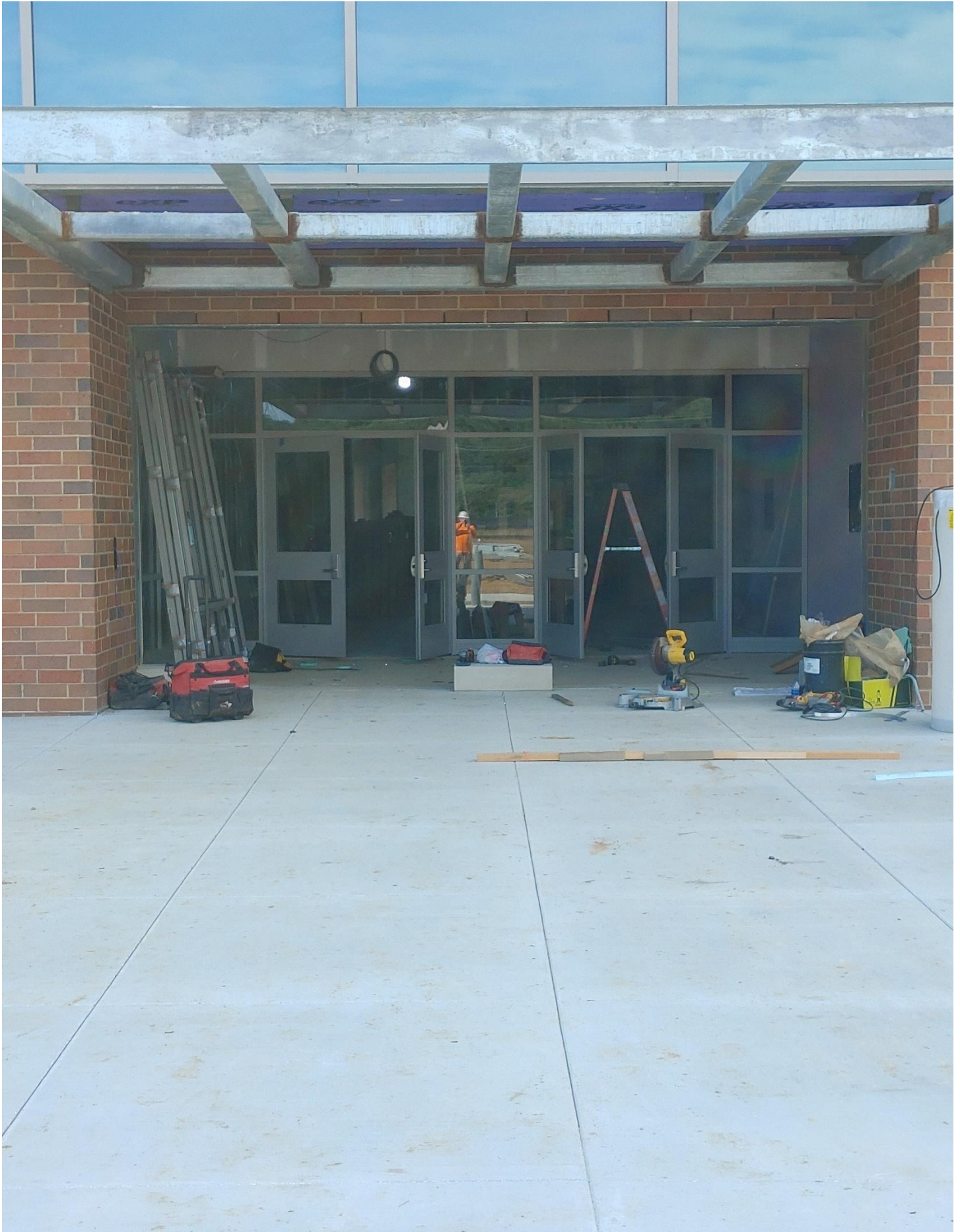
Photo 3 - Front Doors are being installed
