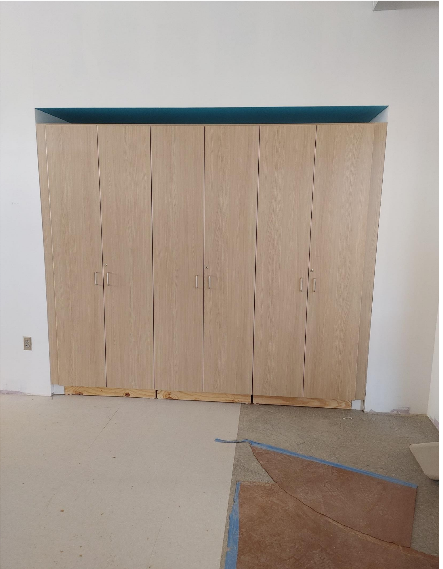
Photo 13 - Cabinetry in A105
