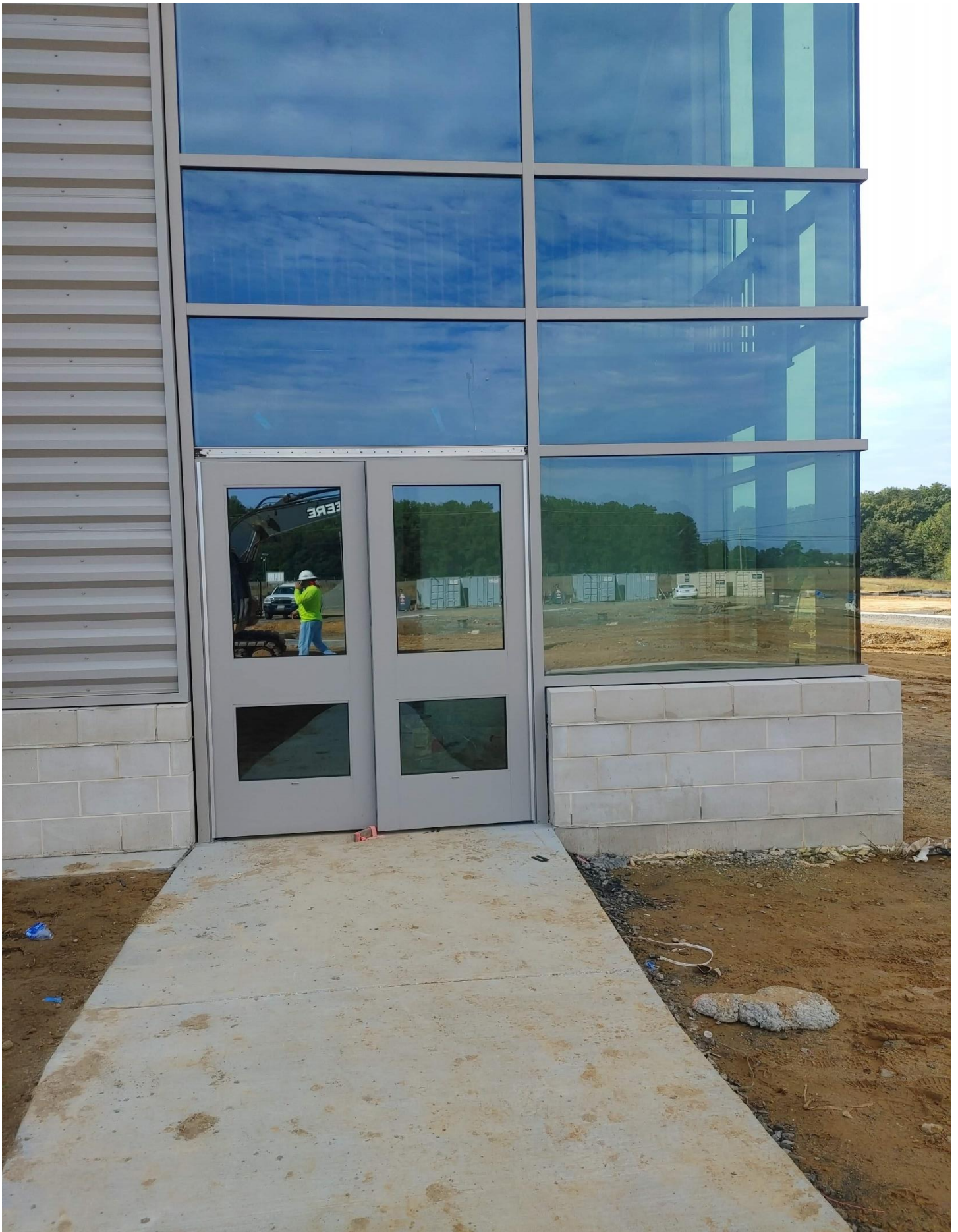
Photo 4 - Doors on Stairwell #2 have been installed
