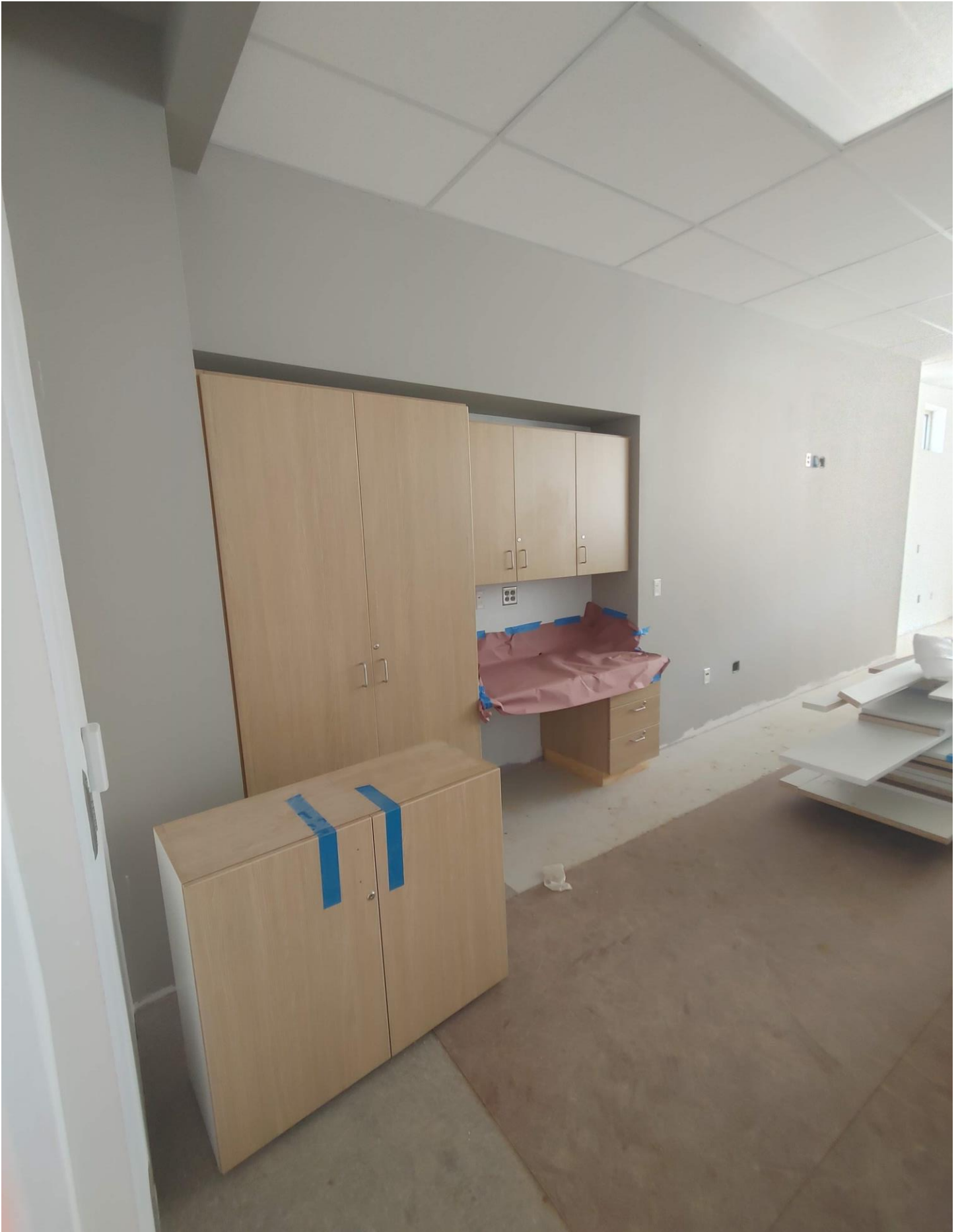
Photo 12 - Cabinetry has been installed in A105
