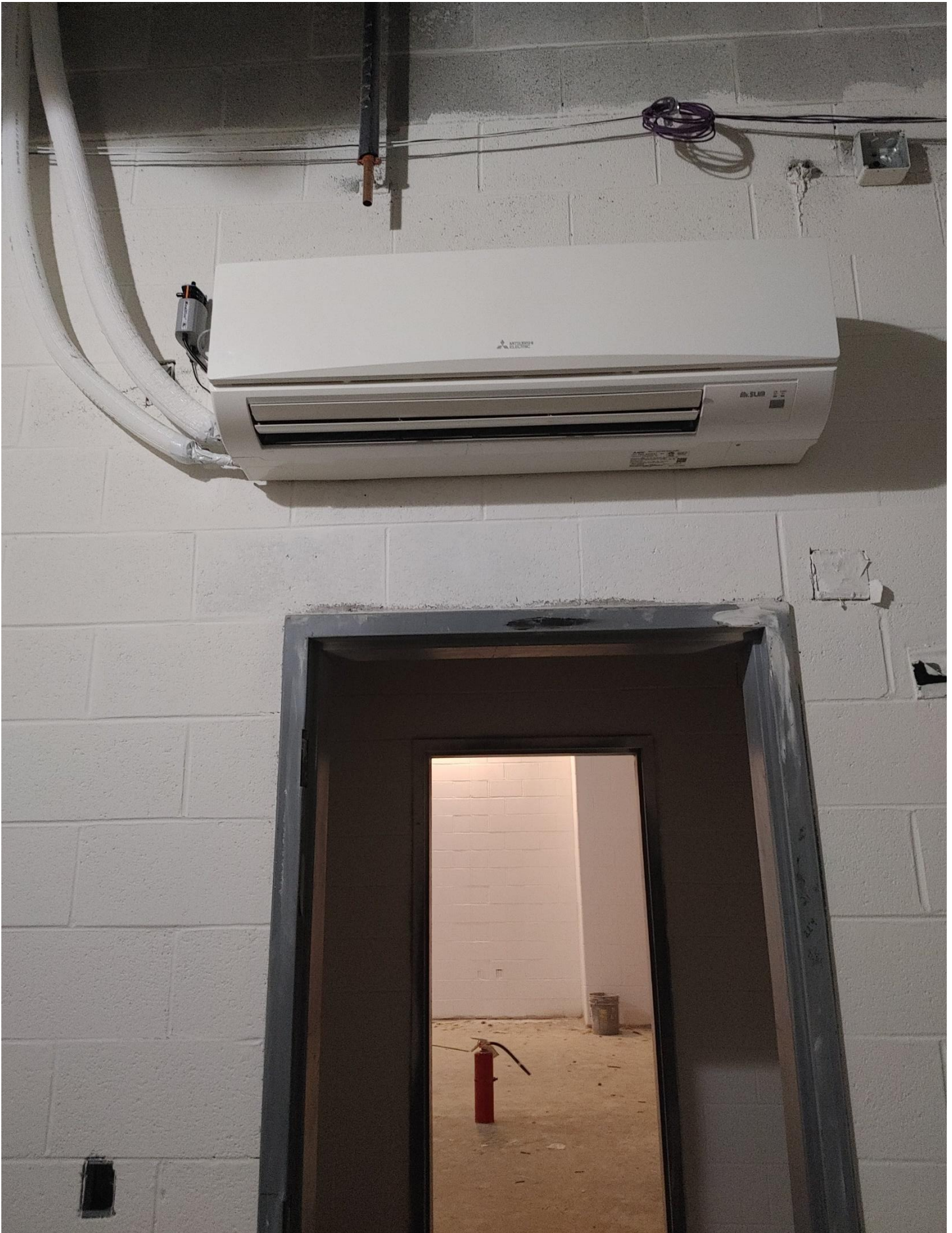
Photo 17 - Mitsubishi Head unit install almost on Door Frame D131.
