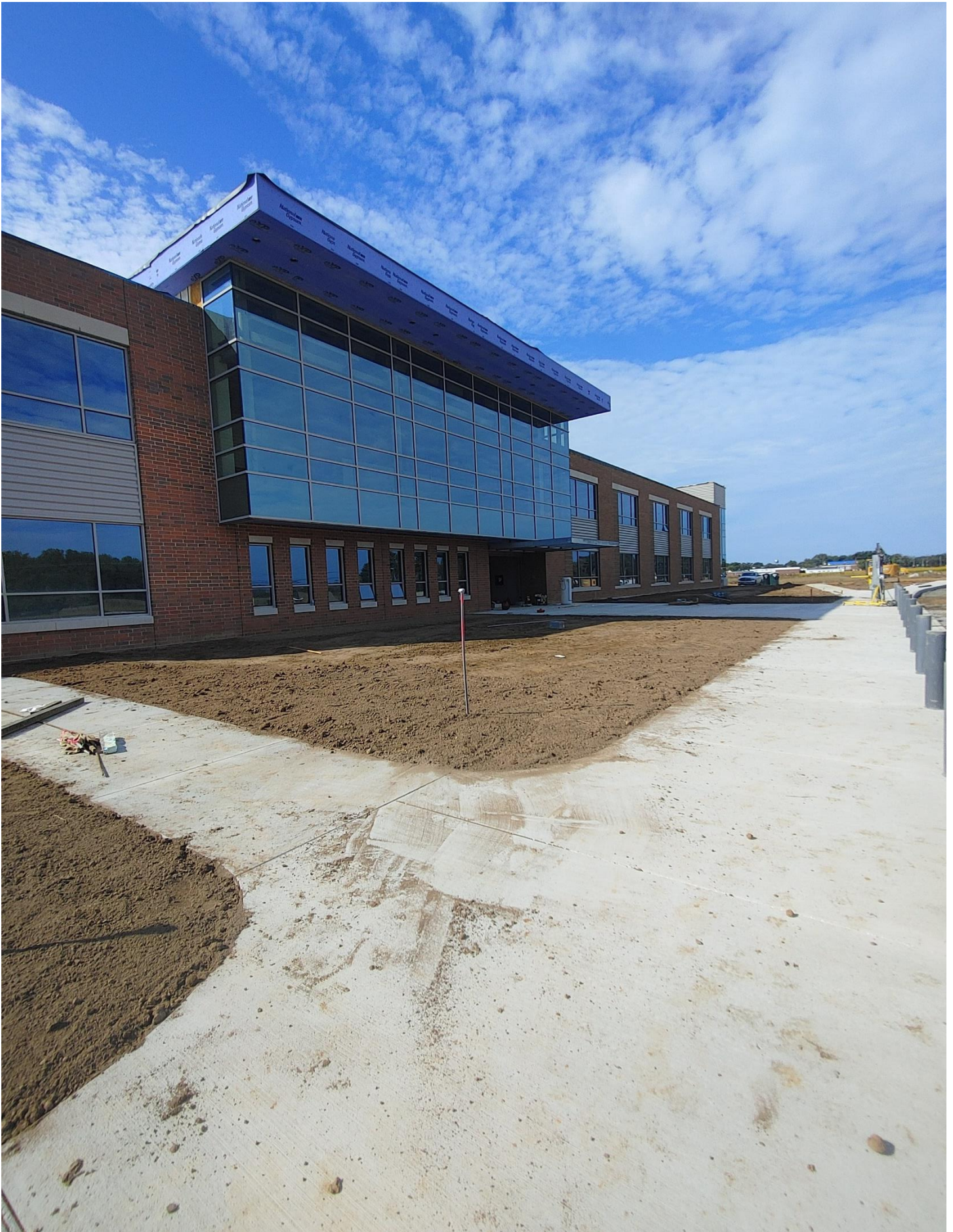
Photo 2 - Top Soil in being spread & Bollards have been installed.
