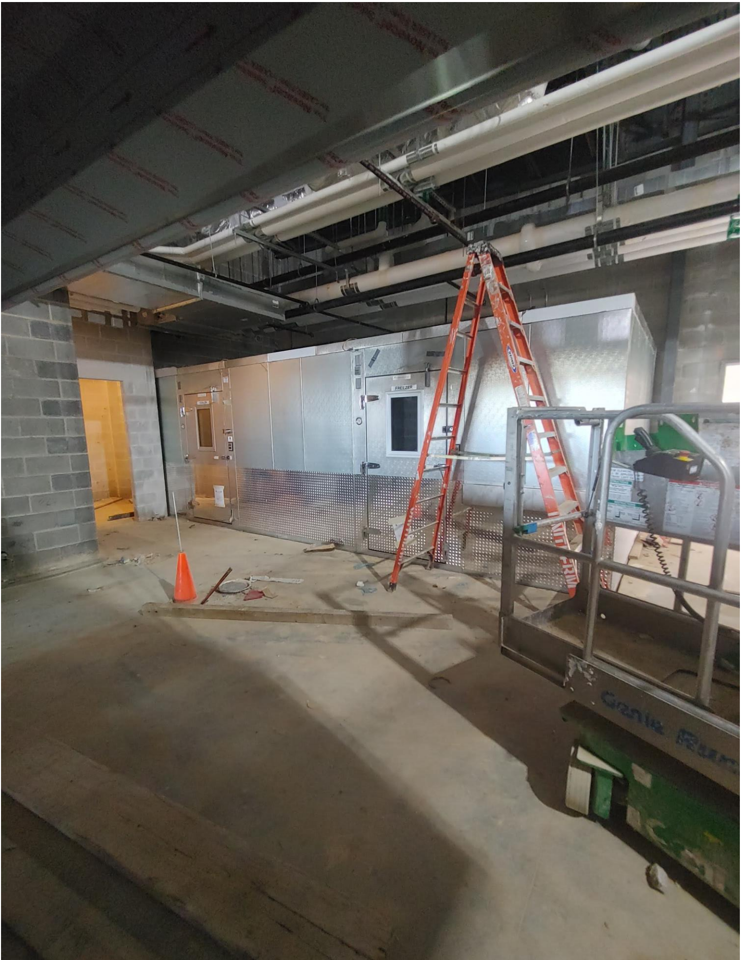
Photo 15 - Cooler and Freezer have been installed
