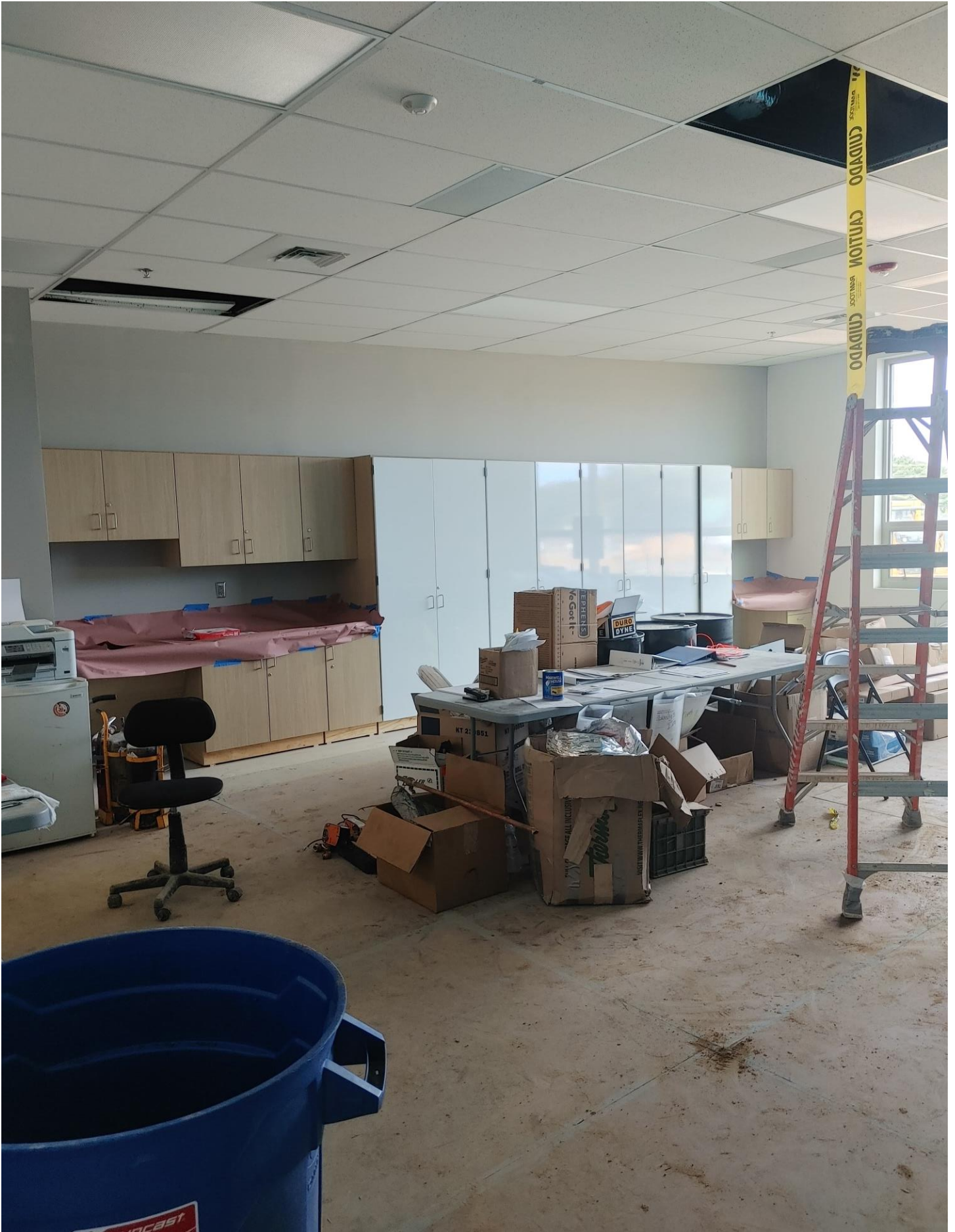
Photo 14 - Cabinetry installed in A103
