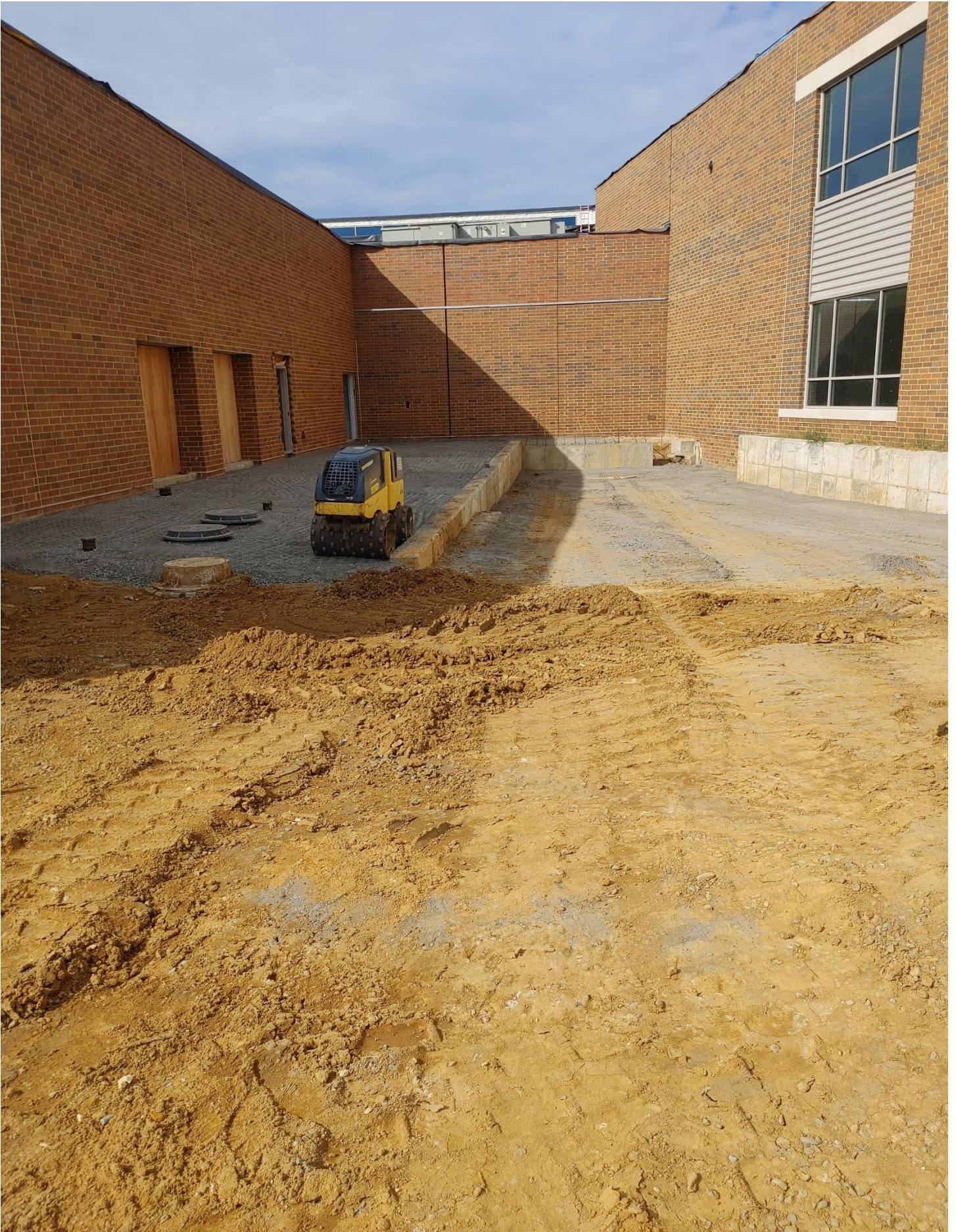
Photo 10 - Load Dock Area is being prepped for Concrete
