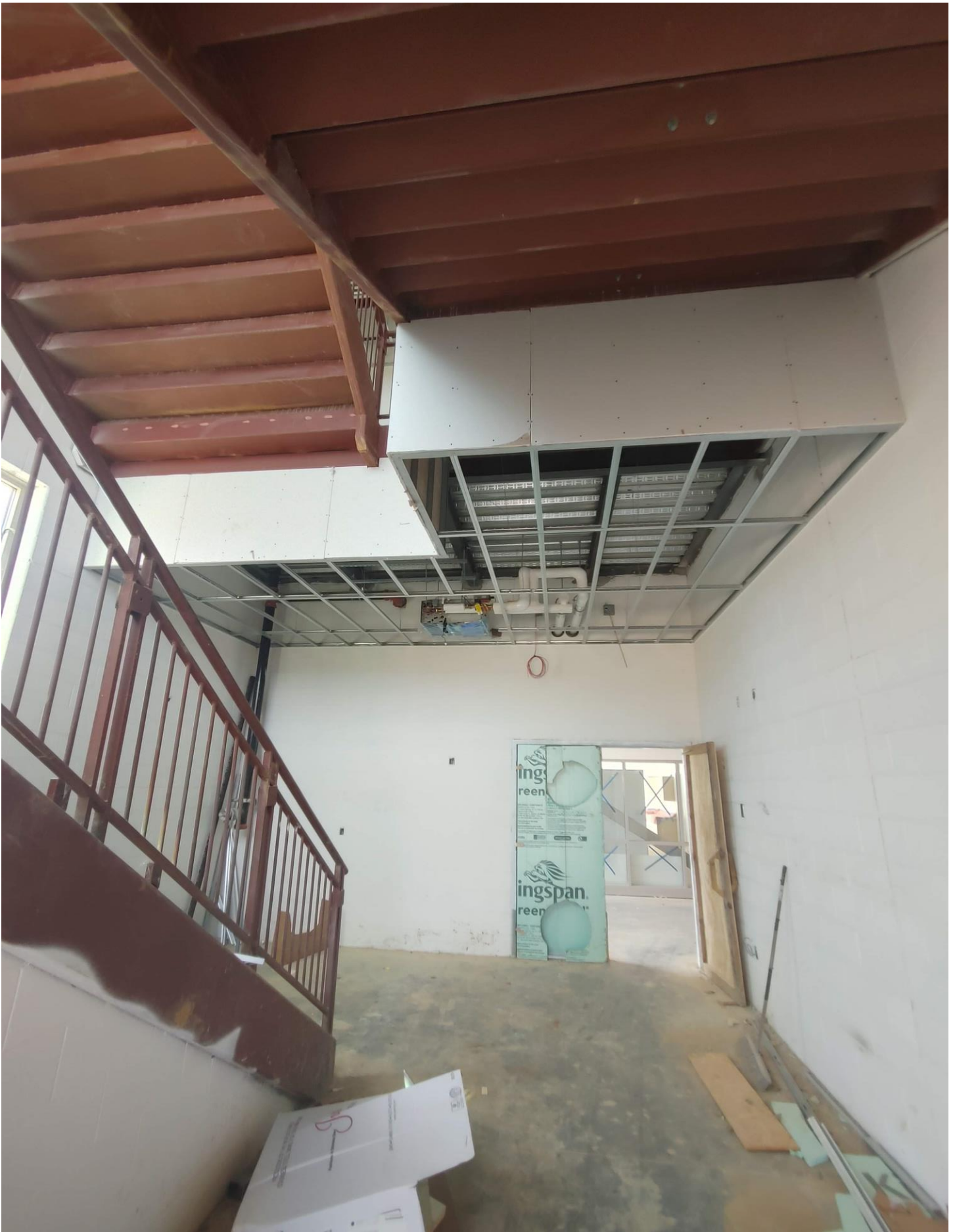
Photo 11 - Sheetrock hung on Bulkhead in Stairwell #1
