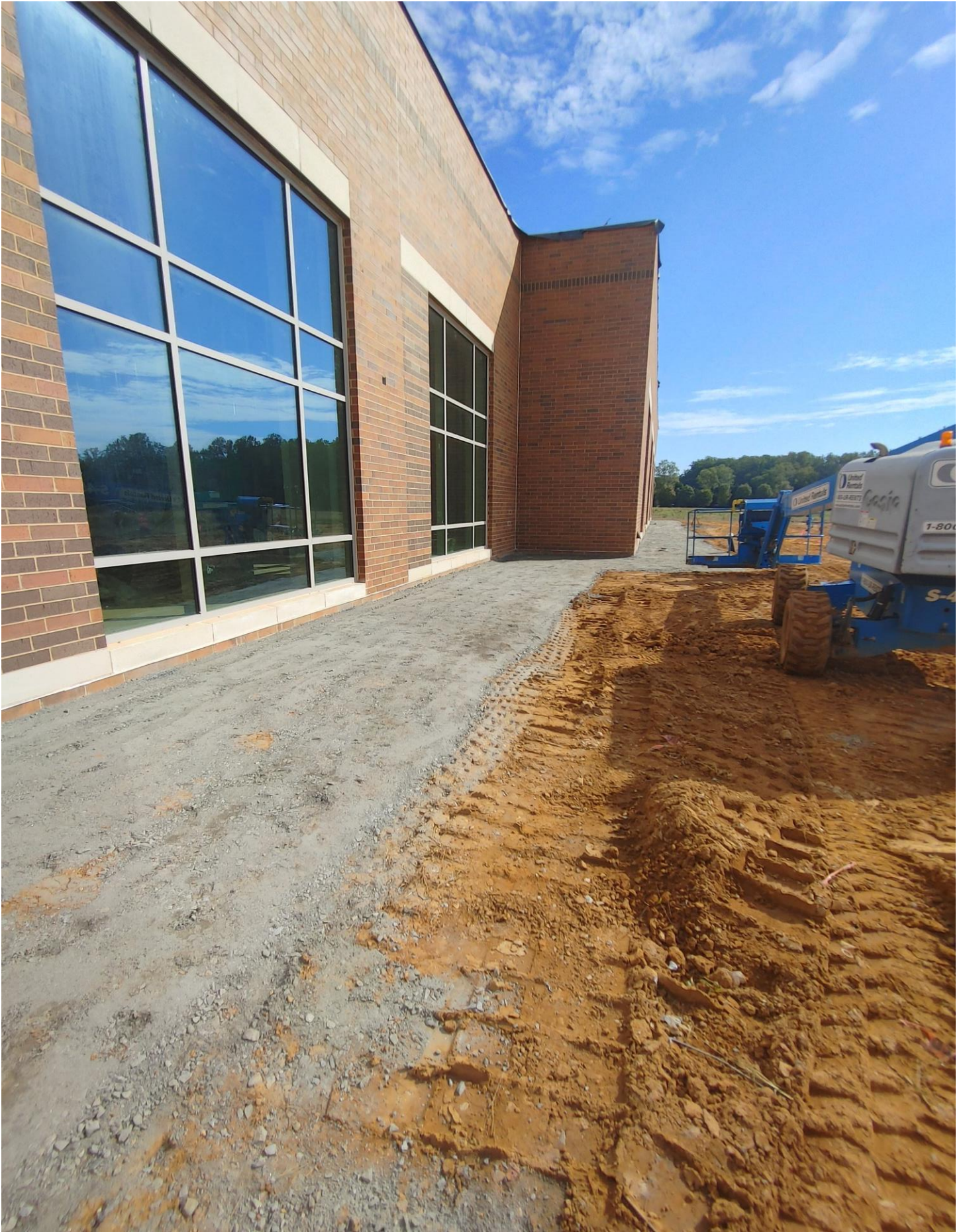
Photo 8 - South side of Area D prepped for Concrete
