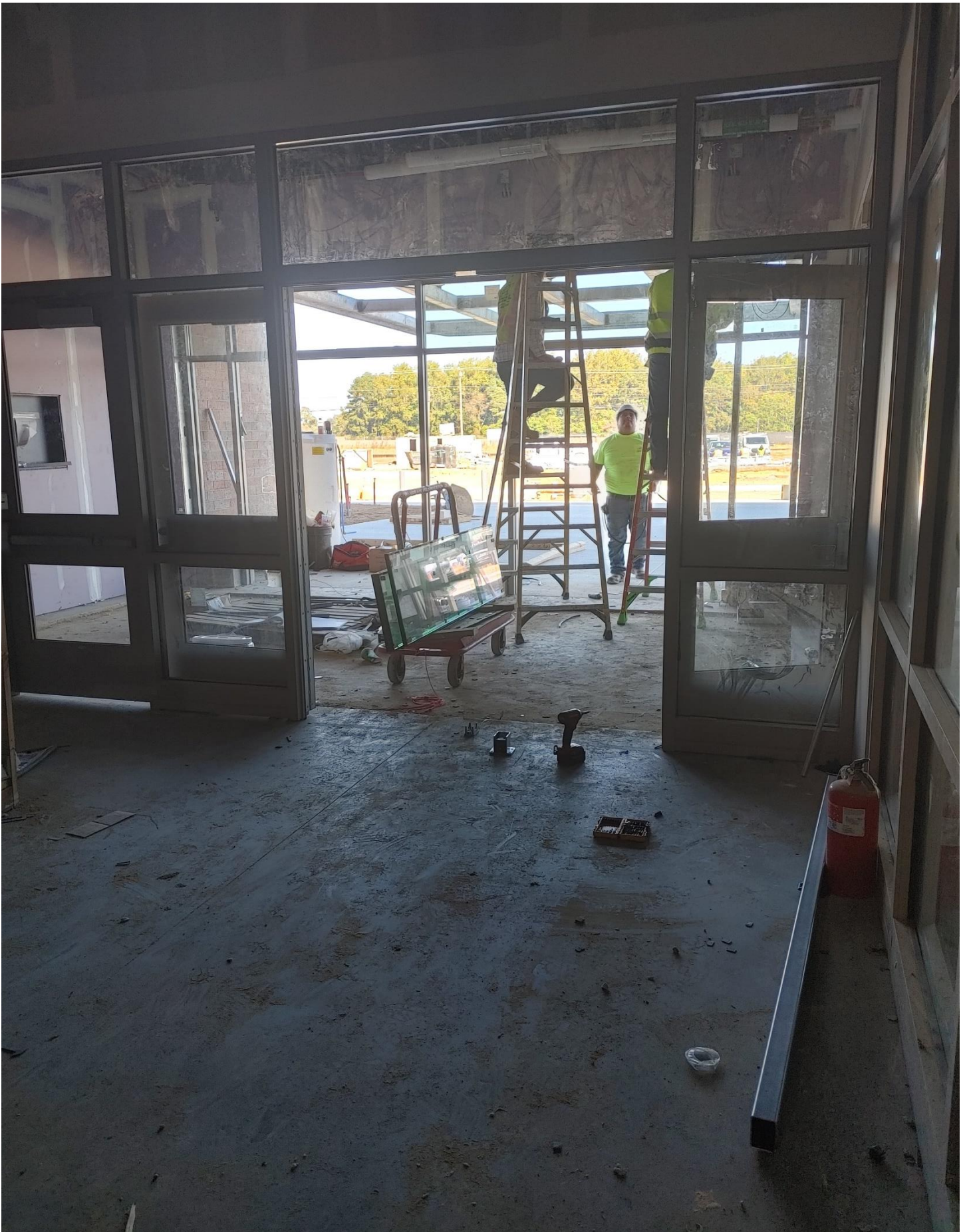
Photo 10 - FG&M is working on SF69
