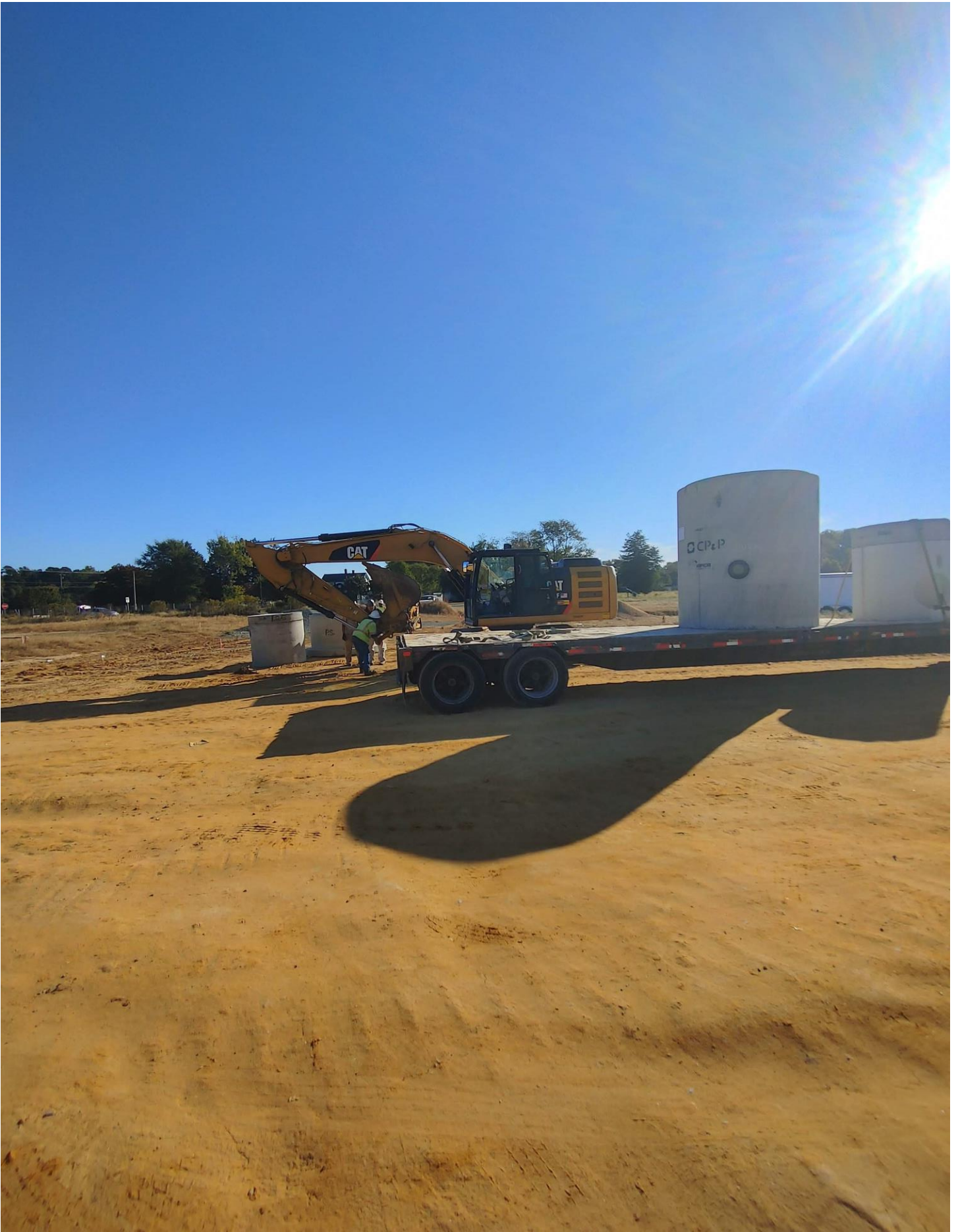
Photo 1 - Sewage Tank is being off loaded
