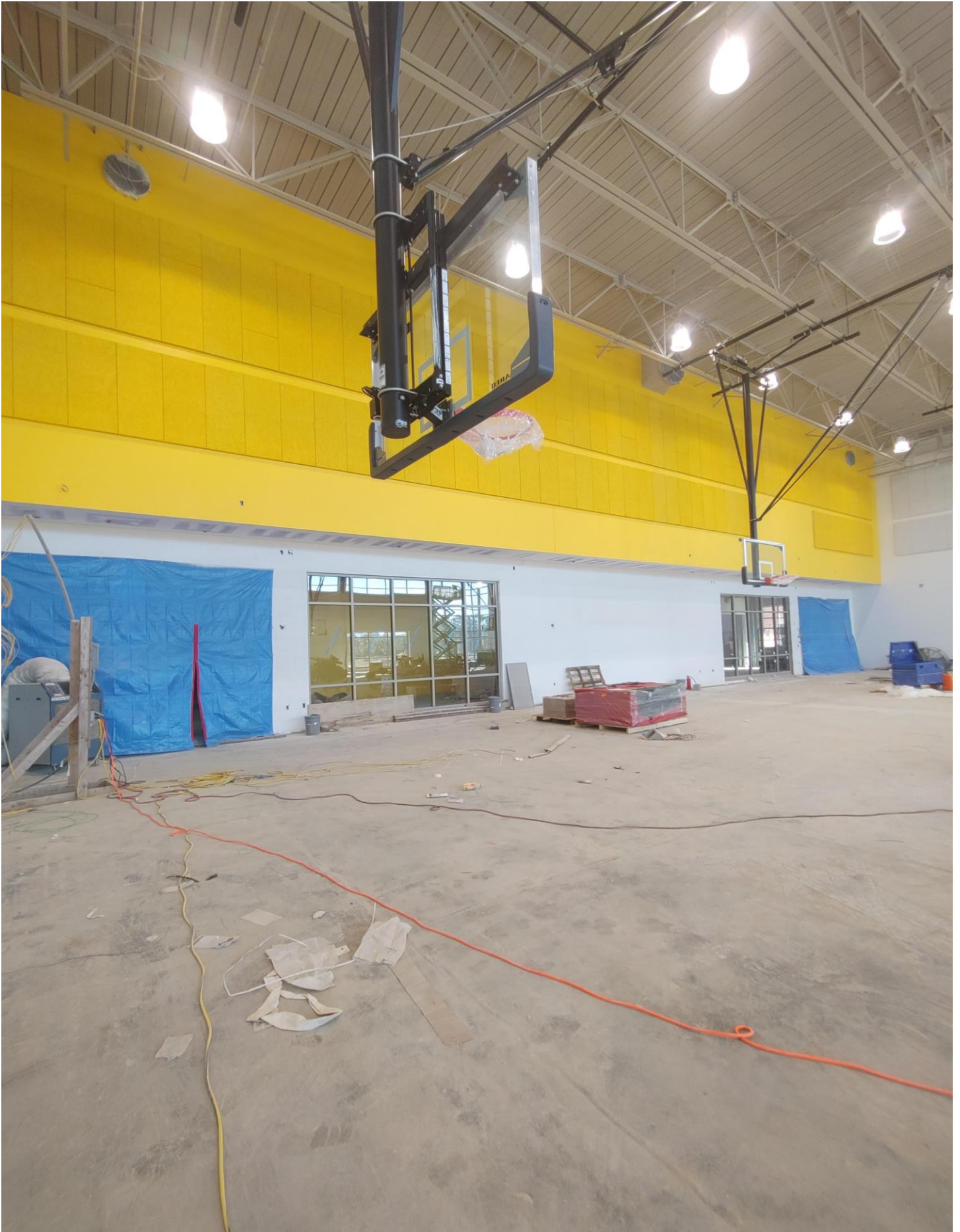
Photo 6 - North wall of Gym has received a coat of paint.
