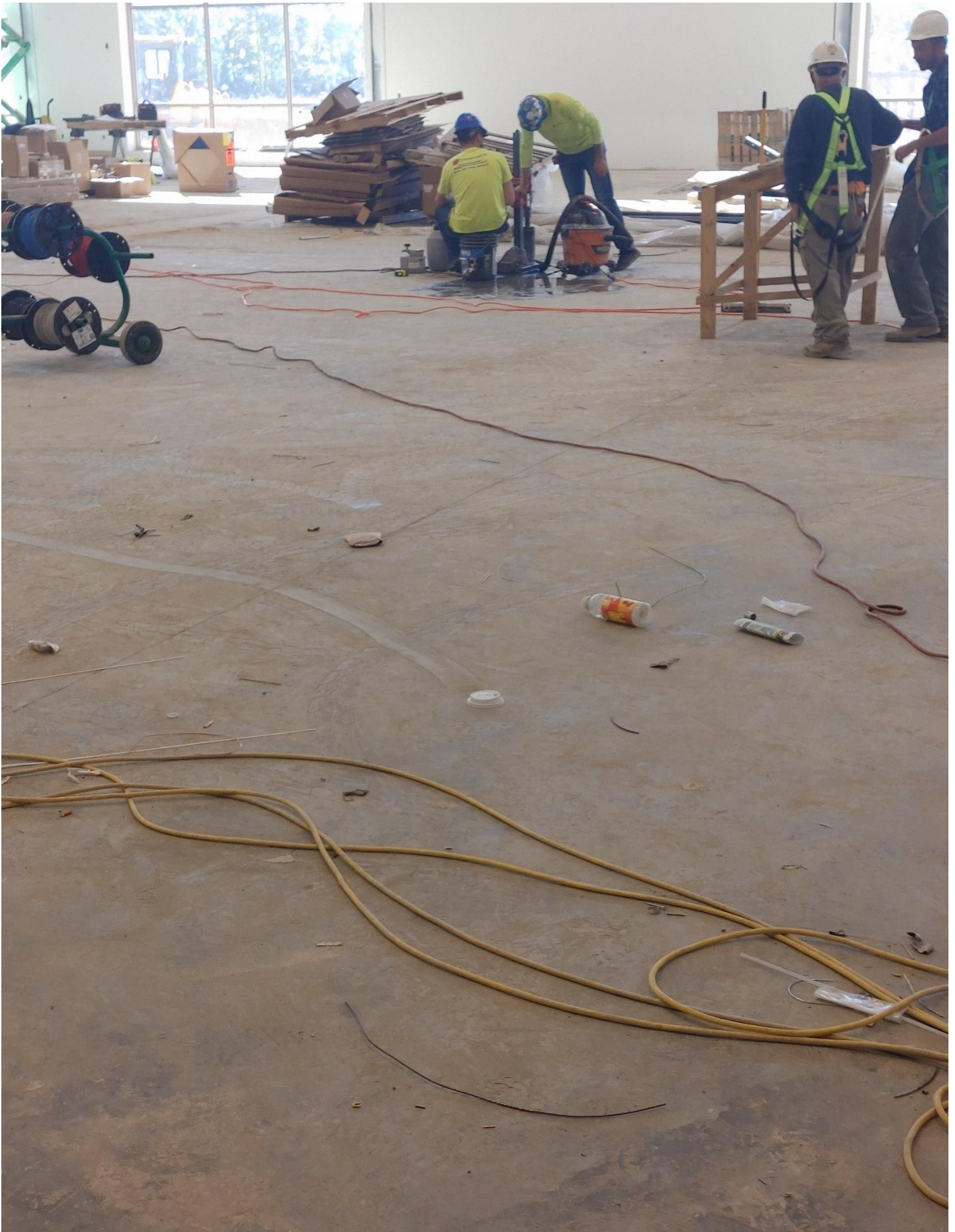
Photo 5 - Gym Floor is being cored for Volley Ball Pole Sleeves.
