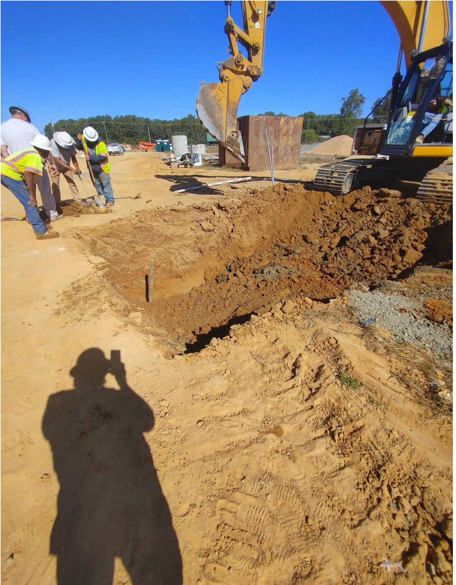
Photo 13 - Excavation for the Sewage Tank has begun.
