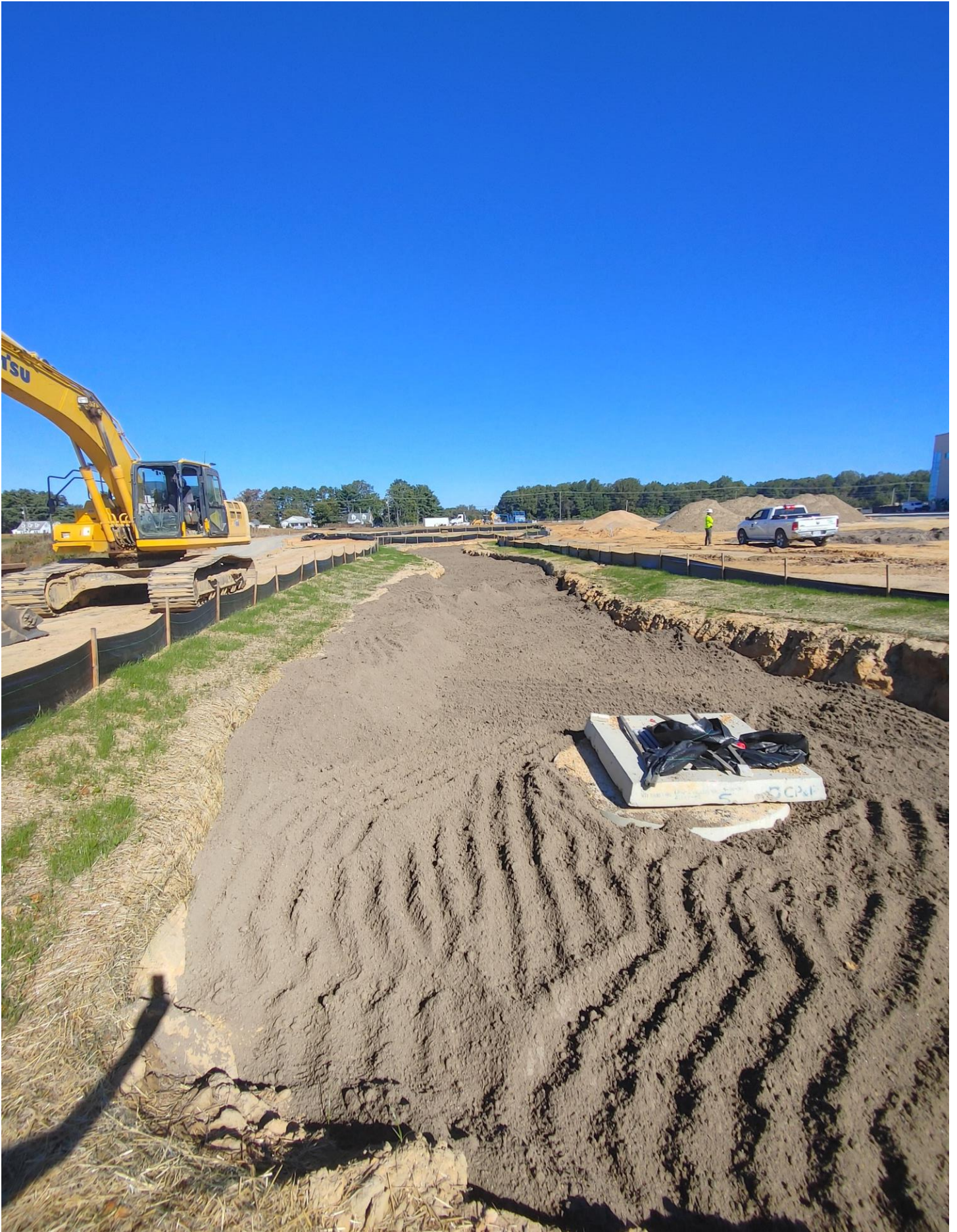
Photo 8 - First lift of Bio Material has been installed.
