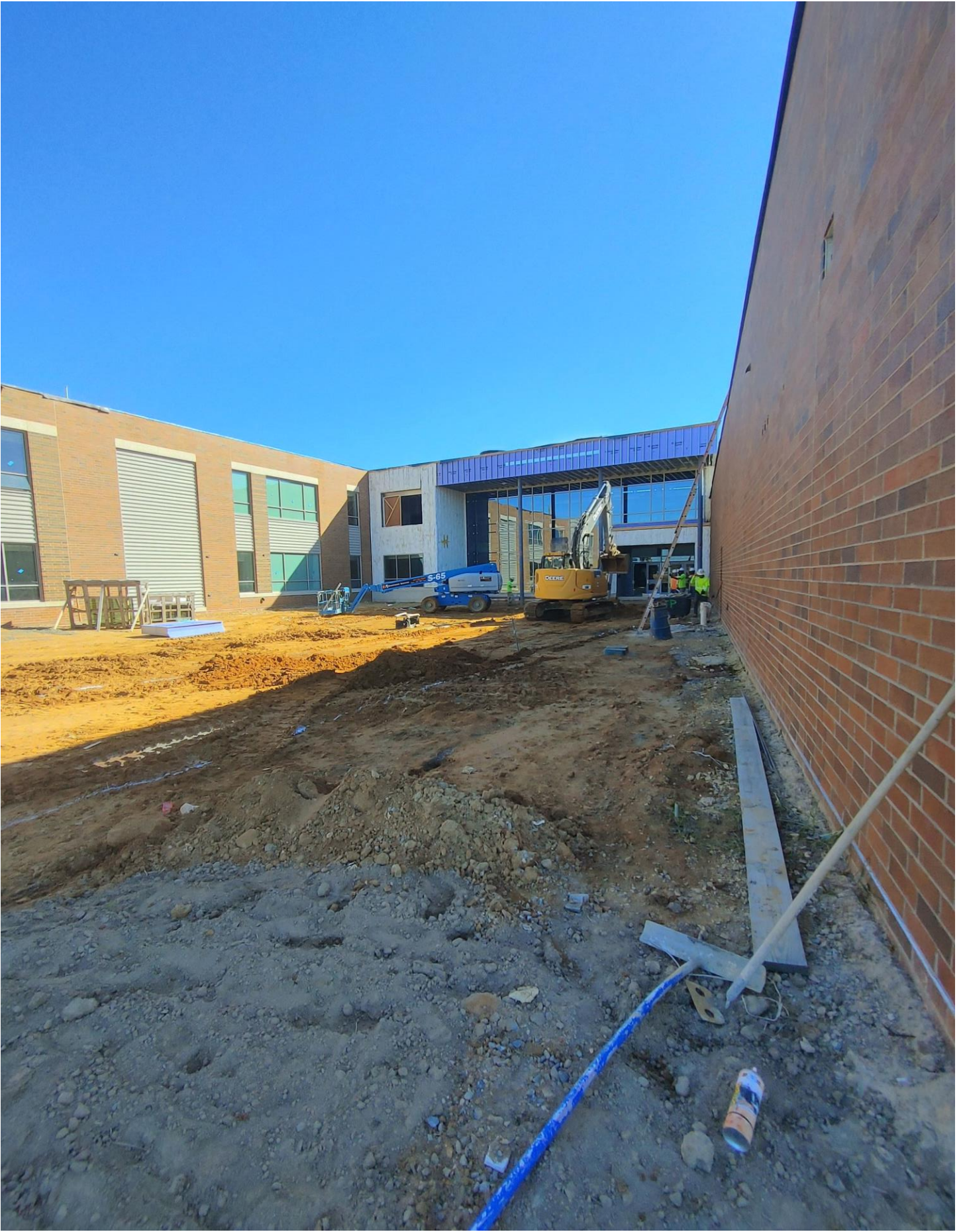
Photo 7 - Beuchert is working on the West side of Area C.
