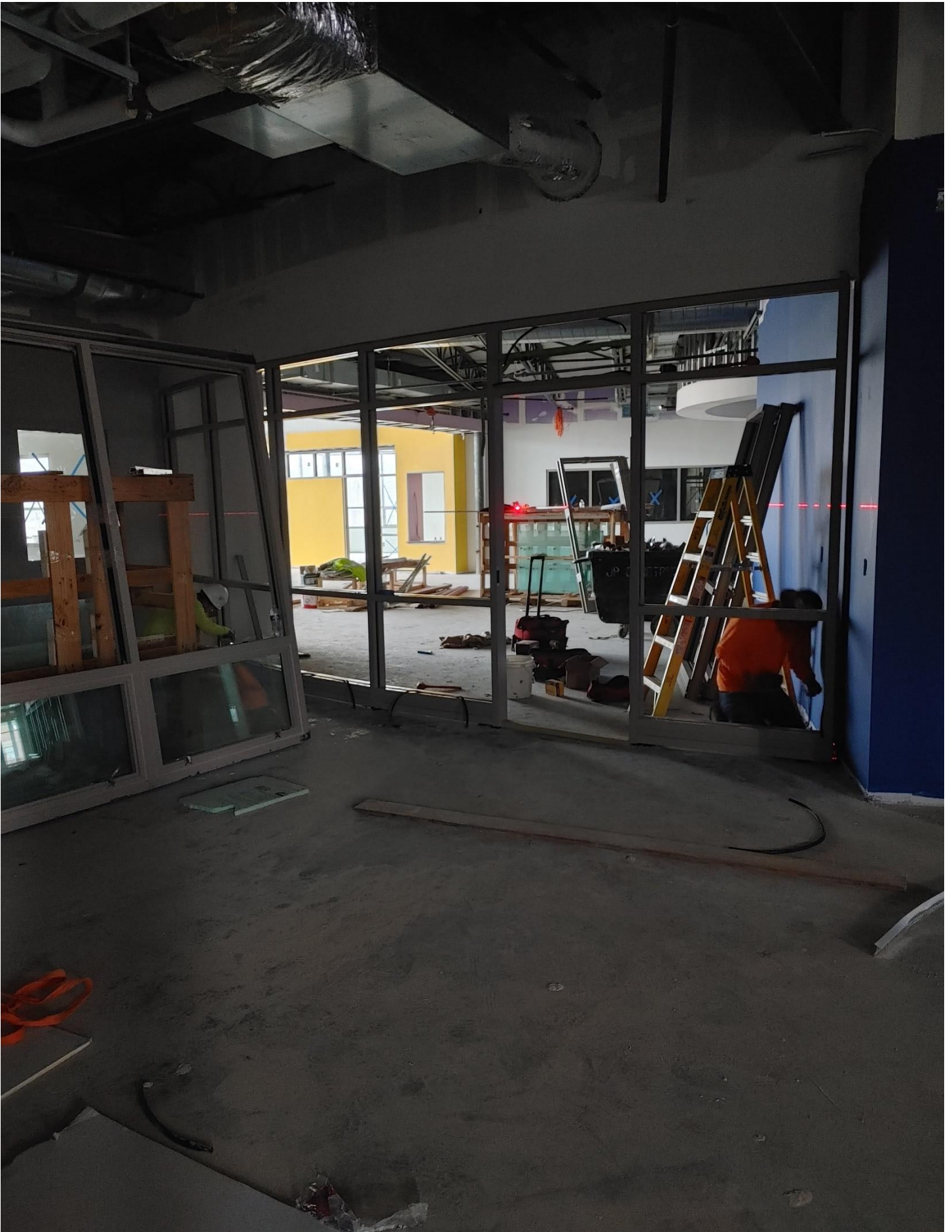
Photo 24 - SF62 is being installed.
