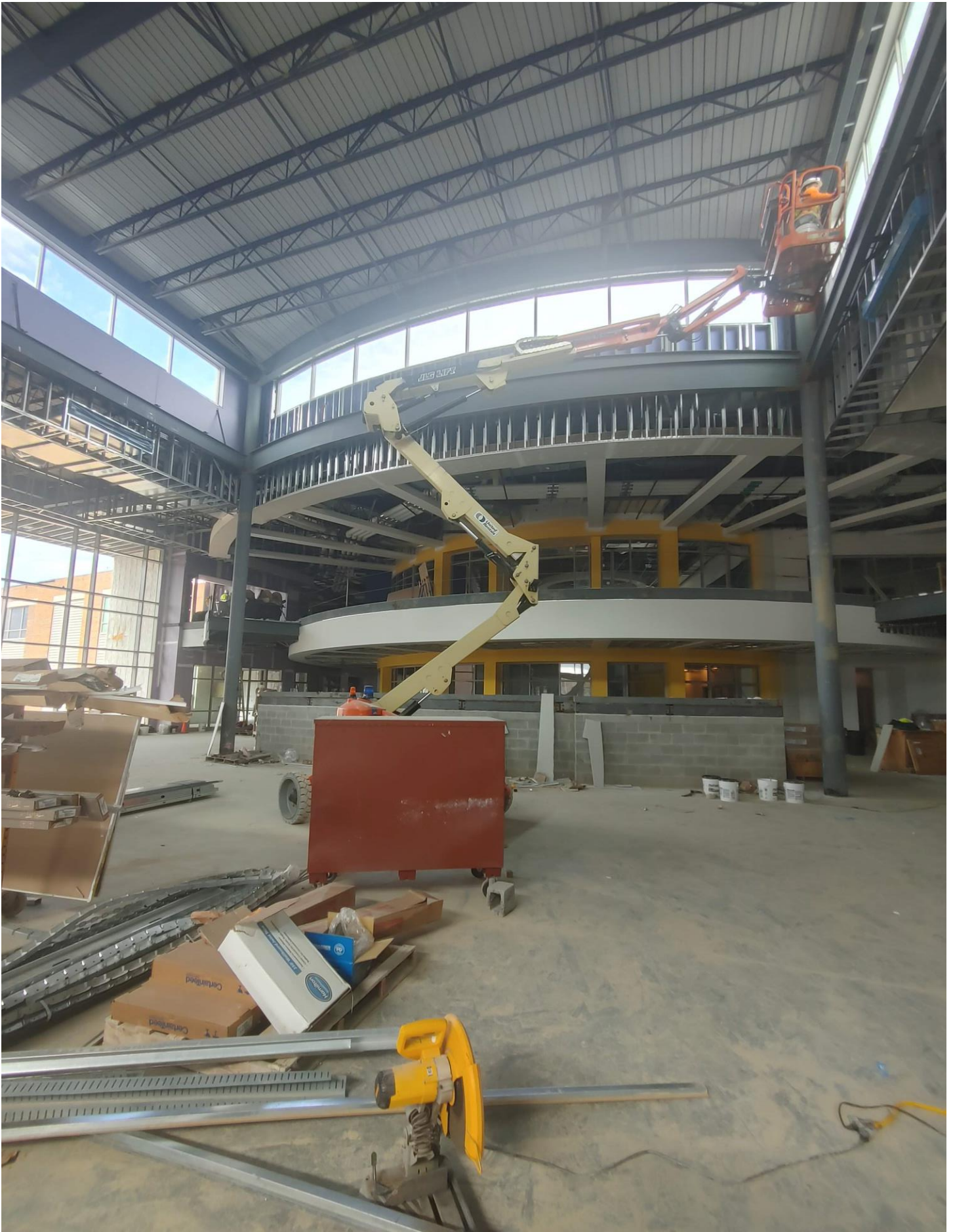
Photo 3 - Sheetrock is being finished in Area C.
