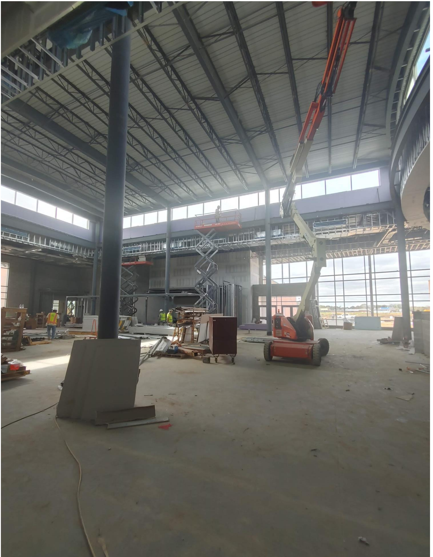
Photo 2 - Sheetrock is being hung in Area C
