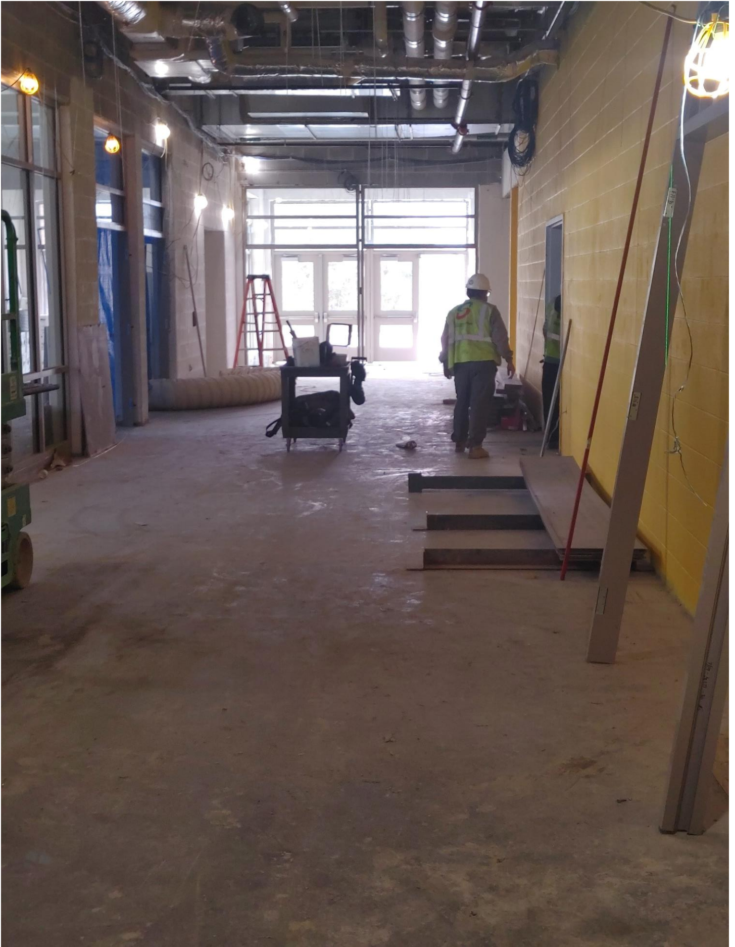
Photo 8 - SF5A has been installed in Area E.
