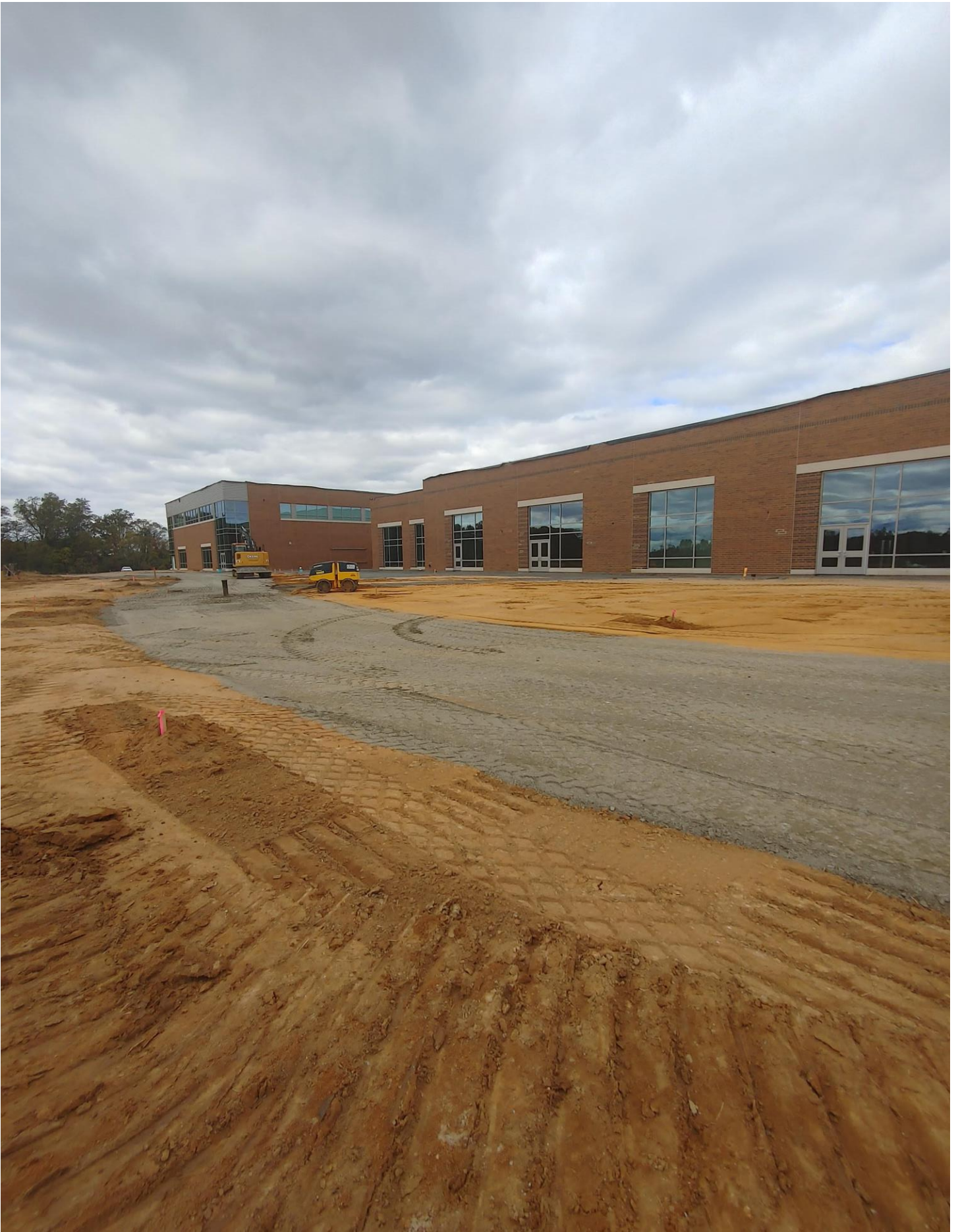
Photo 16 - South side of Areas D & E
