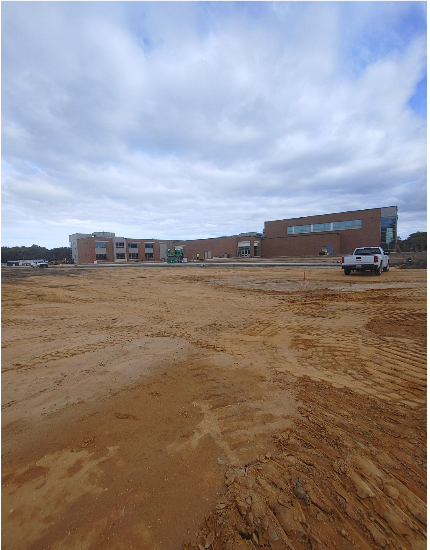
Photo 18 - West side of Building with Bus Loop area.
