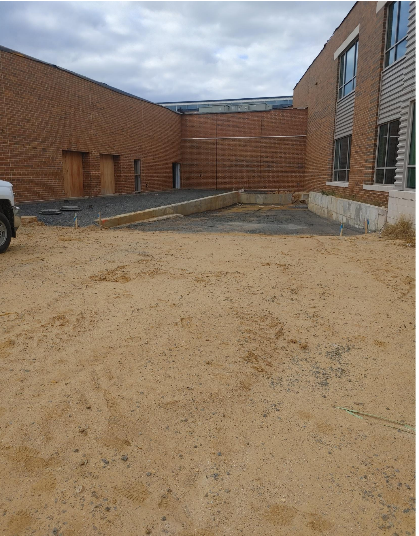
Photo 14 - Stone laid in Loading Dock Area.
