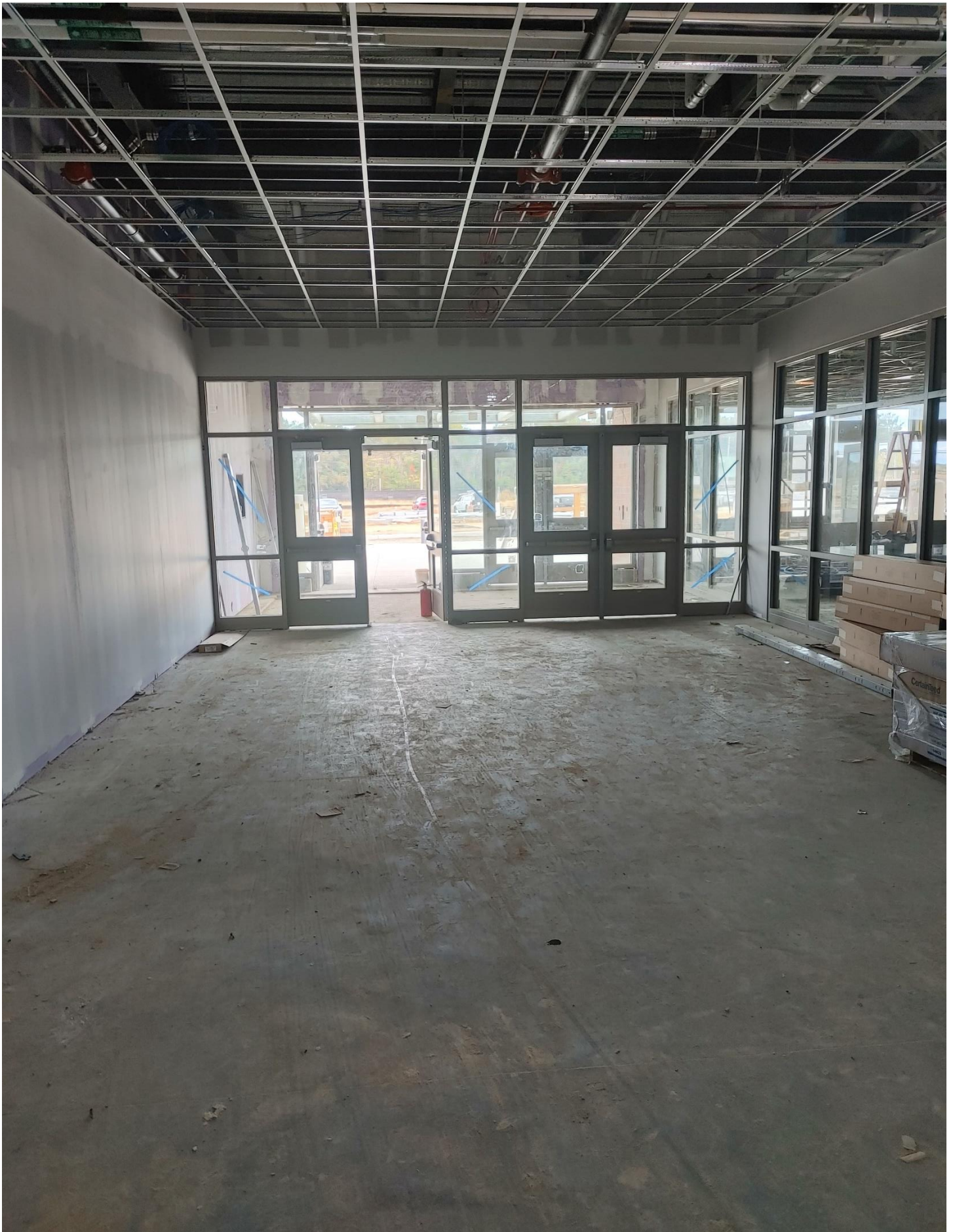
Photo 9 - SF39 has been installed in Area A
