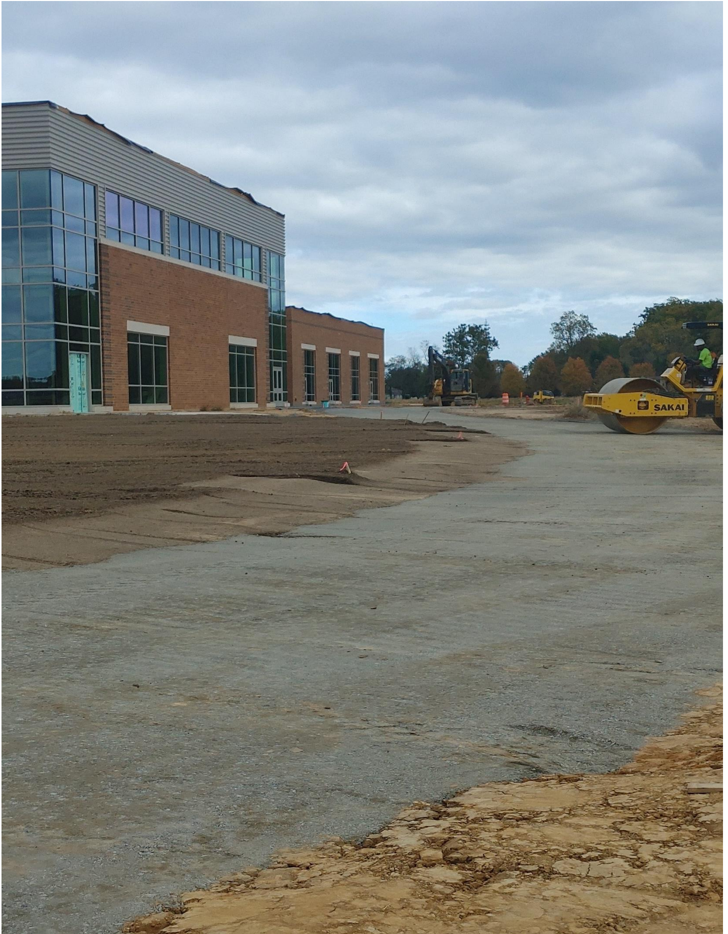
Photo 17 - Access Road on the South side of the Building.
