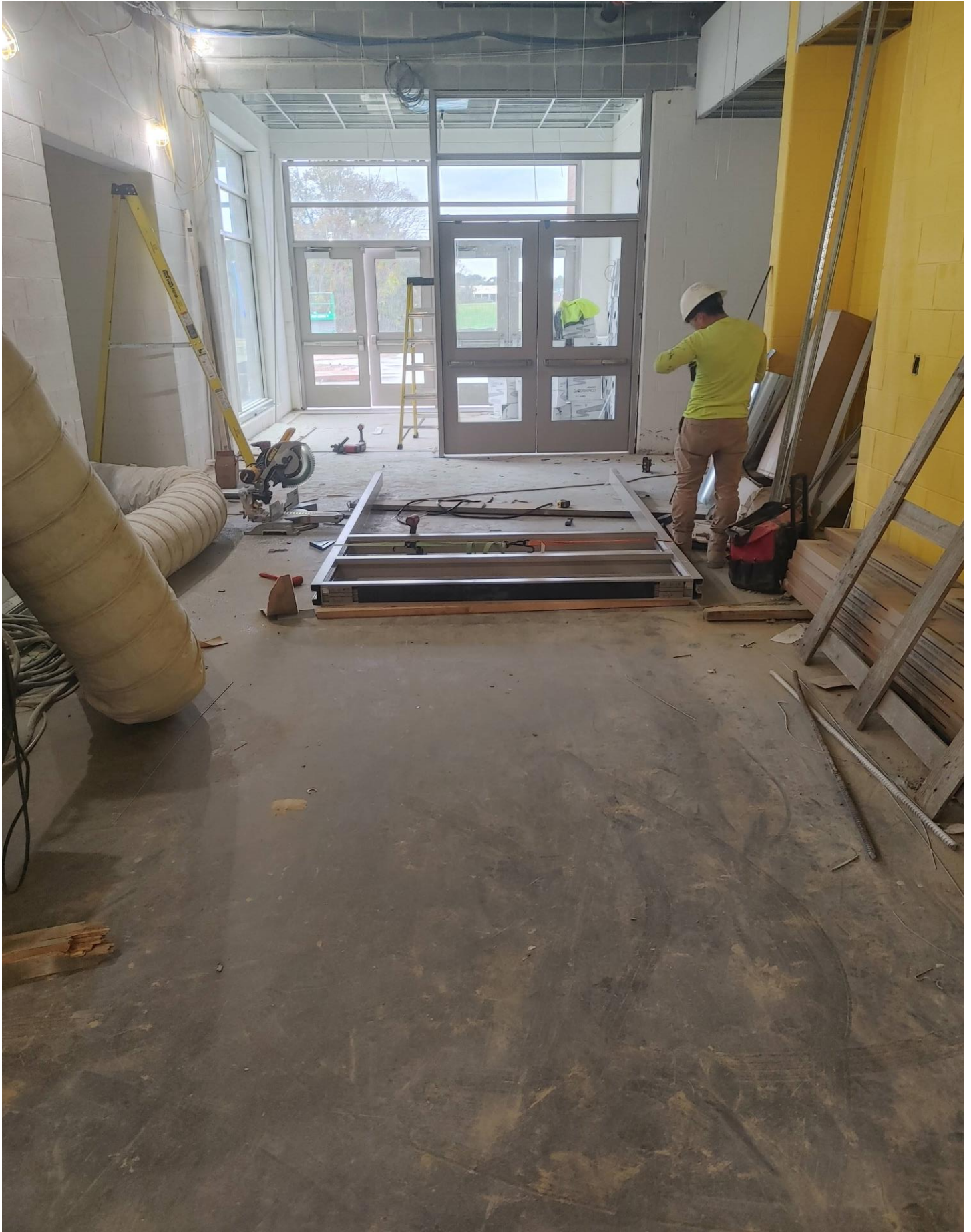
Photo 10 - FG&M continue to work on SF5A in Area E.
