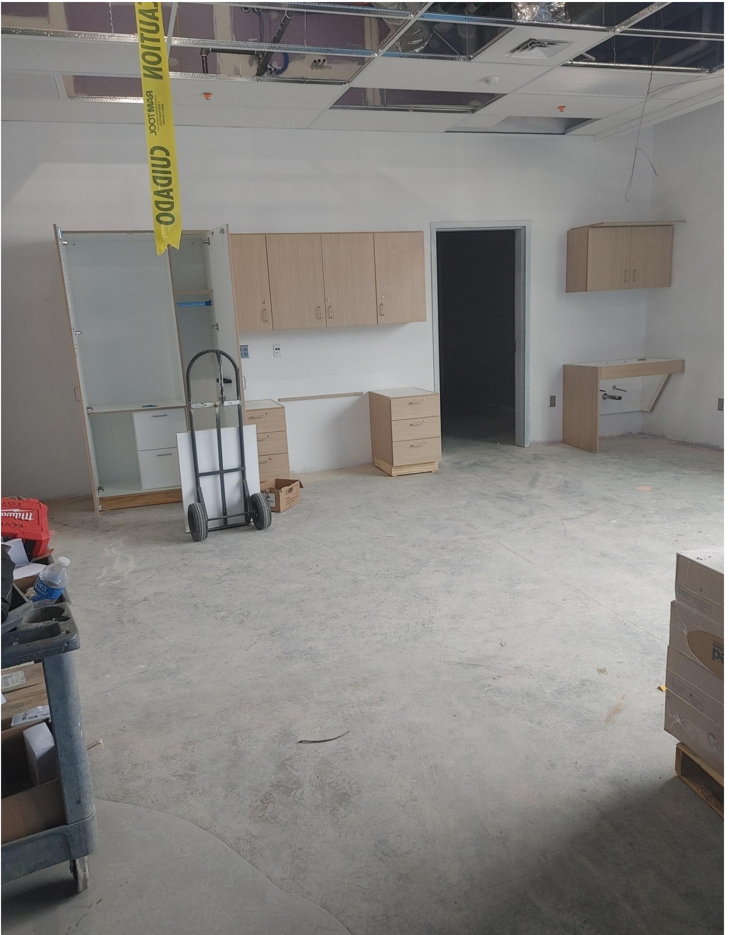
Photo 11 - Cabinetry has been installed throughout Area B
