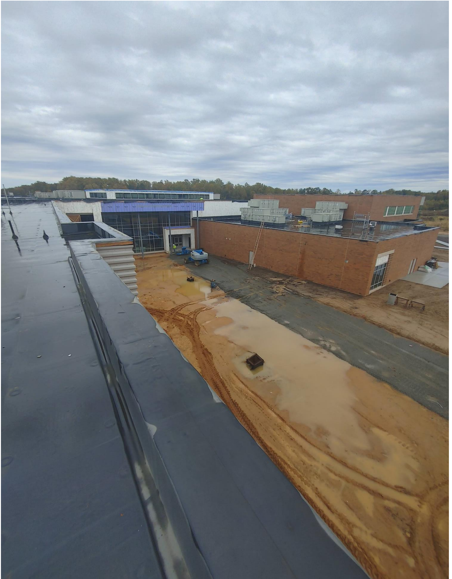
Photo 14 - Stone has been laid between Area B & E.
