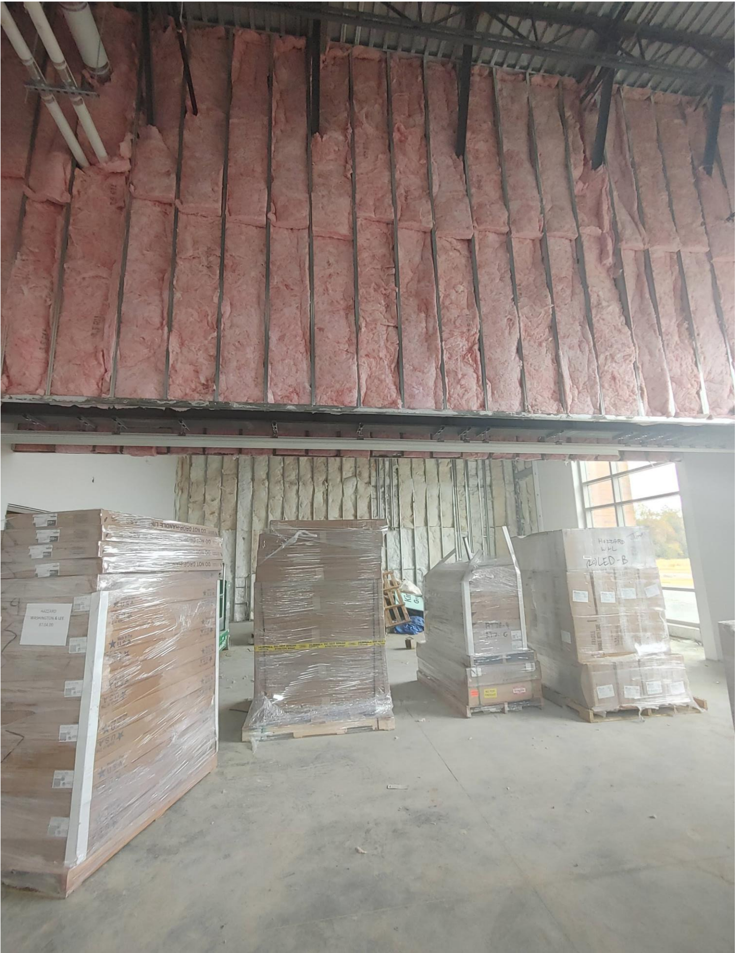
Photo 8 - Insulation has been installed in Area D
