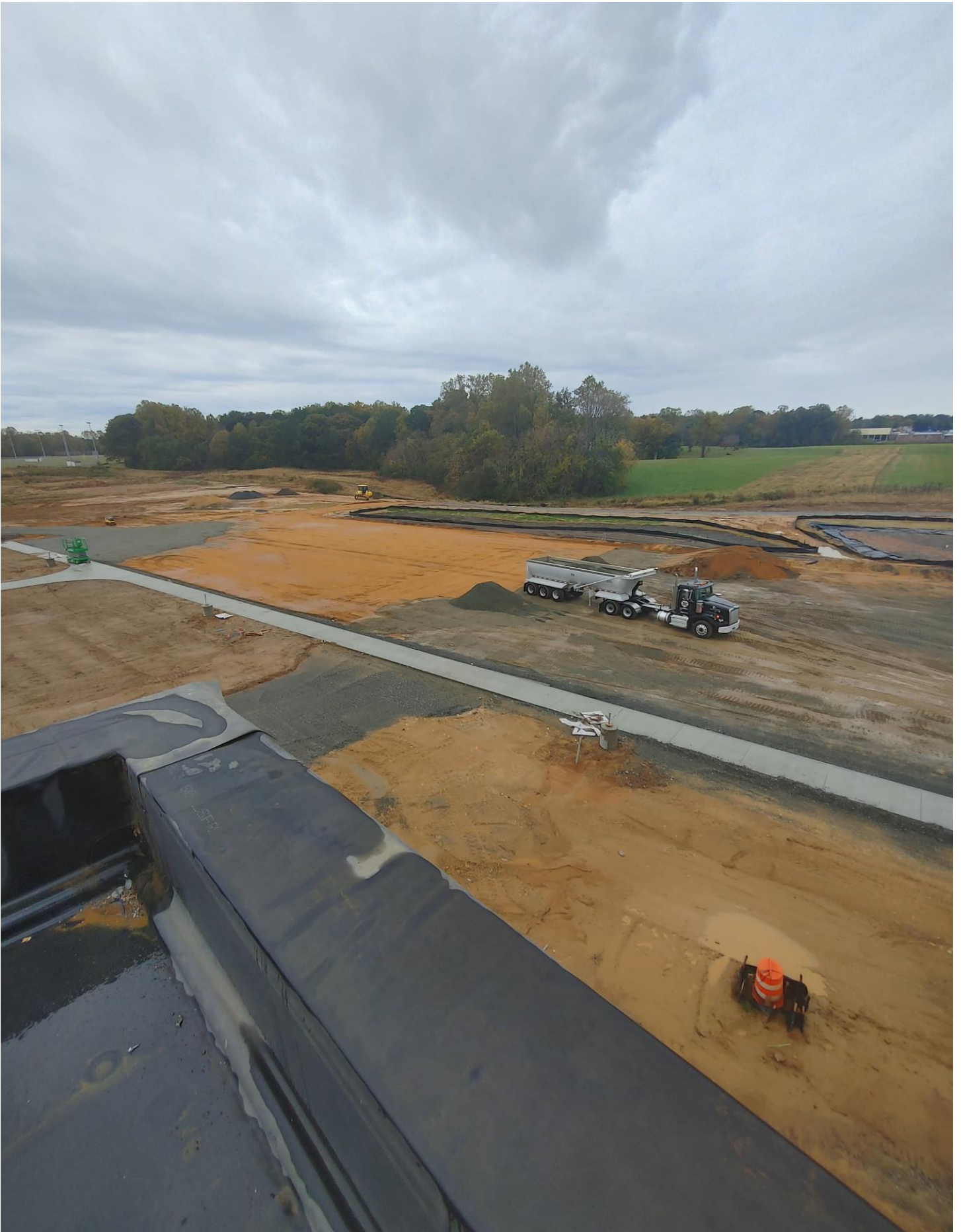
Photo 12 - Stone is being delivered on the West side of the site.
