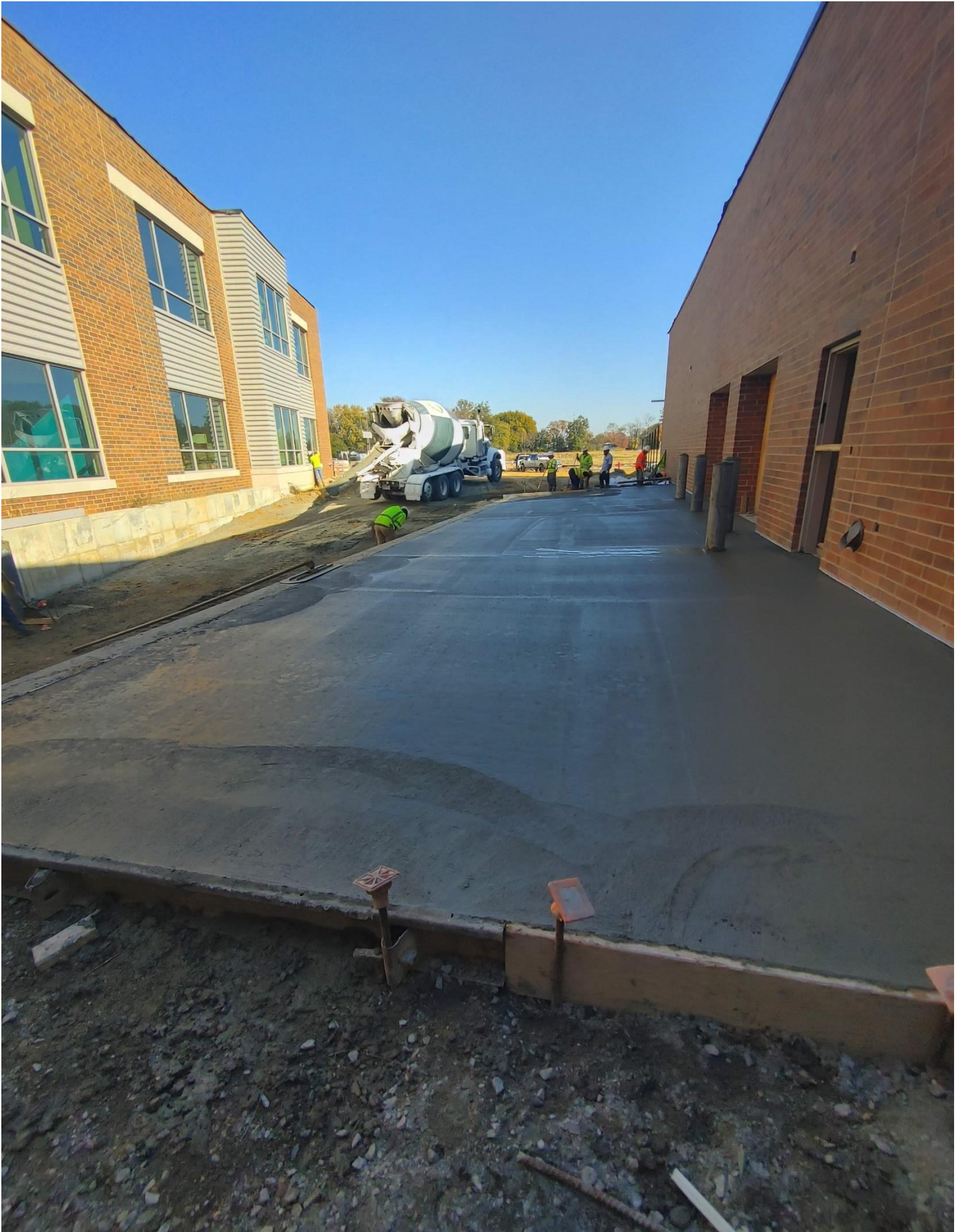
Photo 12 - Concrete is being poured in the Loading Dock Area
