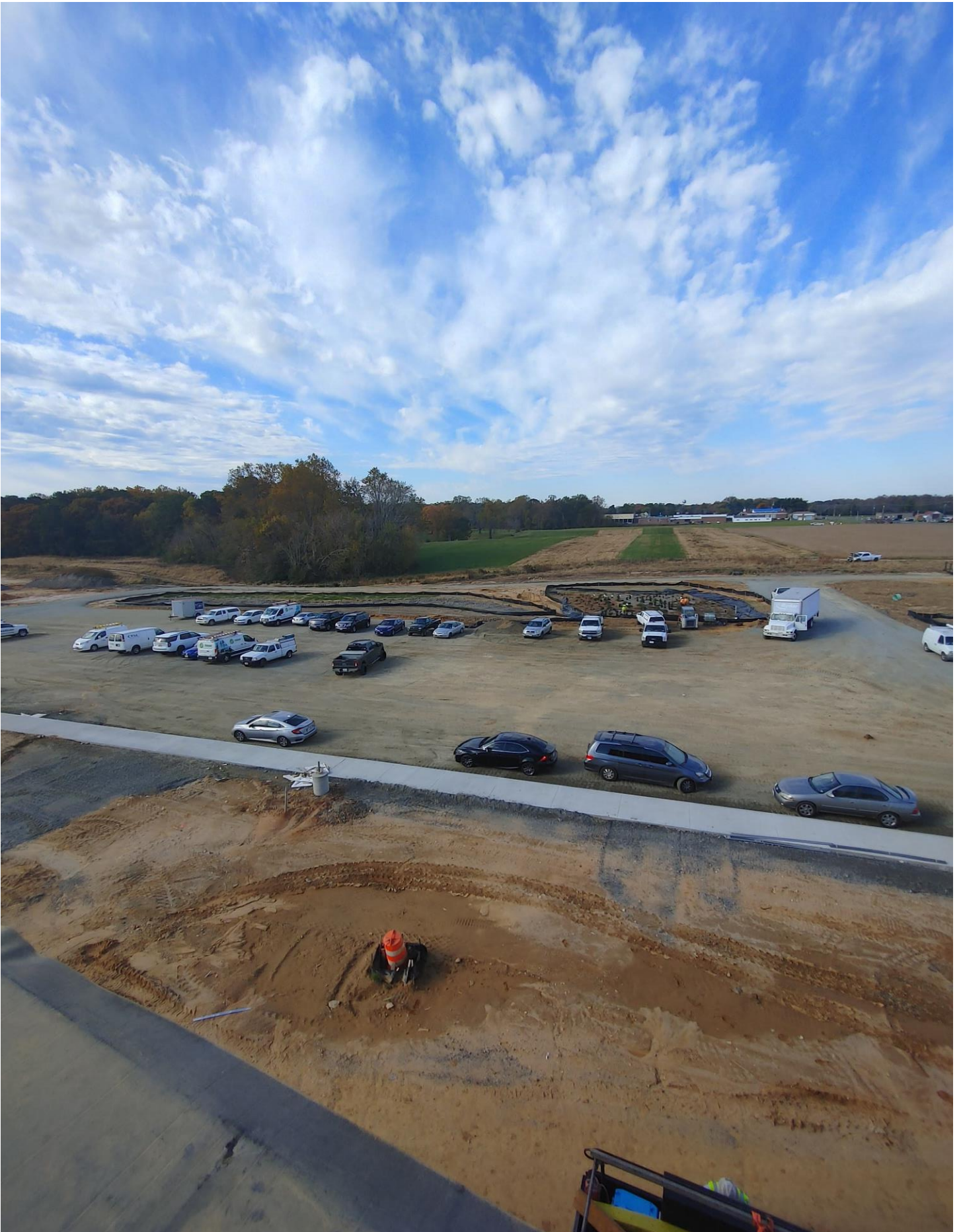
Photo 10 - Bus Loop area
