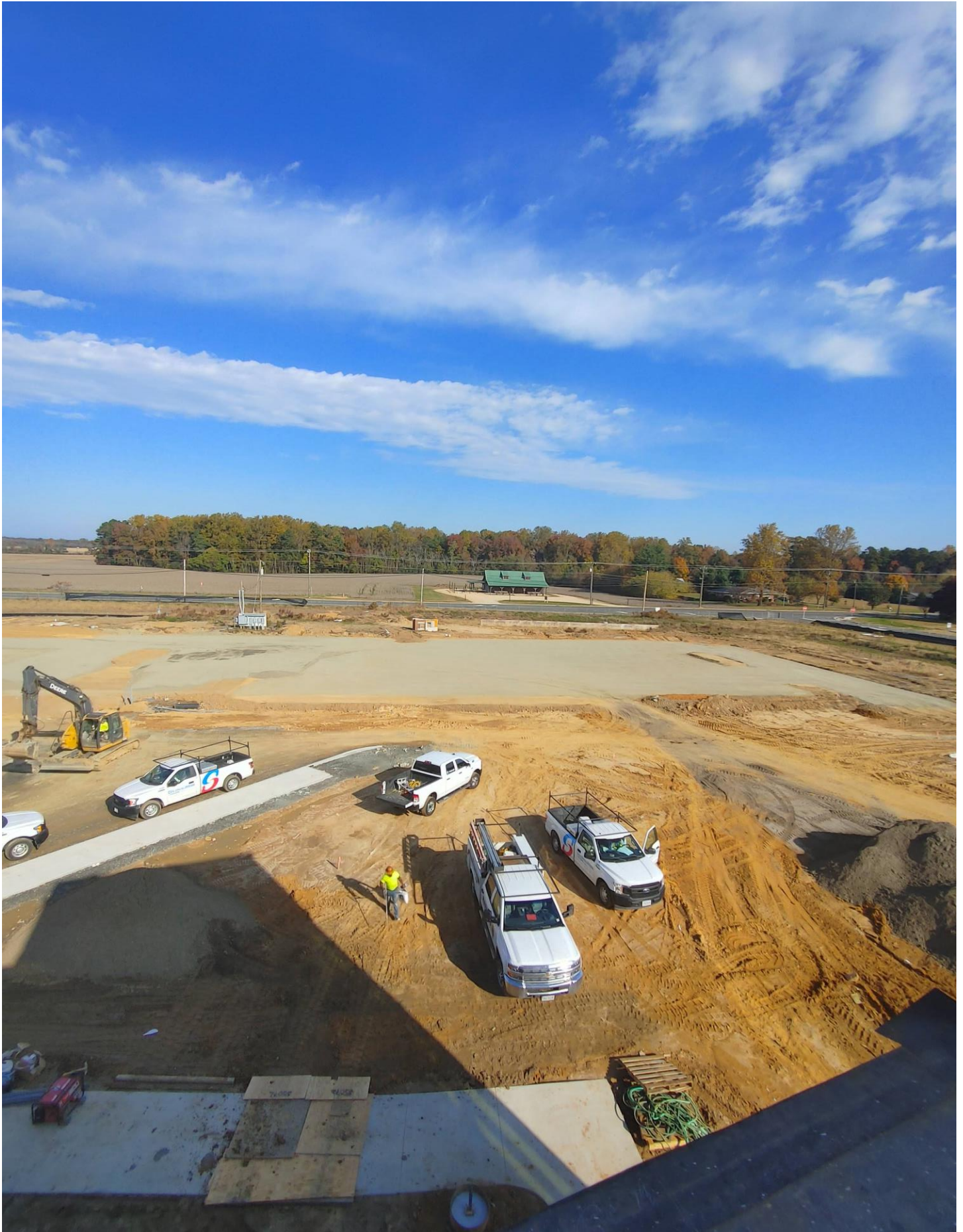
Photo 7 - Progress is being made on the Student Parking lot.
