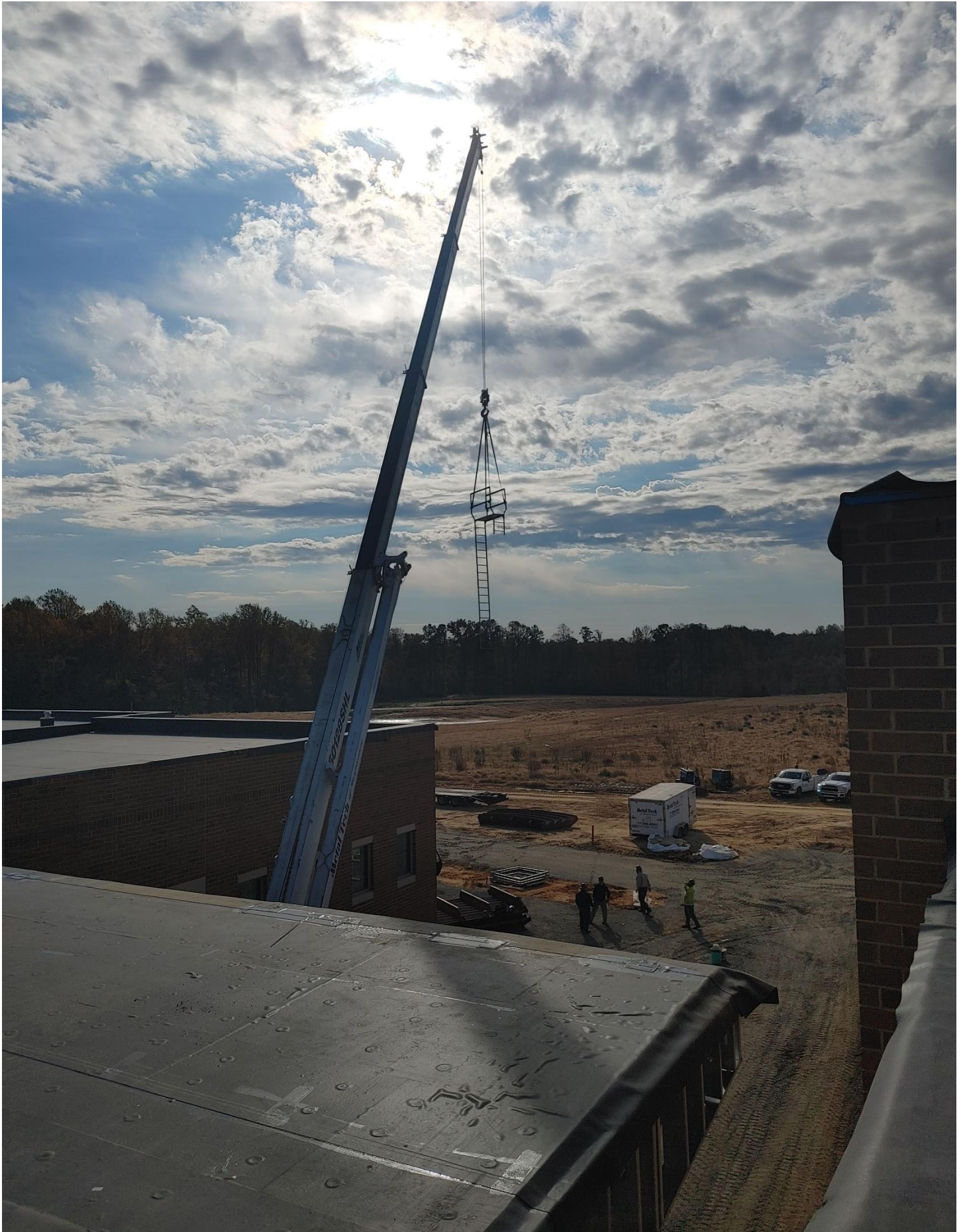
Photo 9 - Ship Ladders are being set on the roof.
