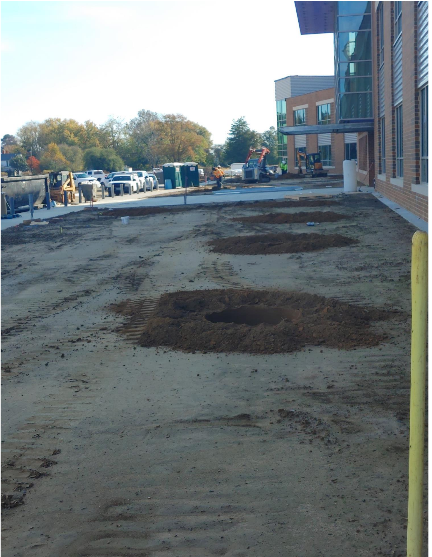
Photo 3 - Holes dug for trees.
