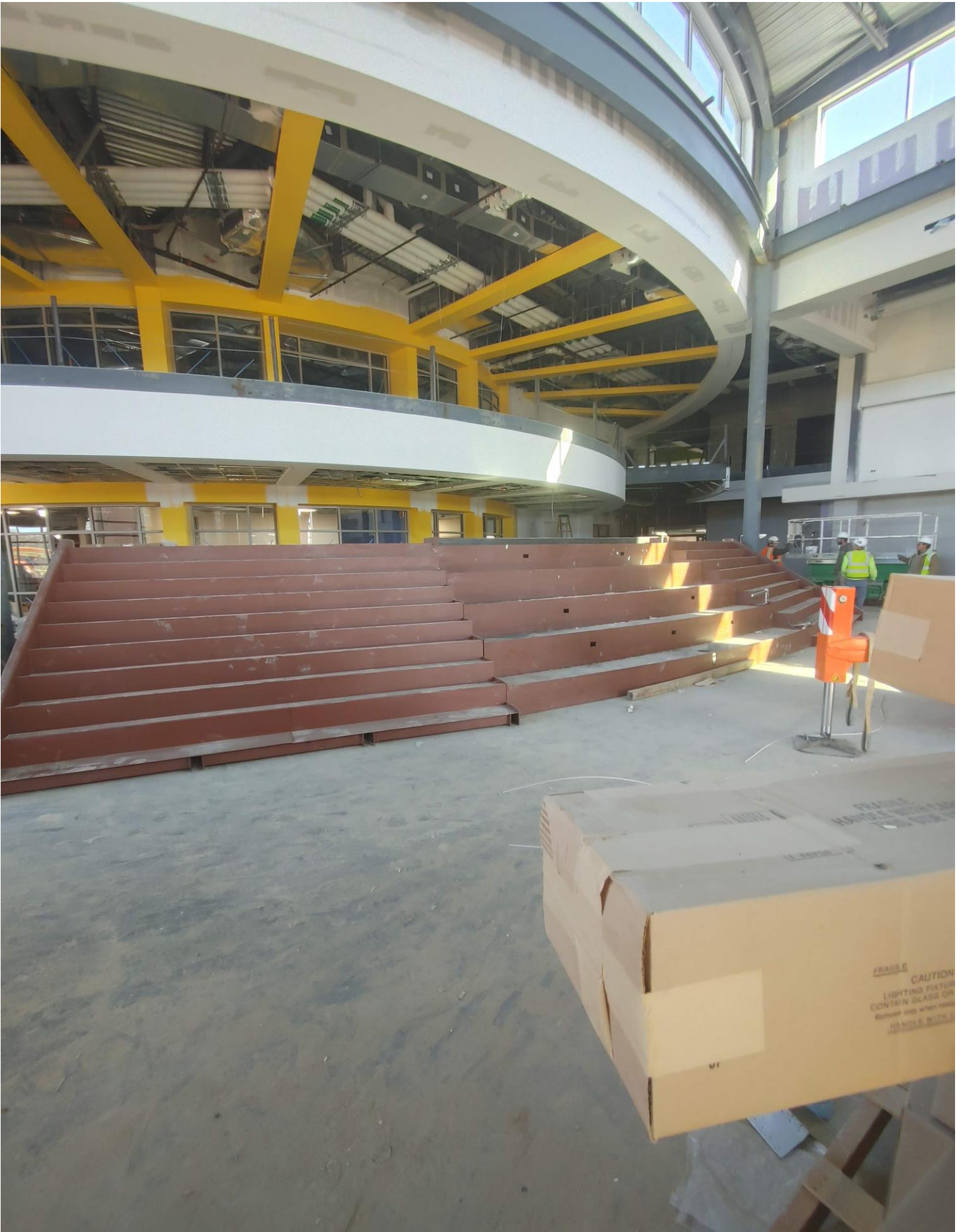
Photo 12 - The erection of the Grand Staircase has begun.
