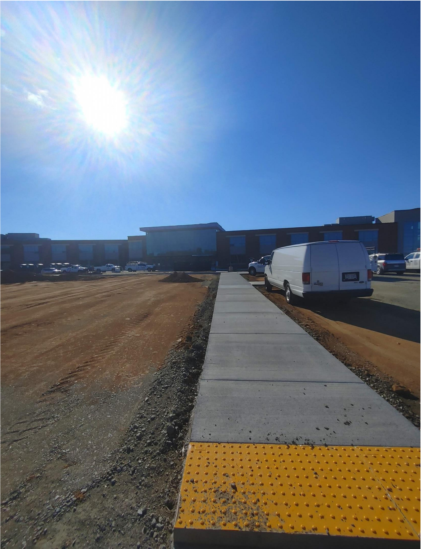
Photo 1 Sidewalks in the Student Parking Lot area have been poured
