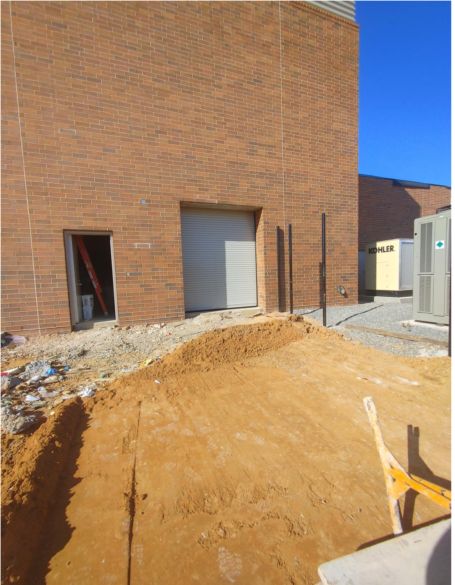
Photo 10 - XD08 Overhead roll-up door has been installed
