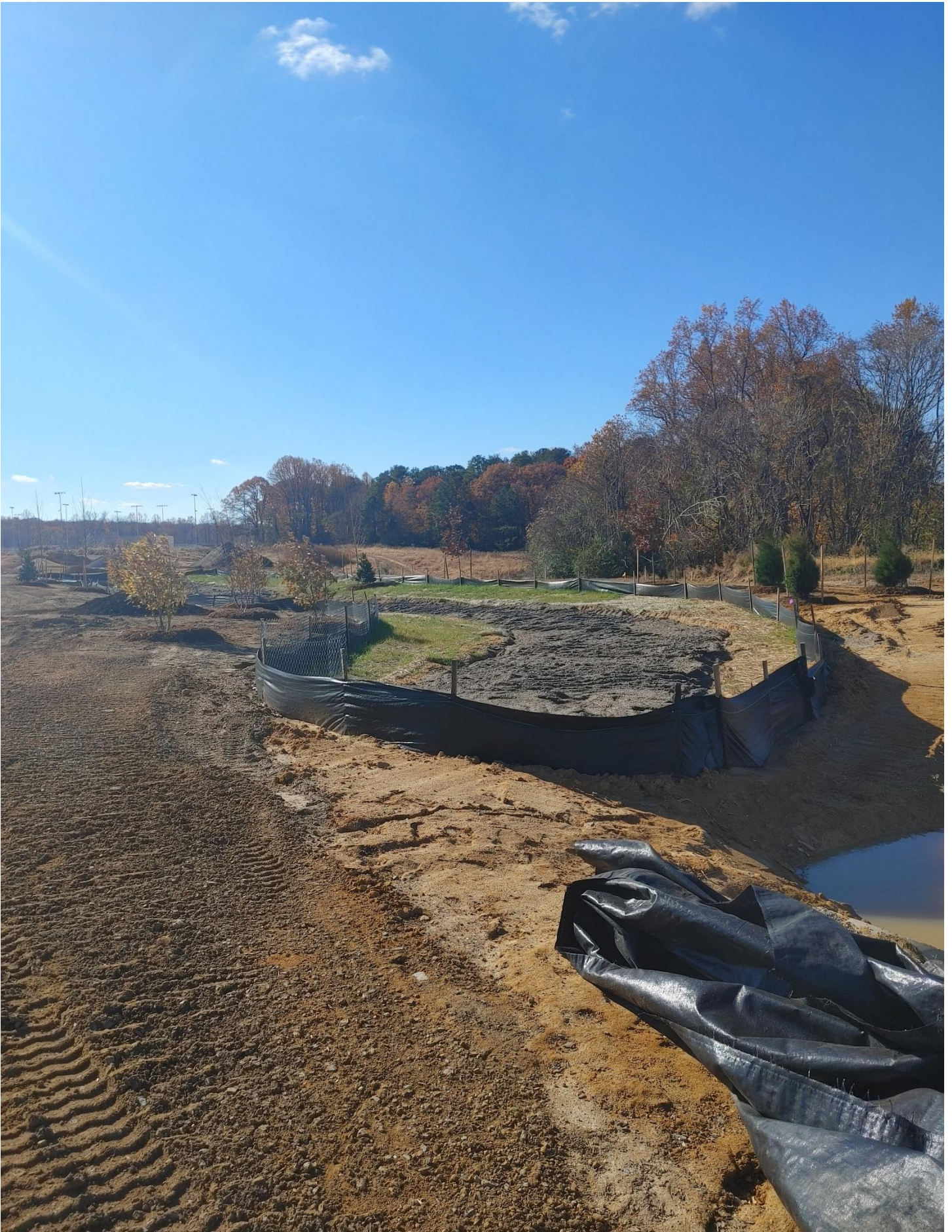
Photo 6 - Trees have been planted around Bio Pond on West side of the site.
