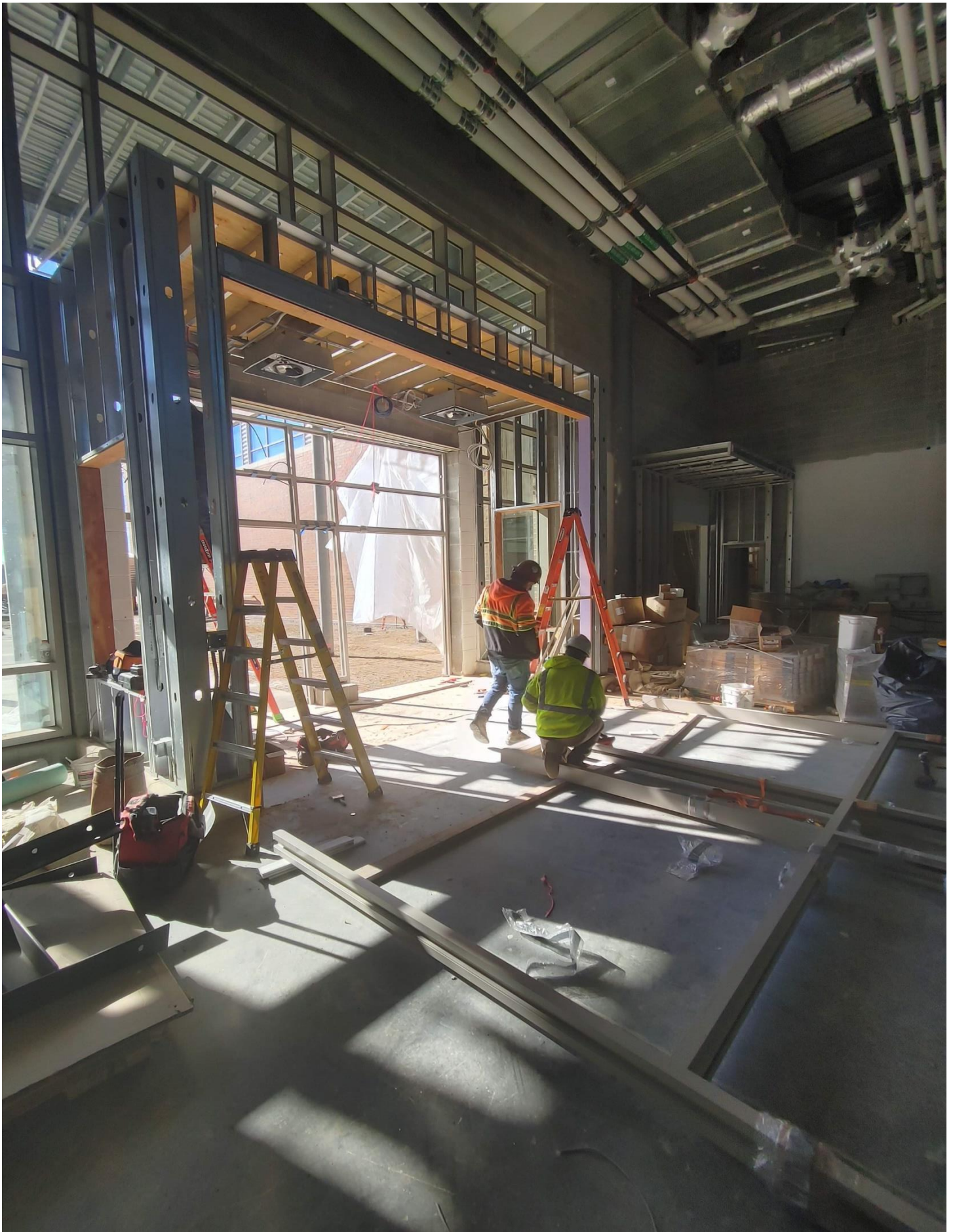
Photo 15 – Preparing to set SF49B in Area C.
