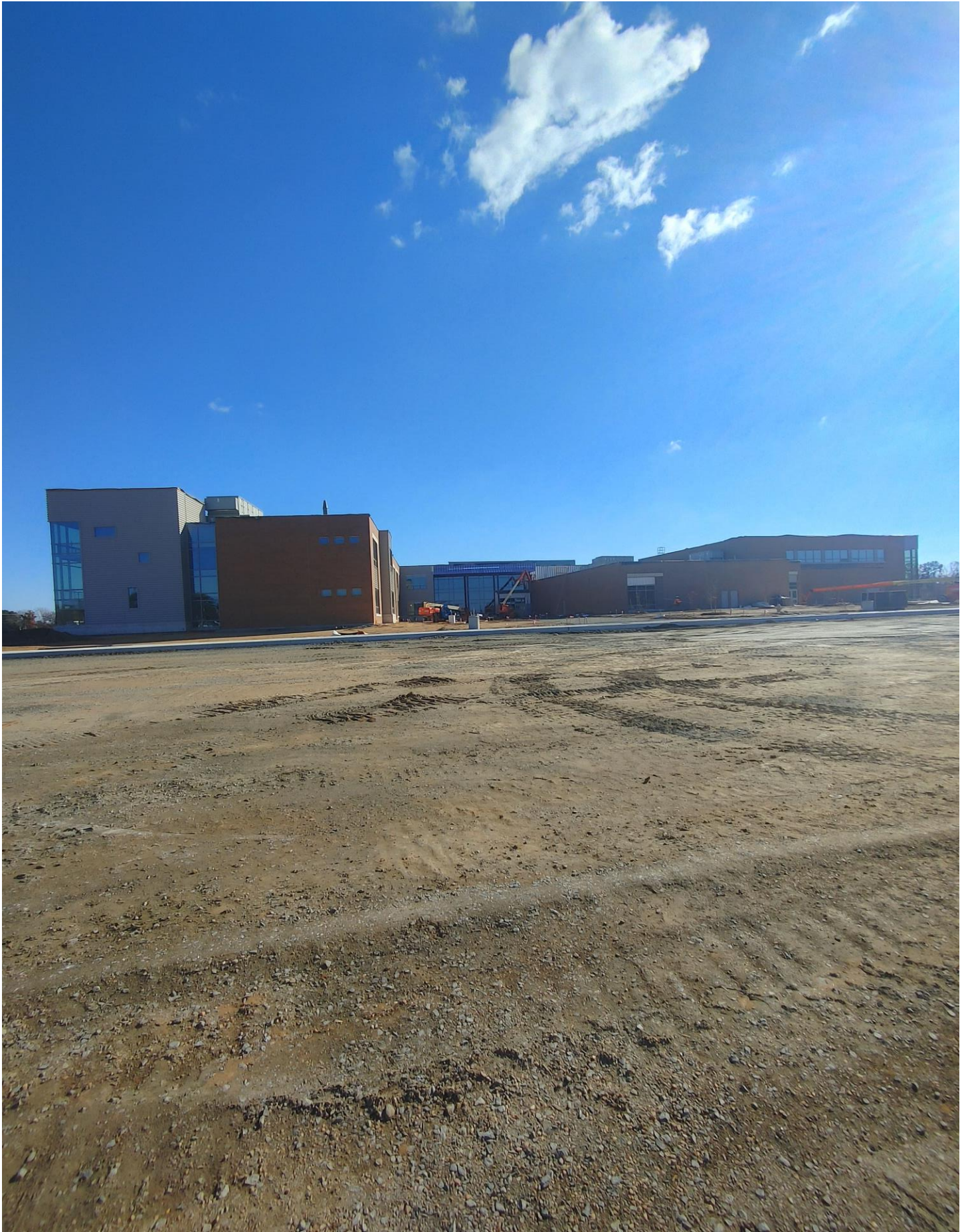
Photo 7 - West side of site
