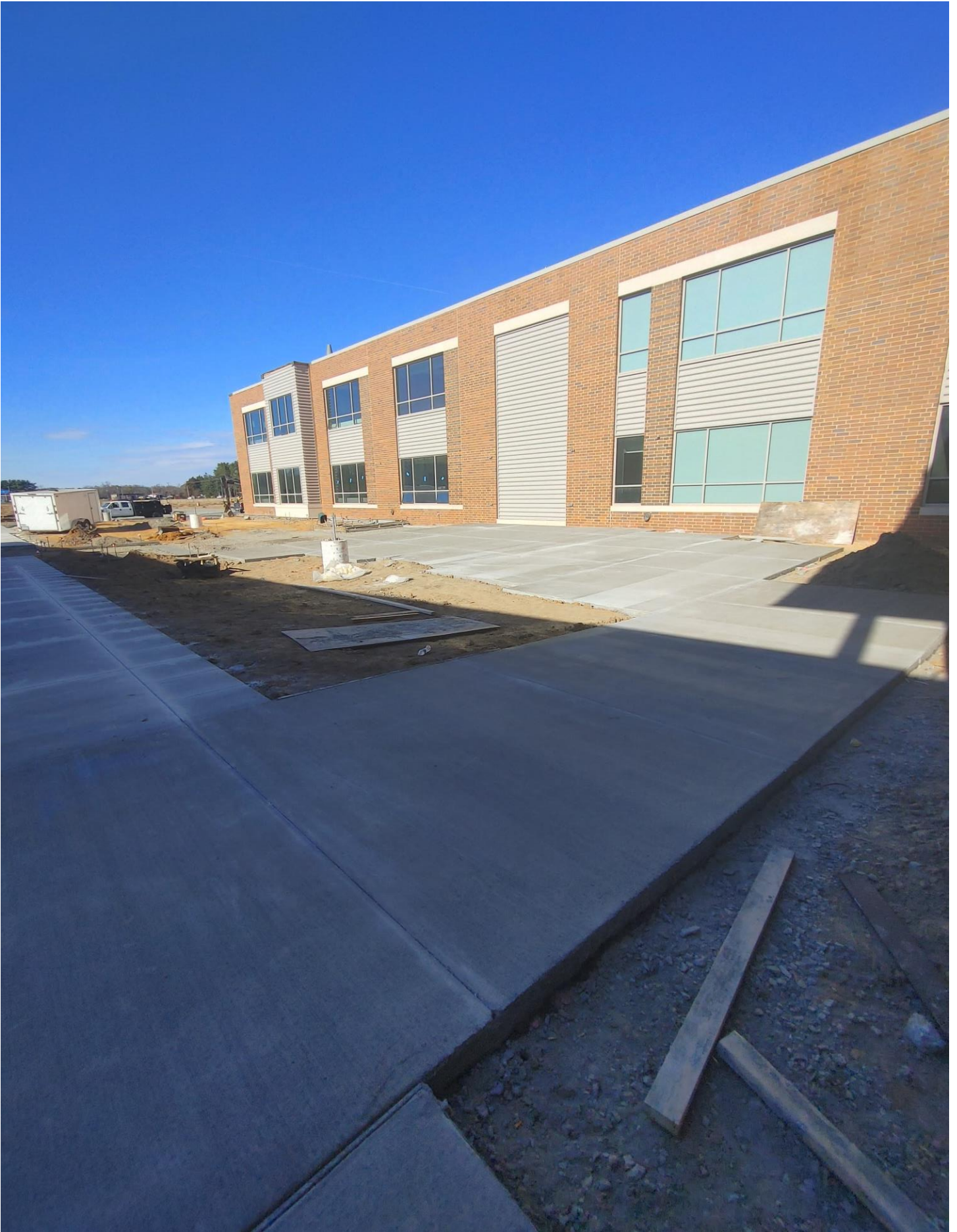
Photo 18 - Concrete between Areas B & E.
