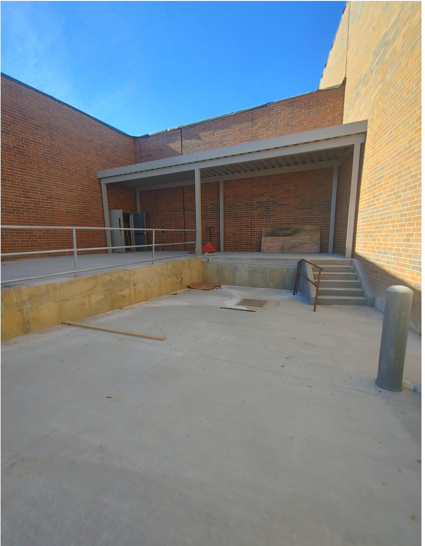
Photo 17 - Railing is being set in the Loading Dock Area.
