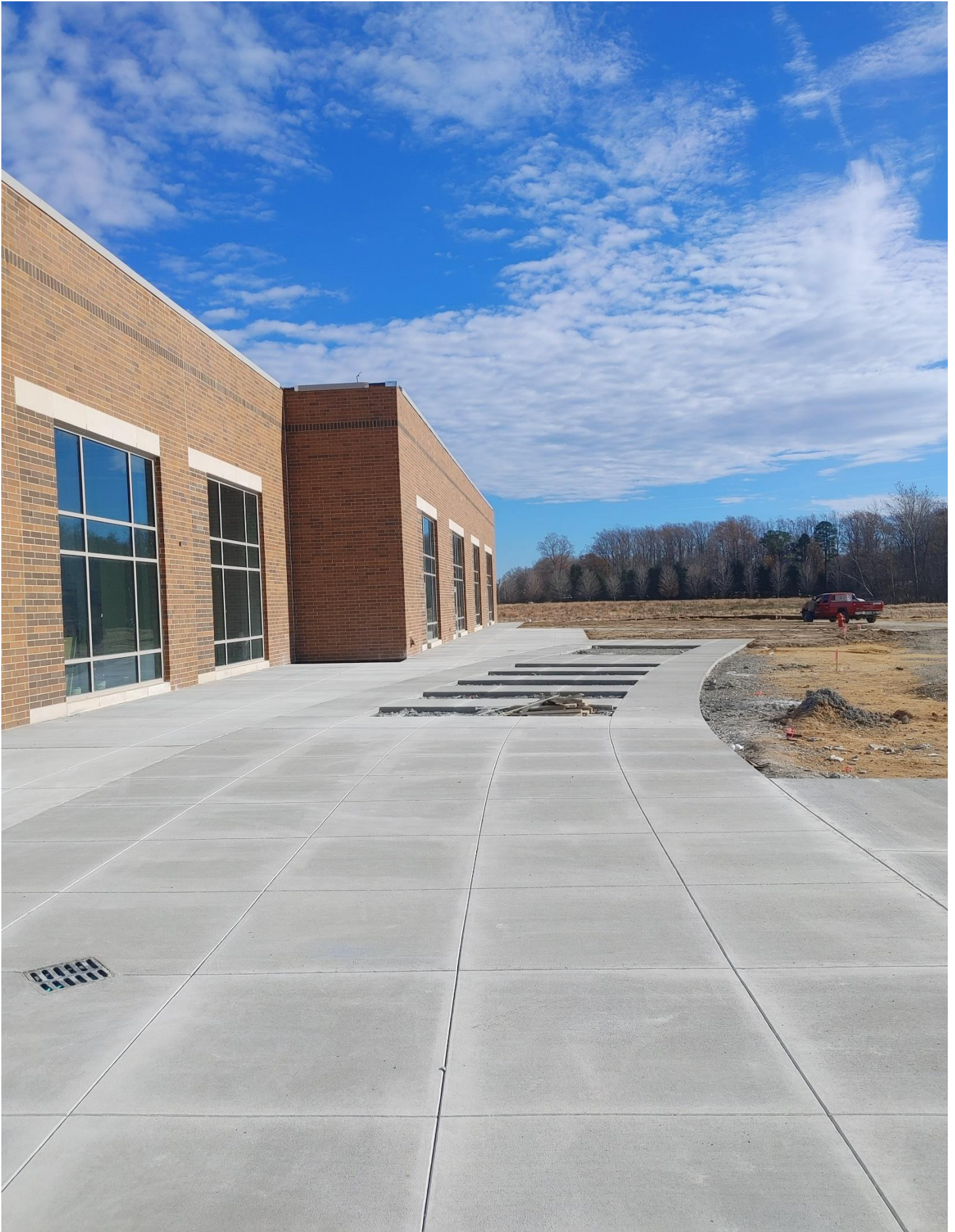
Photo 4 - South Side of Area E
