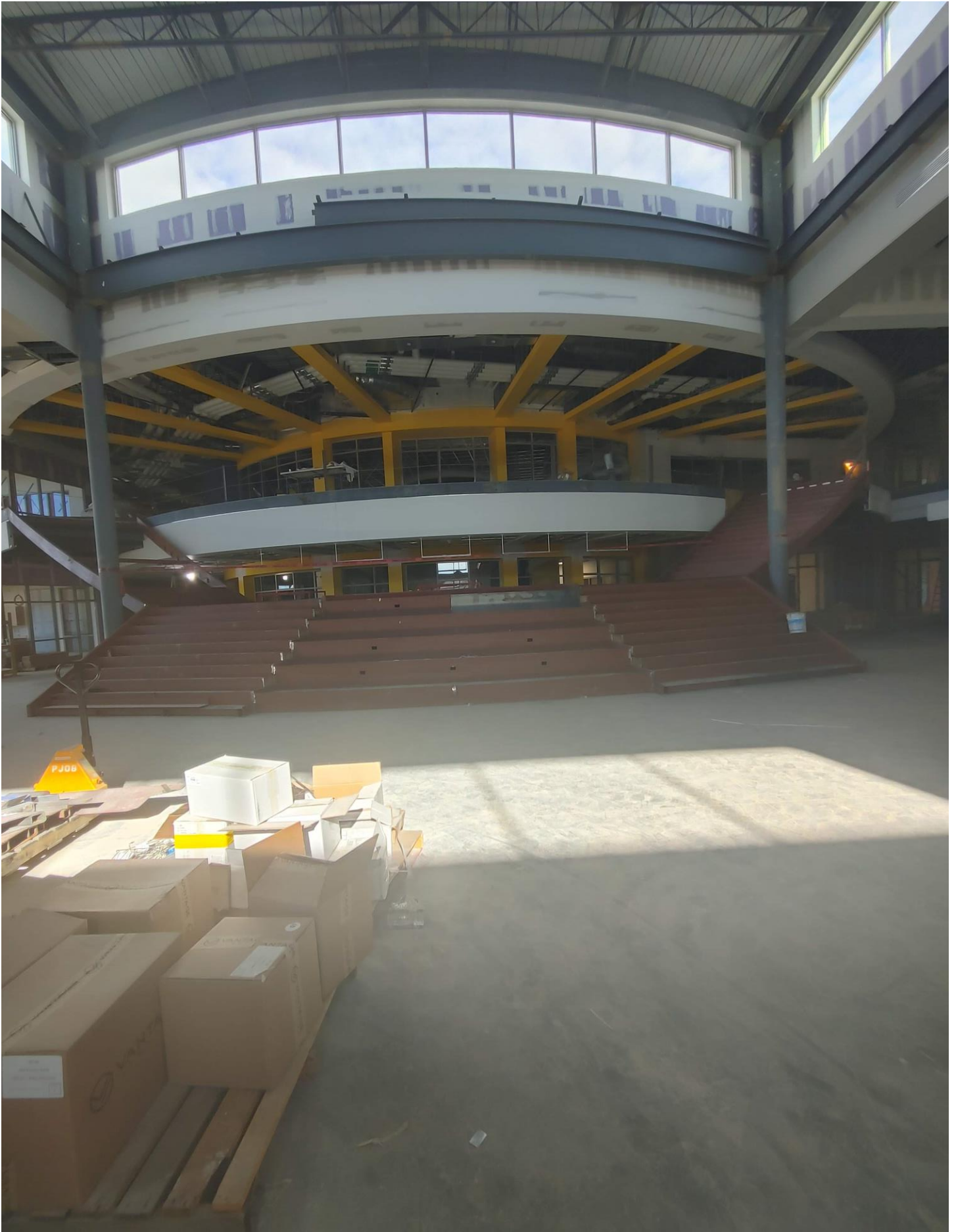
Photo 5 - Grand Staircase is being constructed.
