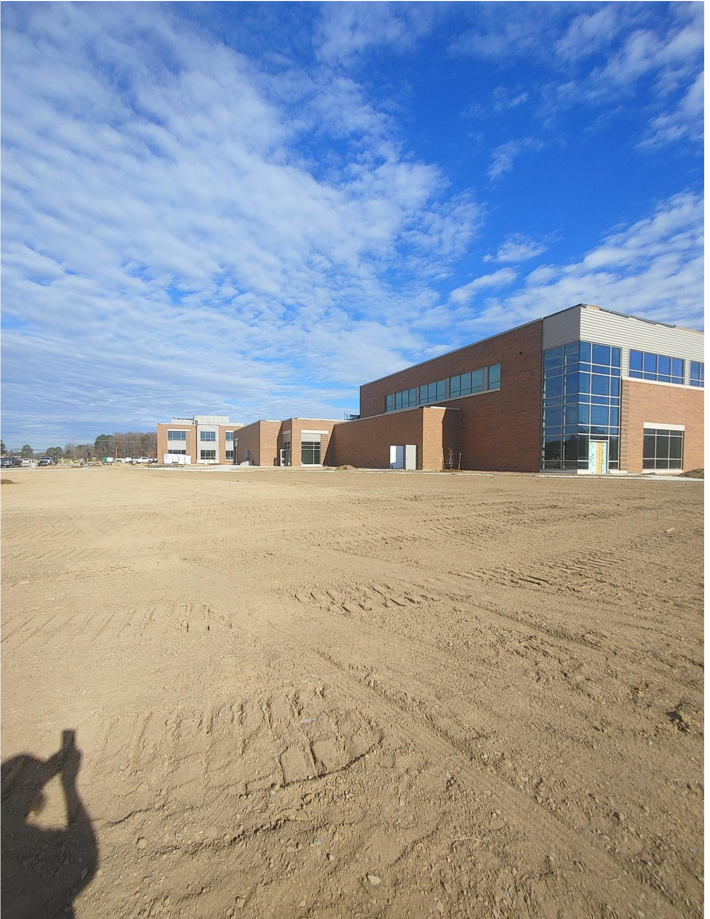
Photo 2 - South West Corner
