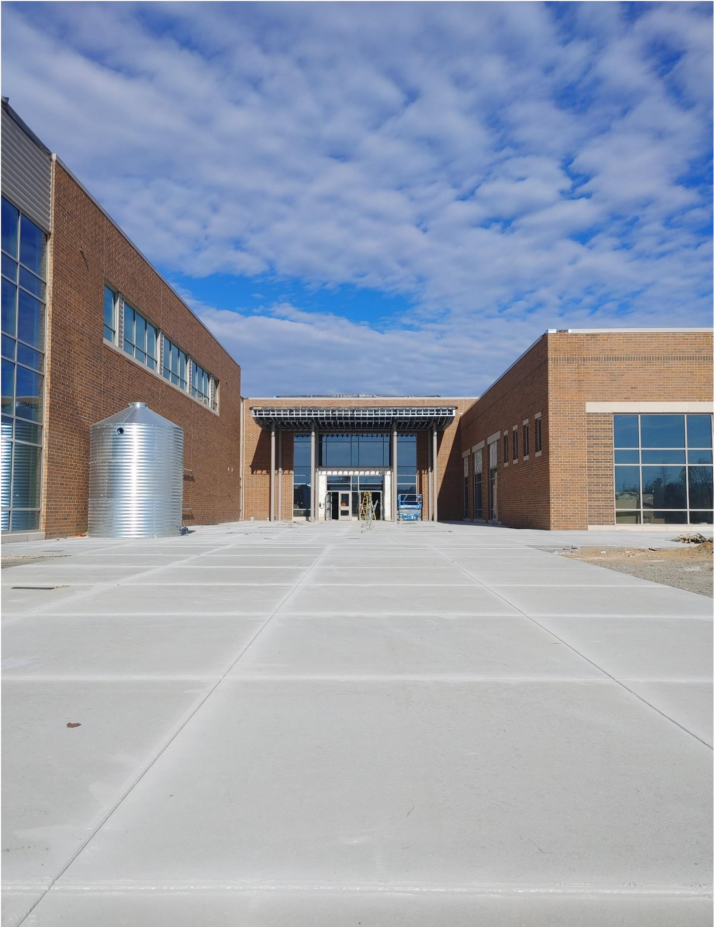
Photo 3 - Concrete has been completed and Cistern has been set
