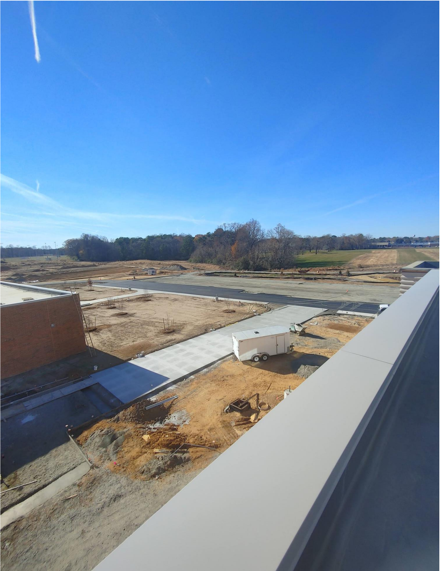
Photo 11 - Bus Loop Area
