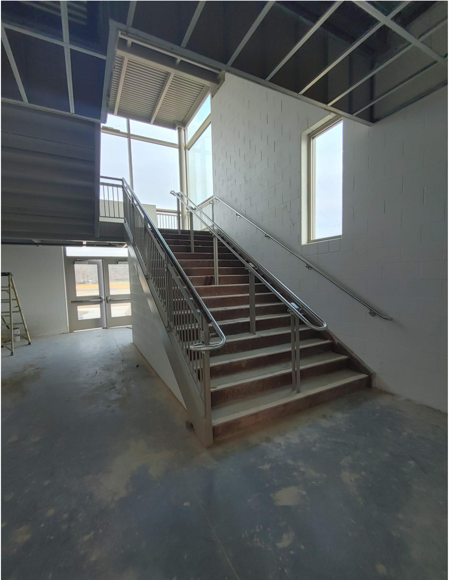
Photo 8 - Railing have been installed in Stairwell #1
