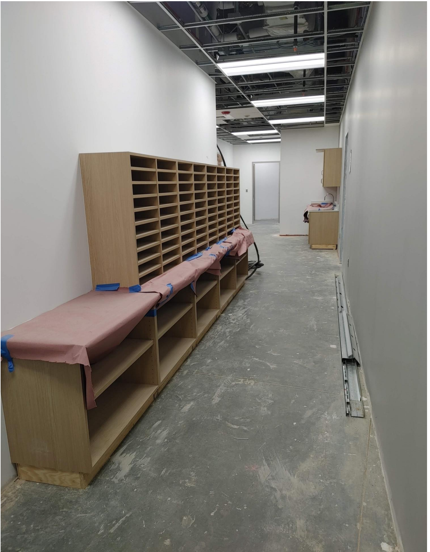
Photo 3 - Cabinetry has been installed in the Administrative Area.
