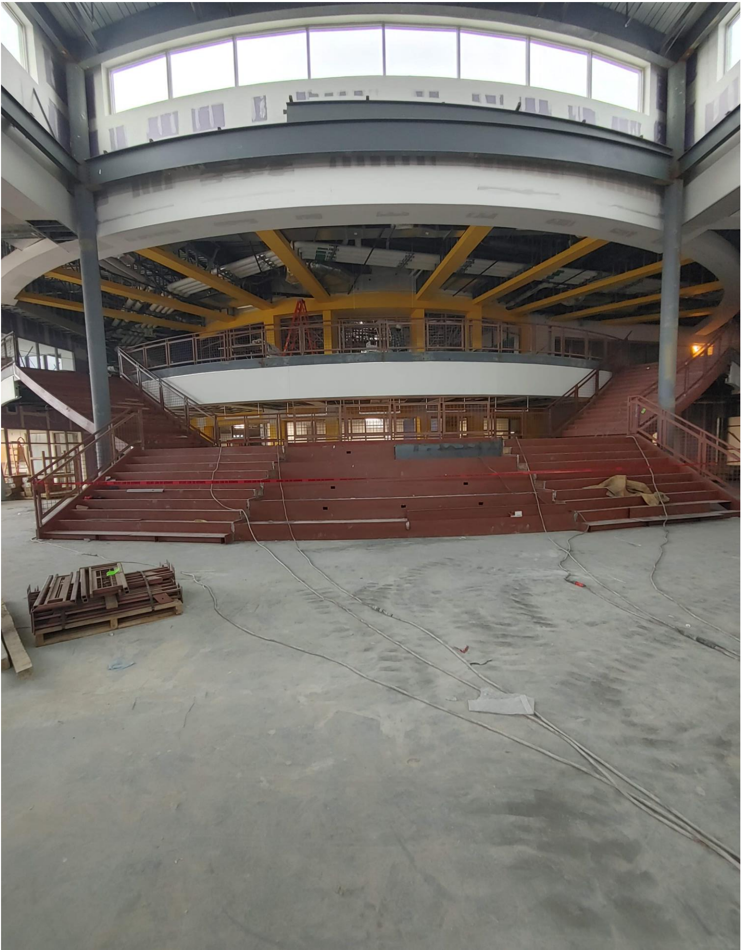
Photo 4 - Progress continues on the Grand Staircase
