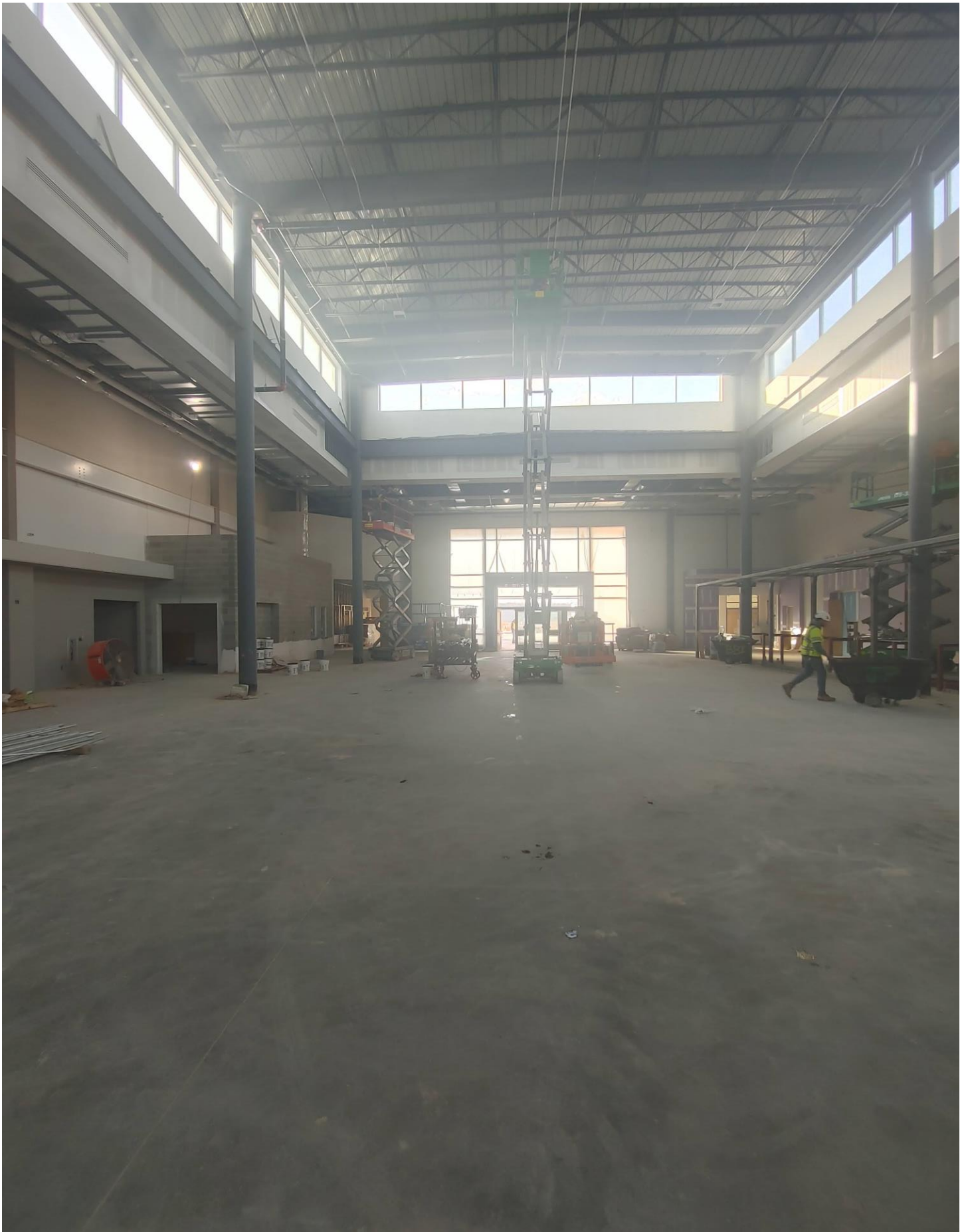
Photo 3 - Sheetrock is being finished in Area C
