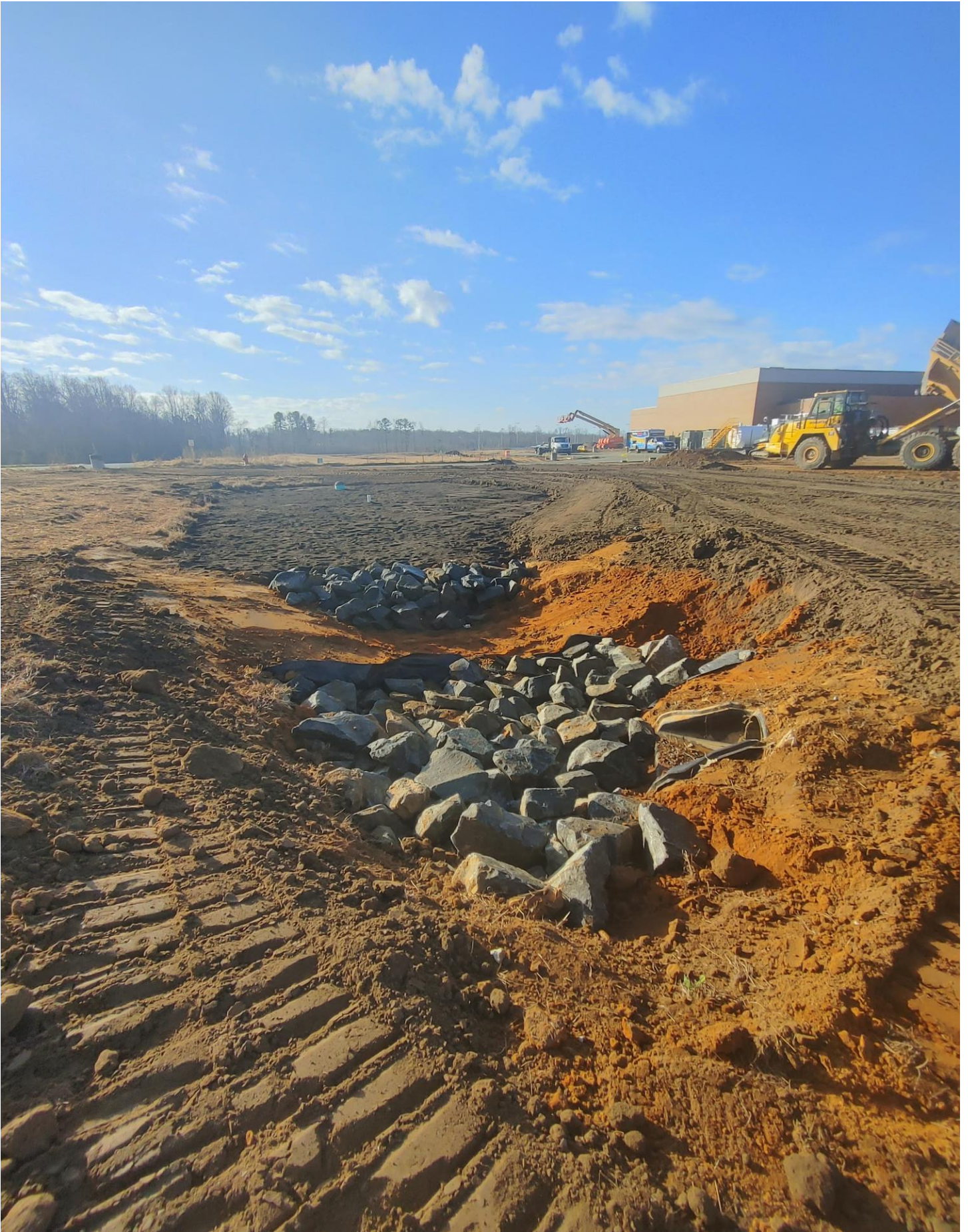
Photo 2 - Bio Retention Pond on the Northeast side of High School
