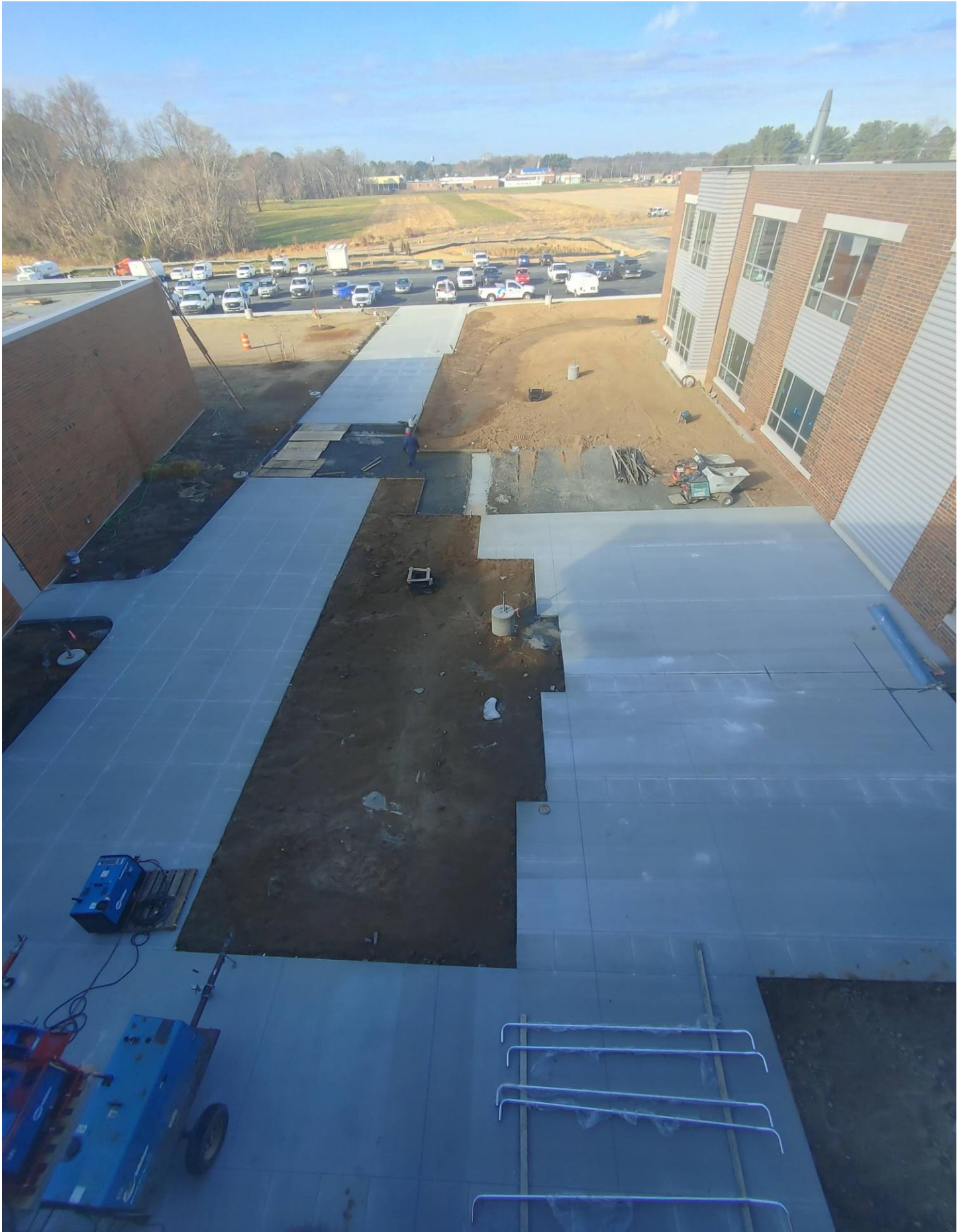
Photo 11 - Student Entrance Area
