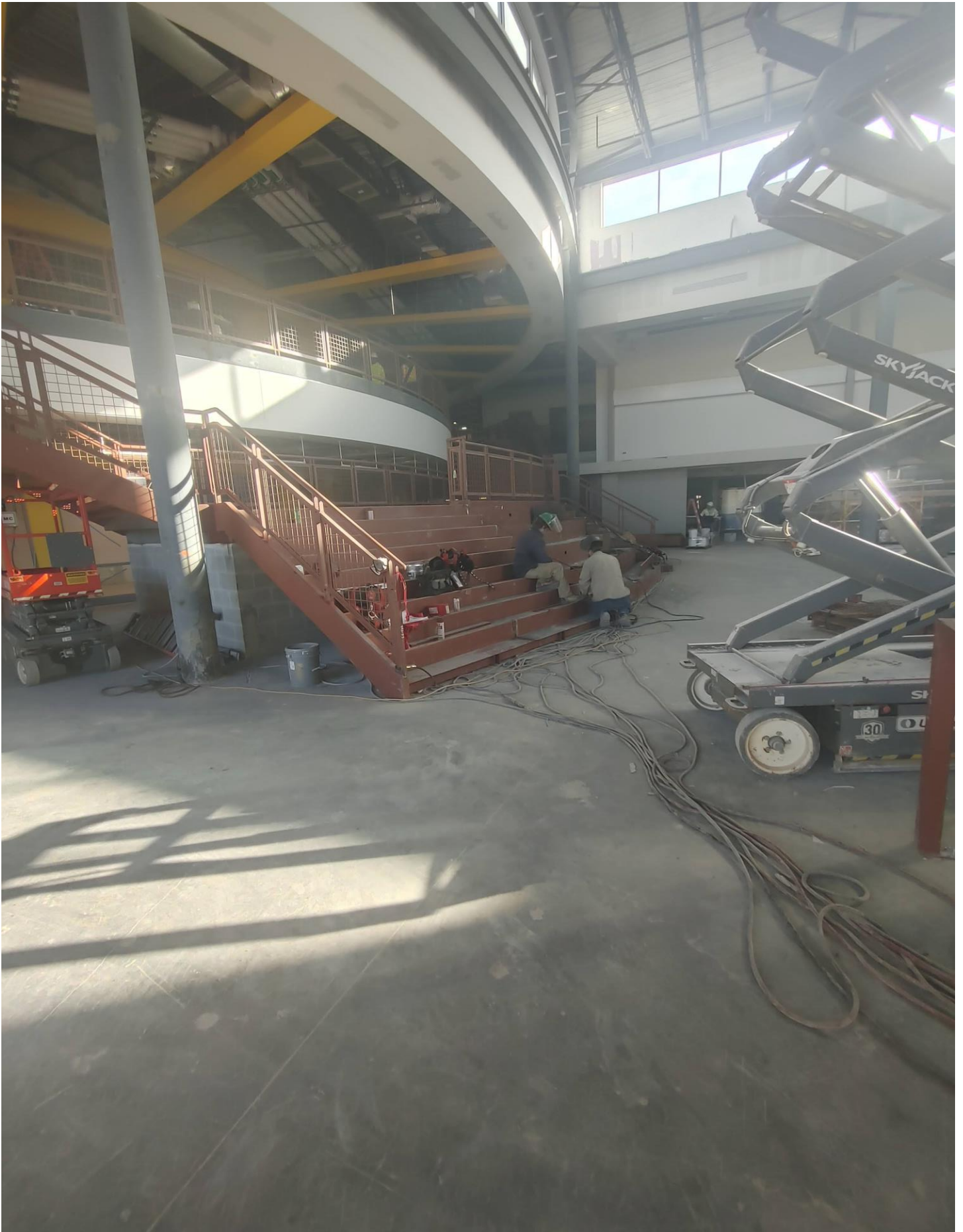
Photo 7 - Work is progressing on the Grand Staircase.
