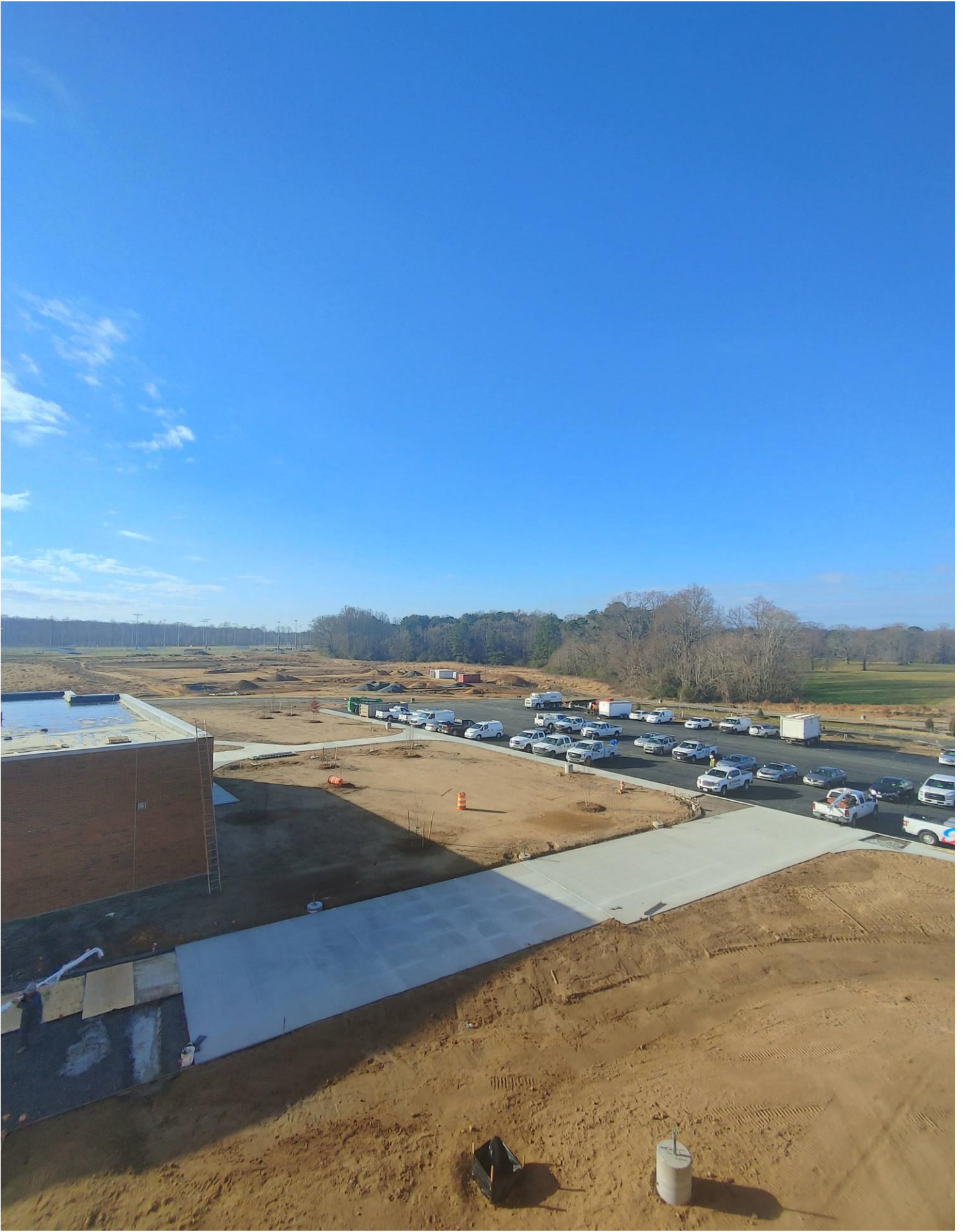
Photo 10 - West side of site
