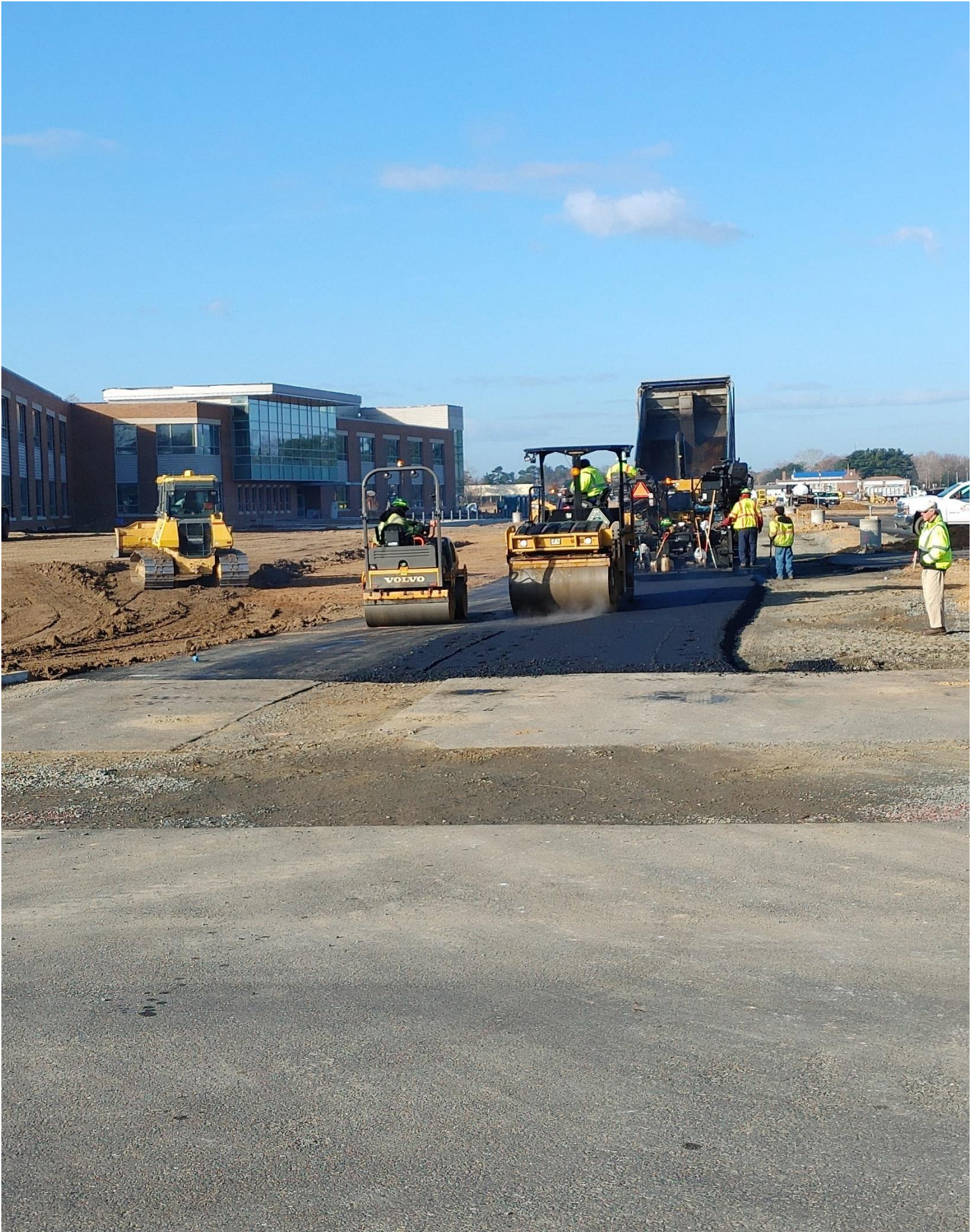
Photo 1 - Base Asphalt is being tied into County Park Drive
