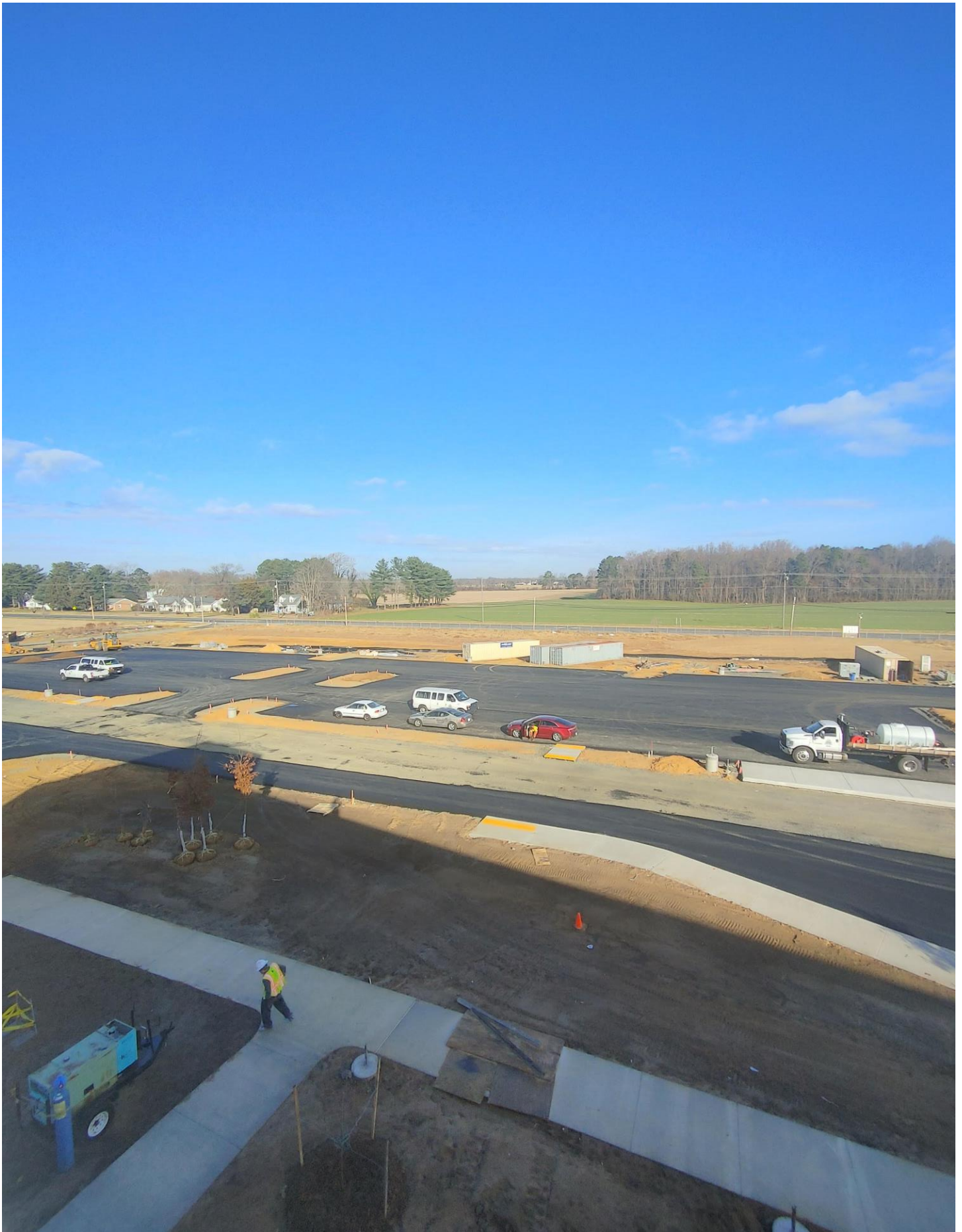
Photo 9 - Northwest Student Parking Lot.
