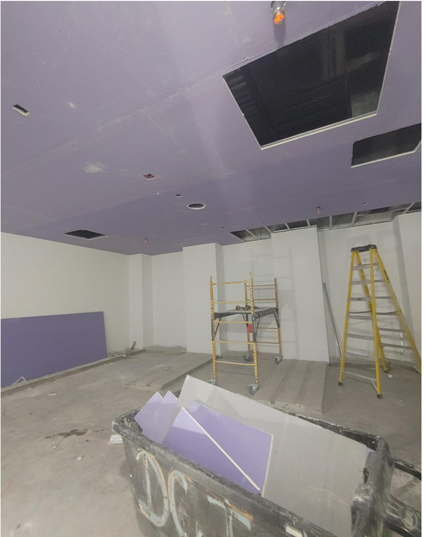
Photo 6 - Ceilings are being hung in locker rooms.
