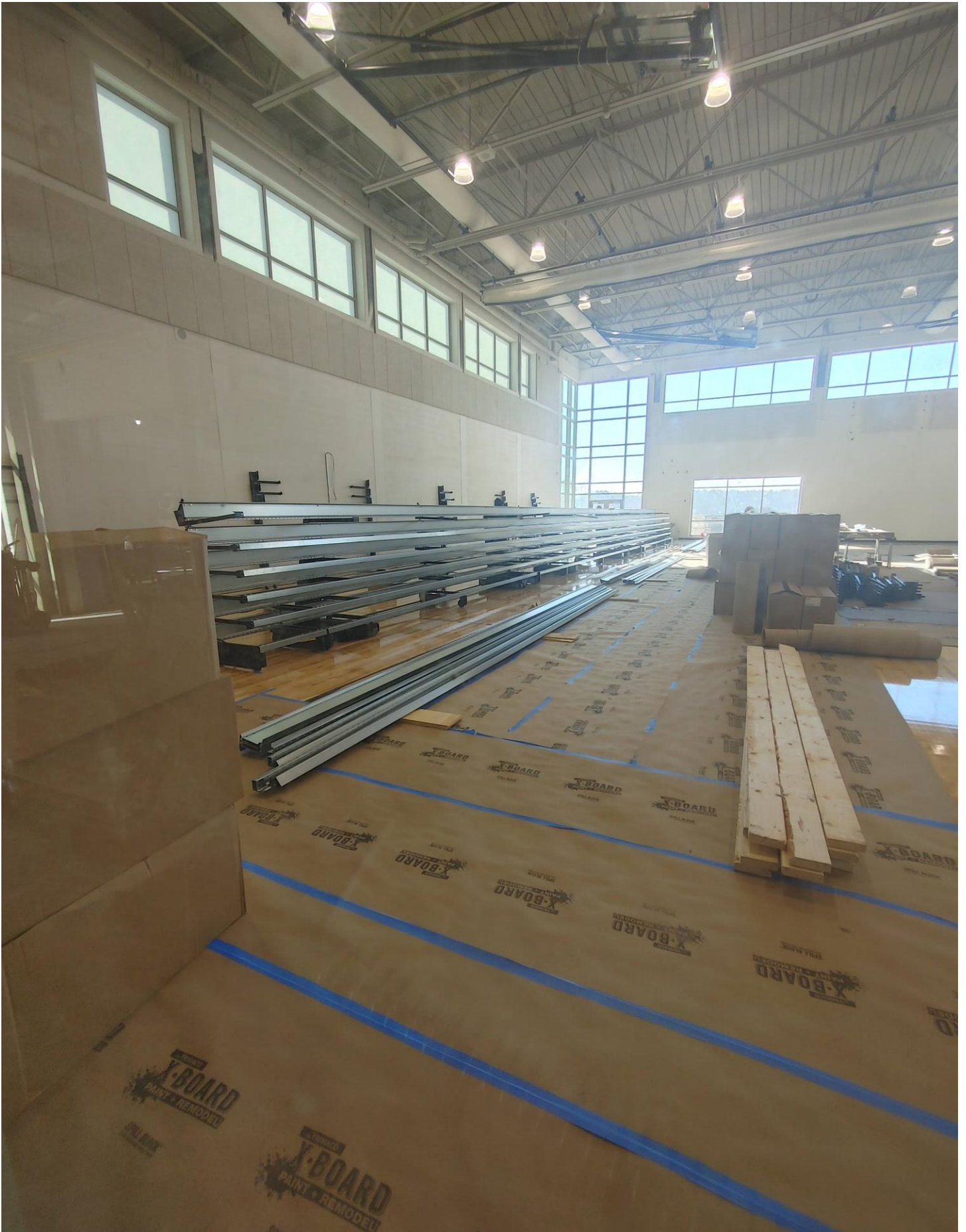
Photo 2 - Bleachers are being erected in the Gym.
