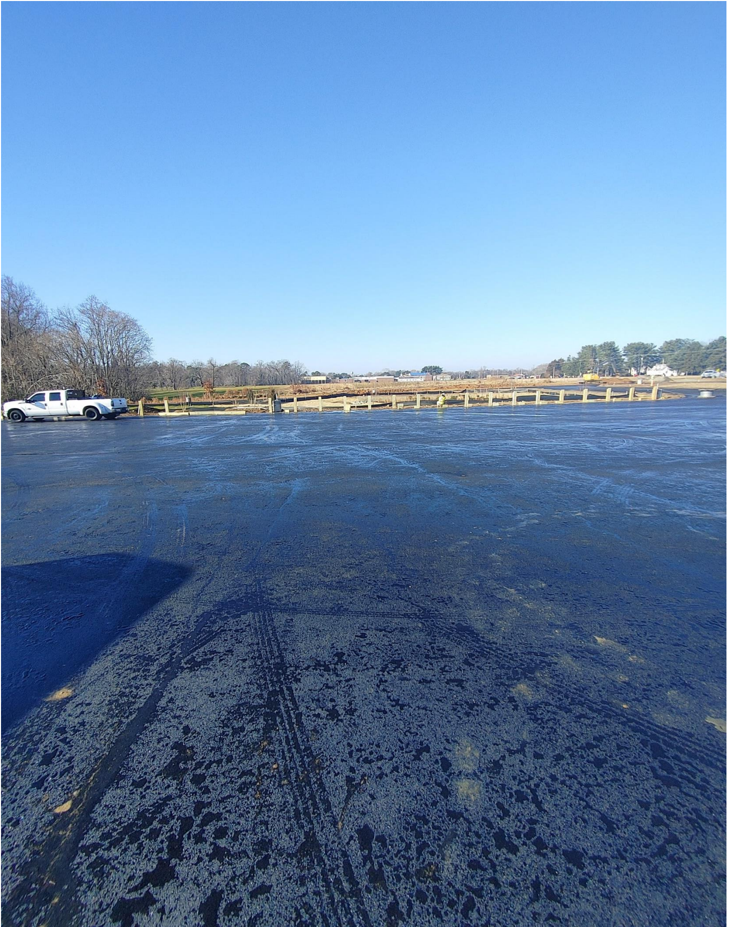
Photo 5 - Fence Posts are being installed
