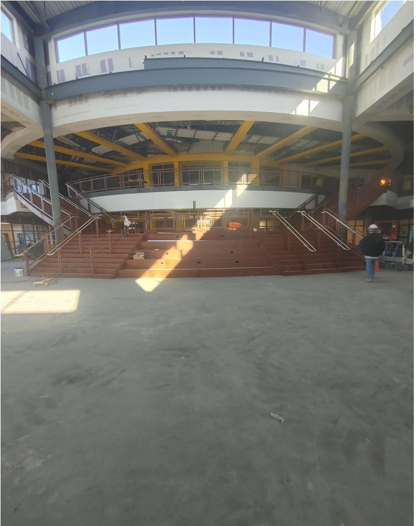
Photo 1 - Work is progressing on the Grand Staircase
