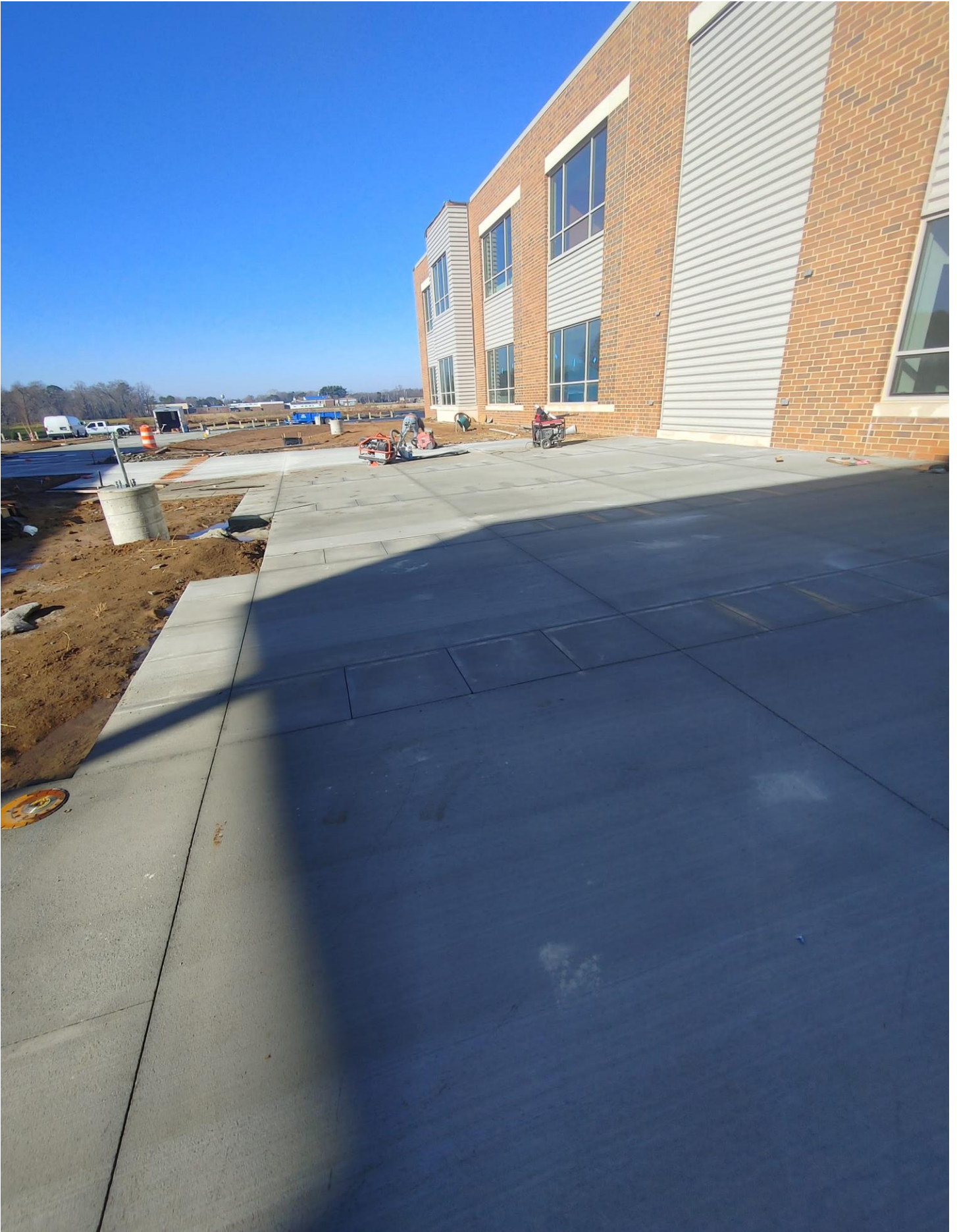
Photo 4 - Concrete is being Scored
