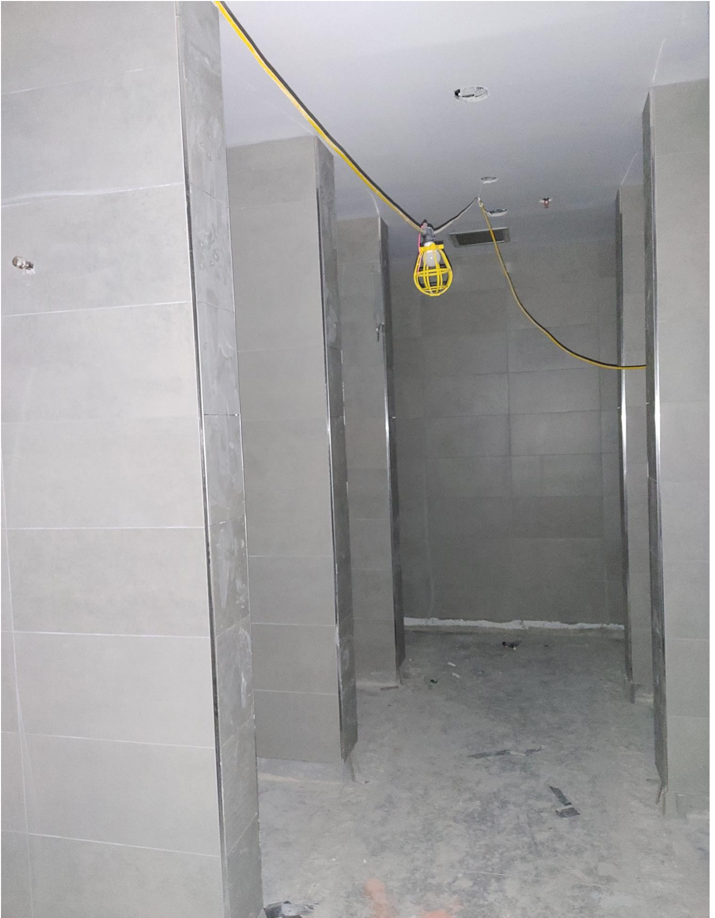
Photo 5 - Wall Tile has been laid in E104 Girls Locker Room
