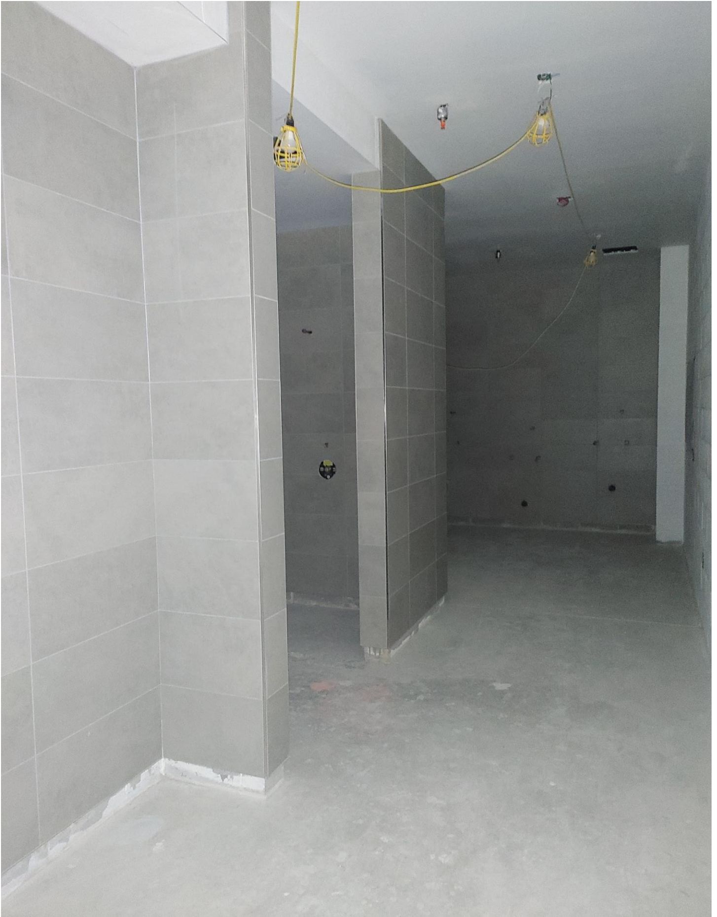
Photo 8 - Wall Tile has been laid in E126 Boy's Locker Room
