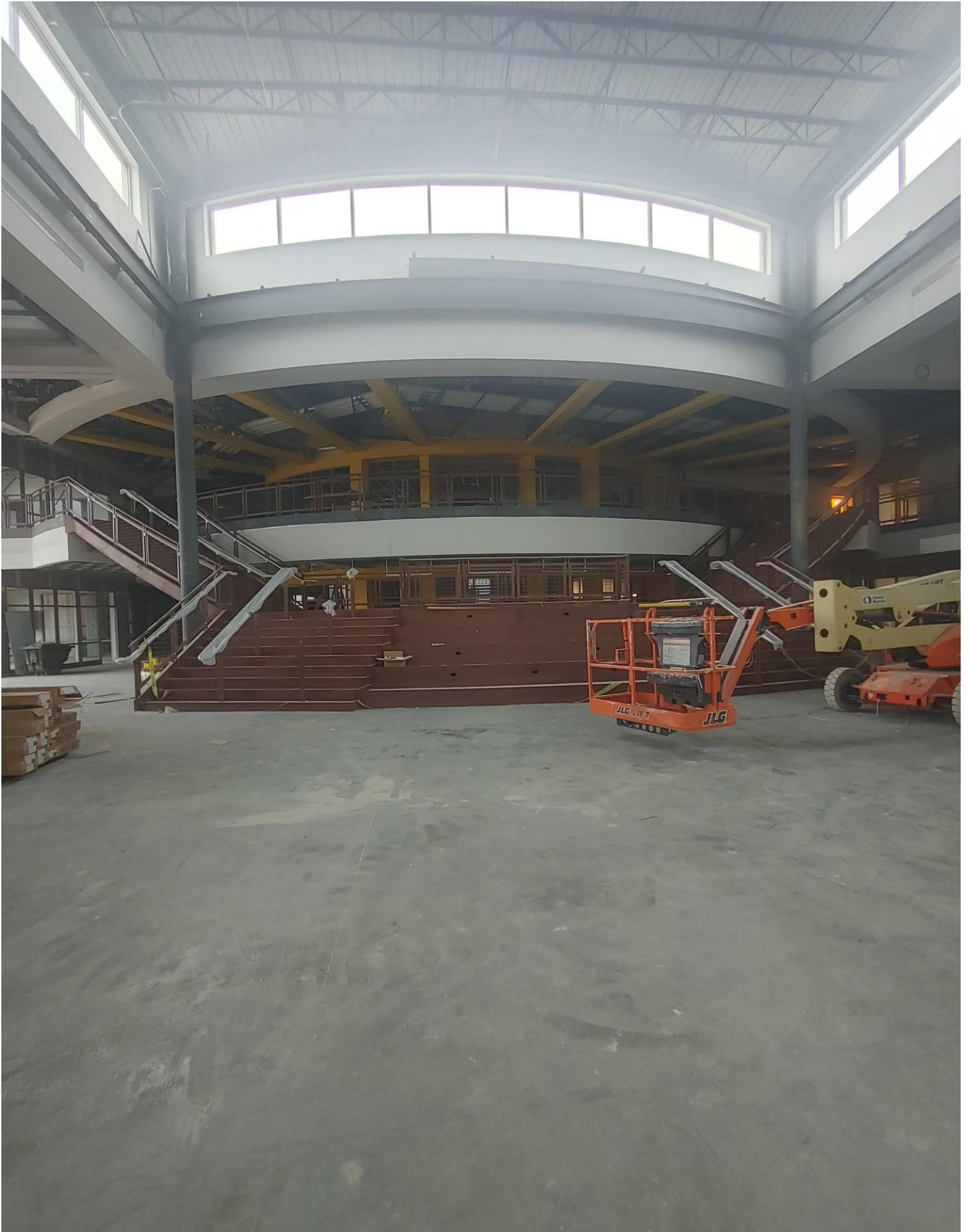
Photo 1 - Work continues on and around the Grand Staircase.
