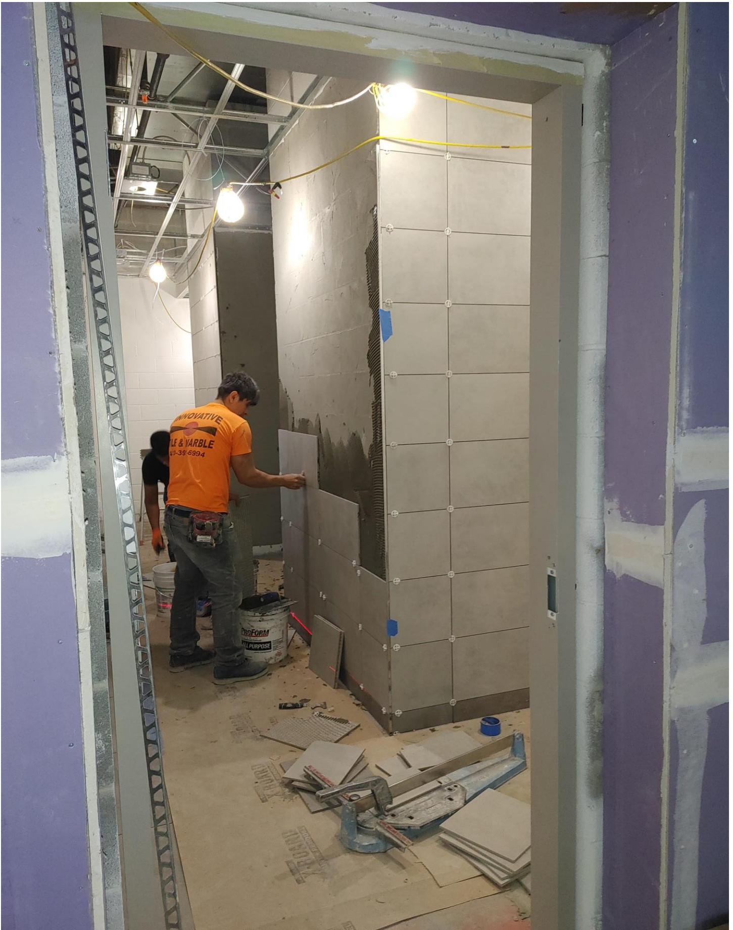
Photo 2 - Tile being laid in the Entryway of E103/E104
