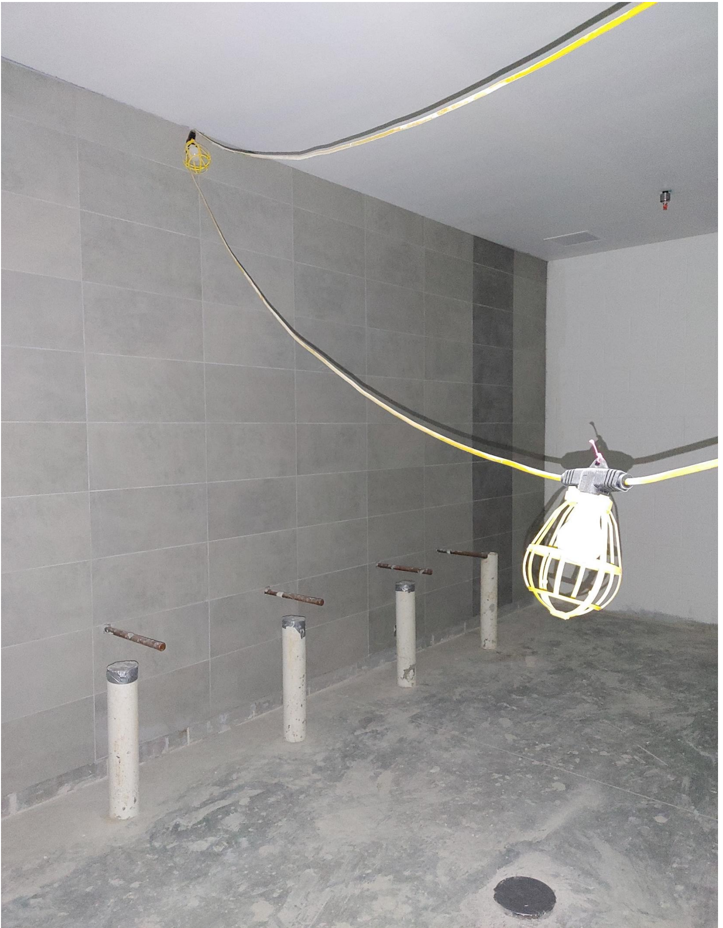
Photo 7 – E124 - Girls Locker Room - Wall Tile has been laid.
