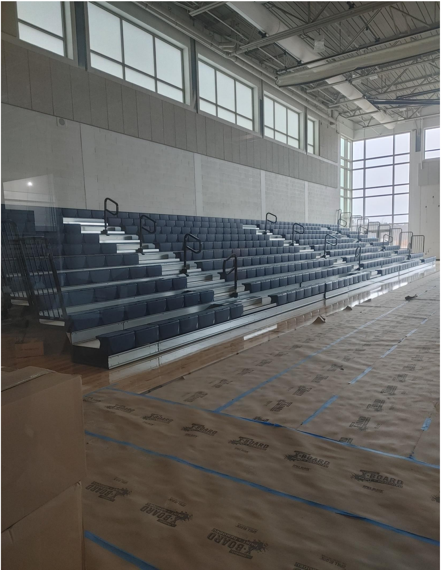
Photo 3 - Bleacher on the East side of Gym have been completed.
