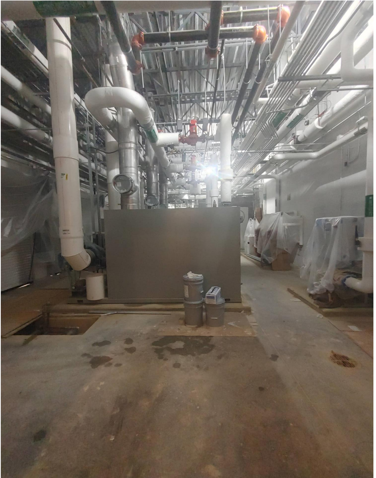
Photo 14 - D154 - Mechanical Room is being painted.
